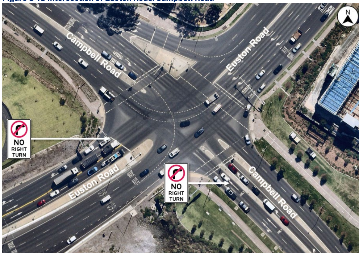
Figure 3-18 Intersection of Euston Road/Campbell Road
