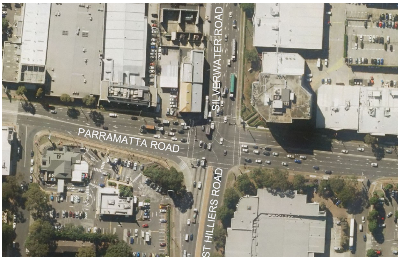
Figure 4-5: Parramatta Road/Silverwater Road intersection
