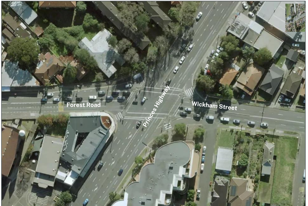
Figure 8: Princes Highway, Wickham Street and Forest Road signalised intersection in 2021
