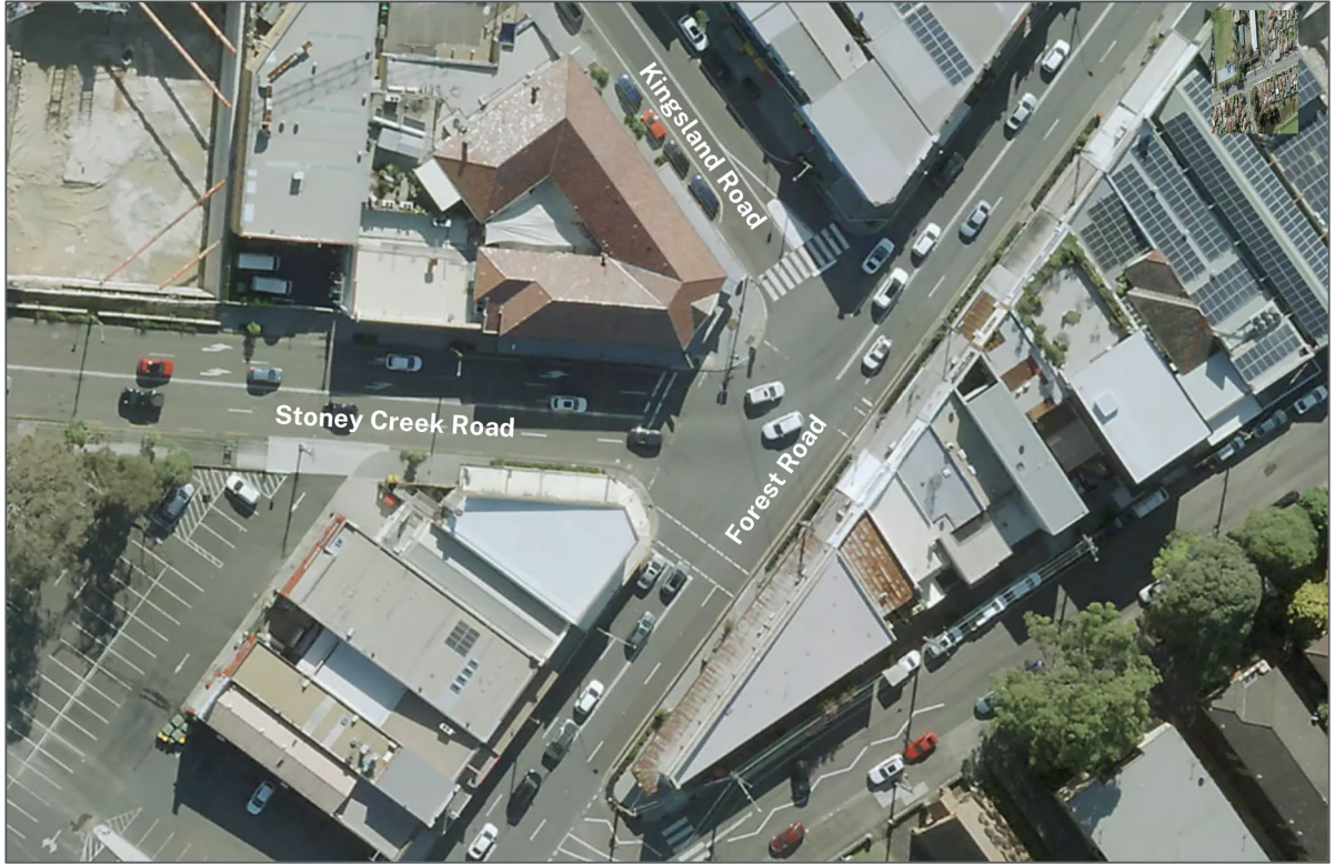
Figure 7: Forest Road, Stoney Creek Road and Kingsland Road signalised intersection (2021)
