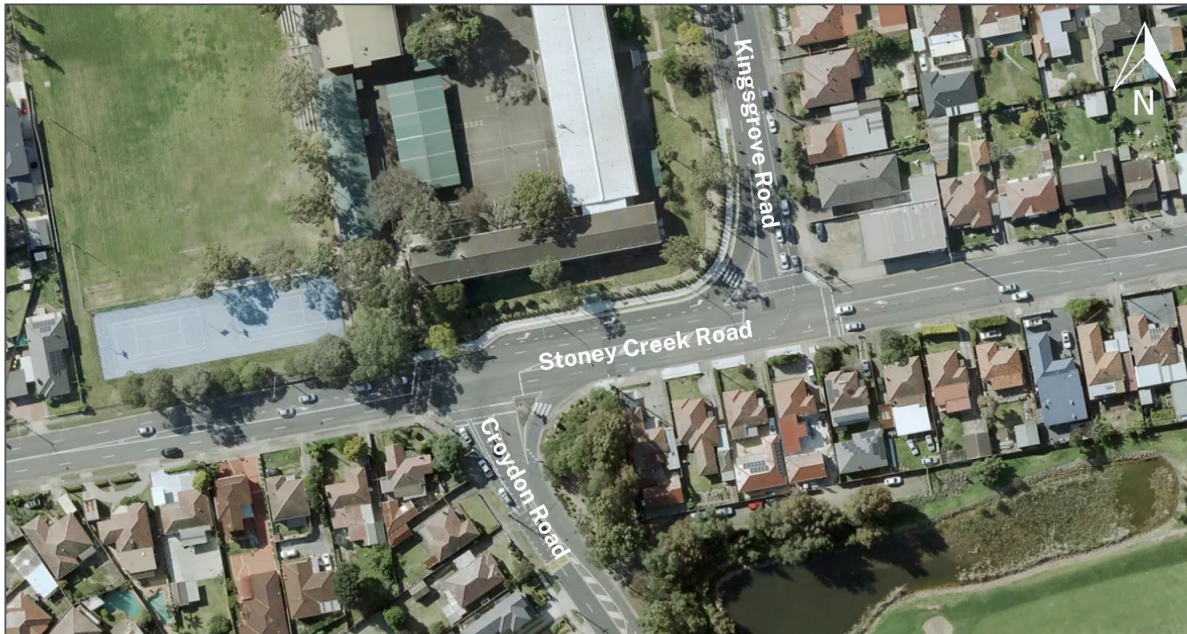
Figure 6: Stoney Creek Road, Croydon Road and Kingsgrove Road signalised intersection (2021)
