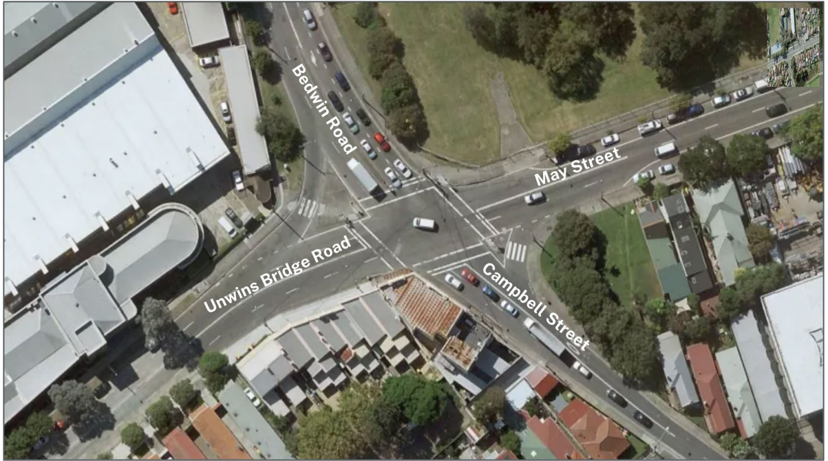
Figure 12: Campbell Street, Bedwin Road, May Street and Unwins Bridge Road signalised intersection pre M8 opening
