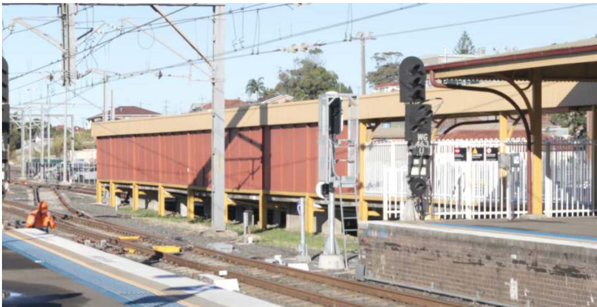
Figure 6-1: Current south west view of southern end of Platform 1 (Jacobs, 2019).
