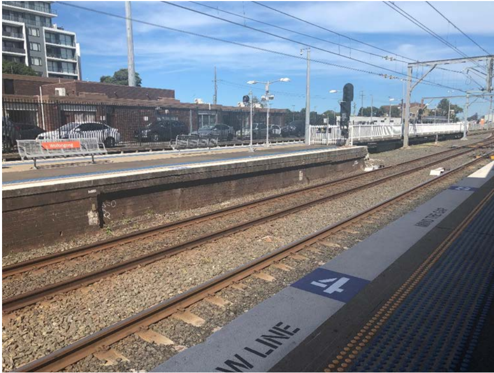
Figure 4-2: The southern end of Platform 2, looking south-east from Platform 1
