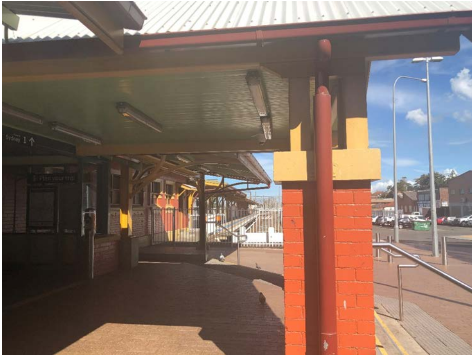
Figure 4-6: Street entrance to Platform 2, looking south. Note dock beyond fence.
