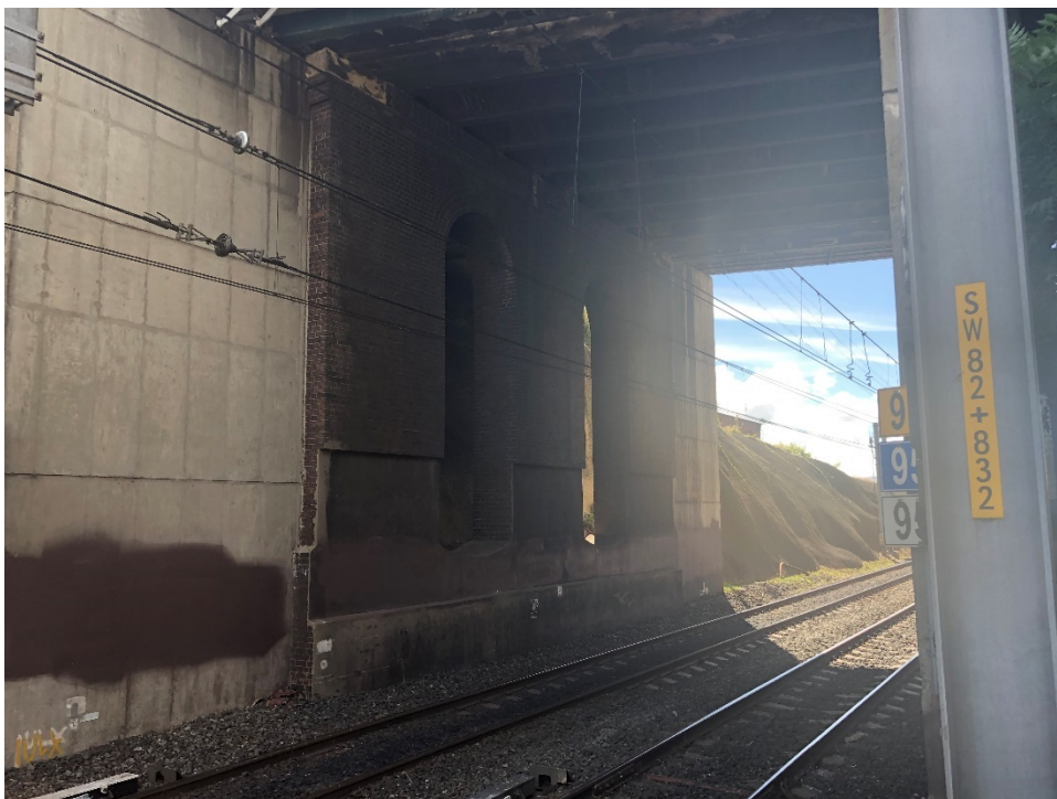
Figure 4-8: Concrete supports flanking brick-arched supports of Crown Street overbridge
