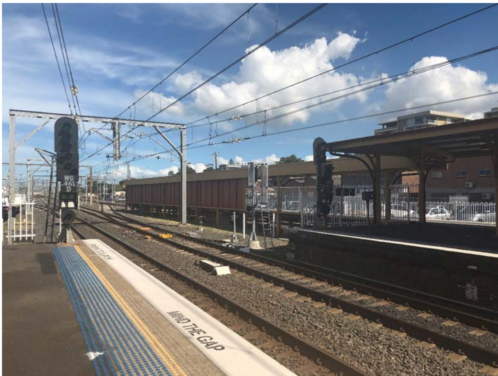
Figure 4-5: Platform extension at Platform 1, looking south-west
