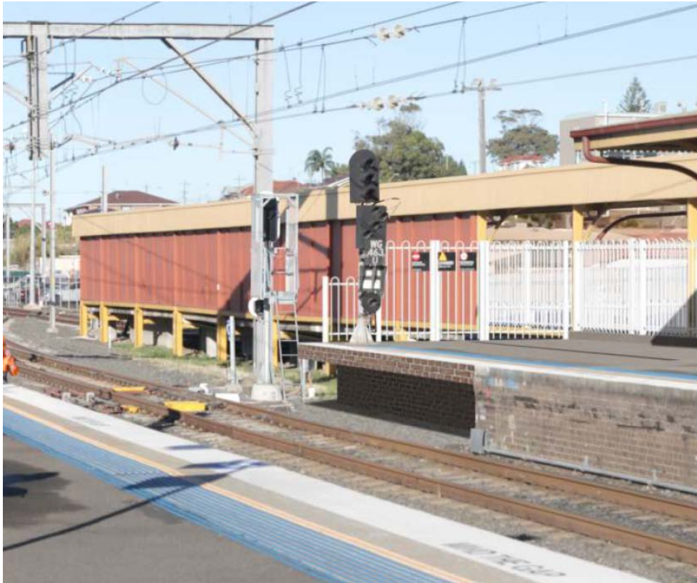
Figure 6-2: Photomontage showing indicative view of the southern platform extension of Platform 1 (Jacobs, 2019).
