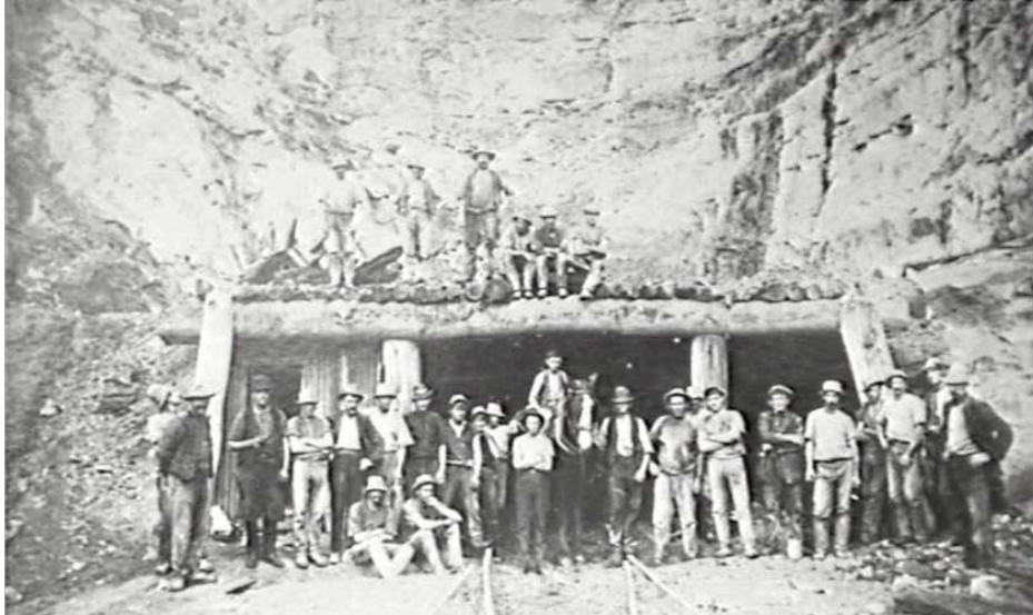
Figure 3-2: Construction of the railway line at Helensburgh, c1880
