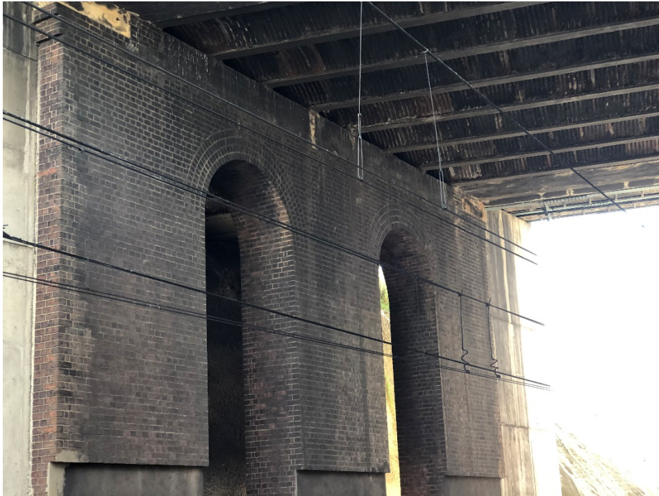
Figure 4-7: Brick-arched supports of Crown Street overbridge, looking north-west
