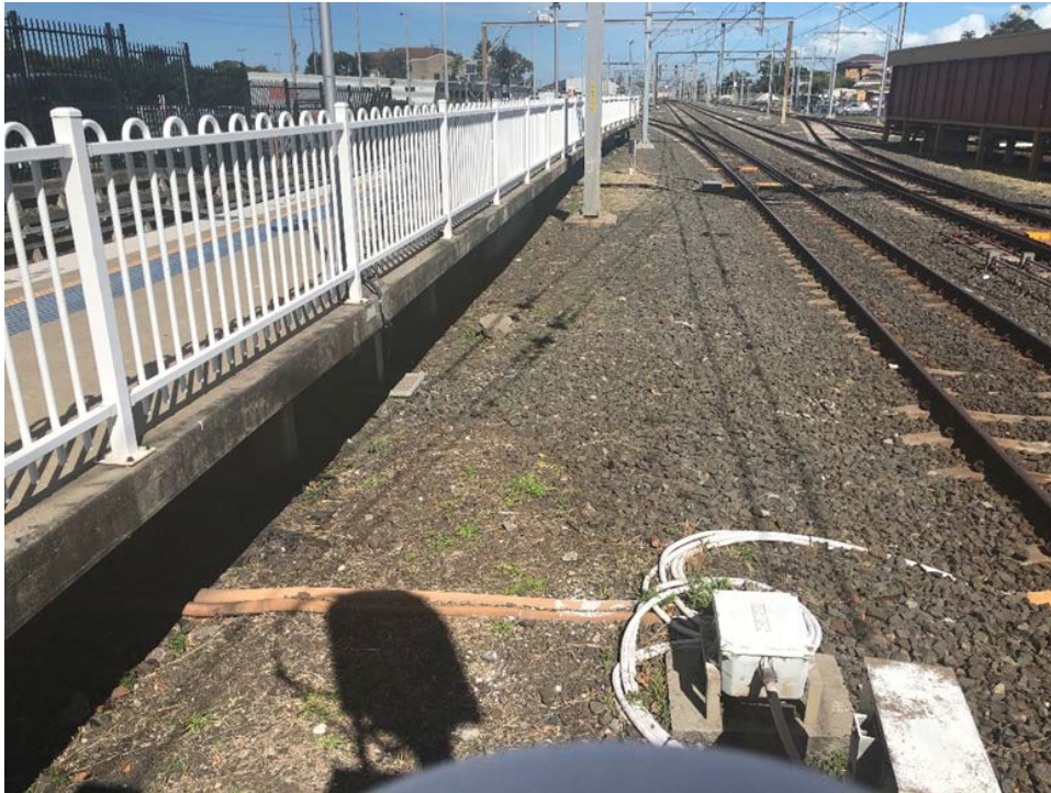
Figure 4-4: Platform extension on Platform 2 (at left of frame), looking south
