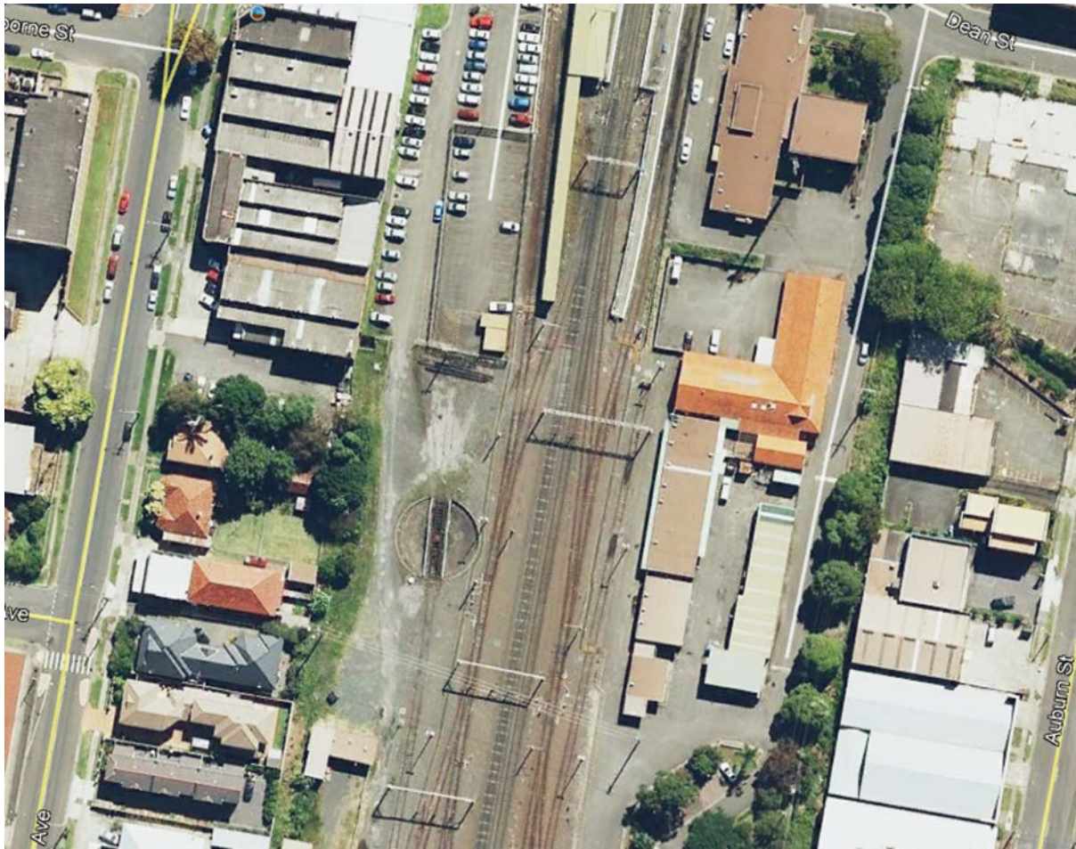
Figure 3-7: Detail of aerial image depicting turntable at Wollongong Railway Station, 2008
