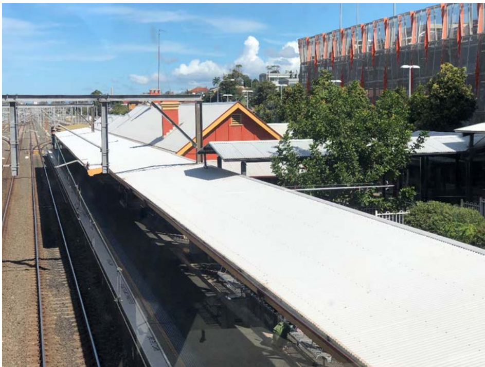
Figure 4-9: Canopies on Platform 1 installed in 2005, looking south from footbridge
