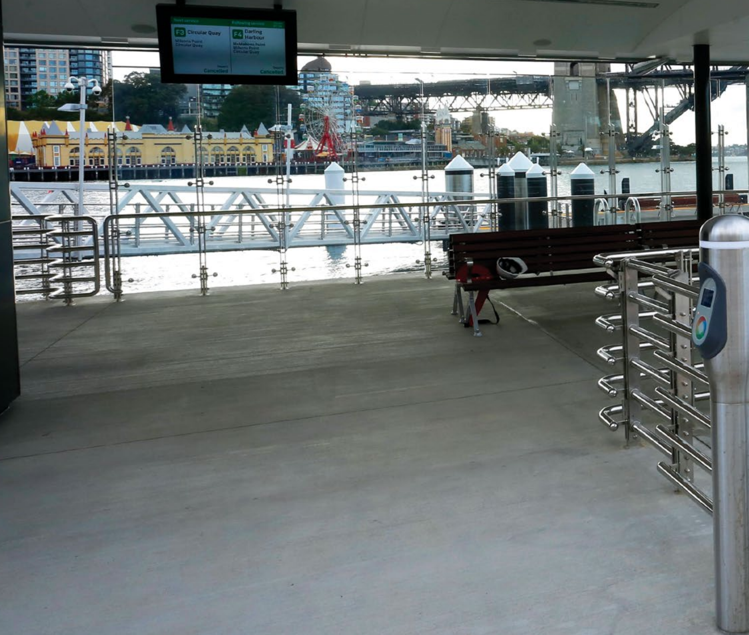
Newly upgraded McMahon's Point Wharf on Sydney Harbour opened in October 2016 as part of the Transport Access Program.
