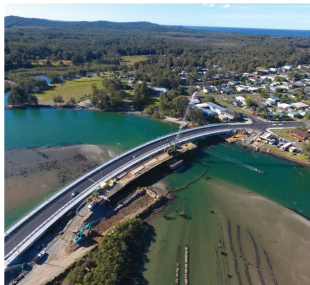
The new Stingray Creek Bridge at North Haven.
