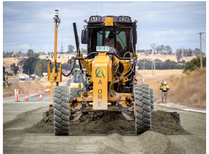
Road grader levelling out the base for the new road.
