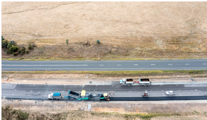
The new northbound lanes are continuing to take shape.
