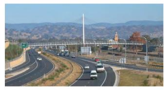
The approach from the north with the Dean Street cable-stay pedestrian bridge and old railway station and yards in view. The terraced retaining walls and noise walls align with the town grid and complement the station.
