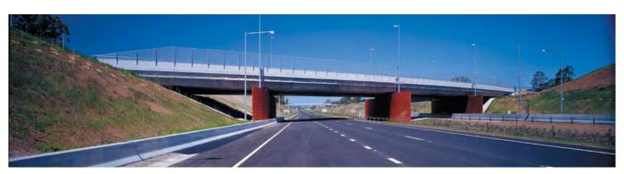
All vehicular bridges have similar properties in terms of coordinated lighting locations, spill-through abutments, tapered safety screens and night lighting. Names of overbridges are neatly integrated with principal designs.
