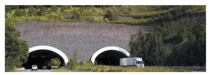
The Cudgen Road tunnel allows the wooded ridge line and wildlife corridor to cross the road and extend down to the edge of the Tweed River. Native planting and seeding is provided to revegetate the edges of the portal. Use of gabion facing is suitable for the natural context.
