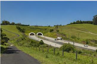
The white tunnel portal collars contrast and highlight the landscape and landform around. They divert storm water and provide a maintenance safety parapet. The landform wrapped around the portals and laid back to natural grades is a long term safe earthworks solution which avoids walls, their maintenance and graffiti.
