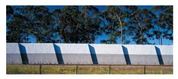
Precast concrete noise walls are designed to serve different purposes and suit different locations. These panels, at a location close to the road, are repetitive and easy to replace. Overpainting is carried out in the event of graffiti vandalism.
