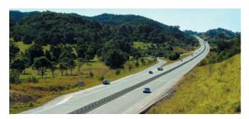
Yelgun to Chinderah: Avoiding cutting through spurs and aiming for saddles and valleys reduces earthworks and creates a more flowing, responsive alignment.
