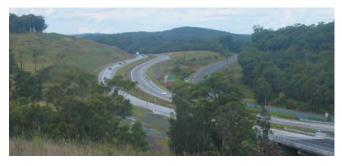
Karuah to Bulahdelah: Rounding off and grading out the slopes to 1:4 create an almost seamless integration with the natural slopes.
