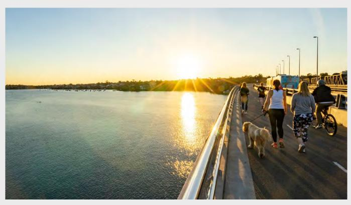
The 4.5m wide shared path provides a fitting continuation of the Bay Run largely superseding the narrow walkway kept on the eastern side of the bridge. The railings are designed to allow views of the bay and a concrete edge to the path naturally provides a strip for walkers to stand and take in the view.
