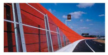
Clear walls always overlap solid walls and primary colours are used to emphasise different character zones along the M7 Motorway. Experience is showing that laminated and toughened glass would be best substituted by transparent plastic products in future.
