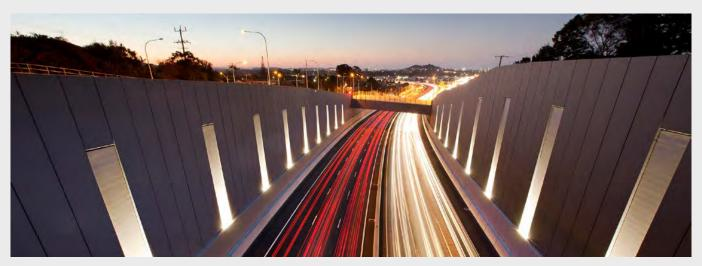
The Banora Point cutting from the land-bridge looking north to the Gold Coast. The retaining walls extend beyond the original surrounding ground plane to neatly provide the noise walls. Lighting is integrated into the walls to break down their expanse and create a night-time effect.
