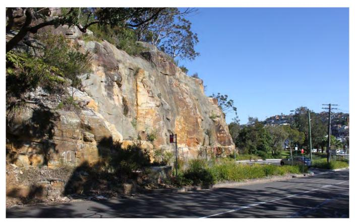
A combination of stable rock with a textured shotcrete applied in minimal areas to stabilise the cutting and provide structural support (The Spit, Sydney)
