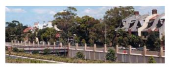
The depressed motorway is hidden from the houses and park. Its retaining walls minimise its footprint and are designed to complement the form of the Victorian terraced houses of Surry Hills.
