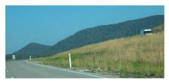
Karuah Bypass: Independently grading the carriageways helps minimise earthworks, provides a more interesting journey and reduces the wide terraced effect of roads on hillsides. Note the gentle gradient of the embankment.
