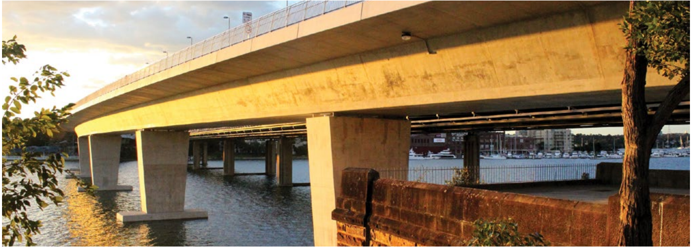
The piers on the new Iron Cove Bridge, seen here at sunset, are parallel in the short elevation and tapered in the long elevation. This taper also follows the direction of angle of the girder edge which helps unify the bridge elements.
