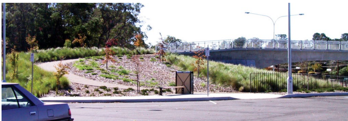
Earthworks have been utilised to cost effectively create the landscaped ramp to the bridge at Falconbridge over the Great Western Highway.
