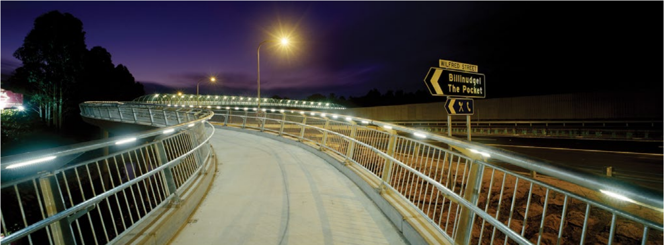
LED lighting in the handrail combined with overhead lighting on the road crossing creates an interesting low maintenance effect on the pedestrian bridge at Billinudgel.
