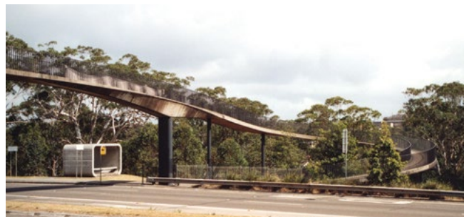
The simple spiral connection of the ramp adds to the value of the bridge. However, adequate space is required for this solution. Also the presence of landings needs to be considered.
