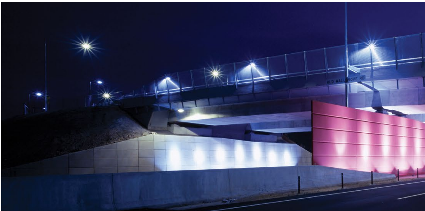
Lighting is used at select locations on the M7 to highlight features such as wing walls, noise walls and overbridges.
