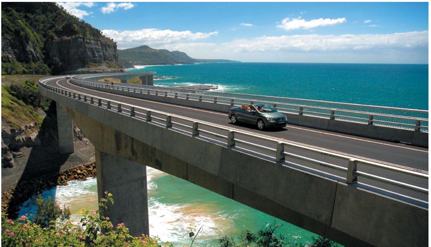
The sweeping form of the Sea Cliff Bridge, north of Wollongong, with two-rail parapet provides panoramic views.
