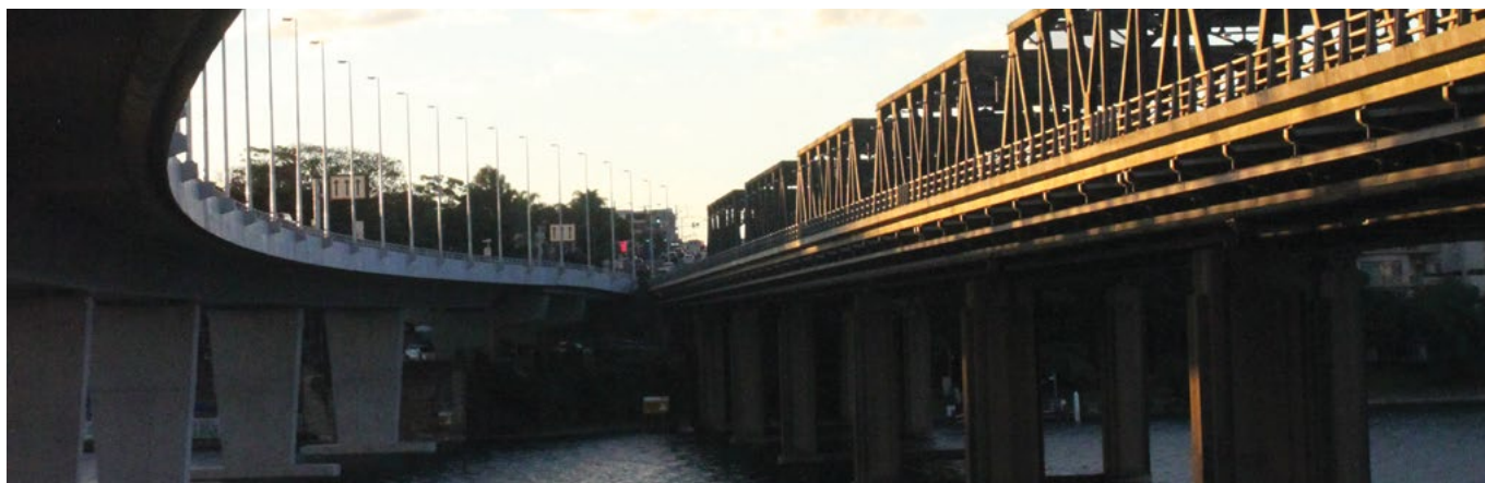
The new Iron Cove Bridge on the left was designed on a simple curvature and simple refined piers and girder, so that it did not conflict with the more complex truss forms on the old Iron Cove Bridge.
