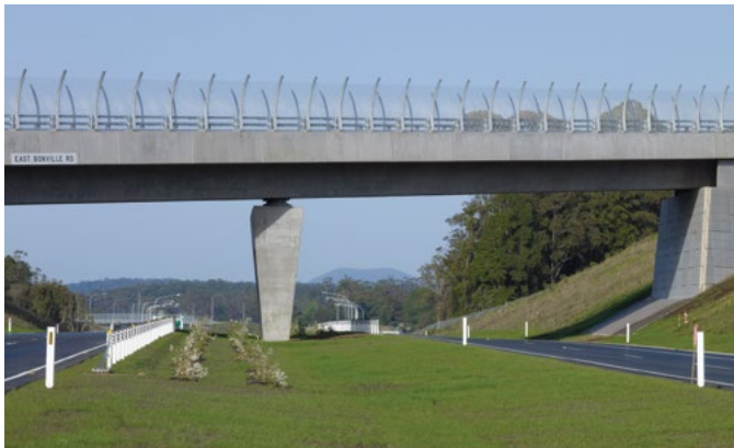
When designing a suite of bridges for a project, for example on the Bonville Upgrade on the Pacific Highway, tapering the piers on the family of overbridges will create different shaped piers if the bridges have different heights. This is because the top and bottom dimensions of the piers are constant. This is not a significant visual problem if the bridge heights are similar. Care should be taken on inverted shaped piers to avoid the effect of a spindly base appearing to support a large load.
