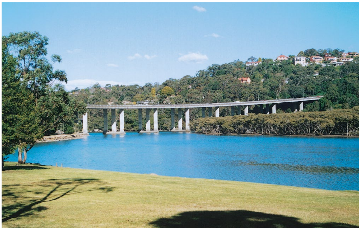
The simple elegance of the bridge over Middle Harbour at Roseville complements the landscape of the National Park.
