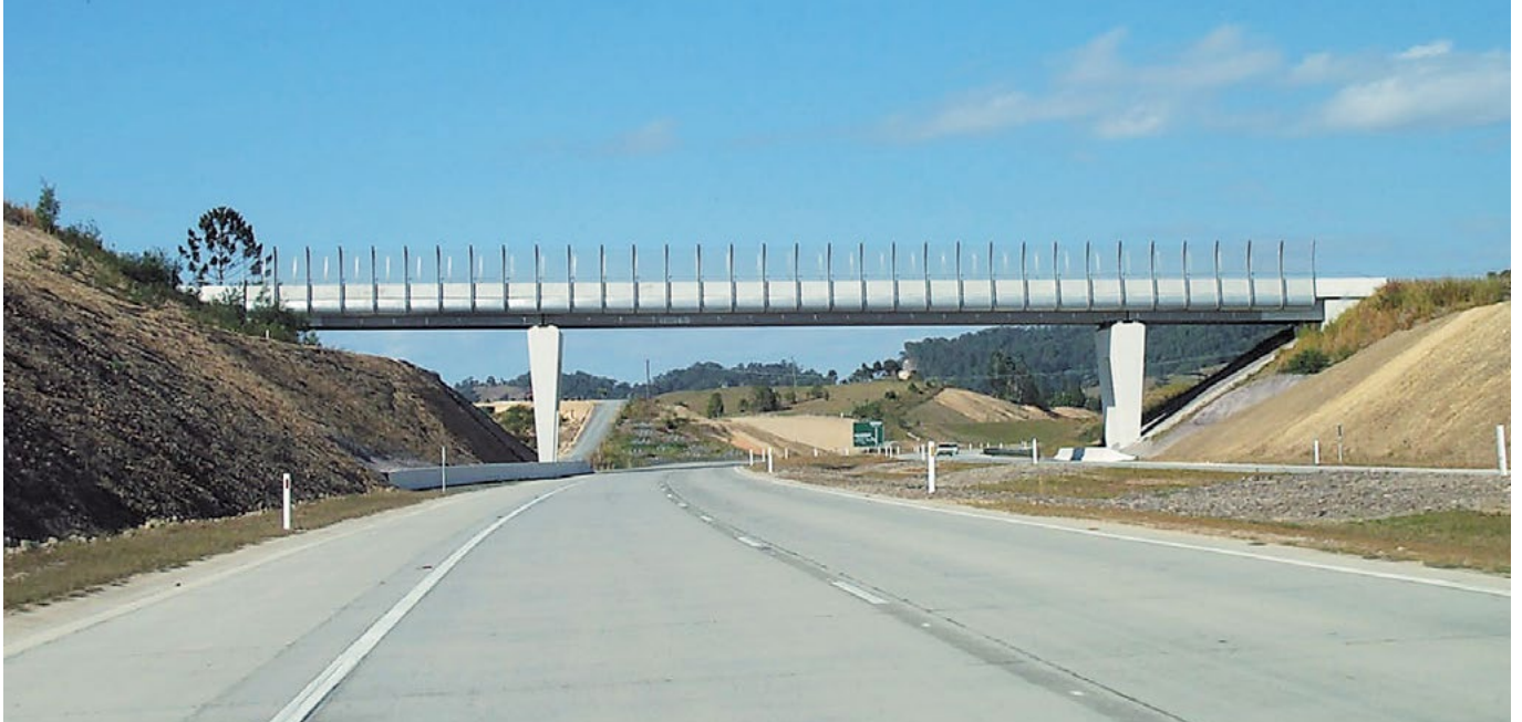
The outer spans of this local road bridge on the Yelgun to Chinderah upgrade of the Pacific Highway are not the same dimension and this affects the symmetry of the bridge.
