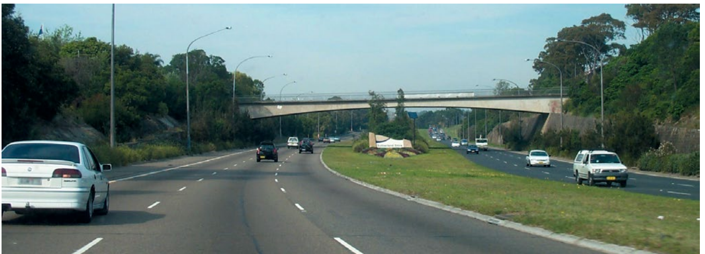
On this bridge over Taren Point Road it is unfortunate that the planting design is not integrated with the bridge design, as it obscures the fact that the bridge is an elegant single-arched span.
