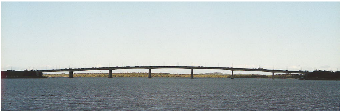
Captain Cook Bridge over the Georges River has a ratio of 1:18 and together with its gentle vertical curve has a very slender appearance.
