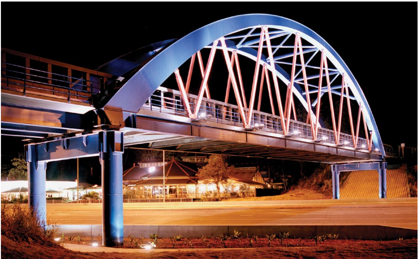
The rail bridge at Coffs Harbour over the Pacific Highway serves as a marker through Coffs Harbour and provides a feature for the town. Its illumination highlights the arched form of the bridge and its critical structural elements to make a night time composition. This is all further enhanced by the strong use of colour on the bridge (see Section 6.1).
