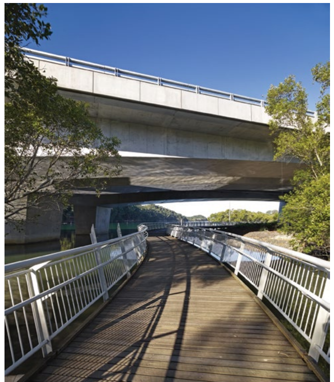
The space under the triple bridge over Brunswick River has a unique character. The public timber boardwalk traverses an area of relocated mangroves, preserved sea grasses and rocky outcrops with framed views towards the ocean and surrounding mountains. Watery reflections on the immense haunched girders overhead provide a fitting ceiling to the space.
