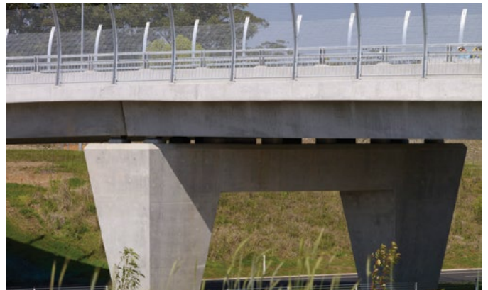
When designing a suite of bridges for a project, for example on the Bonville Upgrade on the Pacific Highway, tapering the piers on the family of overbridges will create different shaped piers if the bridges have different heights. This is because the top and bottom dimensions of the piers are constant. This is not a significant visual problem if the bridge heights are similar. Care should be taken on inverted shaped piers to avoid the effect of a spindly base appearing to support a large load.
