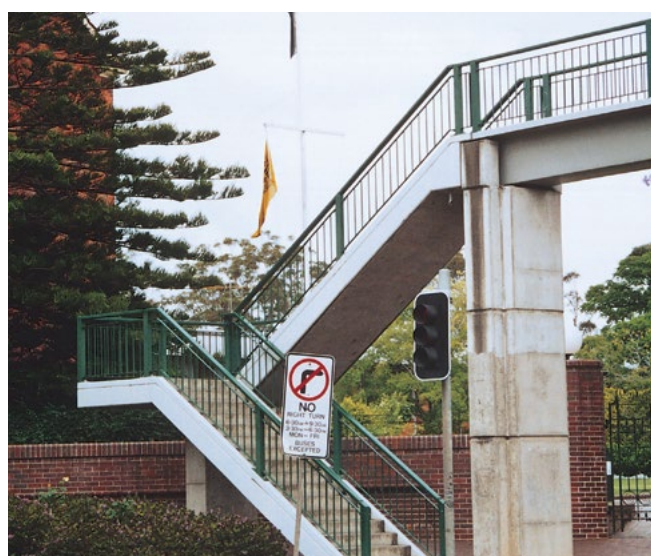
Where space is limited, stairs should be simple and compact as on this bridge over the Pacific Highway on Sydney's North Shore. Note the neat detail of the connection between superstructure and ramp marred only by staining.
