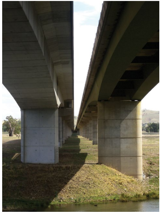
The duplication of the Hume Highway Sheahans Bridge at Gundagai (left) adopted the existing haunch shape and pier spacings. The materials and details are however different styles but there is a design unity.
