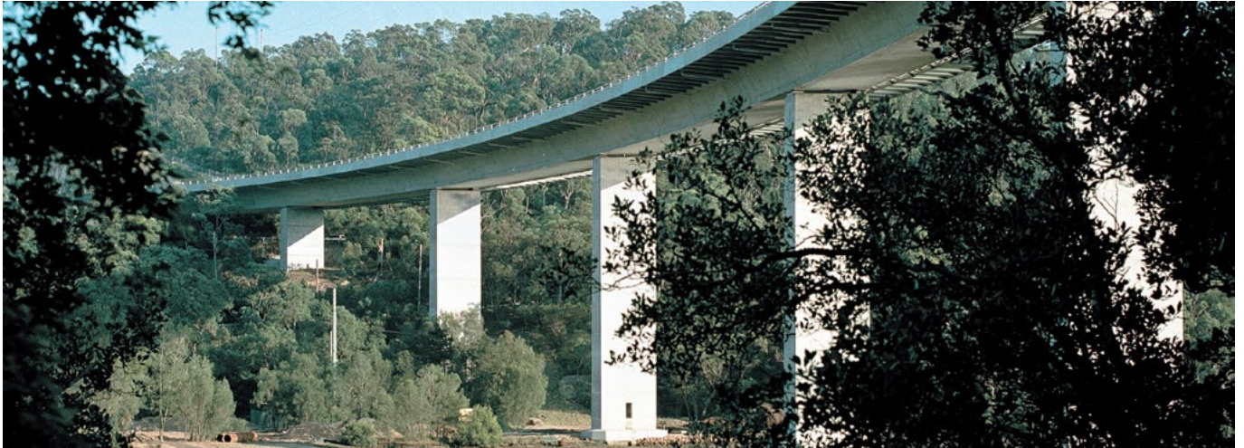
The line of the parapet on the bridge over Woronora River at Sutherland is an important bridge element. It is sharp, smooth, catches the light, helps provide shadow and unifies the structure.
