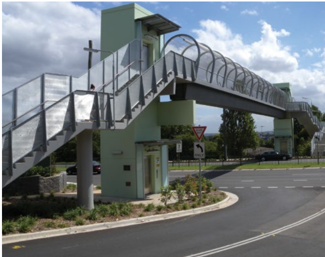
The form and fencing, colours and use of the lift shaft as a pier are visually strong but the bulky pier support detracts from this bridge over Silverwater Road.
