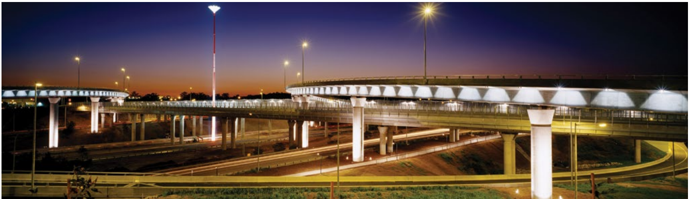
Lighting is used in various ways on the M7 Motorway and M4 Interchange to highlight the columns, ramps and mark the interchange as a whole. This is an entire composition in lighting which makes the interchange visible, safe and beautiful.
