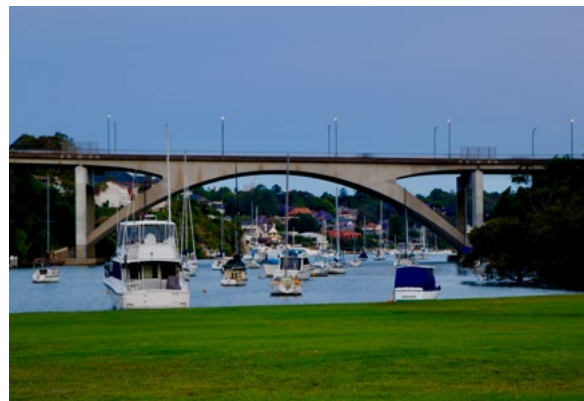
The Tarban Creek Bridge required strengthening of the arches. An innovative solution was required to take the weight of the end spans beyond the arches. A refined portal frame pier, protruding from the bridge envelope, created a separate structure distinguishable from the original bridge.
