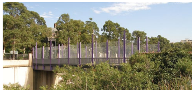
Each of the retro-fitted safety screens on the Eastern Distributor pedestrian bridges has a different distinguishing colour, but they all form part of an integrated approach and colour composition for the corridor.
