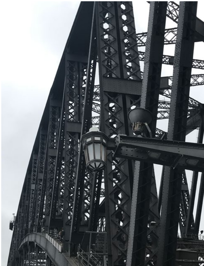
The original lamps of the Sydney Harbour Bridge have been rebuilt using bronze and glass, as well as new LED technology.
