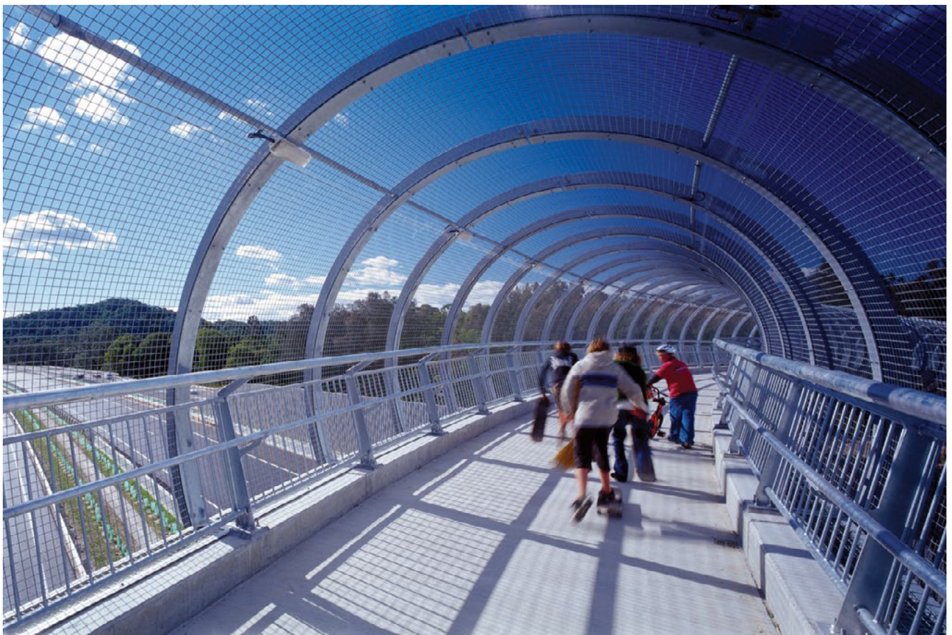
The bridge over the Pacific Highway at Billinudgel has an open feel even through it is caged. It is suited to the bridge and is well designed.
