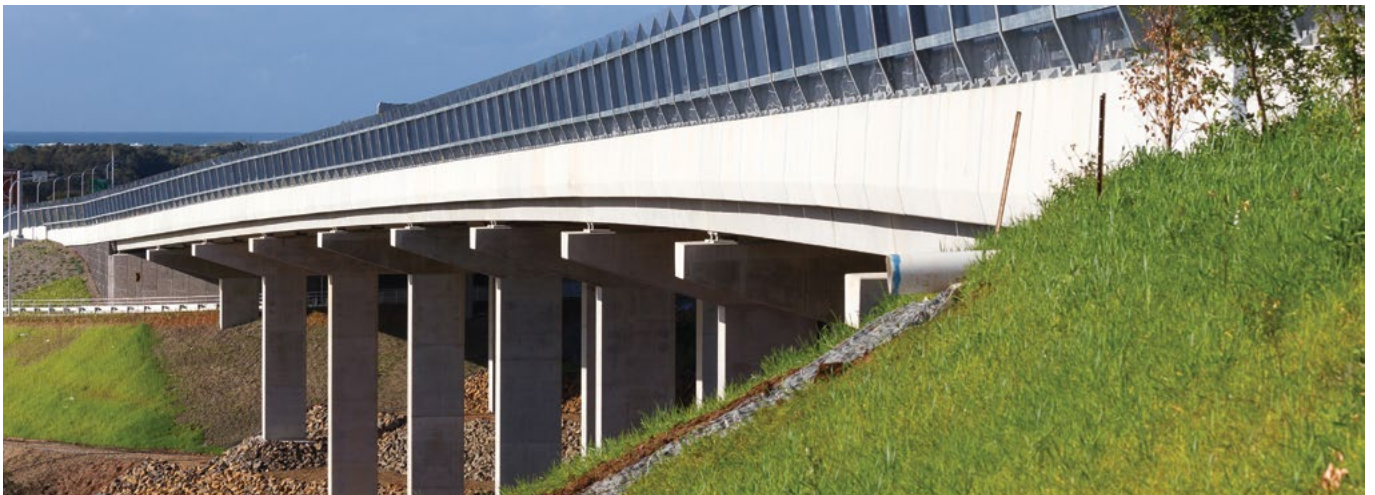
In some circumstances where the parapet is proportionally too deep, a crease line or kink can help visually break down the apparent depth as on this Pacific Highway bridge at Banora Point. The parapet is on a continuous curve to avoid the faceted appearance of the Super T girders.
