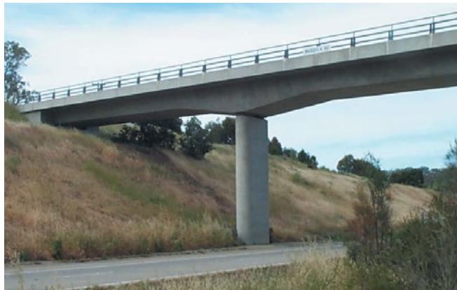
Clean, well designed rounded ends on the piers on this bridge over the Hume Highway complement the bridge and rural setting.
