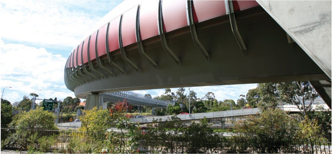
The girder colour on this pedestrian bridge over the Warringah Freeway is standard RTA bridge grey, while the privacy screens use a burgundy coloured perspex sheet in order to create a distinctive opaque visual effect.
