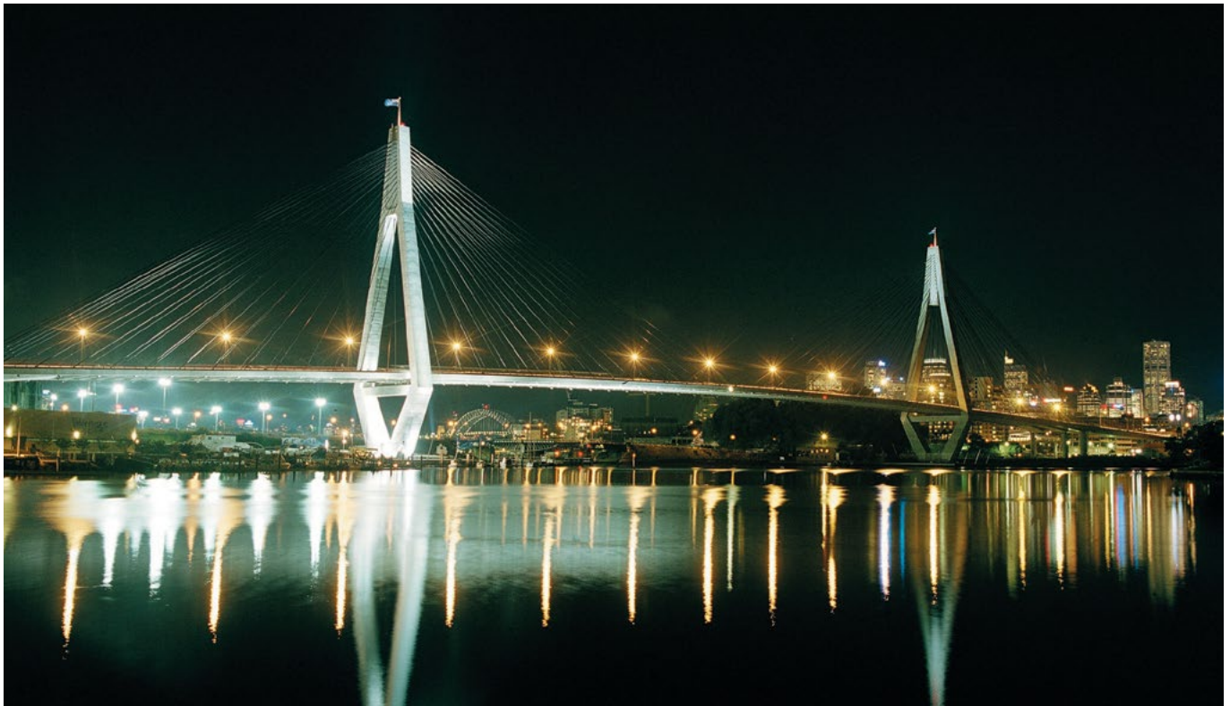
The Anzac Bridge in Sydney as seen in this night time view across Blackwattle Bay.
