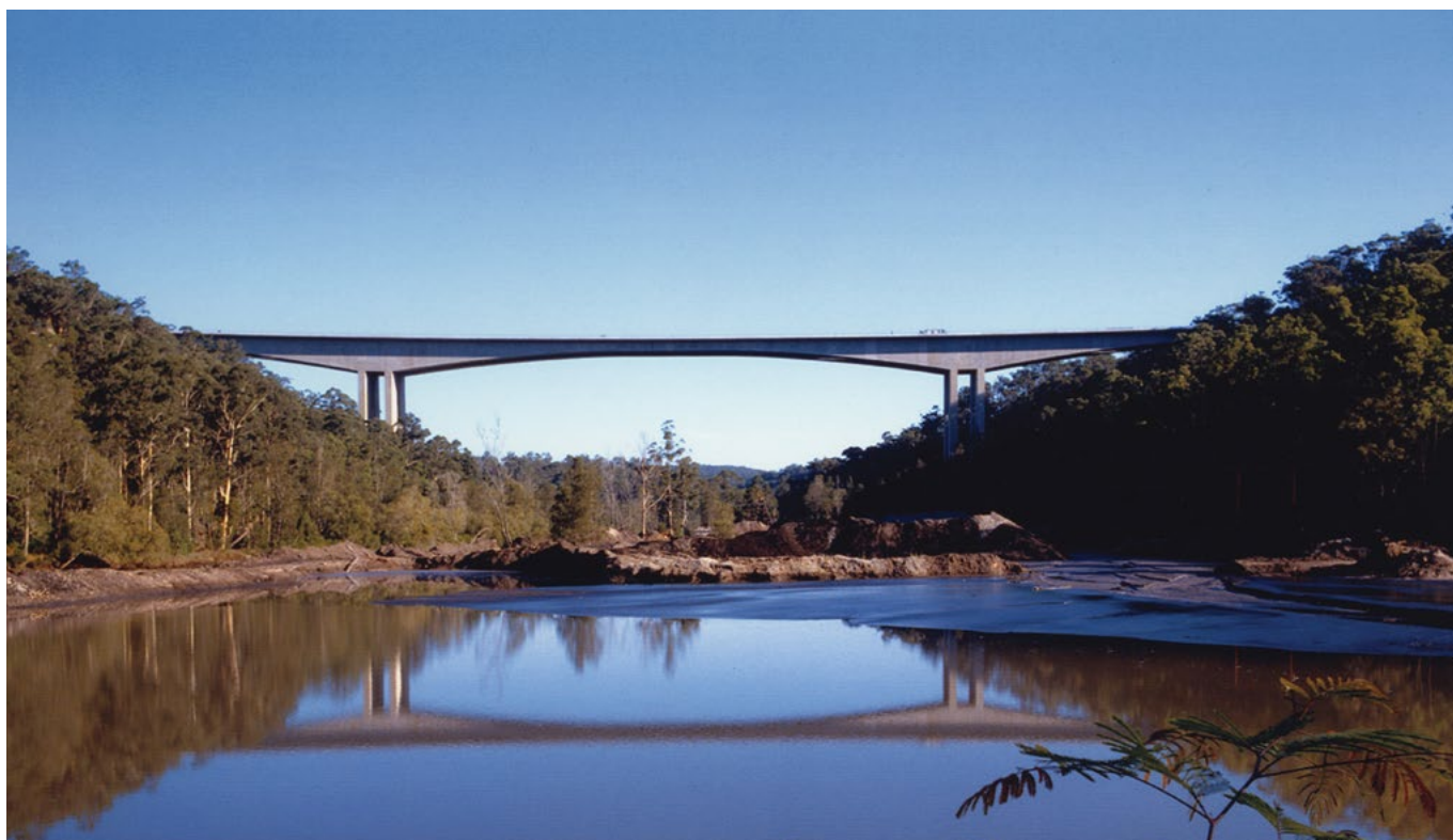
The F3 Freeway twin bridges over Mooney Mooney Creek demonstrate how good engineering design and good aesthetics are synonymous.
