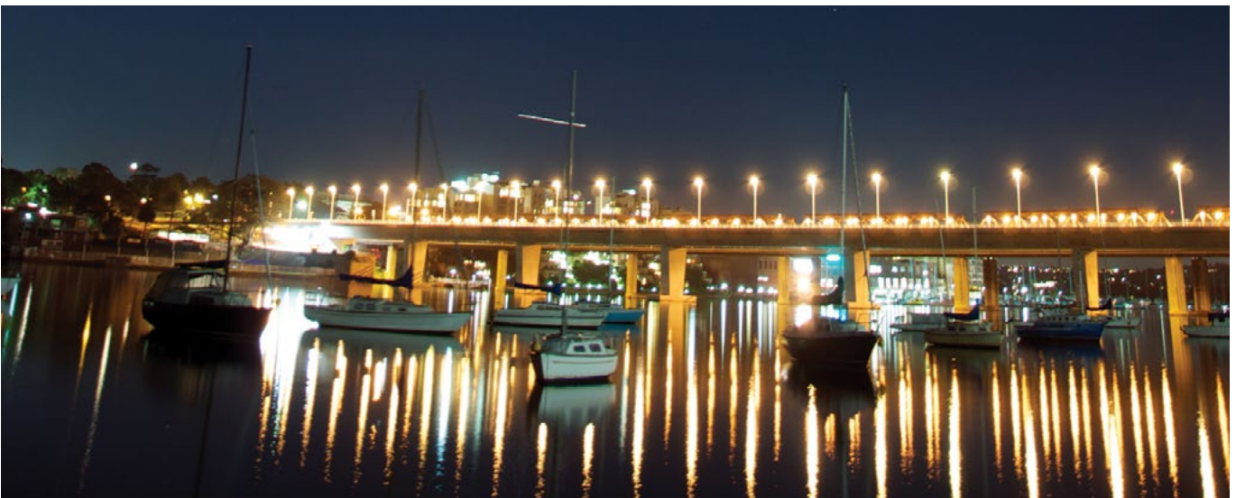
A closer spaced lower height lighting column has been used on the new Iron Cove Bridge to emphasise the curve of the bridge and provide a more rational, neater effect at night.
