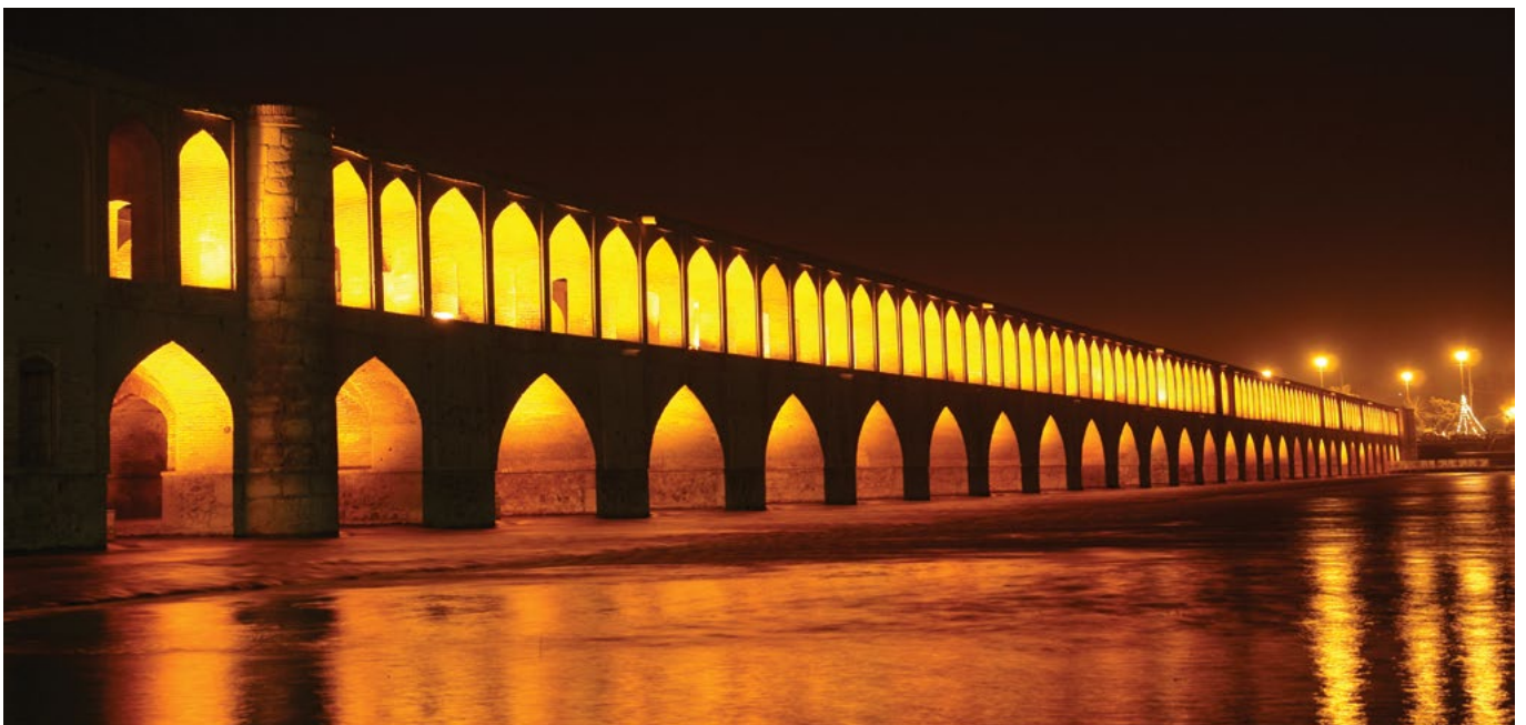
The Ilahverdi Khan Bridge.
