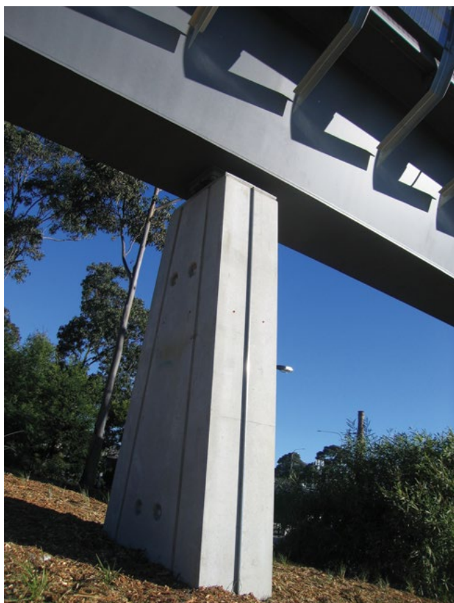
Tapered piers on the Falcon Street pedestrian bridge, which are wider at the base, give an impression of a strong connection to the ground.
