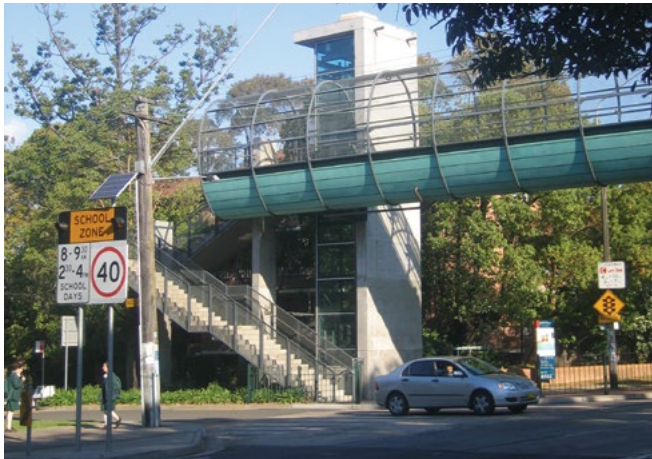
On the pedestrian bridge over The Boulevard in Strathfield the placement of the girder to the side of the piers / lift shafts allows for good district views out from the ends of the bridge.
