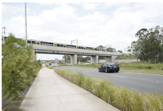
The South East rail link bridge over Camden Valley Way in south east Sydney demonstrates the aesthetic principles applied to railway bridges. The deeper girder and parapet has been shaped to reduce its visual dominance. Wall type piers have been used to simplify the appearance by avoiding headstocks. The abutment walls are set back in the landscape to minimise the impact on the footway and road corridor.
