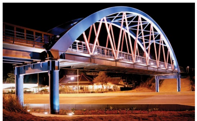
The colours on the rail bridge over the Pacific Highway at Coffs Harbour pick out the different elements of the bridge.
