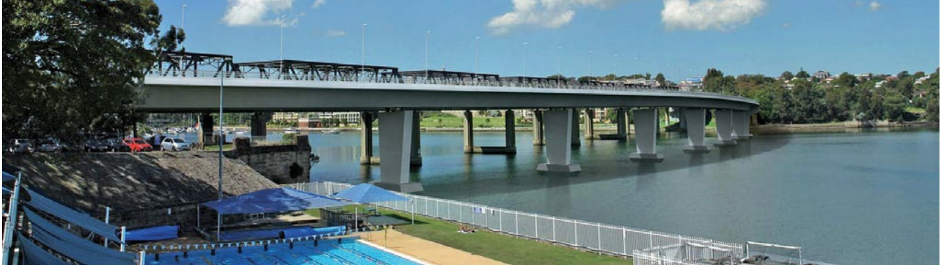
Iron Cove Bridge duplication — photomontage of proposed bridge developed during the concept design (development phase).
