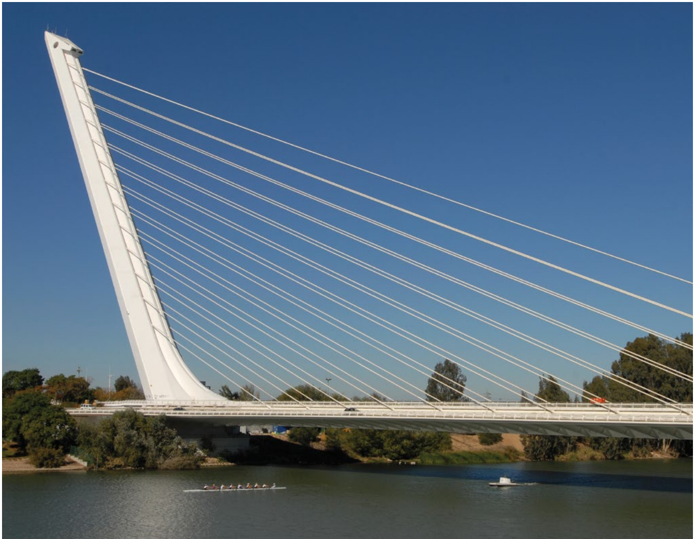
Alamillo Bridge, Seville
