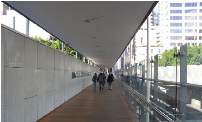
The pedestrian bridge, for the Sydney Harbour Foreshore Authority, connecting King Street with Darling Harbour over the Western Distributor in Sydney is as much a building as a bridge. The crossing takes the form of a large timber deck with shade structure, glazed views south and windows to the north.
