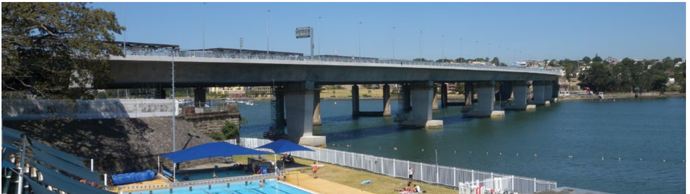
Iron Cove Bridge duplication — completed bridge. The quality and attention to detail in the detailed design and delivery stages, has ensured a close compliance with the agreed design. (Note, however, the later addition of signage which was not considered as part of the visual composition and should have been).
