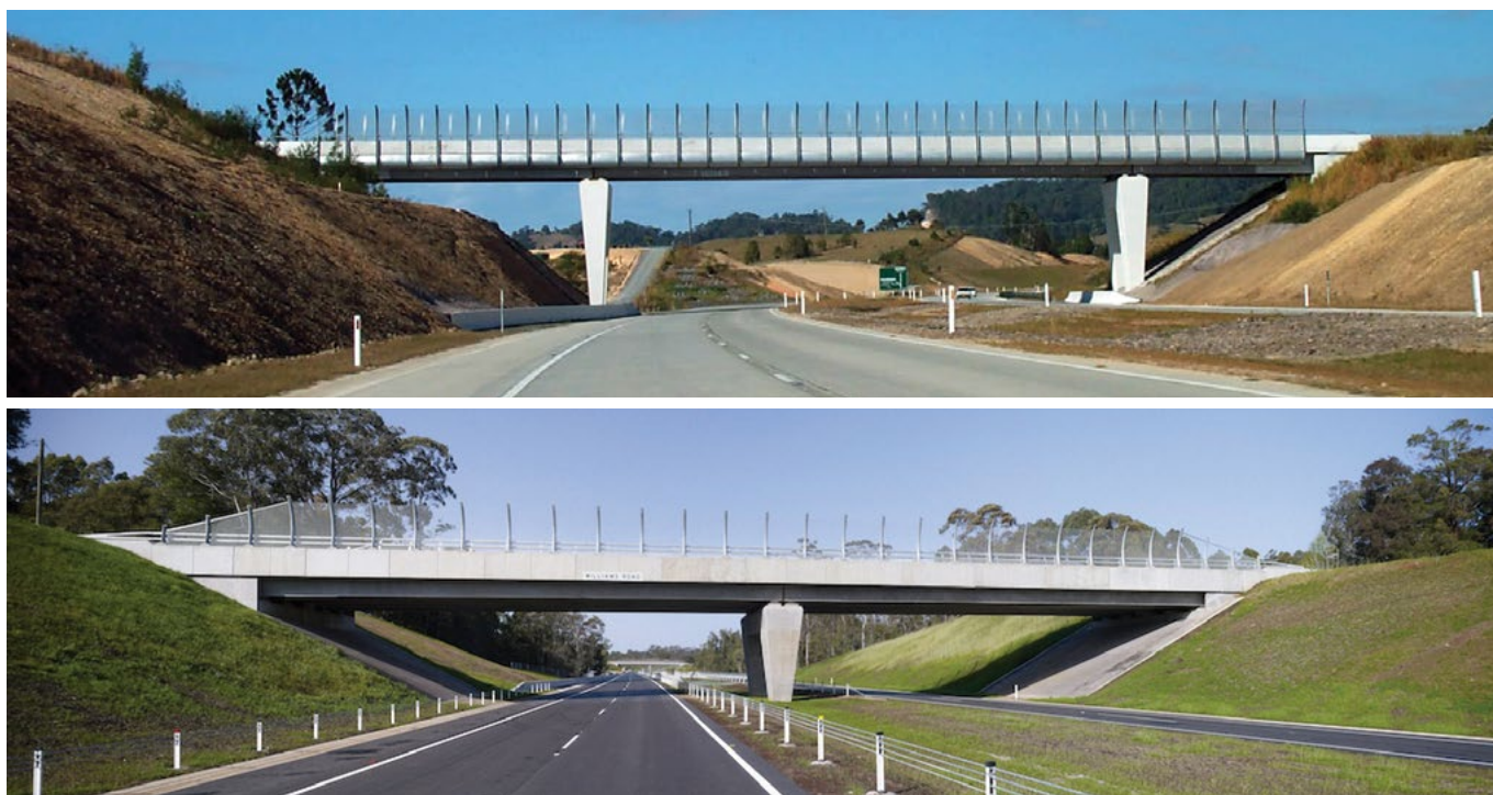
A family of bridges on the Pacific Highway. Top: Yelgun to Chinderah upgrade. Bottom: Bonville upgrade.
