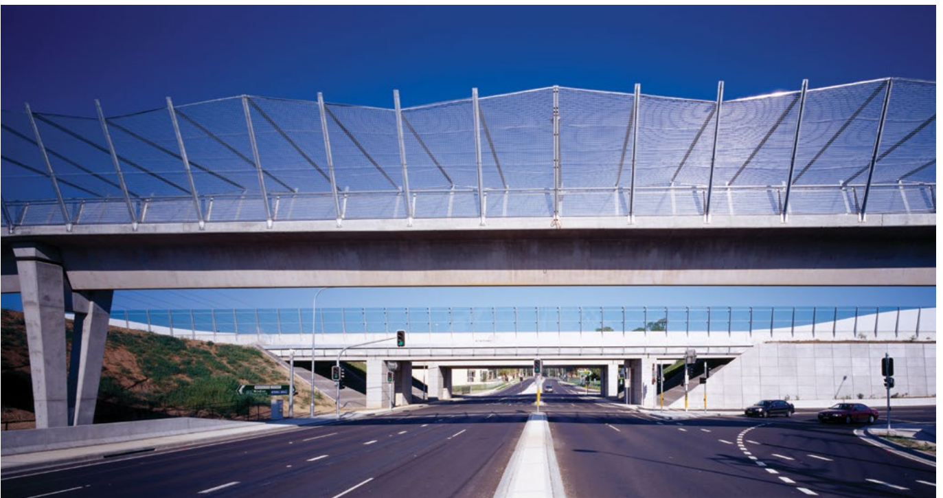
These screens on the M7 have been designed as a feature of the bridge; the flaring of the screens matches the flaring of the piers.
