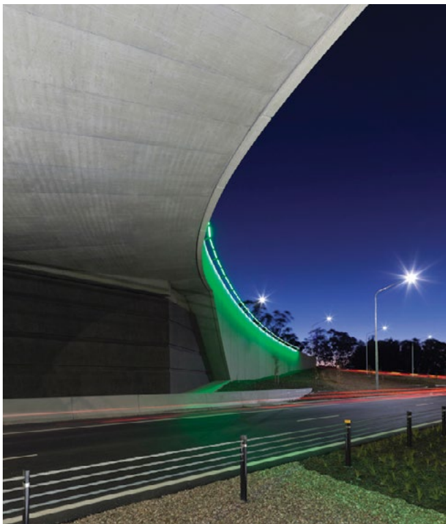
The underside view of the bridge is visually an important part of the space under the bridge. In this example in Canberra the slabbed girder creates a smooth lightly textured surface. LED lighting enhances the effect and also identifies the bridge. (Photo courtesy of Johnson Pilton Walker).
