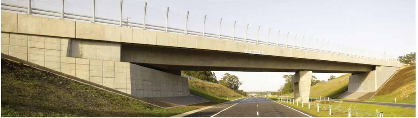
The slight angle of the abutment, around 5% outwards at the top, makes a more aesthetically pleasing outcome, which in this case at Bonville also reflects the pier taper.
