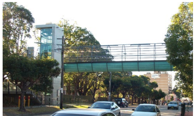
Transparent lift shafts can be attractive and feel safer due to the passive surveillance they allow. They can be fully 'glassed' as on the Cahill Expressway (above) or partially 'glassed' as on the bridge over The Boulevard at Strathfield (below).
