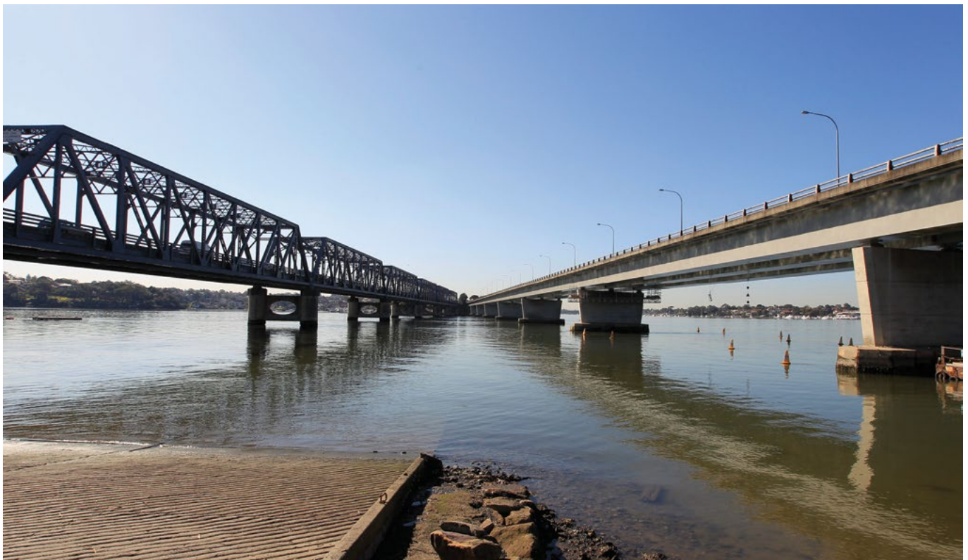
The piers on the concrete bridge over the Georges River at Tom Ugly's are reminiscent of the bow of a ship. They are well proportioned and suitably simple considering the proximity of the adjacent truss bridge. (The taper on the piers is 1 in 8).
