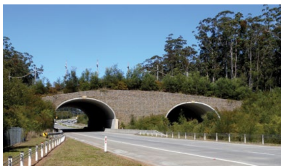
Arched forms and gabions give an impression of strength and an ecological/landscape purpose on the fauna overpass over the Pacific Highway at Bonville.
