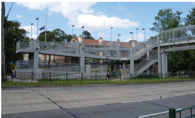
The Auburn pedestrian bridge, Parramatta Road, is not a good aesthetic outcome. The ramps and bridge connection are too dominant, jarring and cluttered. This bridge lacks aesthetic refinement.
