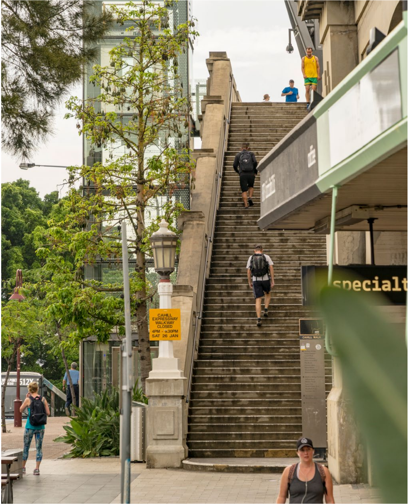
The SHB north lift, adjacent to the stairs, provides step free access to the bridge walkway from the north.
