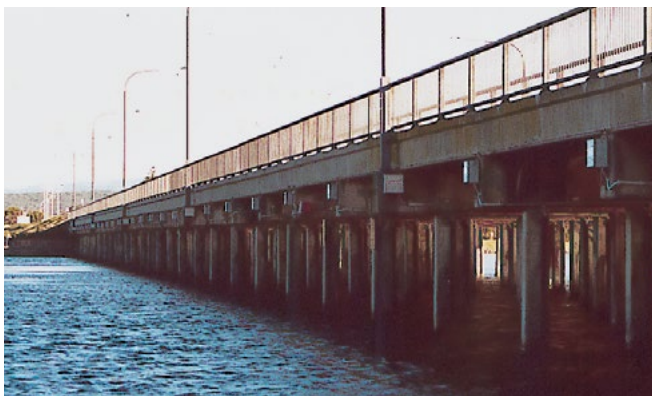
Many piers on the bridge over the inlet to Lake Illawarra creates an overall complex, wharf-like visual effect which does not create a graceful appearance.
