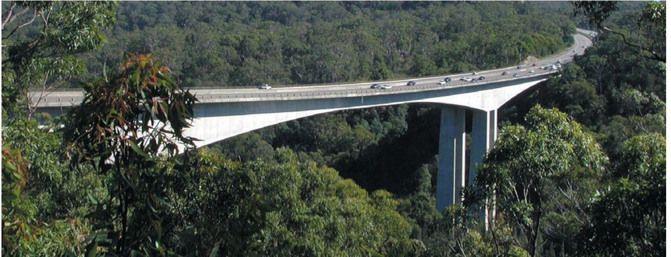
The haunched girders on the twin bridges over Mooney Mooney Creek on the F3, demonstrate the principles of span, taper and curvature.
