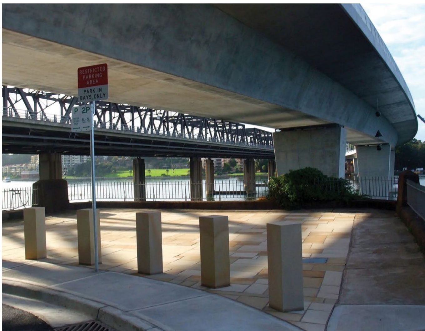
The sensitive use of sandstone paving and bollards, at the heritage abutments under the new Iron Cove Bridge in Rozelle, has created a place to view the evolution of harbour crossings at this point – from early ferries to timber truss to Art Deco steel truss to concrete incrementally launched girder.
