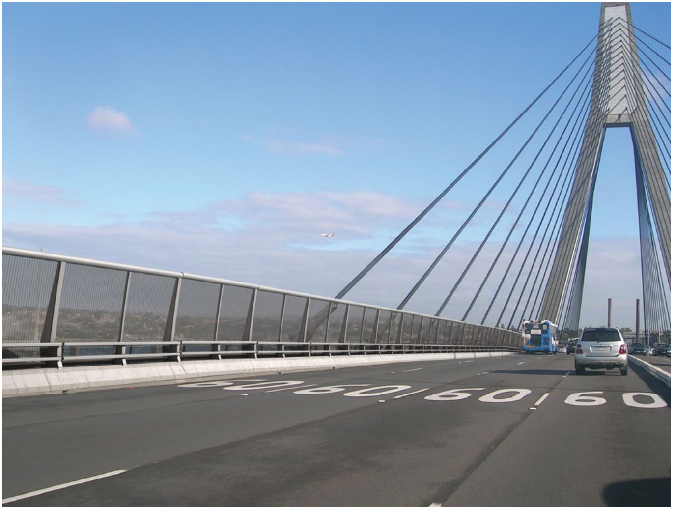
Photomontage of new fencing for the Anzac Bridge, the design of which was developed by a collaboration between the urban designers and the engineers.
