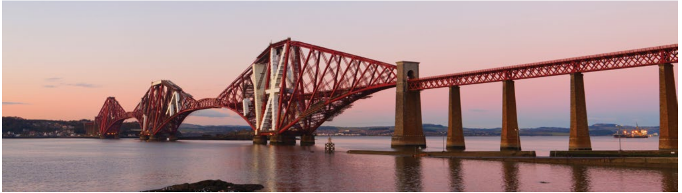
The rail bridge over the River Forth estuary, Edinburgh.
