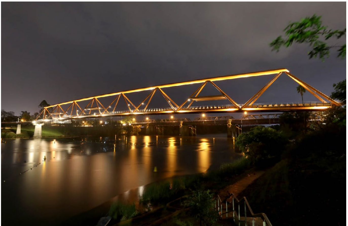
Lighting at the Yandhai River Crossing highlights the structural elements of the bridge. Lighting fixtures follow the diagonal path of the truss structure.
