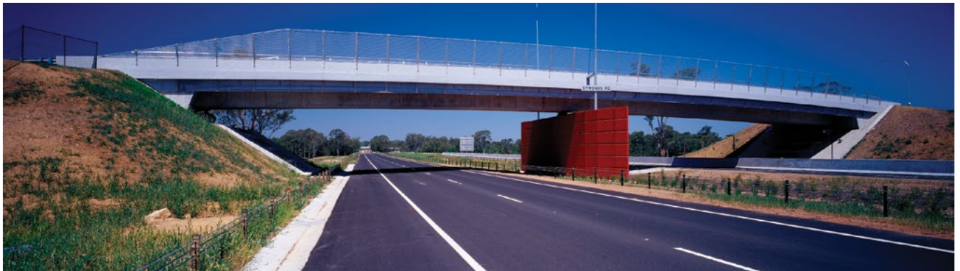
The inward angled abutments on this M7 bridge are an attractive detail which visually emphasises the span. On this bridge the central pier is encased in an architectural wing wall feature as part of the corridor aesthetic. In general it is preferable to express the structure honestly and integrate aesthetics and engineering as this document espouses.
