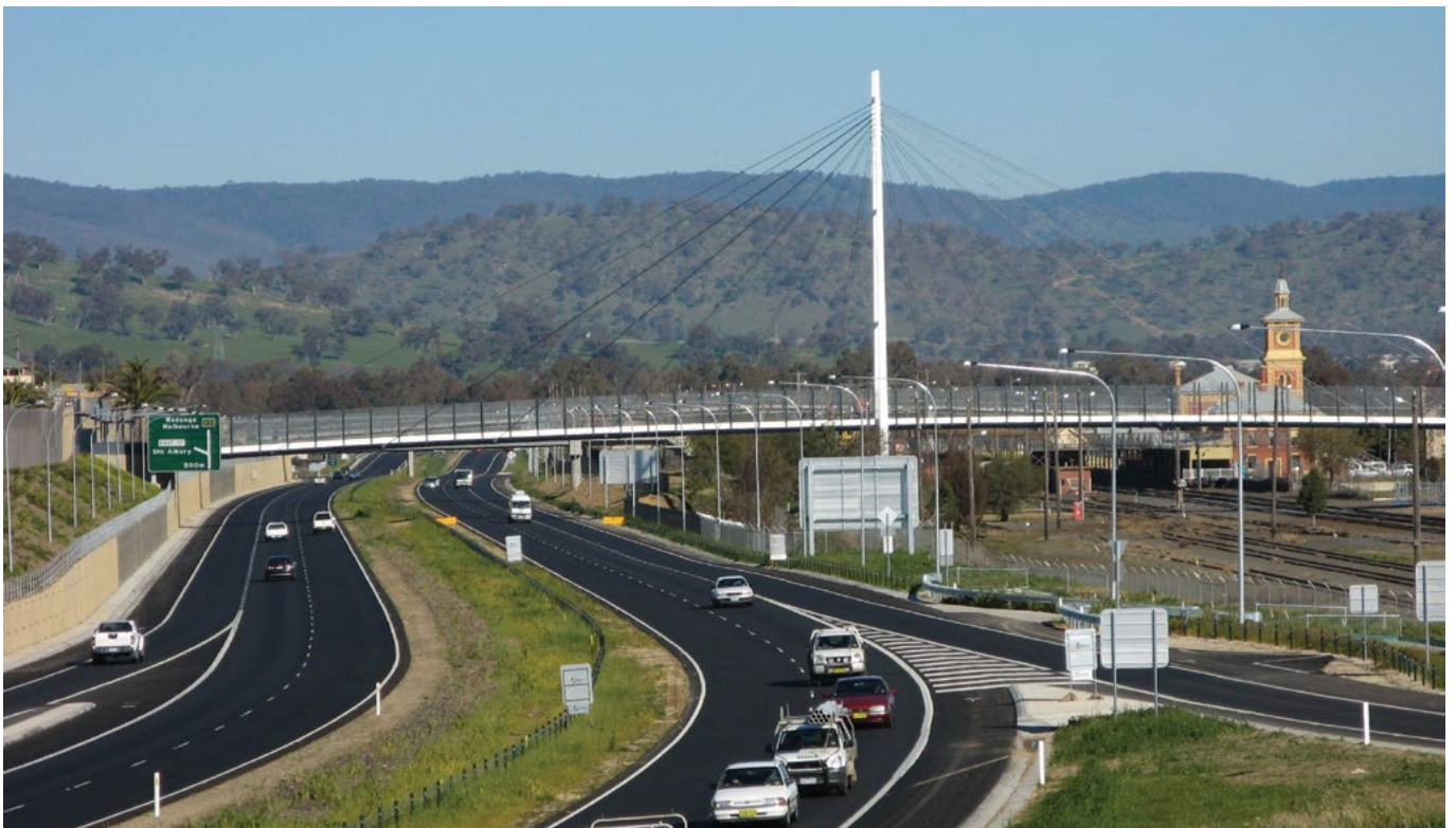
A white painted finish can help emphasise the main features of a bridge. On the Albury bypass, selecting the white colour matches the white war memorial at the opposite end of the Dean Street visual axis but also marks the position of the bridge in the corridor.
