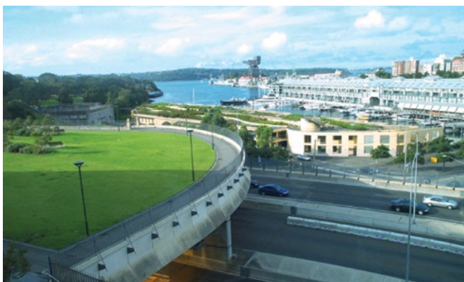
Land bridges are valuable solutions for bridges in urban areas where it is important to re-establish open space that otherwise would be used for the road corridor as on the Eastern Distributor at the Art Gallery precinct.
