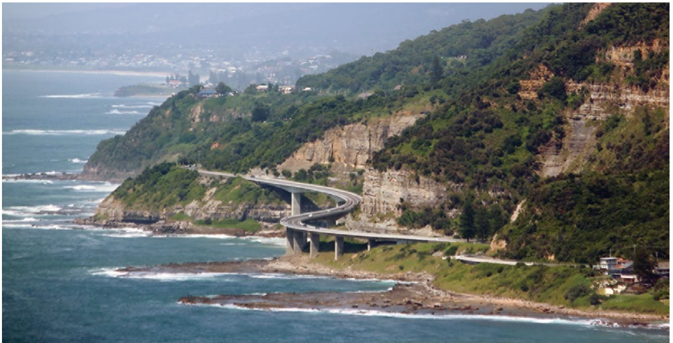
The Sea Cliff Bridge, Lawrence Hargrave Drive, is a seamless combination of incrementally launched and balanced cantilever structures. It's design is simple, expresses it's structure and provides a foil to the rugged coastal landscape.
