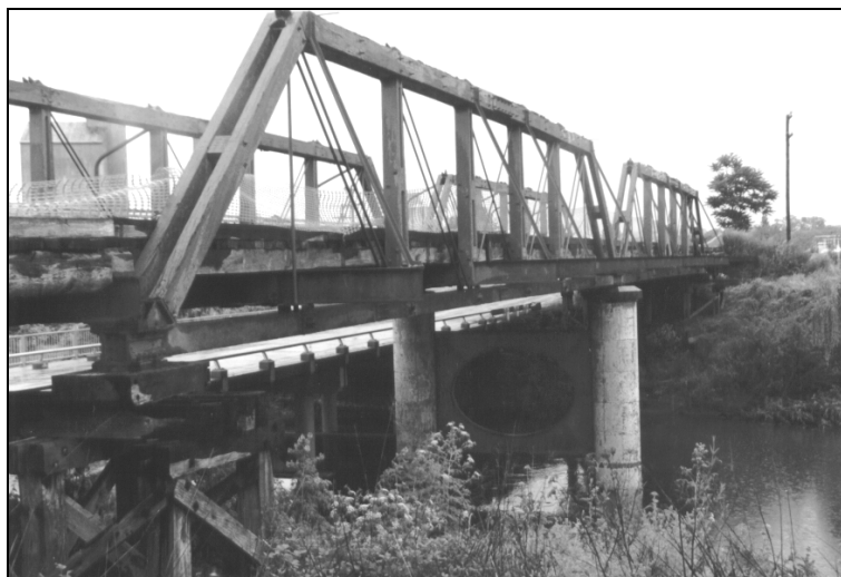
Figure 1.3.5b – The bridge over the MacIntyre River at Inverell was one of DeBurgh's early Pratt trusses with sloping end members.
