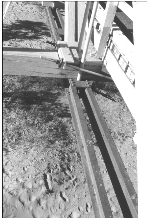
Figure 1.3.6b – The pair of steel channels that made up the bottom chord utilised the tension characteristics of steel along with the compression characteristics of the timber.
