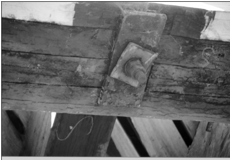
Figure 1.3.2g –Four flitch bottom chord - View from underside
