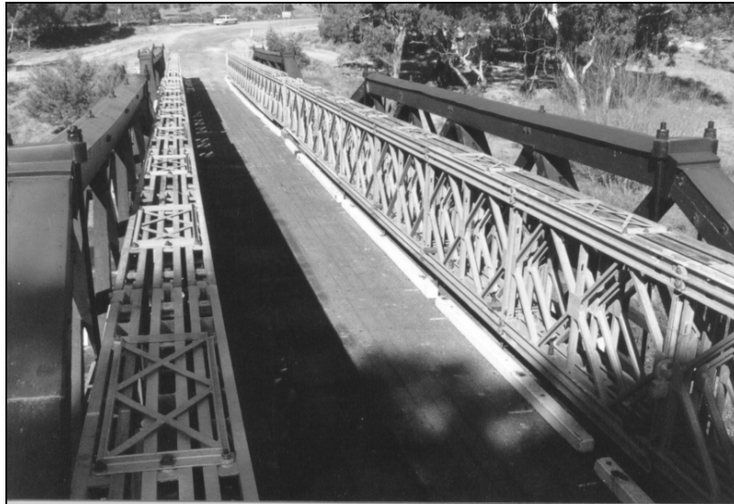
Figure 1.3.3h – Bailey Bridges became the preferred method of temporary support during maintenance and rectification works.
