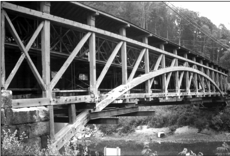
Figure I.3.1e – A typical Burr truss exposed during restoration work, Barrickville, West Virginia
