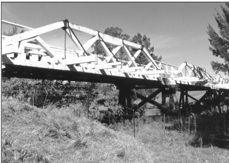
Figure 1.3.2c – Typical Old PWD truss (Monkerai Bridge over the Karuah River )
