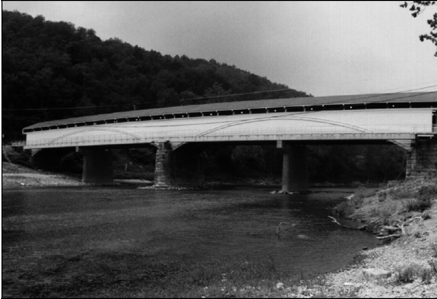
Figure I.3.1d – Typical American covered timber bridge, the Philippi Bridge, West Virginia
