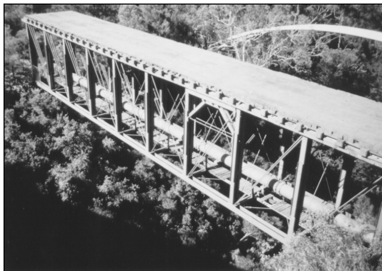
Figure 1.3.5d – The 1901 DeBurgh Bridge over Lane Cove River. DeBurgh's greatest achievement with a 165ft (50.3m) deck span was damaged in the 1994 bush fires.
