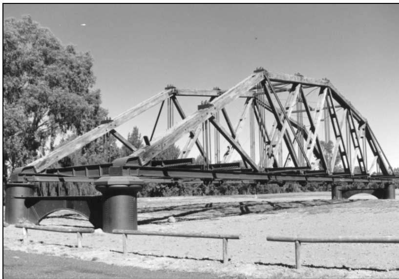
Figure 1.3.3i – A span of the original Lachlan River Bridge at Cowra on display at a nearby riverside park. The bridge utilised steel tension members and timber compression members in an early example of composite design.
