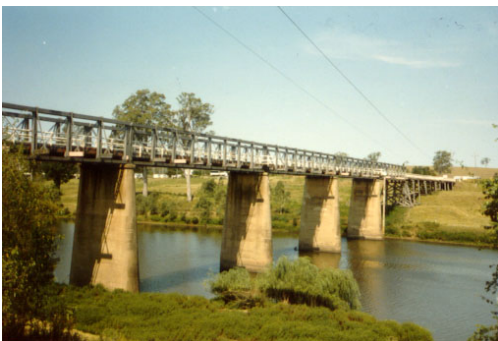
Solutions beyond the limits of timber beam bridges, left, timber trusses on concrete piers over the Clarence River at Tabulam, right, iron lattice trusses on cylindrical iron piers over the Snowy River at Dalgetty.
