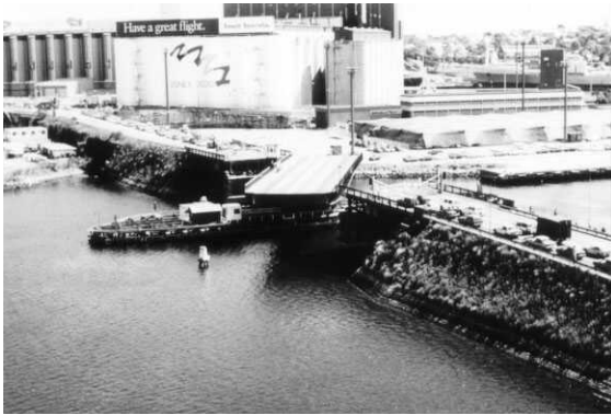
Glebe Island swing bridge
