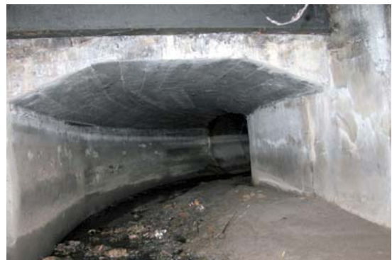
Arched connection from slab culvert to circular pipe under footpath
