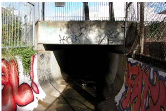
Entrance to culvert under Parramatta Road Burwood
