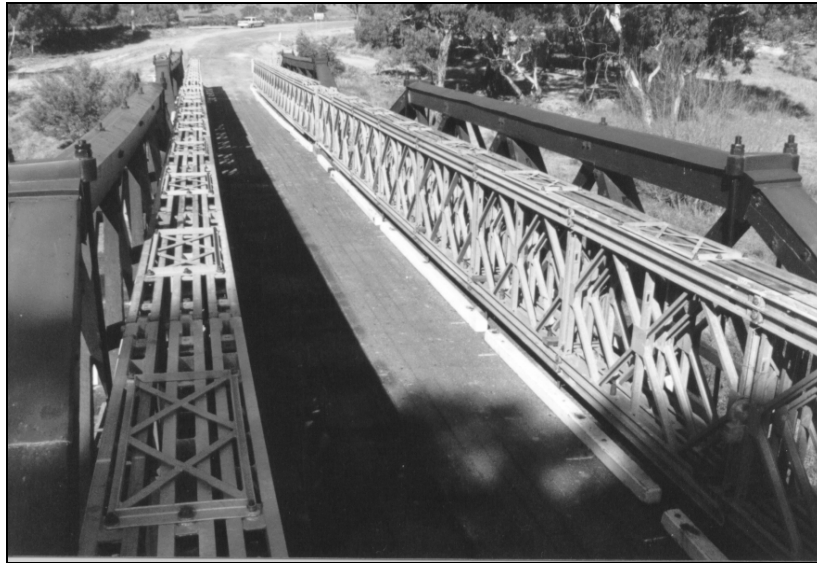
Figure 1.3.3h – Bailey Bridges became the preferred method of temporary support during maintenance and rectification works.
