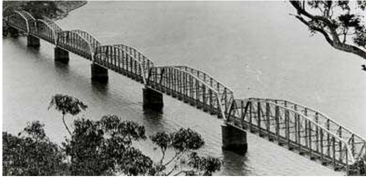
The largest bridge in colonial New South Wales, the American designed Hawkesbury River railway Bridge.
