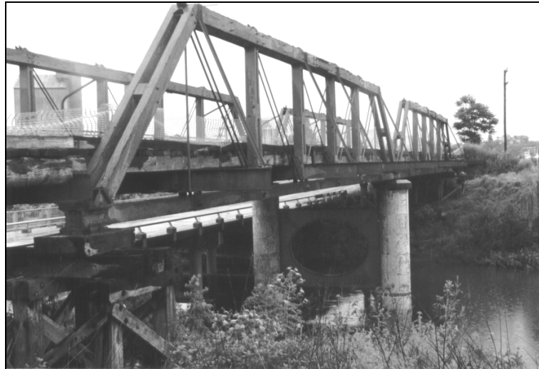
Figure 1.3.5b – The bridge over the MacIntyre River at Inverell was one of DeBurgh's early Pratt trusses with sloping end members.
