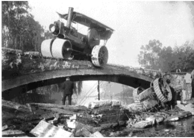
Kings Bridge collapse during load test by steam and traction engines – both visible (source http://home.vicnet.net.au/~aholgate/jm/ )
