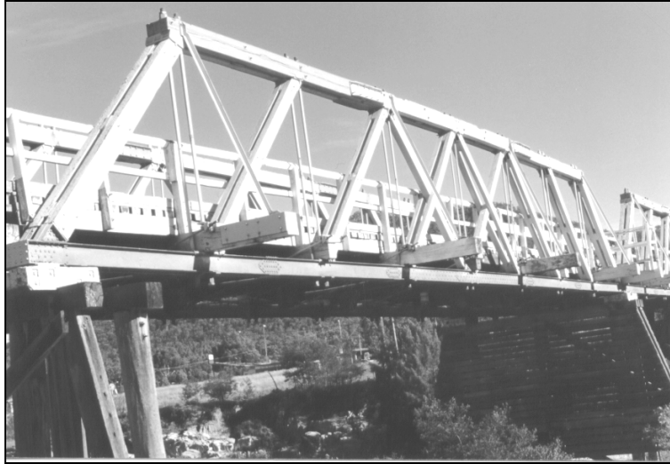
Figure 1.3.6a – Bulga Bridge over Wollombi Brook is typical of Dare's design.
