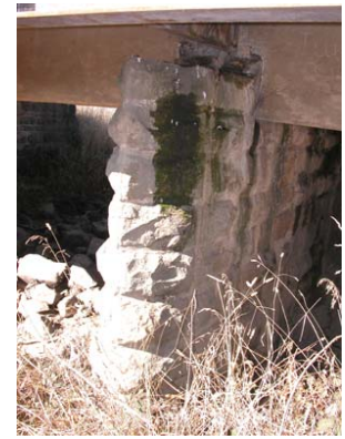
Bowning Creek Bridge (RTA Bridge No 6474) Stone wall pier
