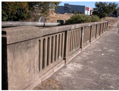
Haslams Bridge (RTA Bridge No 307) Original reinforced concrete railings
