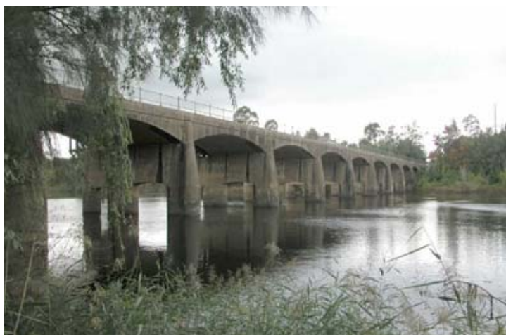
Bridge over Hawkesbury River at Richmond 1905 (RTA Bridge No 429)
