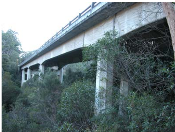
Woronora River (RTA Bridge No 152)
