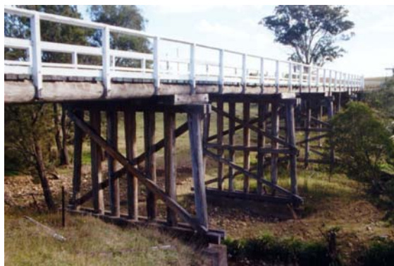
The 1894 timber beam road bridge
