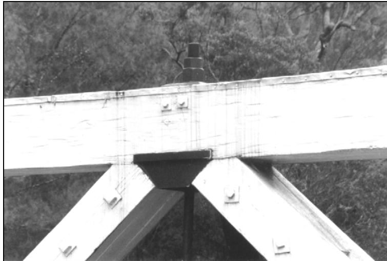
Figure 1.3.3e – Connection of diagonals to top chord via cast iron plates provided a superior transfer of force.
