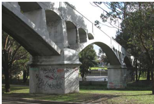
Whites Creek Aqueduct, Annandale
