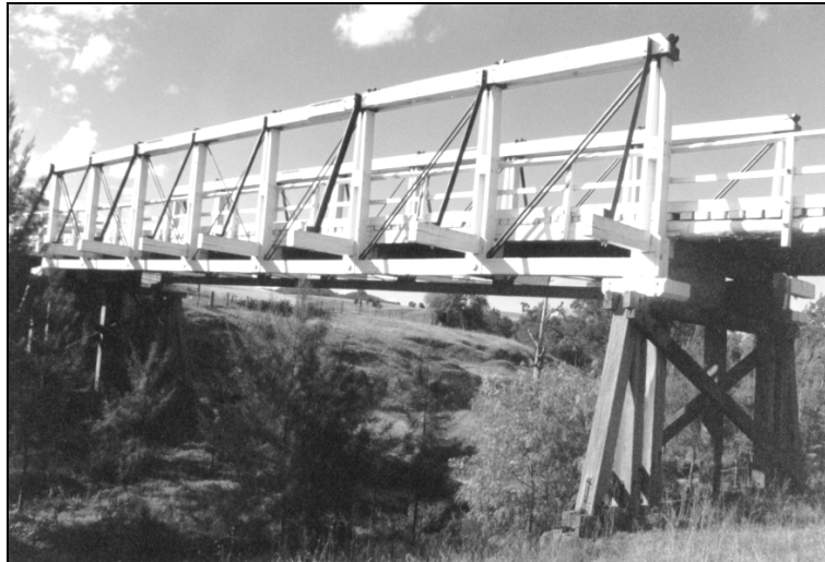
Figure 1.3.5c – The square ends that are typical of the DeBurgh truss.
