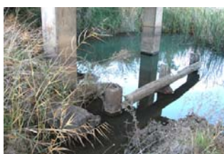
Previous pier timbers, Tyagong
