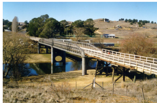
Solutions beyond the limits of timber beam bridges, left, timber trusses on concrete piers over the Clarence River at Tabulam, right, iron lattice trusses on cylindrical iron piers over the Snowy River at Dalgetty.
