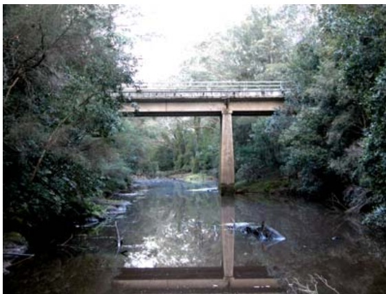
Wandandian Creek (RTA Bridge No 723) This sturdy high level structure was erected in 1929 replacing a set of three low level timber bridges vulnerable to flood. As well as motor traffic, the bridge was used by bullock teams dragging logs to the Wandandian Sawmill
