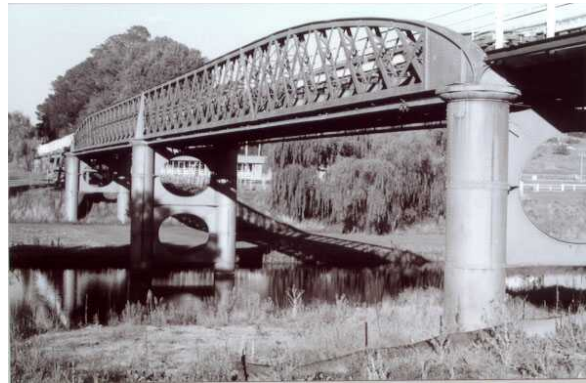
Typical lattice truss
