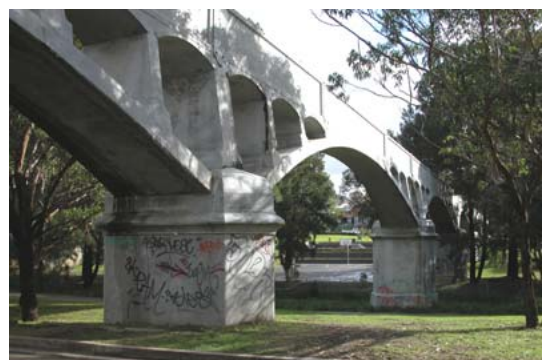
Whites Creek Aqueduct, Annandale
