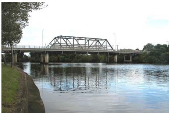
Bridge over the Dawson River at Cundletown (RTA Bridge No 1803)
