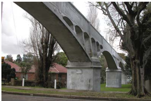
Johnstons Creek Aqueduct, Annandale
