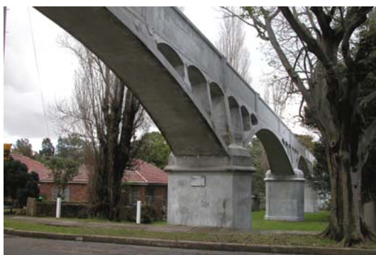
Johnstons Creek Aqueduct, Annandale
