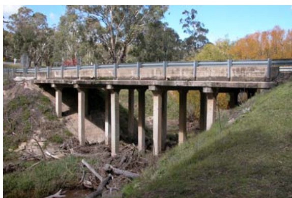
Surveyors Creek Walcha 1916 (RTA Bridge No 3485)
