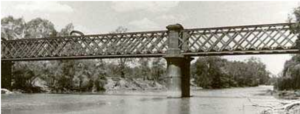
An 1884 sturdy British lattice bridge and the 1901 American Pratt trusses.
