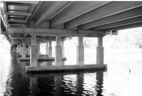
Steel beams at Wallarah Creek
