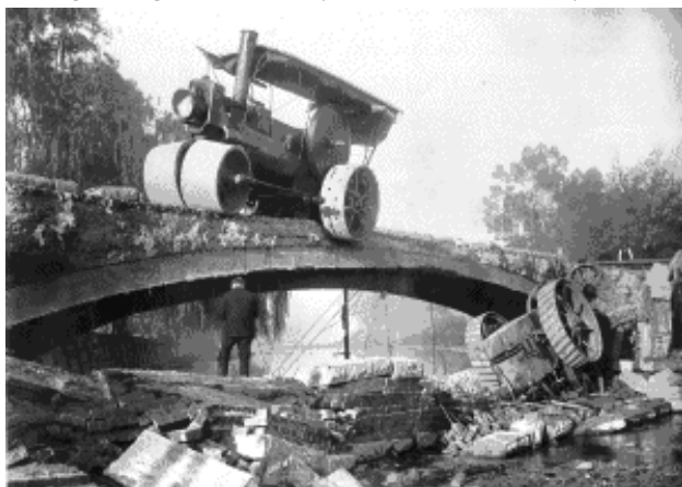
Kings Bridge collapse during load test by steam and traction engines – both visible (source http://home.vicnet.net.au/~aholgate/jm/ )
