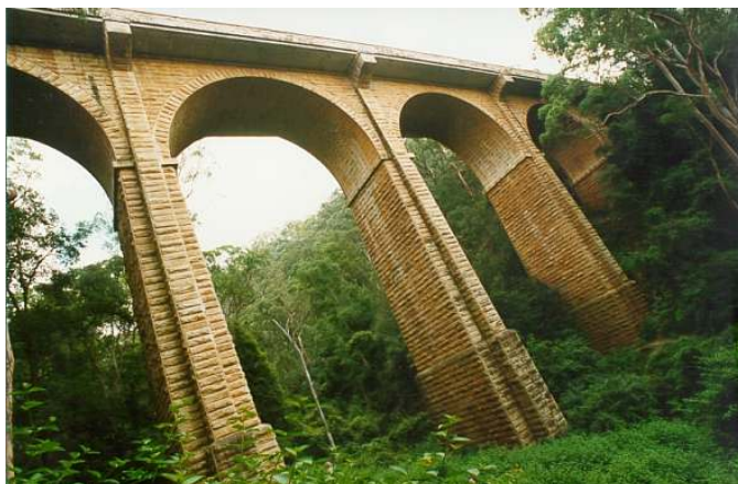
Lapstone masonry arch bridge (RTA Bridge No 967) (Photo NPB Photographics)
