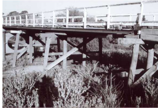
Elevation of timber approach.
