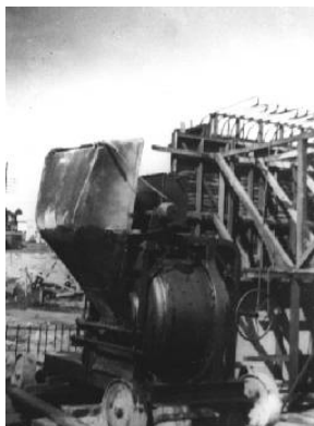
Concrete mixer 1947 – Cockle Creek railway bridge (Photo Max Broadbent)
