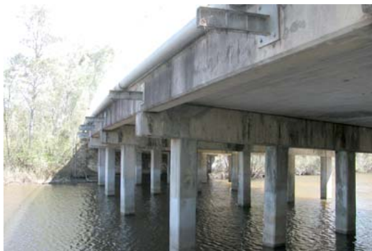
Middle Creek No 3 (RTA Bridge No 148) – delayed by War
