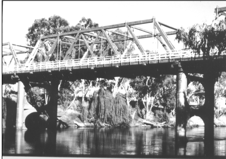
Figure 1.3.4e – Hampden Bridge, Wagga Wagga. The first of Allan's large overhead through truss bridges with 3 truss spans, each of 110ft (33.5m).
