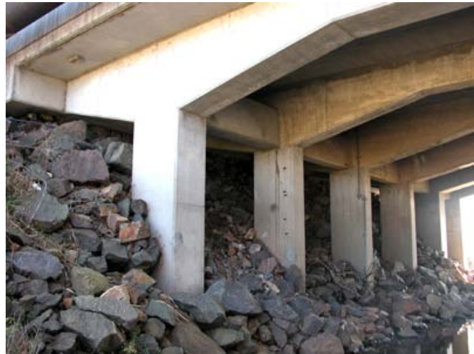
Stapletons Bridge Albion Park (RTA Bridge No 881) showing original frames, centre, and widening frames
