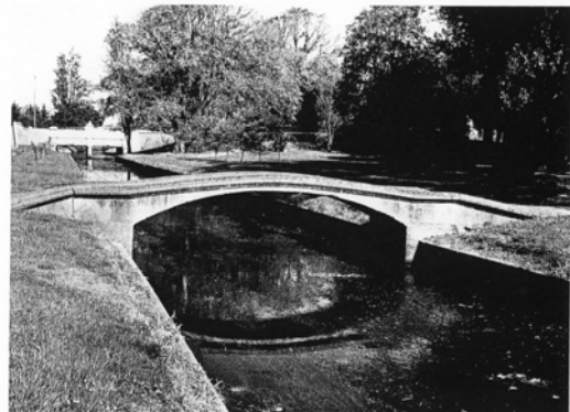
Otepunu Gardens footbridge c1899 (source Bridging the Gap by G Thornton)
