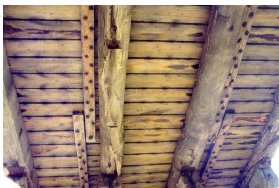
First layer of cross planks on the girders
