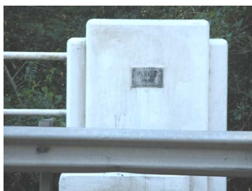
Middle Creek Bridge (RTA Bridge No 147) Post art deco endpost
