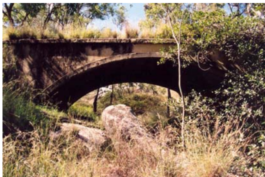
Reads Gully Bridge, Tamworth
