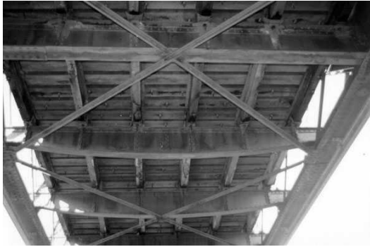
Typical timber beam bridge deck, its log girders and plank deck.
