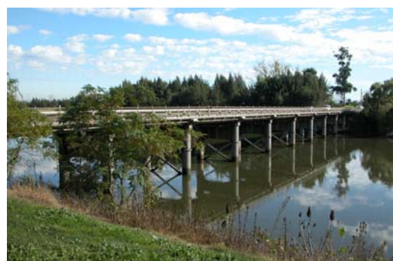
Hawkesbury River (RTA Bridge No 415) Viewed from riverbank parkland
