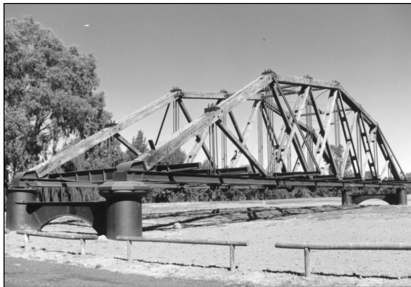
Figure 1.3.3i – A span of the original Lachlan River Bridge at Cowra on display at a nearby riverside park. The bridge utilised steel tension members and timber compression members in an early example of composite design.
