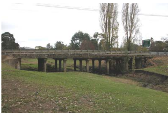
Muttama Creek Cootamundra 1914 (RTA Bridge No6438)
