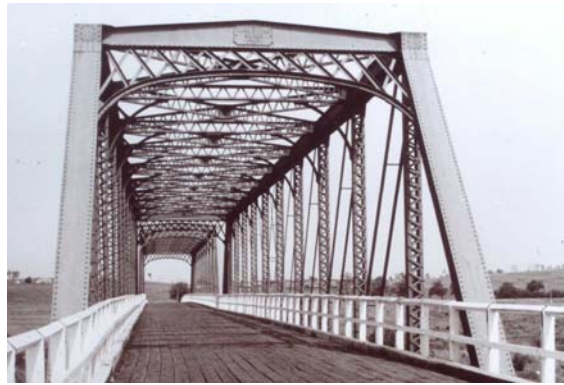
The Luskintyre trusses are a good example of a through bridge.
