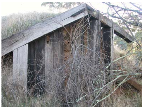
Mummel Bridge (RTA Bridge No 6677) Old abutment
