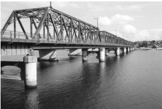
Overhead braced truss
