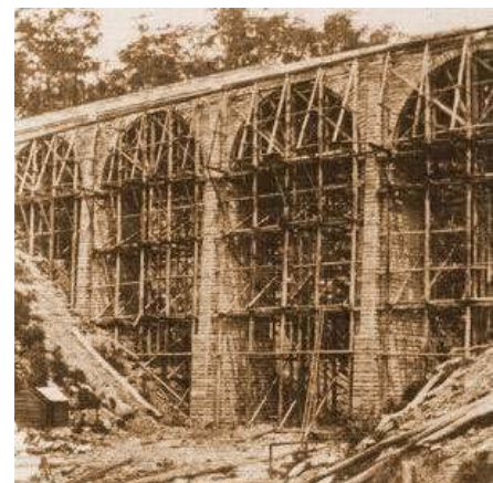
Lapstone Bridge during construction (source http://info.mountains.net.au/rail/lower/lapstone.htm )
