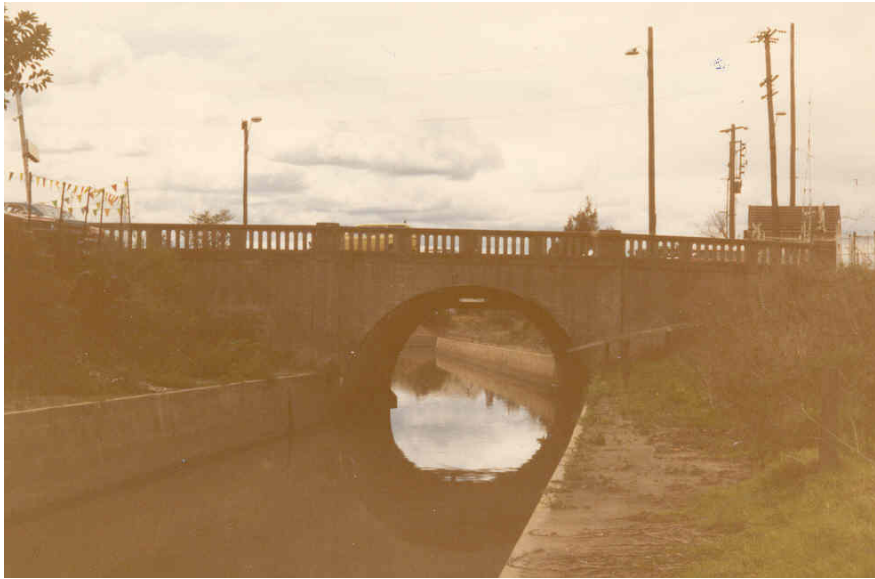
Figure 1.8: View of the Duck Creek Bridge at Granville looking north.
