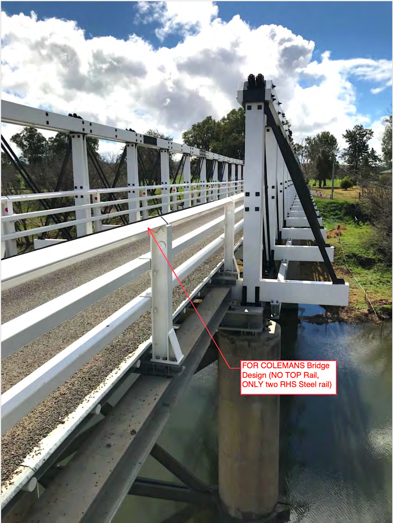
FIGURE 30: INDICATIVE NEW TRAFFIC BARRIER (GLENNIES CREEK, MIDDLE FALBROOK)
