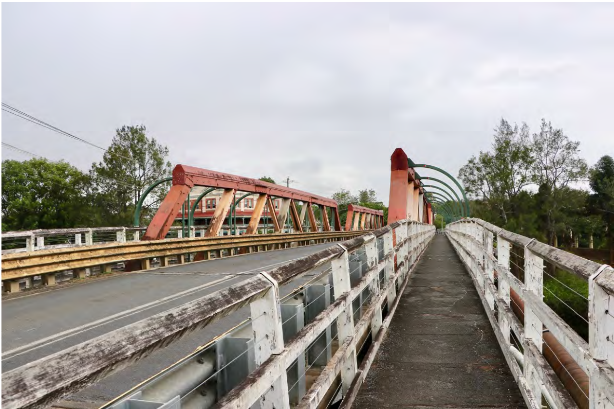
FIGURE 21: DETAIL OF WALKWAY, DECK, THRIEBEAM BARRIER + TRUSSES (WEST END)
