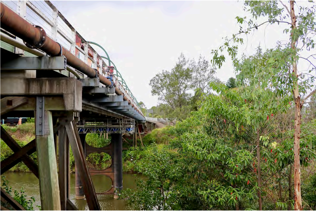
FIGURE 22: DOWNRIVER SIDE OF COLEMANS BRIDGE (SUBSTRUCTURE)
