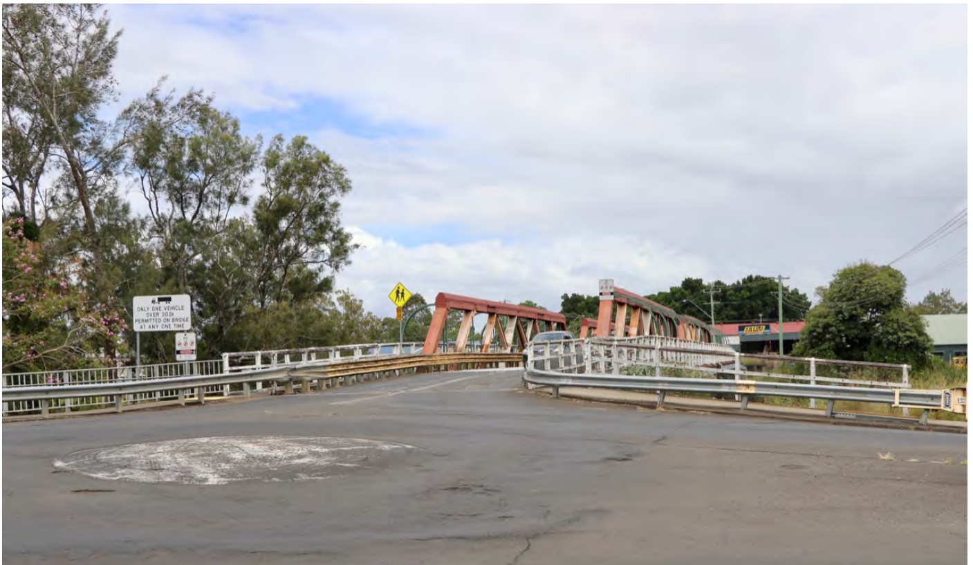
FIGURE 15: EASTERN APPROACH (WITH ROAD JUNCTION IN FOREGROUND)
