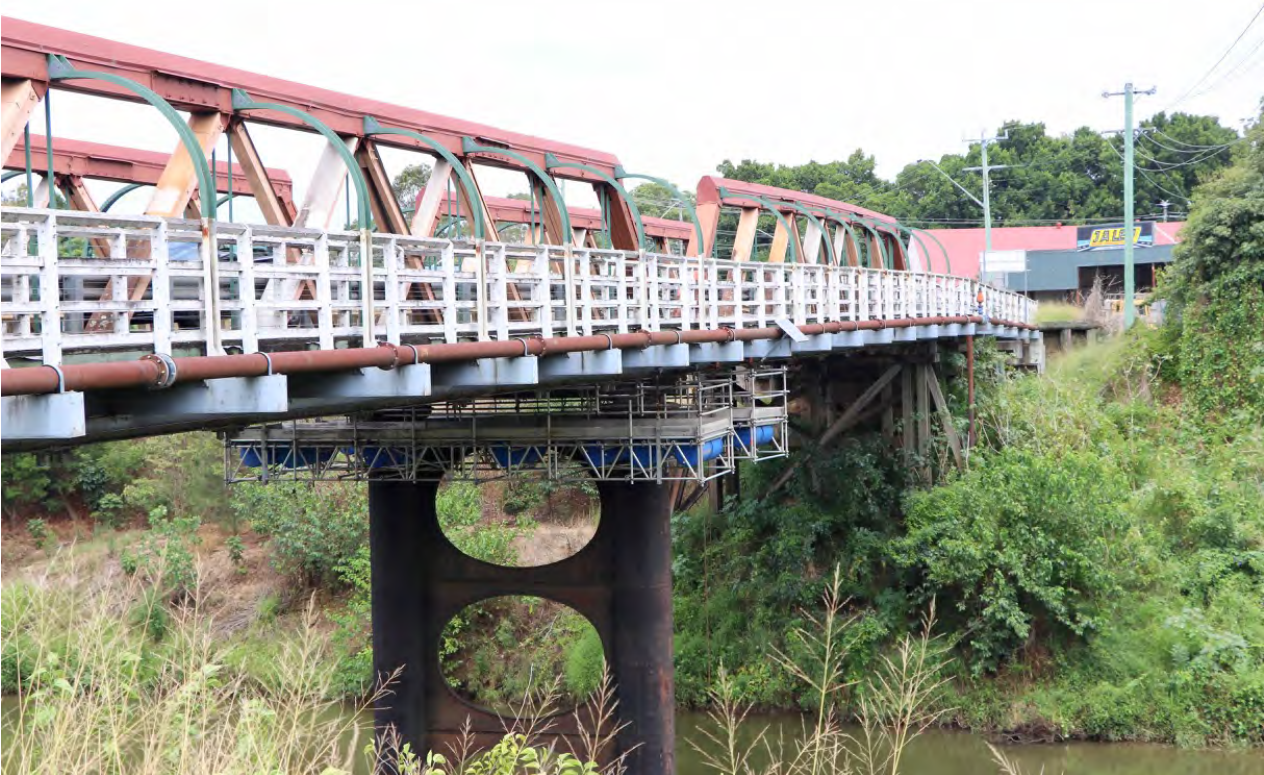
FIGURE 17: TRUSS SPANS + IRON PIER NO.3 + WALKWAY (UPSTREAM SIDE DETAIL)
