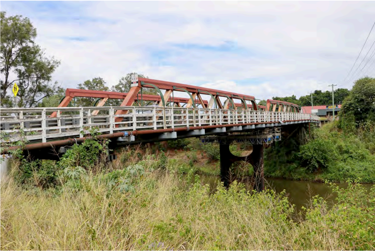
FIGURE 16: TRUSS SPANS
