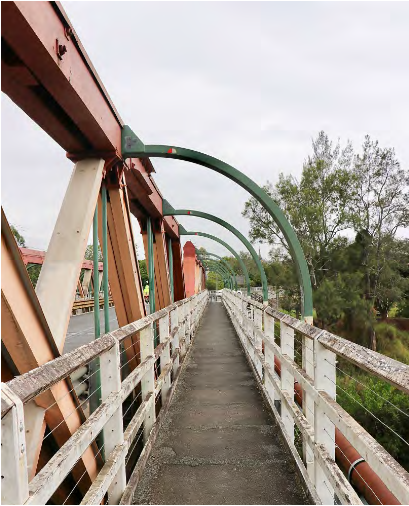
FIGURE 35: EXISTING SWAY BRACING THRIEBEAM BARRIER DAN TUCK 2019
