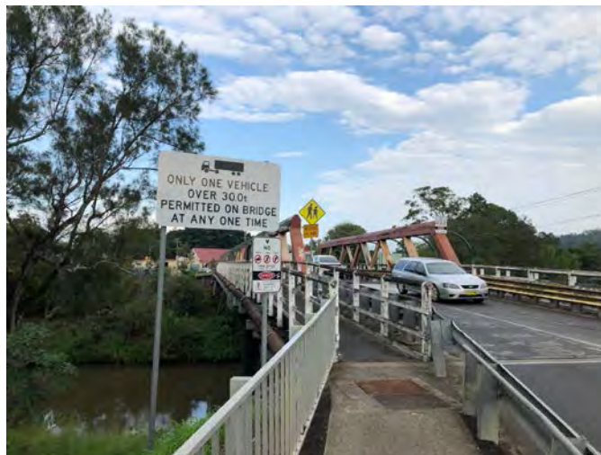
Plate 2-2 - View of bridge from eastern abutment (southern walkway)
