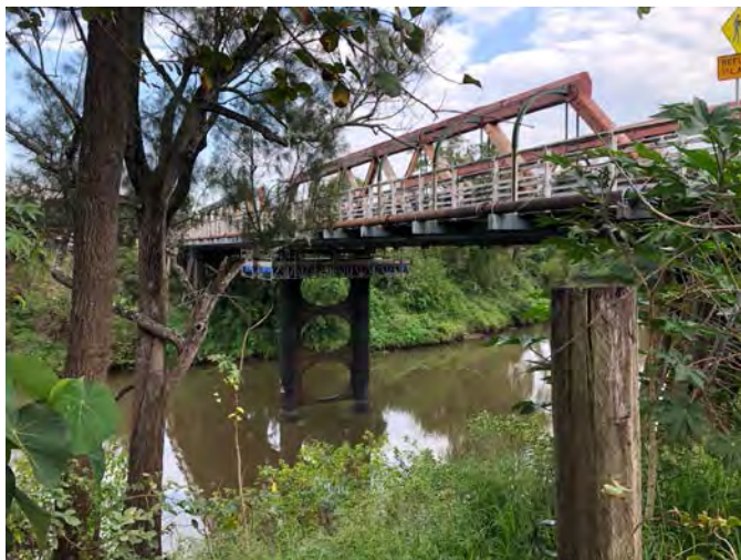
Plate 2-1 - Colemans Bridge viewed from the eastern abutment (southern side of bridge)
