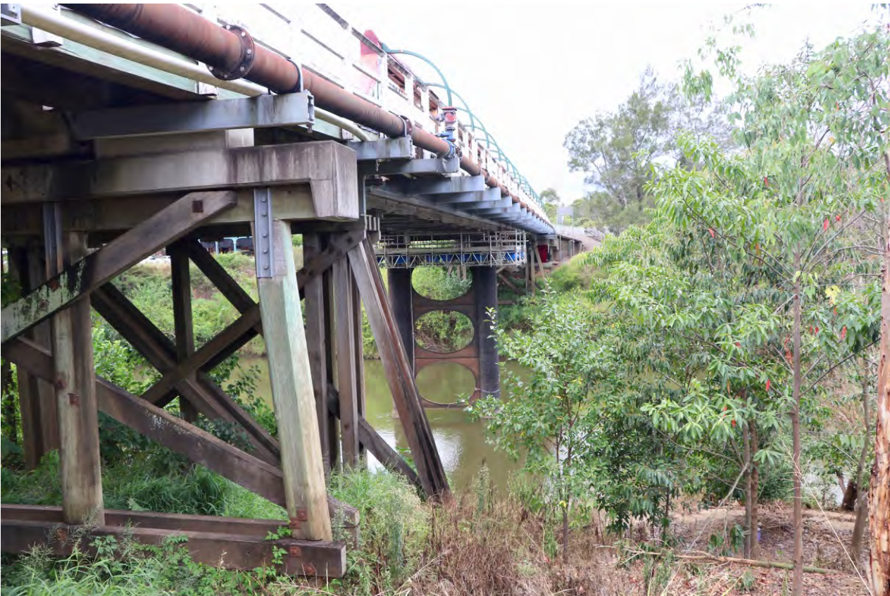
FIGURE 23: DOWNRIVER SIDE OF COLEMANS BRIDGE (TRESTLES; SOFFIT & CENTRAL IRON PIER)
