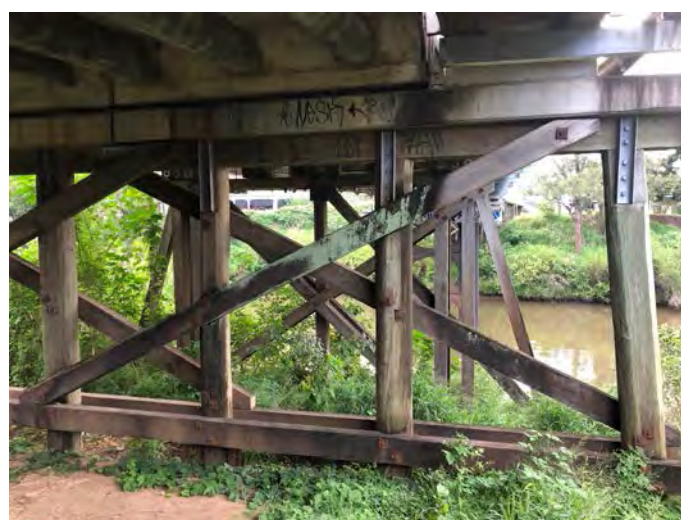
Plate 2-4 -Timber trestle piers on the western river bank
