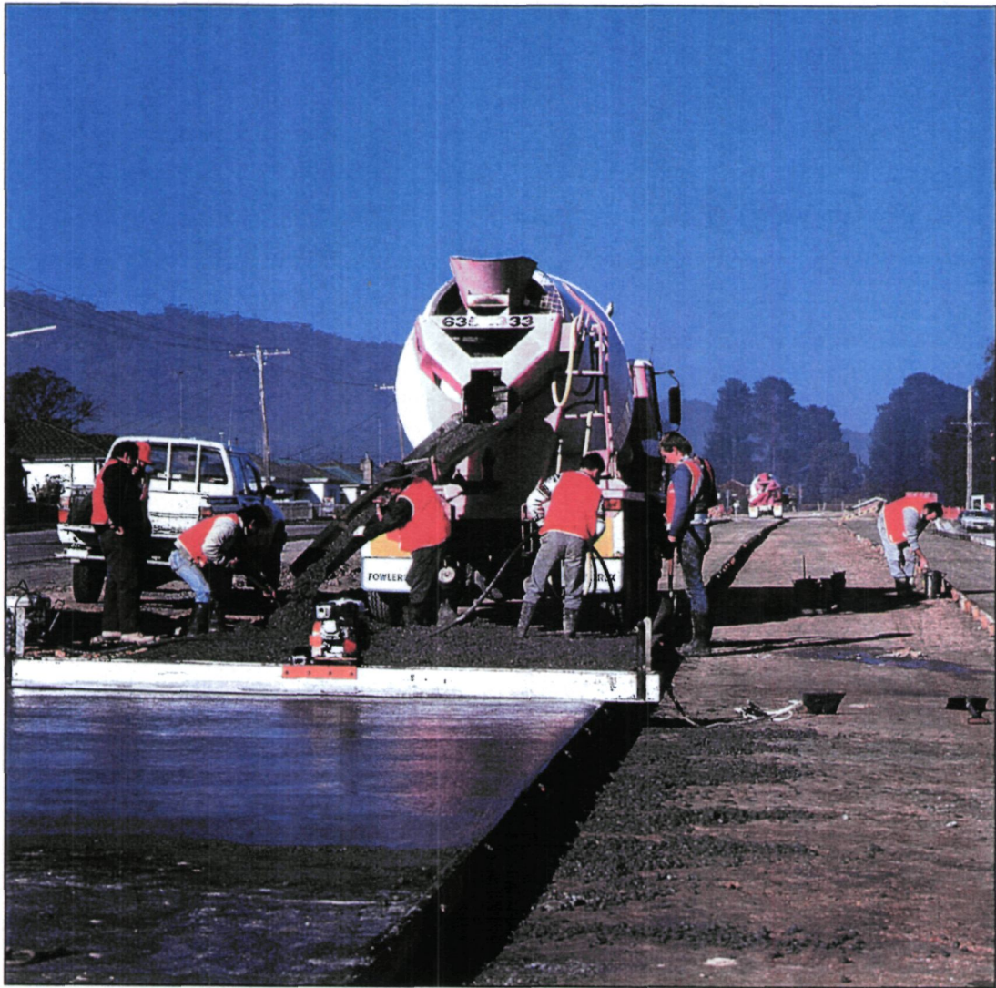
Concreting work at Bowenfels, 1990
