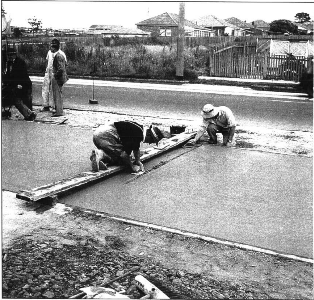
Tooling of edges at transverse expansion joint, 1955
