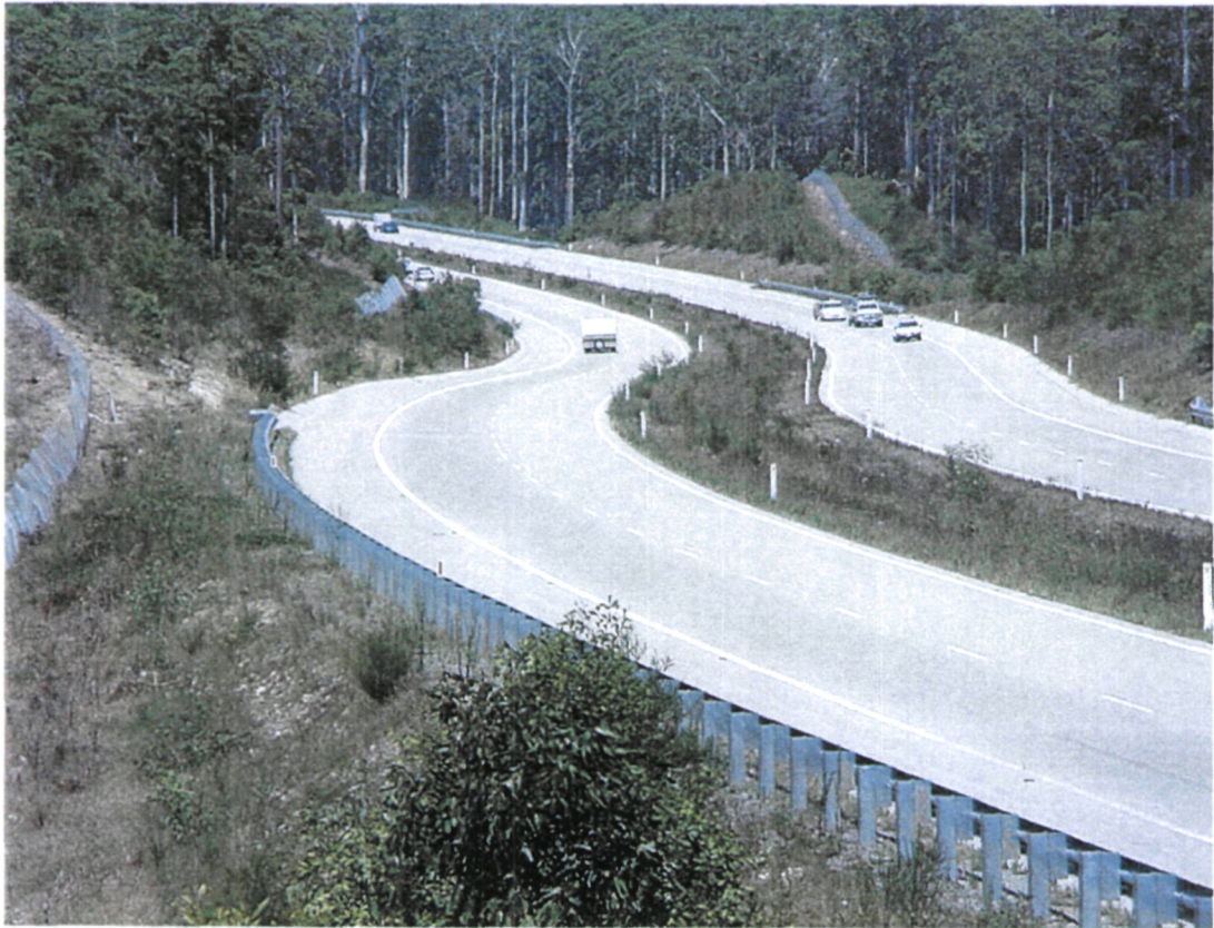
Pacific Highway Deviation at Bulahdelah
