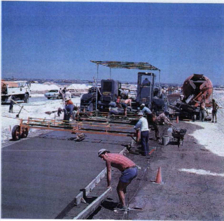
The paver at work on Foreshore Rd, 1979
