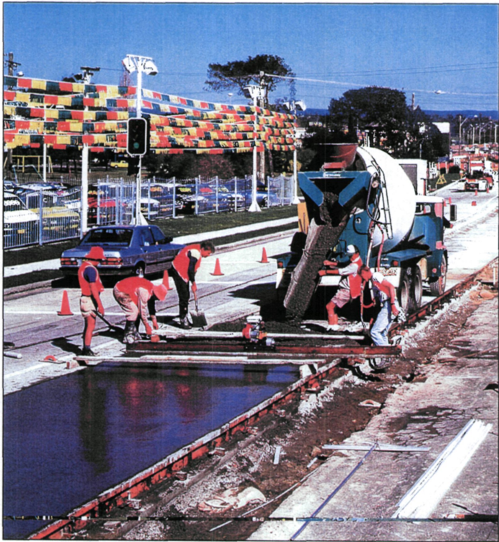
Concreting work at St Marys, 1985
