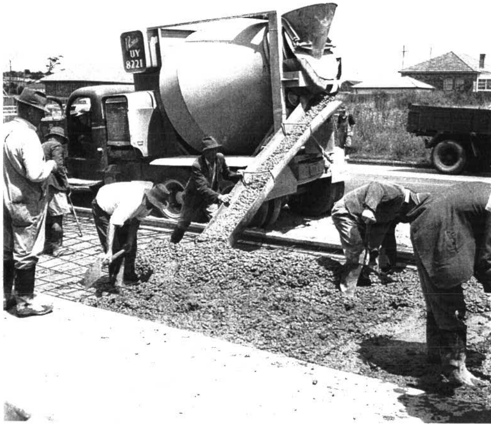
Delivery and spreading of concrete, 1955
