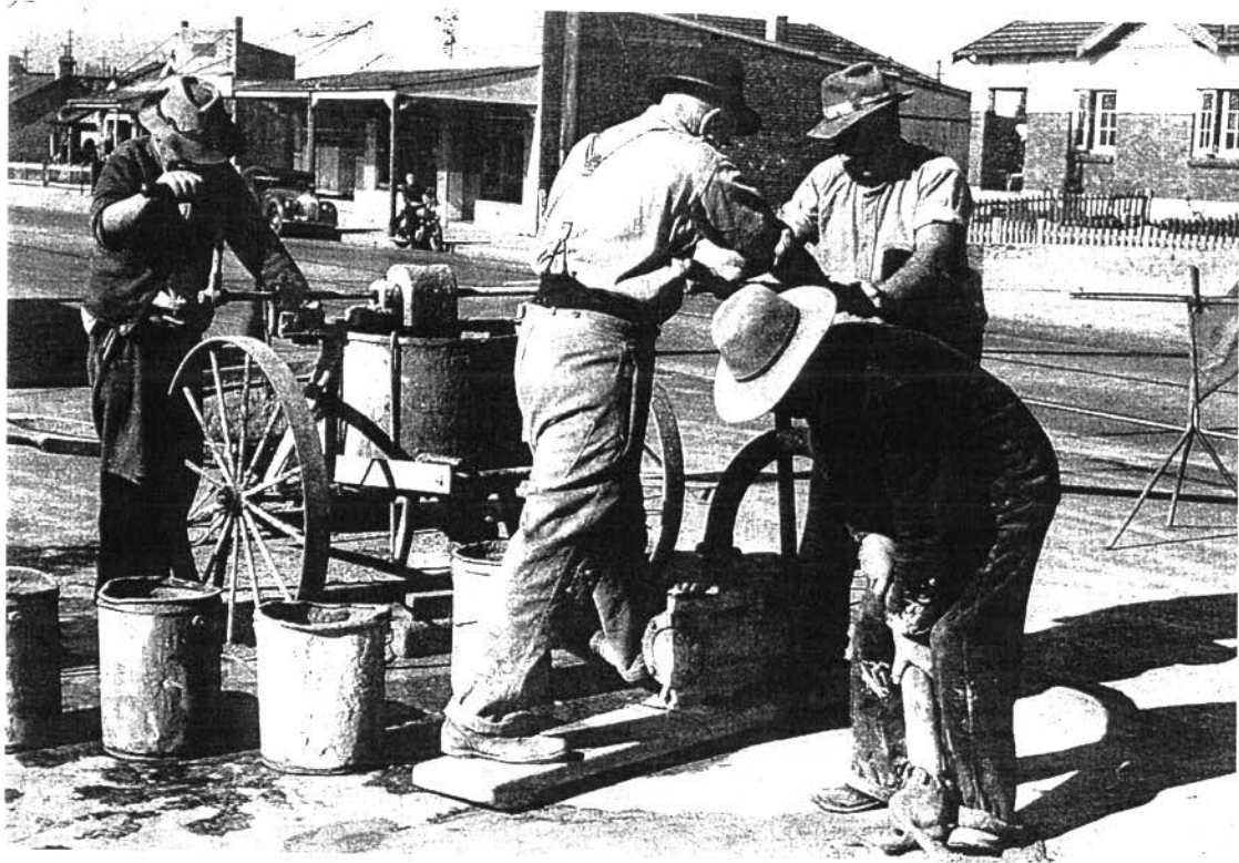
'Raising sunken concrete pavement slabs on Parramatta Road, using the 'Mud-jacking' method, 1949
