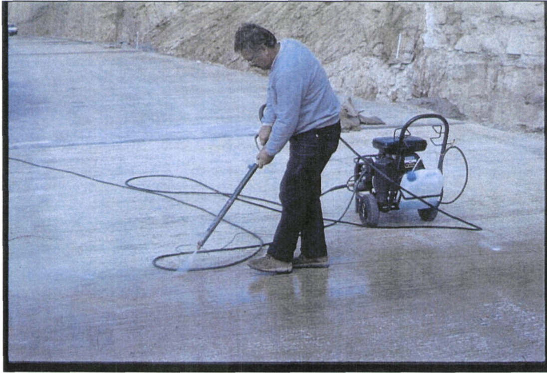
Cleaning a sawn transverse control joint with high pressure water
