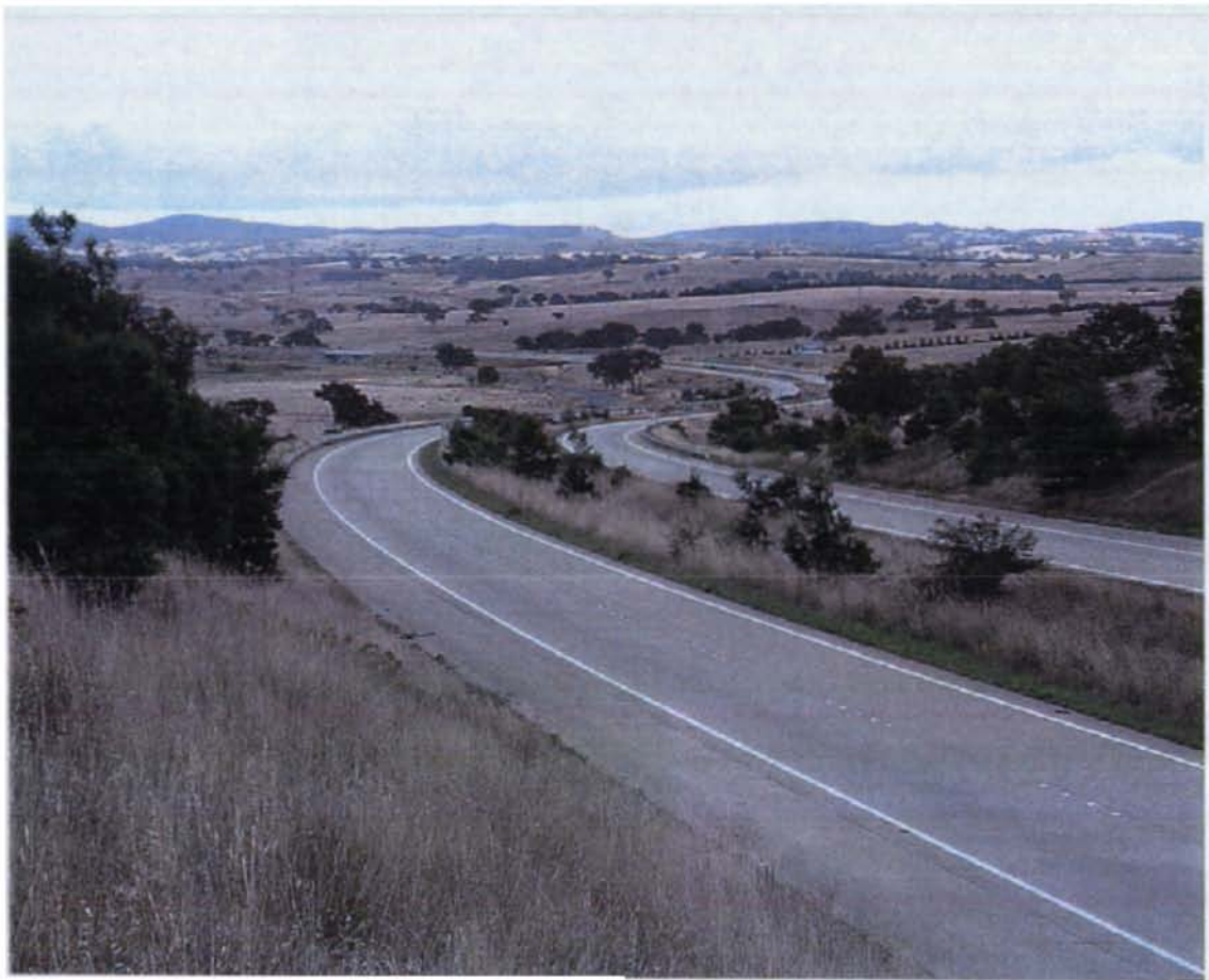
Hume Freeway near Yass, constructed in 1996
