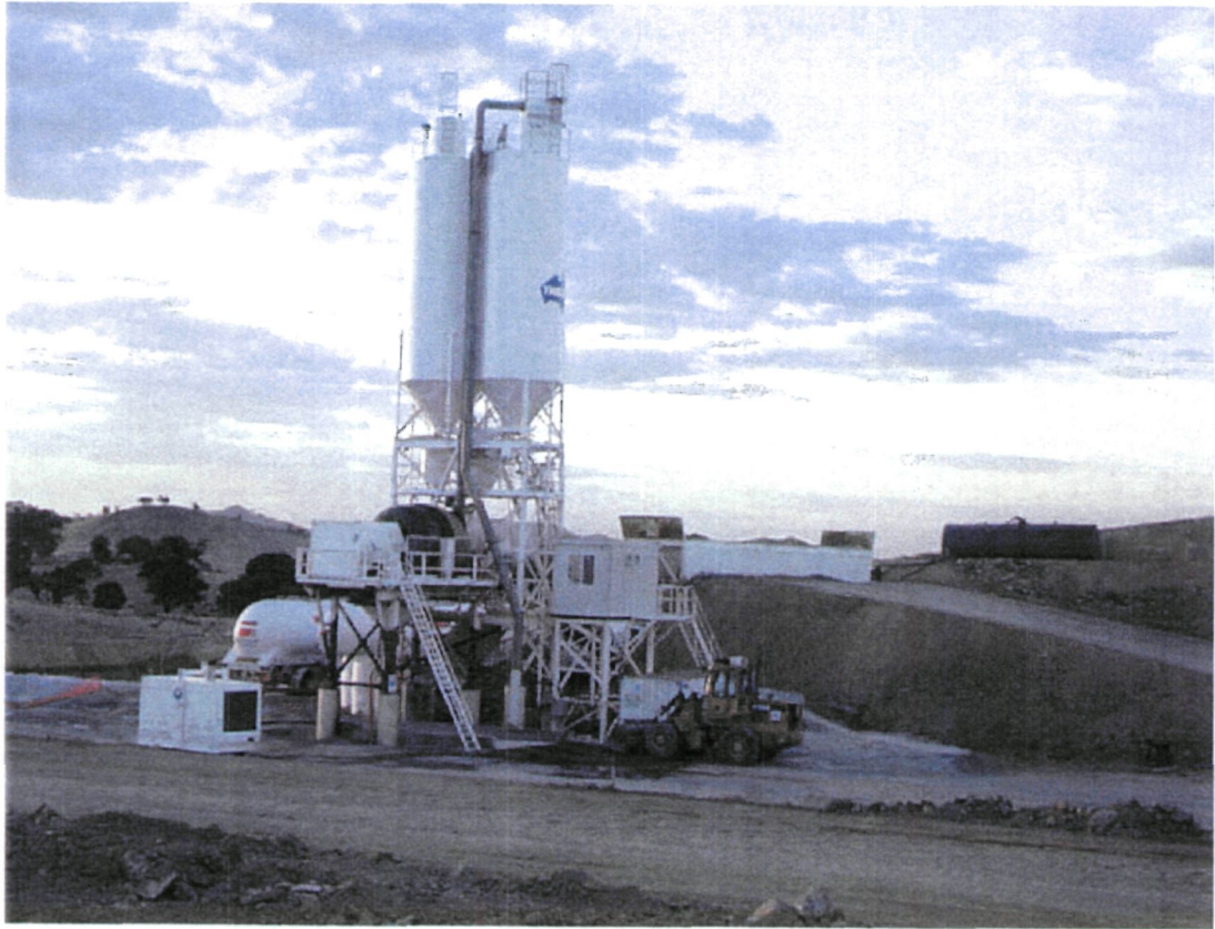
Typical mobile rural concrete production plant
