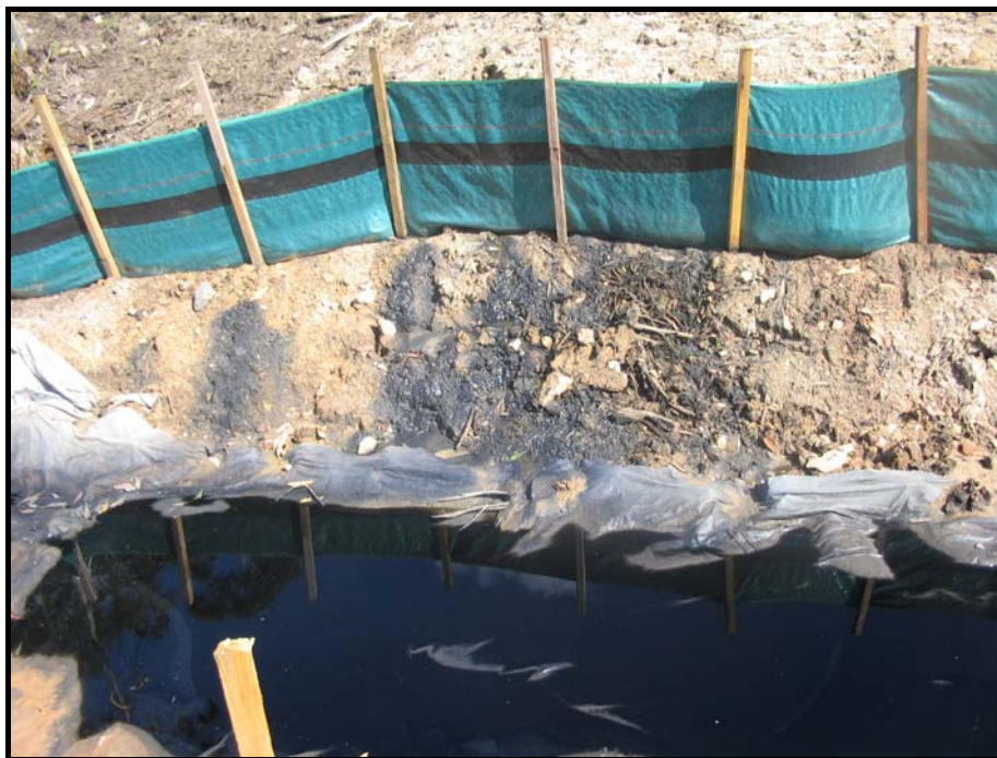
Plate 5: Tannins in a drainage line generated from very thickly applied mulch on the batter above. Note that the sedimentation fence is not effective in treating the tannins.
