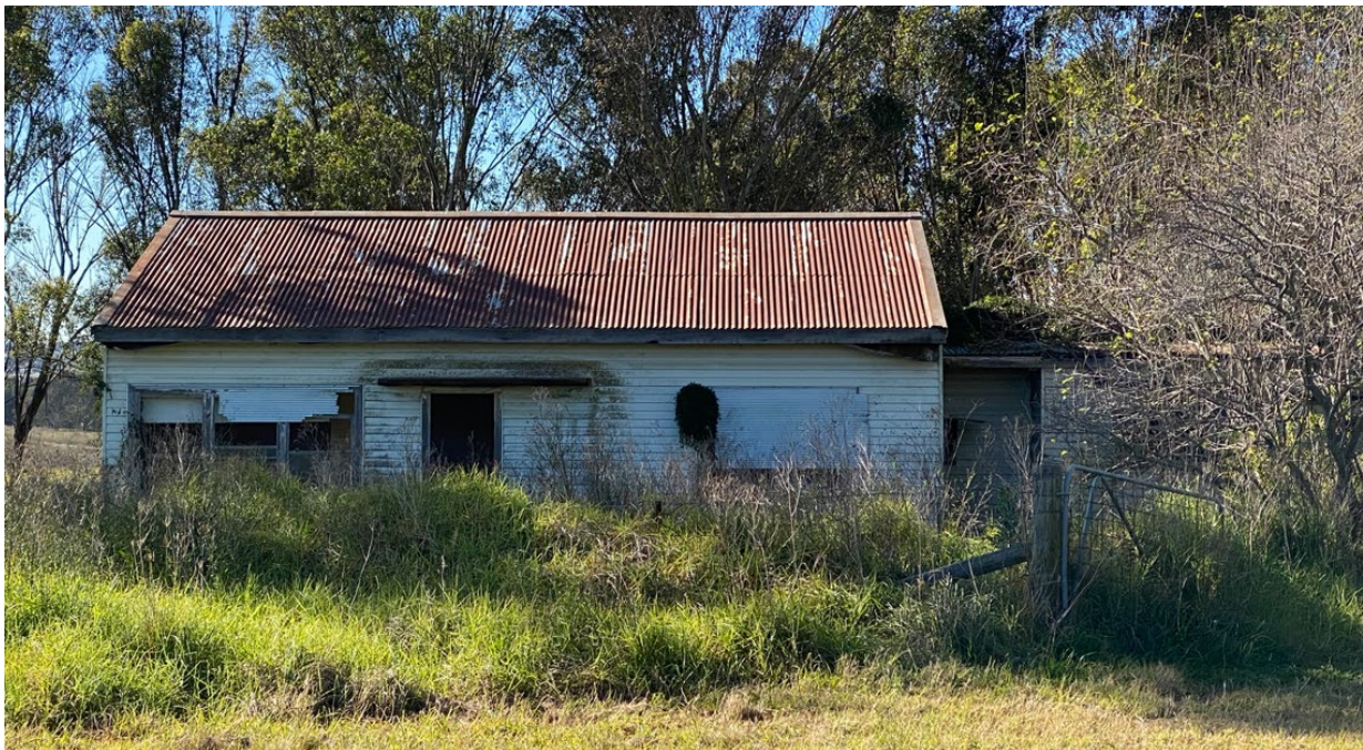
Figure 5-15: McGarvie Smith 10 (AECOM, 2022)
