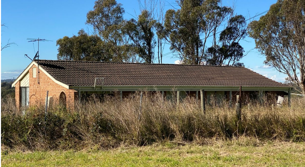
Figure 5-16: McGarvie Smith 11 (AECOM, 2022)
