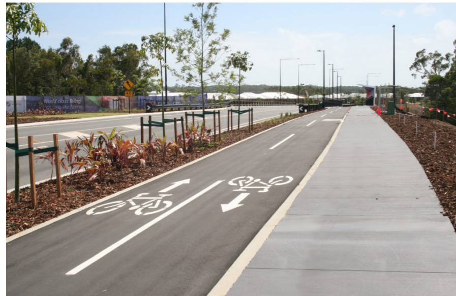
Figure 42: Typical shared path (active travel link) with 3.0m wide bi-directional cycle path and 1.5m wide pedestrian path on both sides of the road corridor
