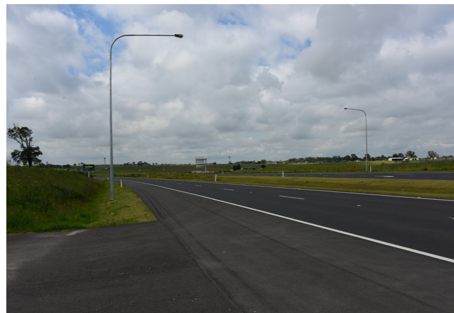
Figure 29: Verges adjacent to other stretches of road are not formally planted
