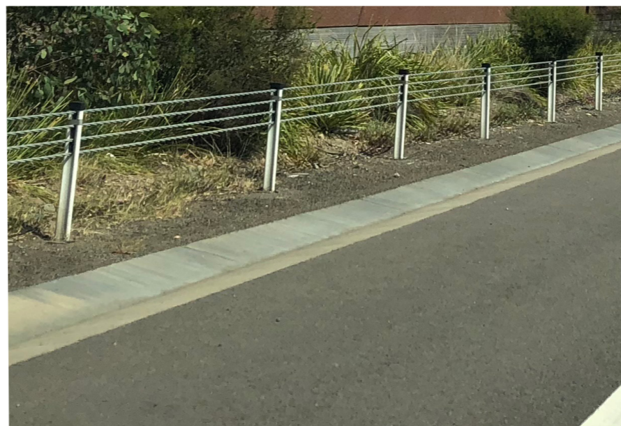
Figure 38: Proposed wire rope barrier along the median
