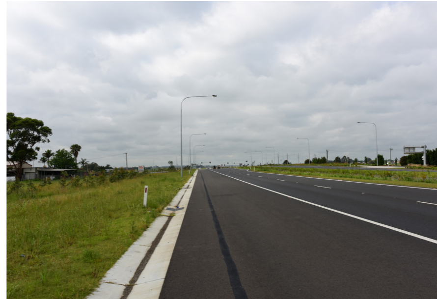
Figure 27: The Northern Road comprises a wide corridor with two lanes and a wide road shoulder in either direction separated by a central median strip
