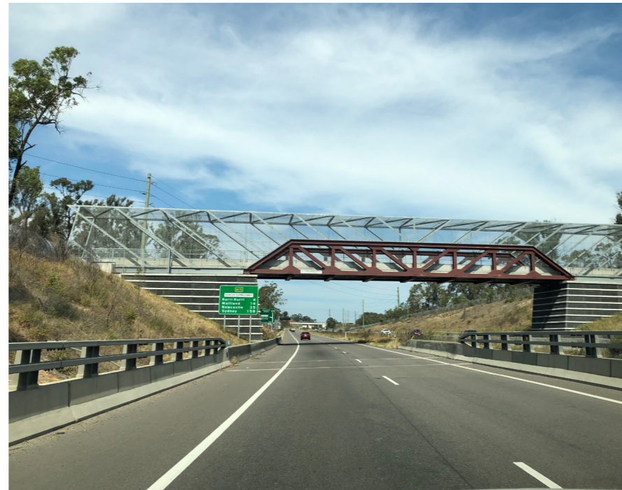
Figure 37: Twin-rail medium performance safety barrier transitioning to type F concrete barrier proposed to Cosgroves Creek Bridge (BR01)
