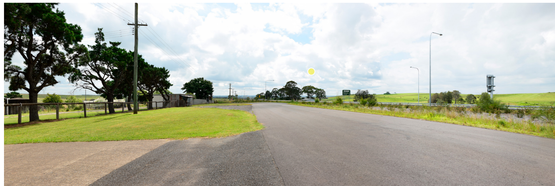
Figure 59: Panorama showing the existing view looking east along Elizabeth Drive from the driveway of 2289 Elizabeth Drive
