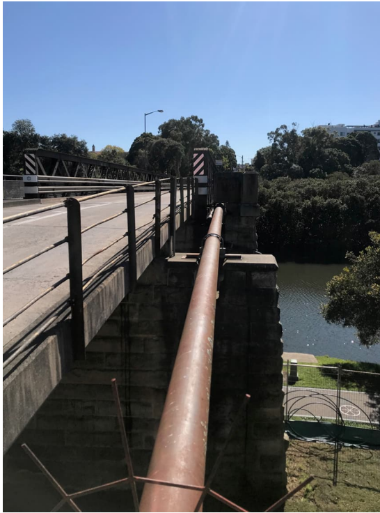
Photo 3-1: Water main facing north
