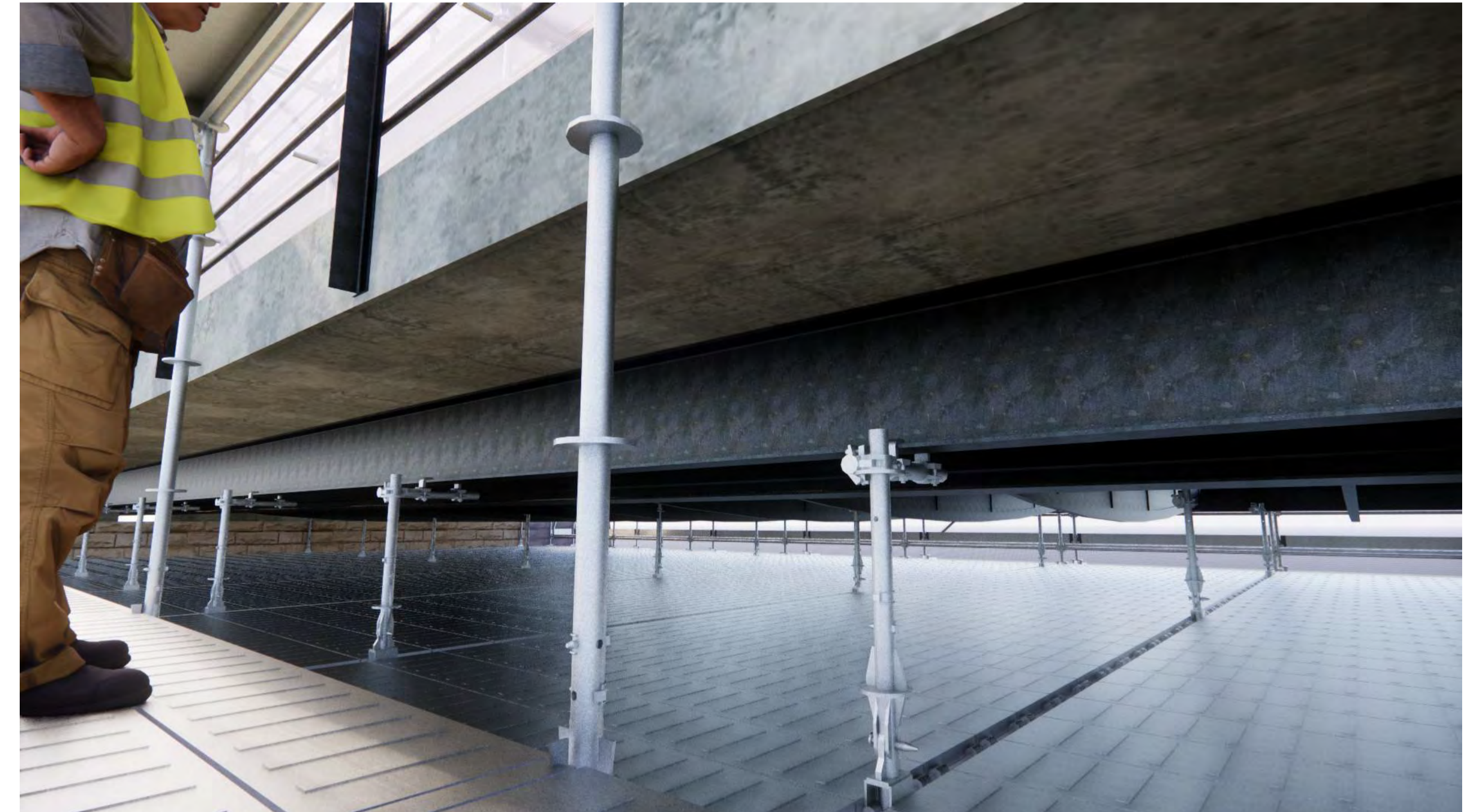
ACCESS PLATFORM UNDER BRIDGE
