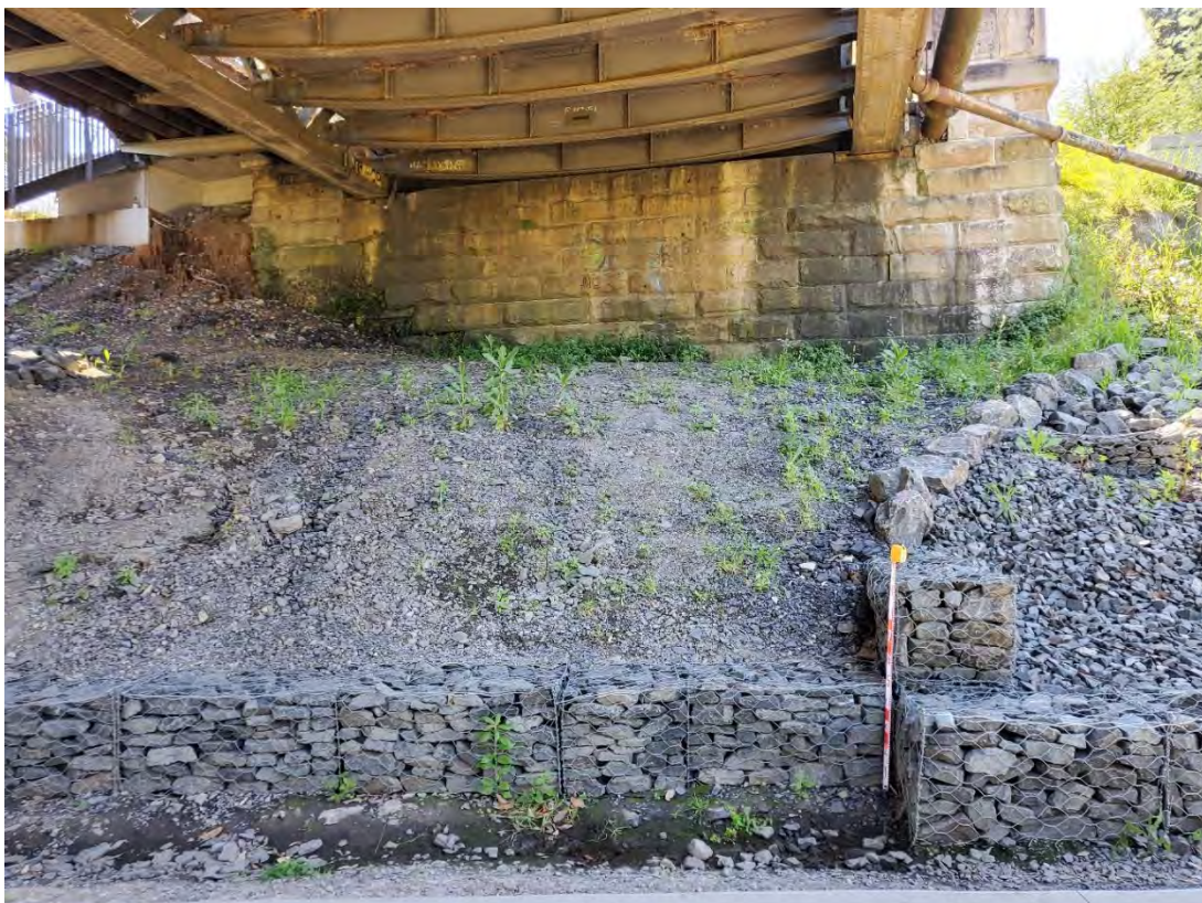
Figure 5.8 North facing view showing northern abutment of bridge.
