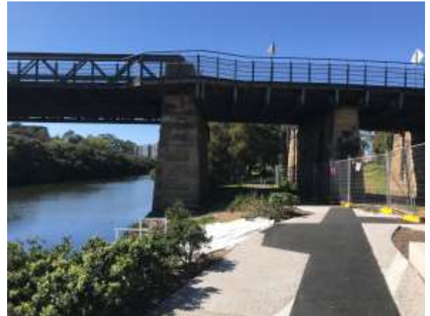
Photo 6-2: Pedestrian routes beneath the Gasworks Bridge – southern side
