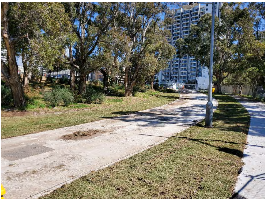
Figure 5.12 South-west facing view showing new road surface and pavement. Note the manhole cover to west (left).
