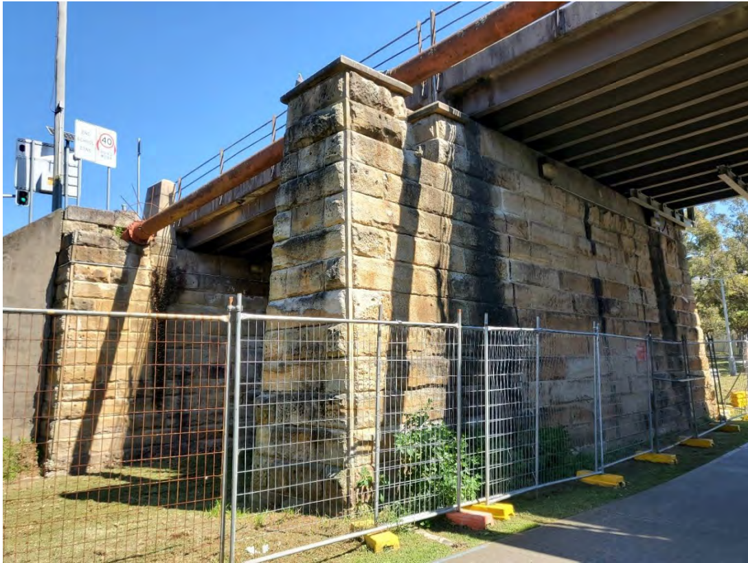
Figure 5.16 South-east view showing southern abutment and piers of bridge.
