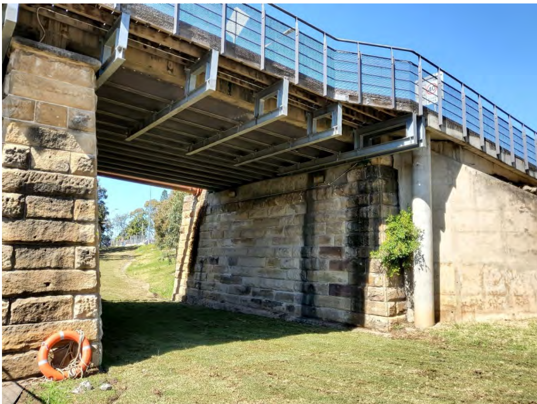
Figure 5.17 South-east view showing southern abutment of bridge and former underpass alignment.
