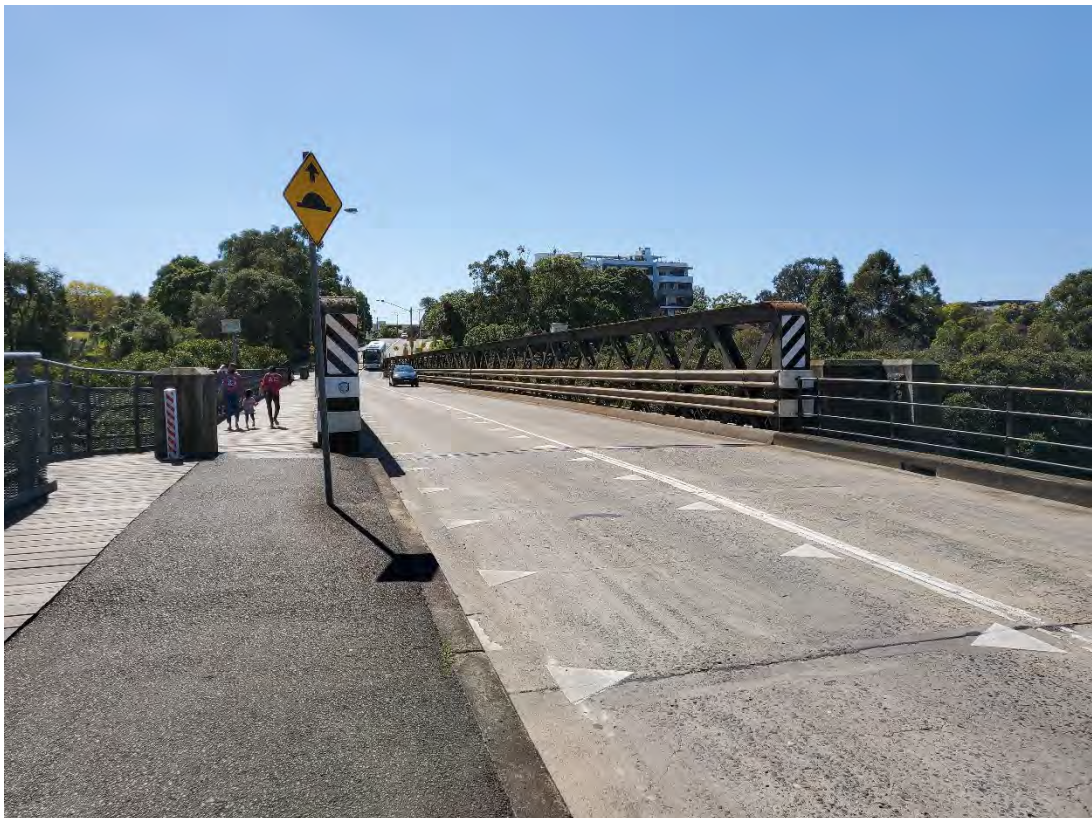
Figure 5.21 North facing view showing southern terminus of bridge.
