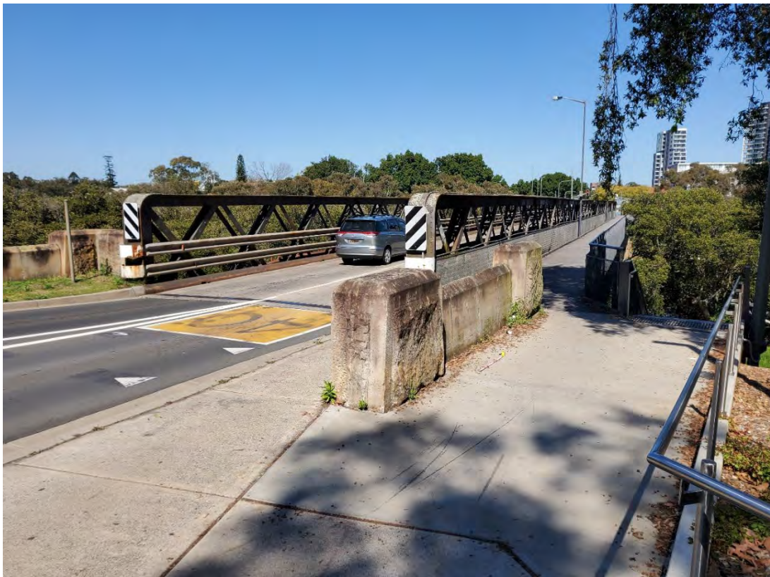
Figure 5.19 South facing view showing northern end of the bridge.
