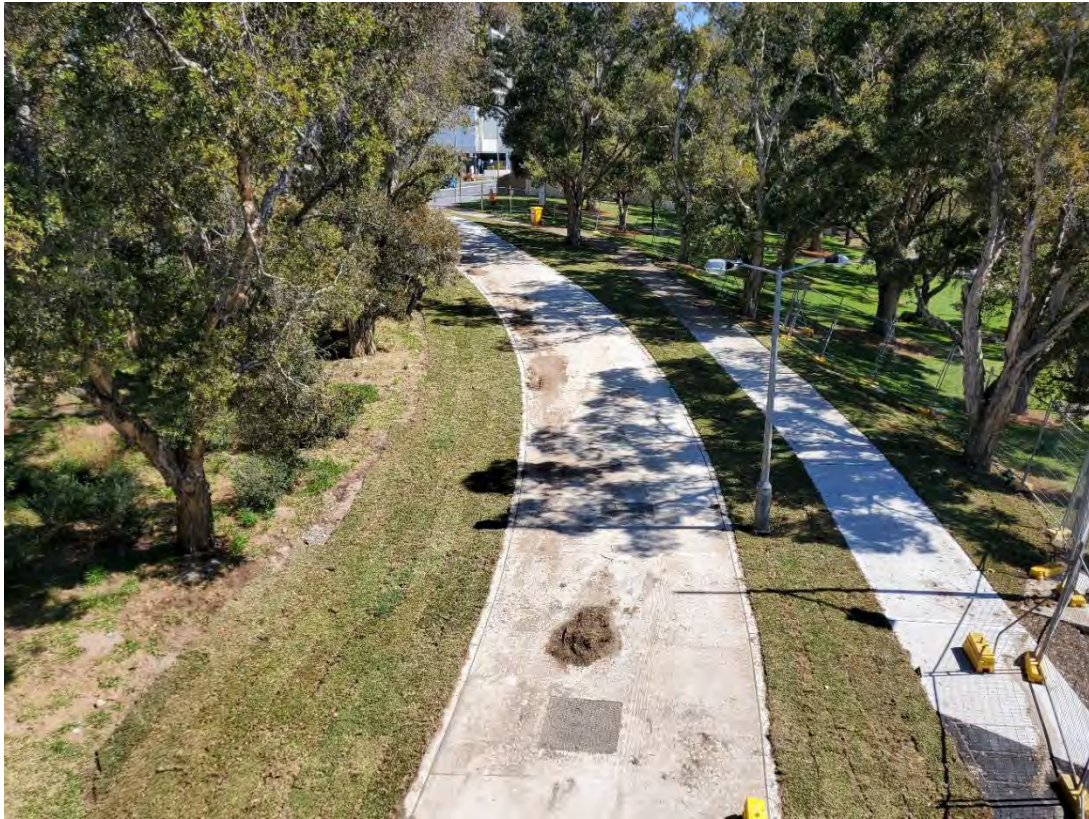
Figure 5.11 West facing view showing proposed laydown area to the west of the bridge.
