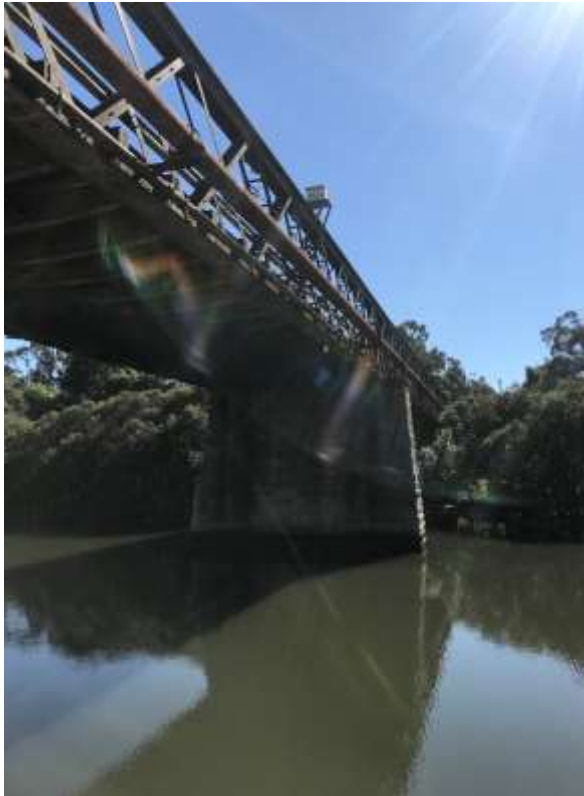
Photo 1-1: Gasworks Bridge, looking north
