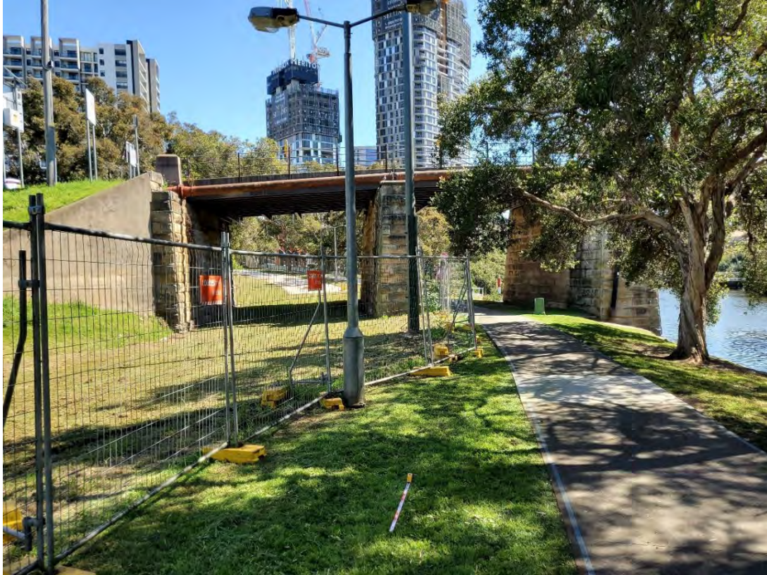
Figure 5.15 West facing view showing approach to southern end of bridge.
