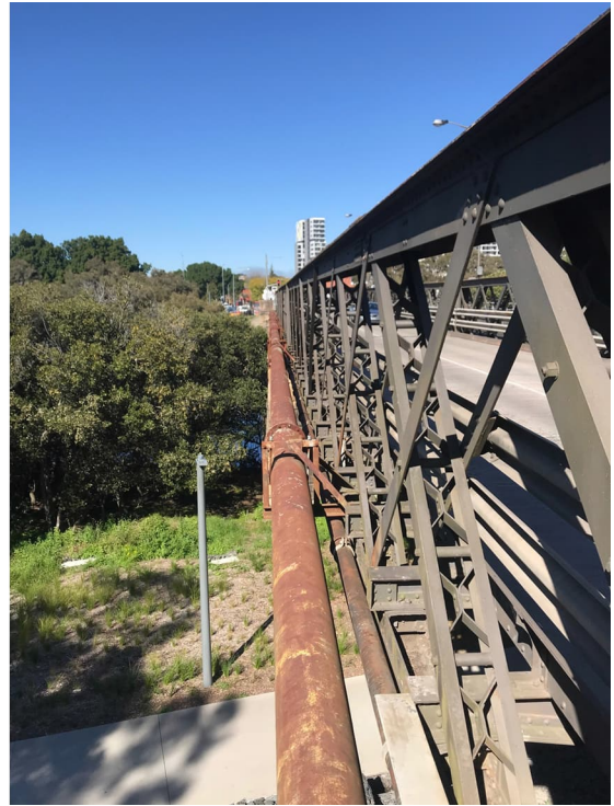
Photo 3-2: Water main facing south
