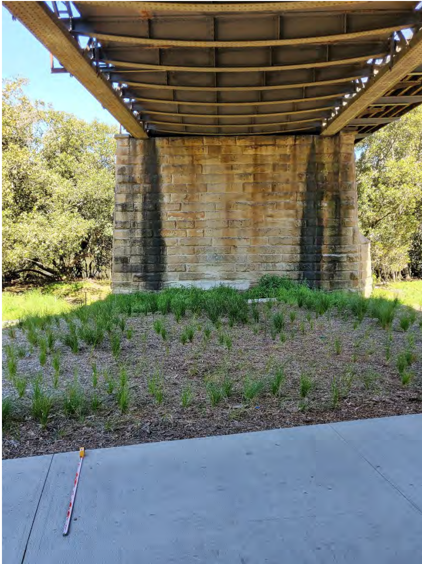
Figure 5.9 South facing view showing underneath of bridge and northern-most pier.
