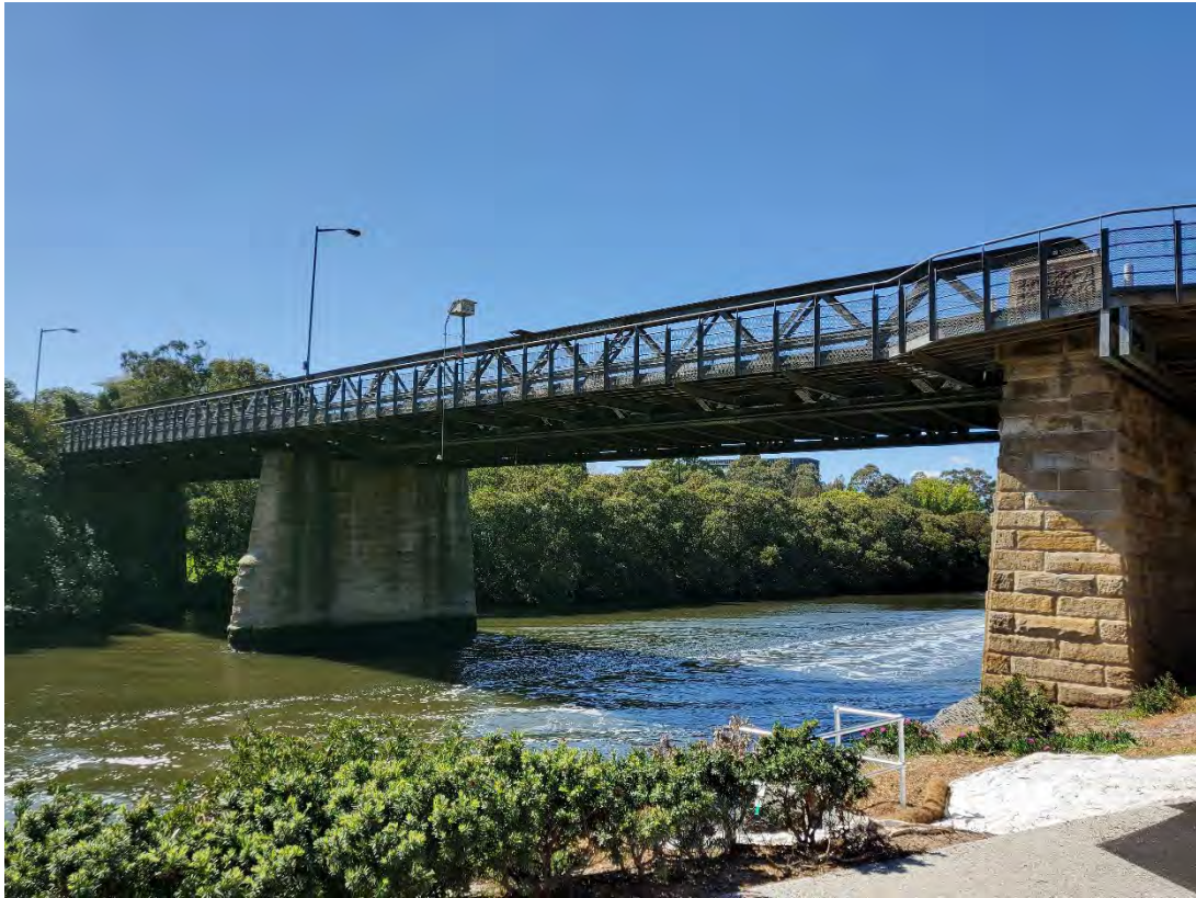
Figure 5.22 East facing view showing western profile of the bridge.
