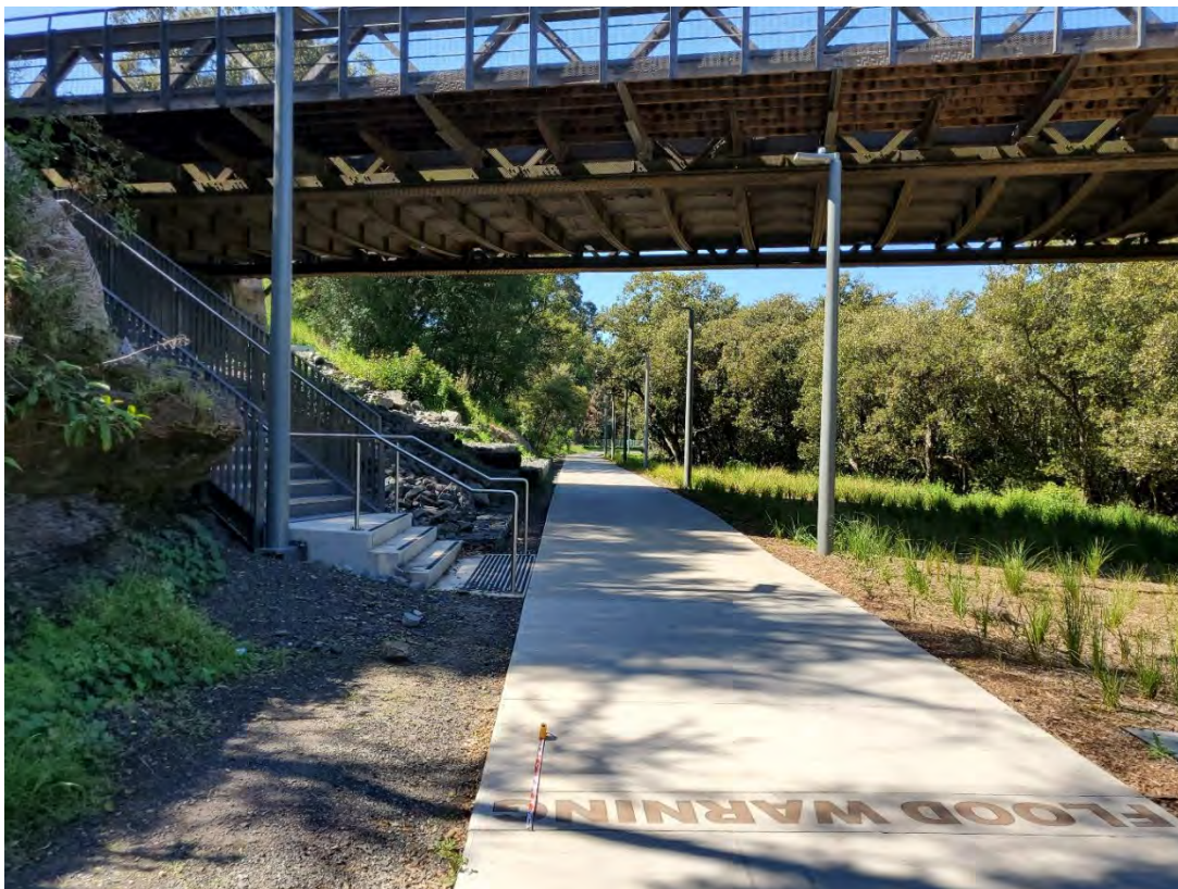
Figure 5.10 East facing view showing the bridge and pedestrian addition, as well as new staircase.
