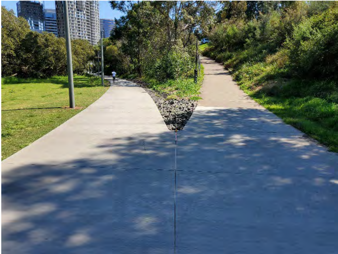
Figure 5.5 West facing view showing junction between upper path and riverside path.
