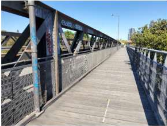
Photo 6-1: Gasworks Bridge shared pathway
