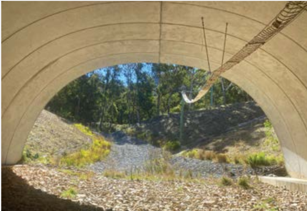
Existing combined drainage culvert and fauna underpass at Whites Creek
