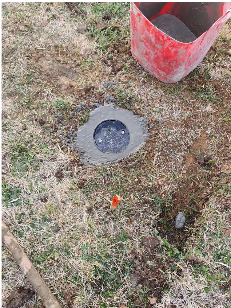
Photograph 6 – Newly installed groundwater well
