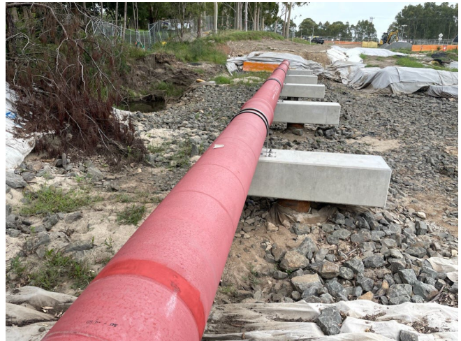
Utility relocation works in progress - February 2023
