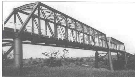
The Luskintyre Bridge (S1)
