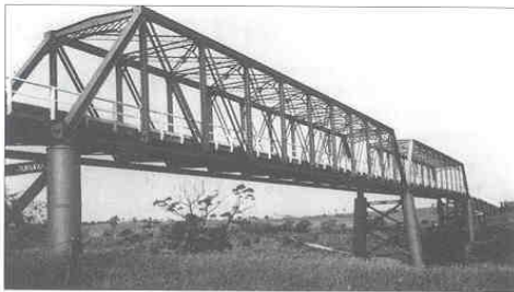
The Luskintyre Bridge (S1)
