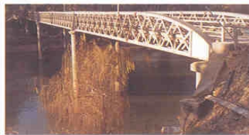
When McMillan, Britton & Kell were contracted to duplicate the bridges at Aberdeen (I5), they chose to match the appearance of the 1893 lattice bridge (right) with a welded Warren truss completed in 1986.
