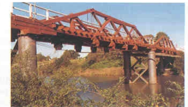
One of the oldest PWD timber truss bridges, Clarendontown Bridge (O1)
