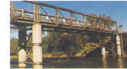
A typical DeBurgh truss
