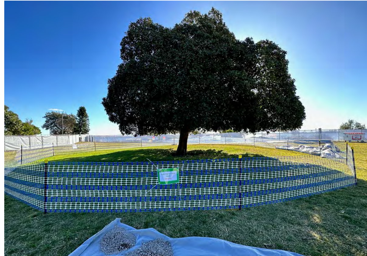
Tree protection installed
