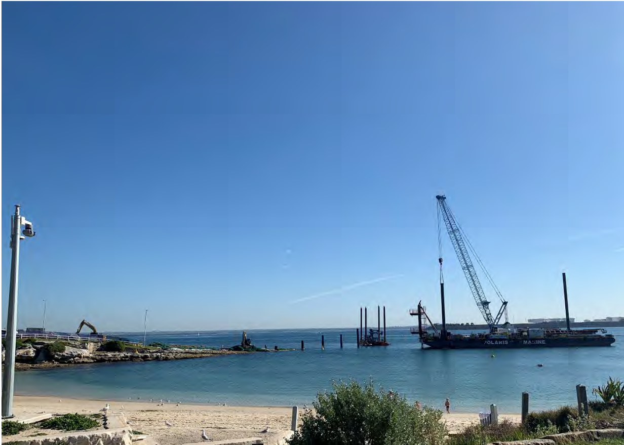
View of the piling equipment from Frenchmans Bay
