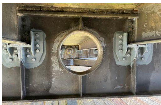
Installed steel brackets and bolts
