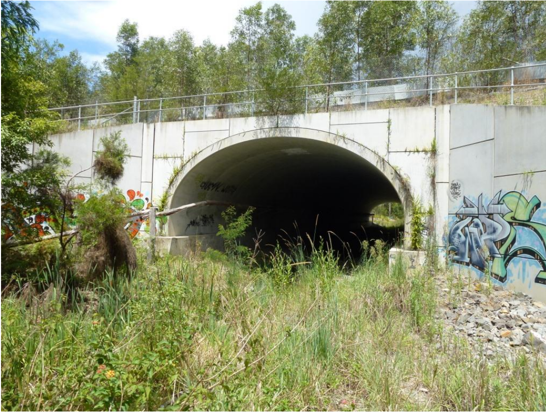
Plate 1: Boat Harbour Creek Underpass
