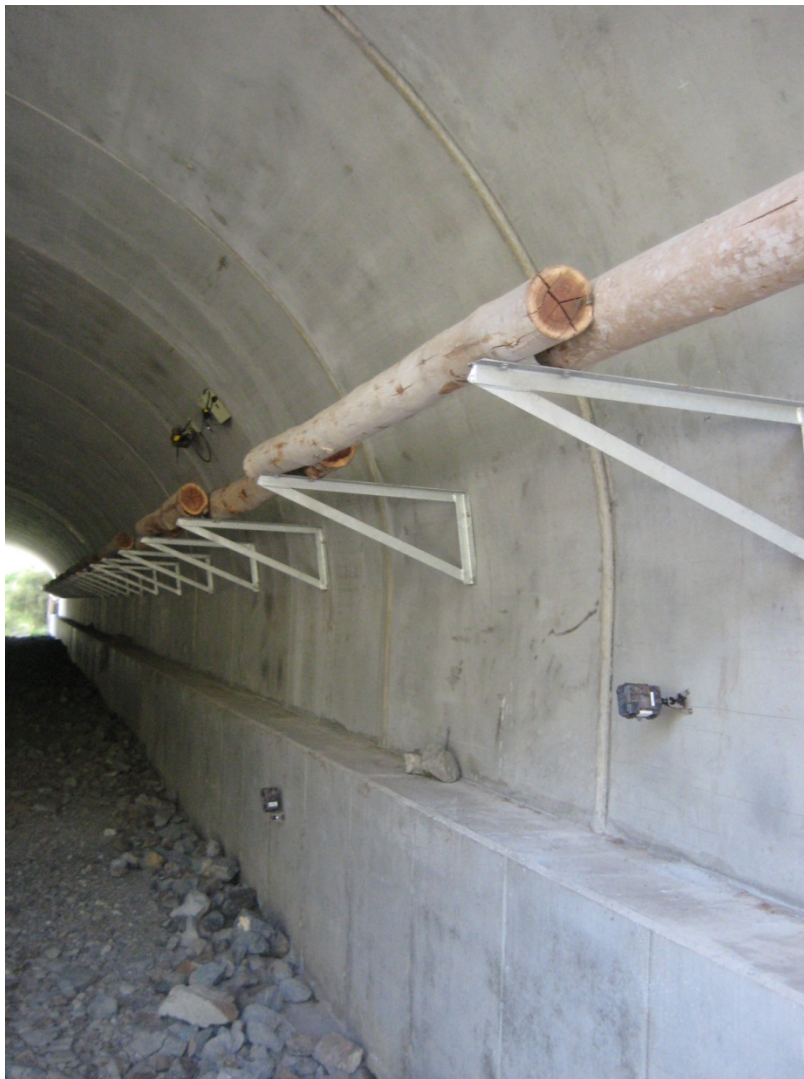
Photograph 2.1 West Side of Boat Harbour Creek Showing Three Cameras Trained on the Ground, Concrete Bench and Fauna Furniture
