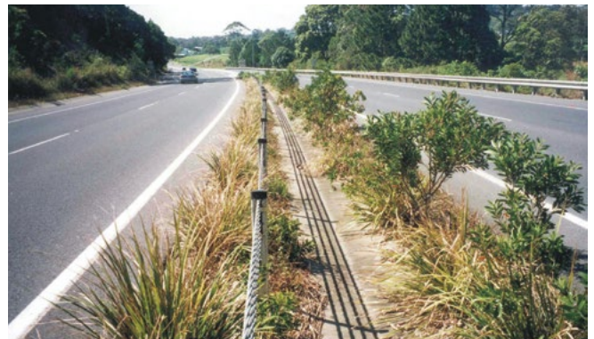
This median is not wide enough for this type of landscape treatment and the result is visually poor and hard to maintain. A simple turf strip or paved surface would be preferable.
