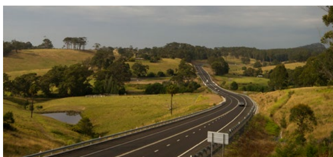
Simple, ecologically benign, low maintenance road reserve design with a two metre wide mown verge adjacent to the carriageway. Note that natural regeneration has resulted in vegetation within the clear zone which if non-frangible would need to be removed.
