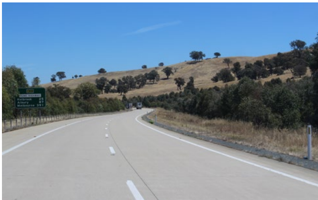
Simple native shrub and tree tubestock plantings in seeded pasture grasses provided in wide, grade-separated median and cuttings, six years after planting.
