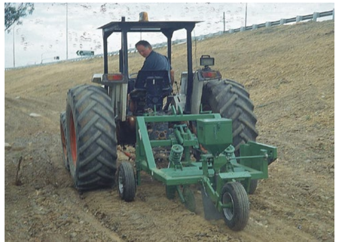
Tractor seeding on a batter shallower than a 3:1 slope.
