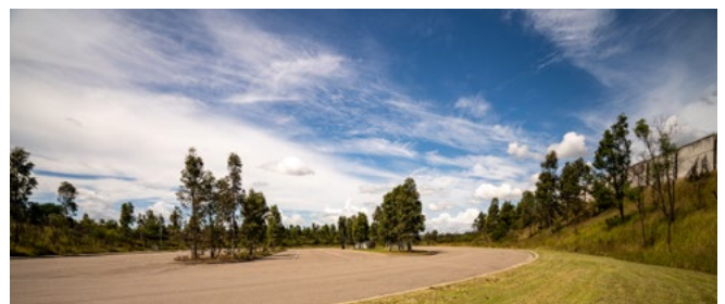
Heavy vehicle rest area on the Hunter Expressway shortly after completion and 8 years later. The batters (cuttings and embankments) vary in grade from 4H:1V to 2H:1V. There has been a good plant growth and the area is appropriately secluded.
