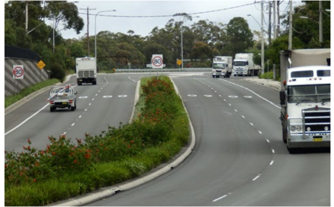
Example of safe planting in the median clear of non-frangible hazards and with open sightlines at bends and intersections.
