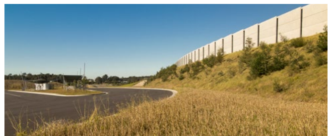
Space for vegetation at the base of the cutting improves the appearance of the cutting and helps stop debris from the cut reaching the carriageway.
