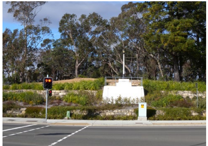
The opportunity exists to provide something special to enliven the journey. This should not be overdone and the design must address future maintenance issues. Areas of gravel should be carefully considered as the constant removal of weeds is required, generally by chemical means.
