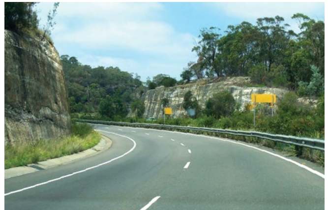
Space for vegetation at the base of the cutting improves the appearance of the cutting and helps stop debris from the cut reaching the carriageway.
