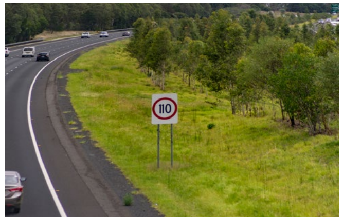
Trees set over 10m from the edge of the travel lane of the carriageway on the Hume Highway.
