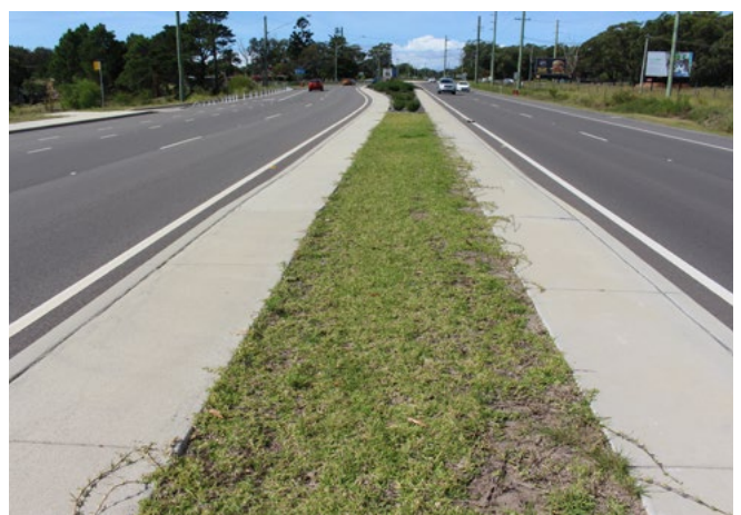
A grass sward is an appropriate finish to a narrow median. It is sufficient to provide relief to the expanse of bitumen in the road user view, however in this case is too narrow and poses maintenance problems.
