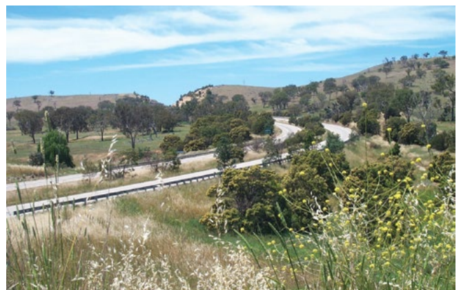
The design of this road helps restore the landscape and blends the road corridor into the adjacent context by continuing vegetation patterns and local species across the road reserve and median.
