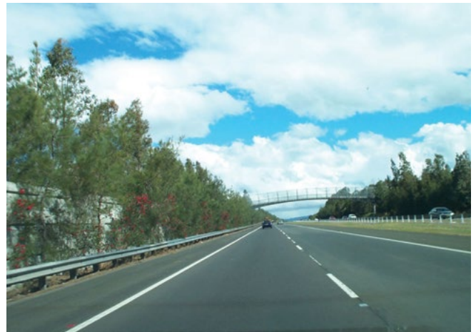
Smaller frangible shrubs such as bottlebrush help filter views of the wall and provide a greener corridor than would otherwise be achieved.
