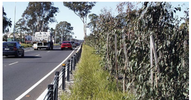
Dynamic deflection zones must be maintained behind the safety barrier.
