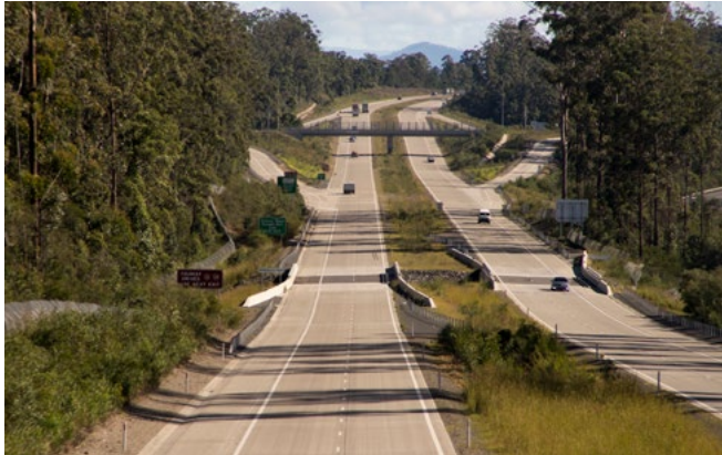
Frederickton to Eungai median – Median revegetated with grasses, groundcovers and frangible shrubs through both seeding and planting to suit the longitudinal alignment.
