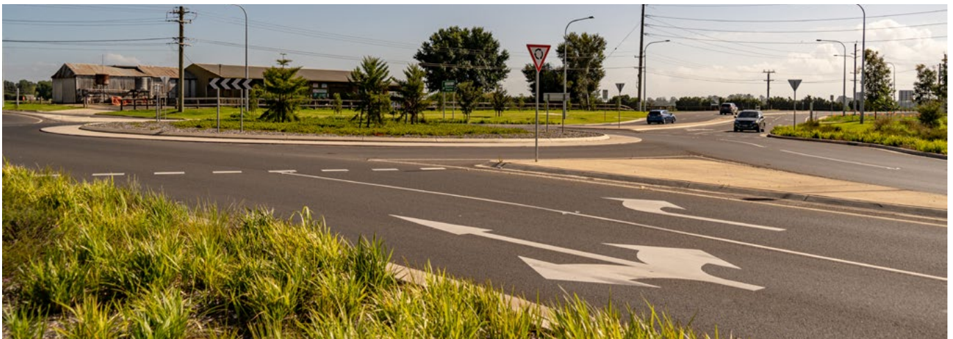
Roundabout in Windsor helping signal the town ahead and integrated with the project landscape design.
