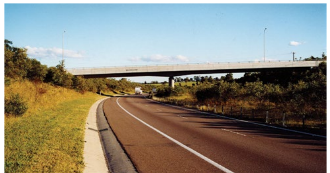
The clear zone varies for different speed roads. Slower speed urban roads (upper) have narrower clear zones than high speed rural roads (lower).
