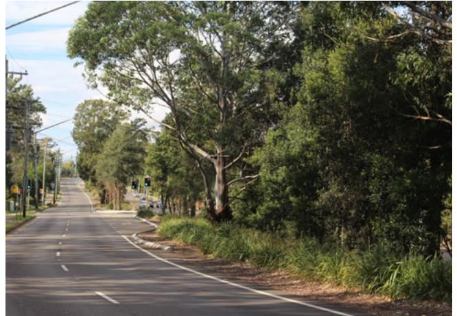
Simple planting of groundcovers creates an attractive and safe median that does not obscure safe sight distances.
