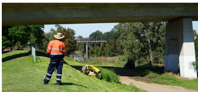
Emerging technology such as this remote control mower may inherently improve safety of maintenance activity on our corridors.
