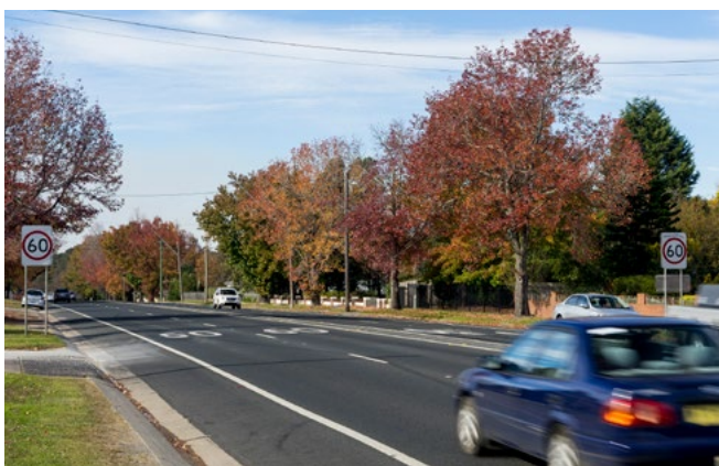
Deciduous trees planted at the edge of the clear zone mark the approach to a town and provide a distinctive milestone. The same approach could also be used at intersections providing access to local towns along freeways and highways.
