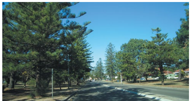
The setback of trees should vary for different speed roads. Higher speed rural roads need a greater setback for trees than lower speed urban roads.
