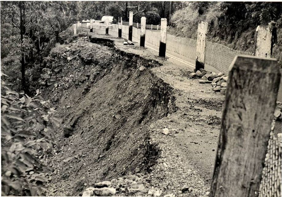
Embankment failure, 1940
