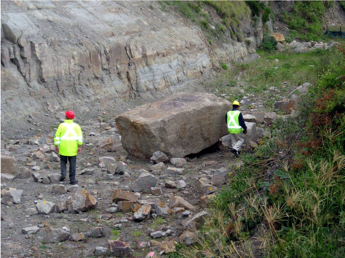
40-tonne rock which fell into the ditch, 2002
