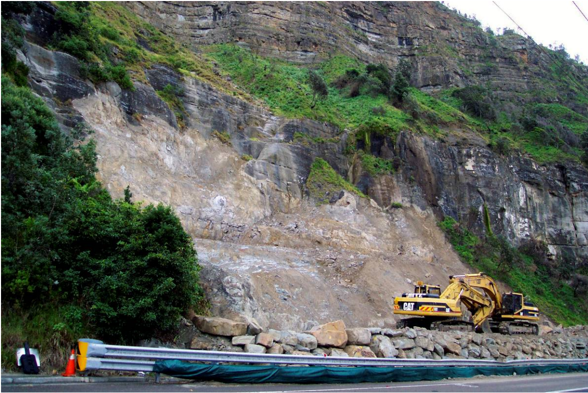
Construction of berm, 2002
