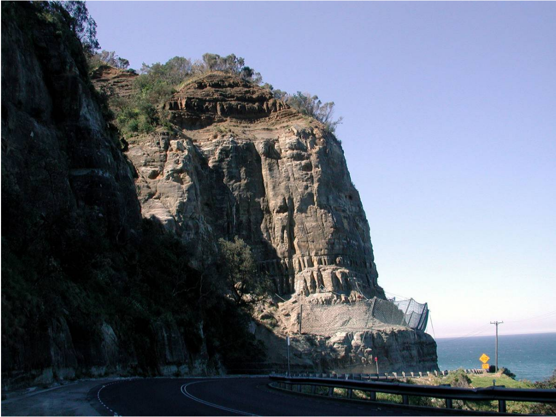
Geobrugg fence around headland, August 2002
