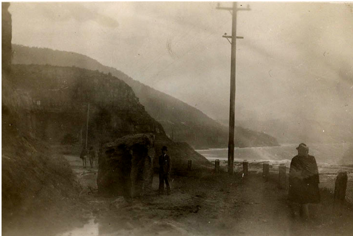
Very large rock fall, Lawrence Hargrave Drive 1949
