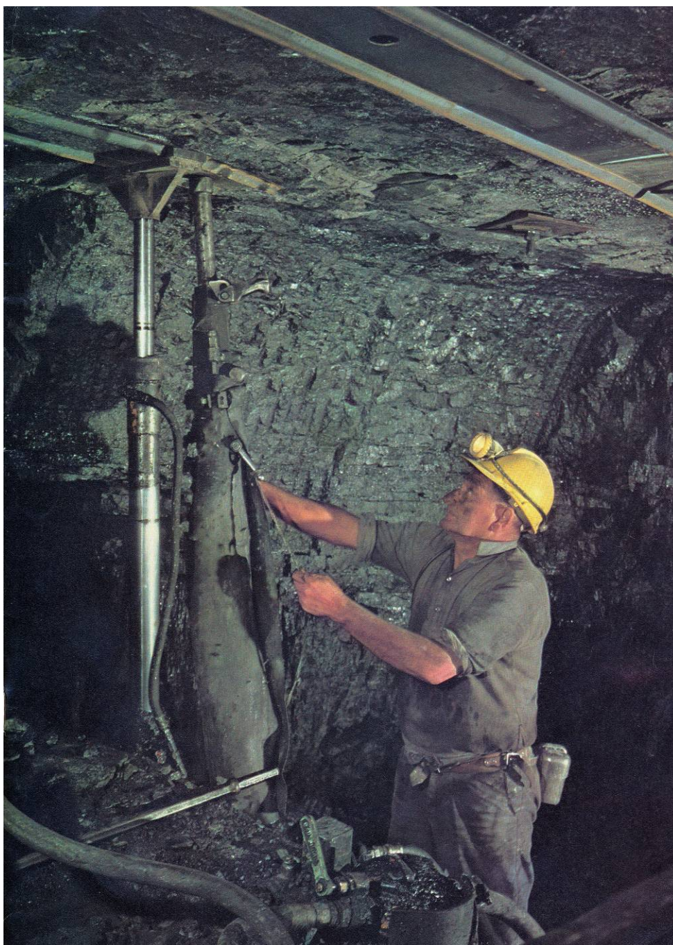
Rock bolting in the mine at Coalcliff, 1970s.
