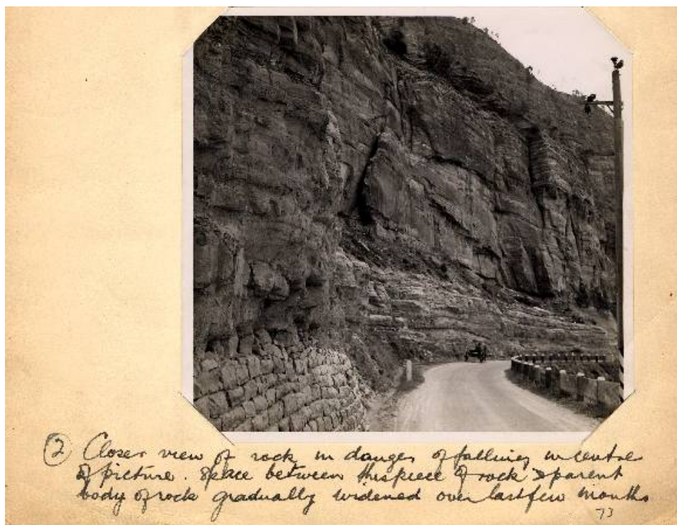
Lawrence Hargrave Drive, 1947 (Source: DMR files)
