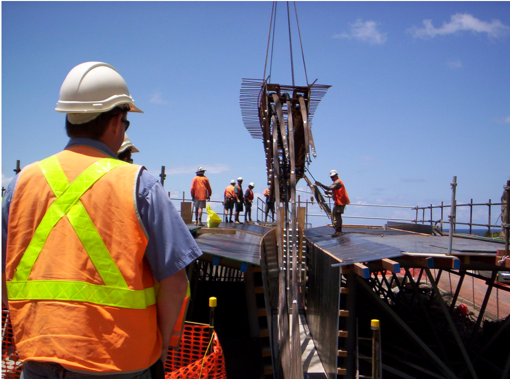
Placing reinforcement for the first deck section in the casting yard
