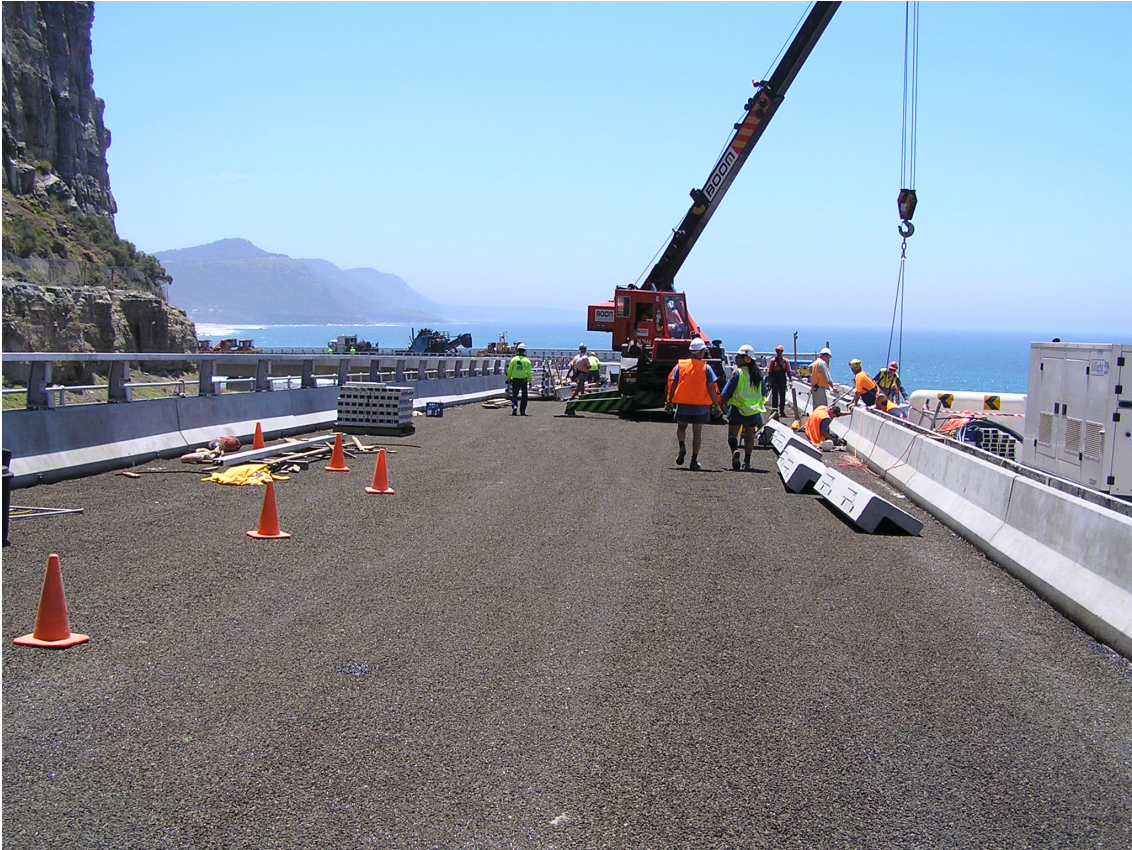
Kerb and railing placement
