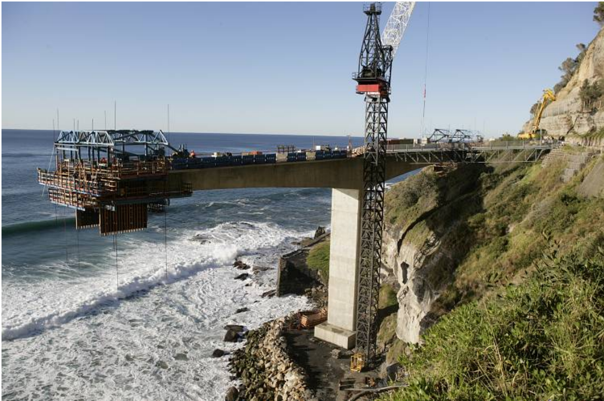
Southern balanced cantilever bridge nearing completion (Pier D)
