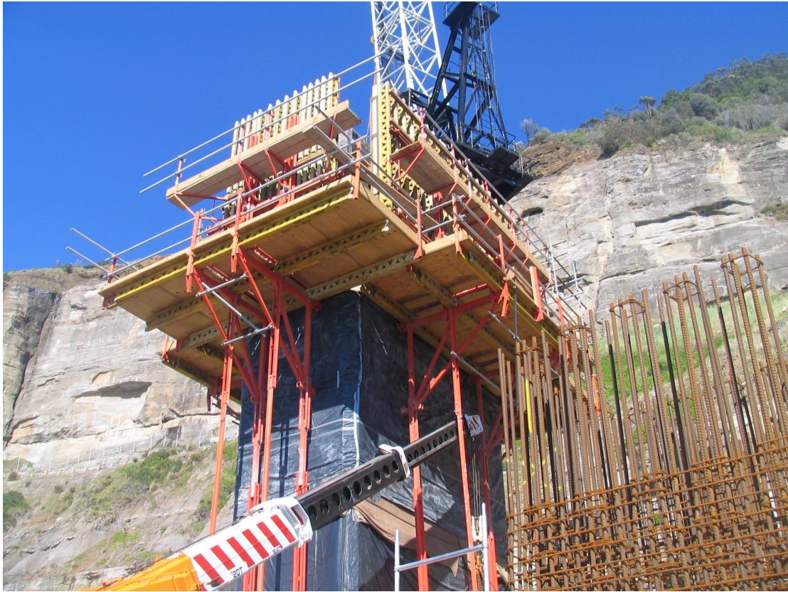
Pier almost complete
