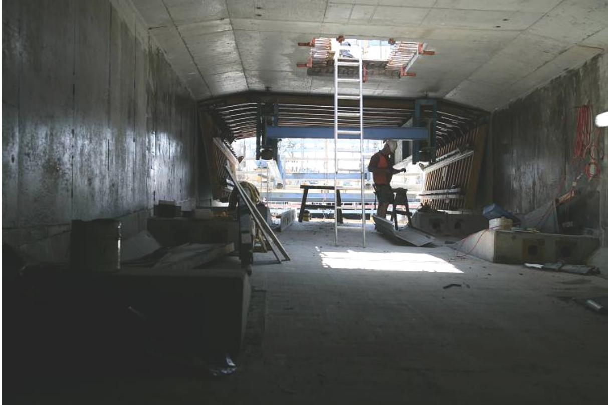
Inside the span
