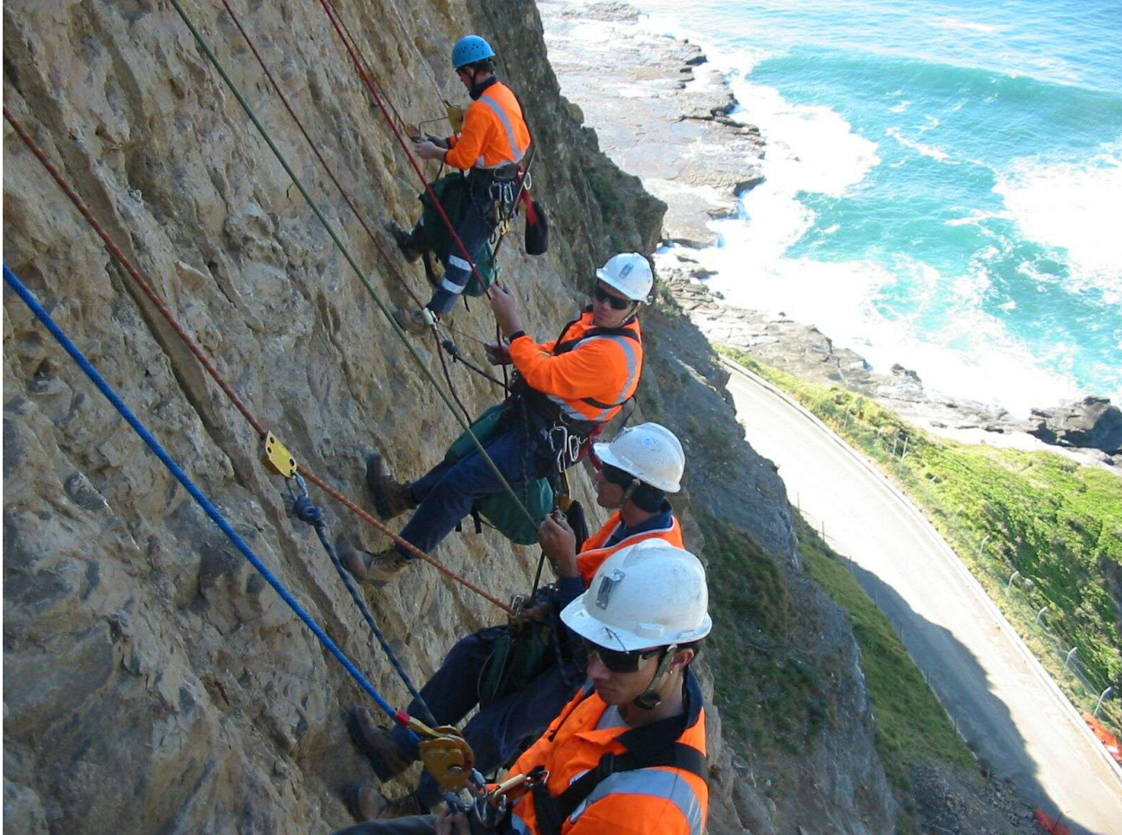
Cliff stabilisation works
