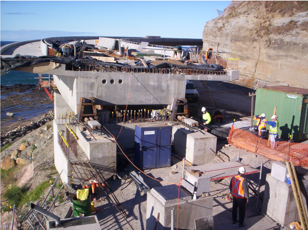
Northern incrementally launched bridge – jacking almost complete
