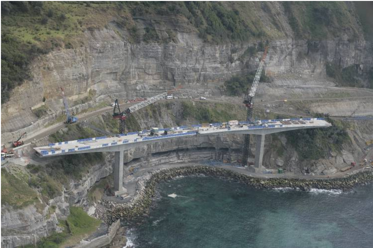
Southern balanced cantilever bridge
