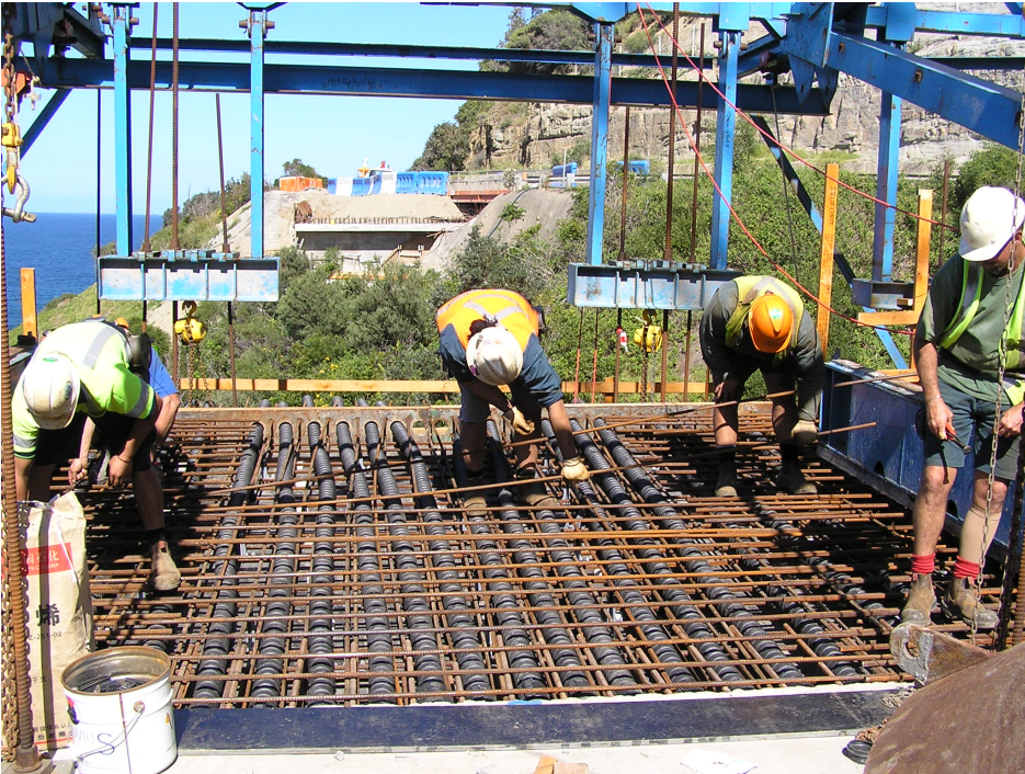
Placing reinforcement
