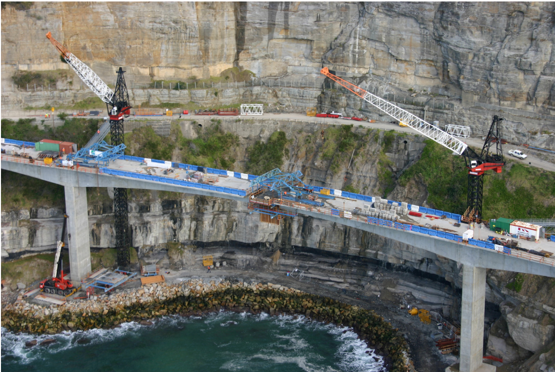
Pier D (on left) complete and traveller being dismantled
