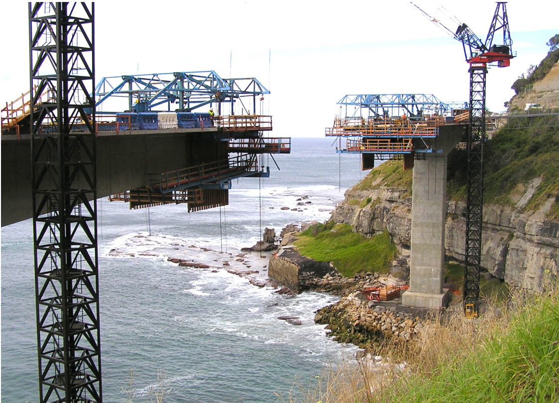
Balanced cantilever bridge spans approaching
