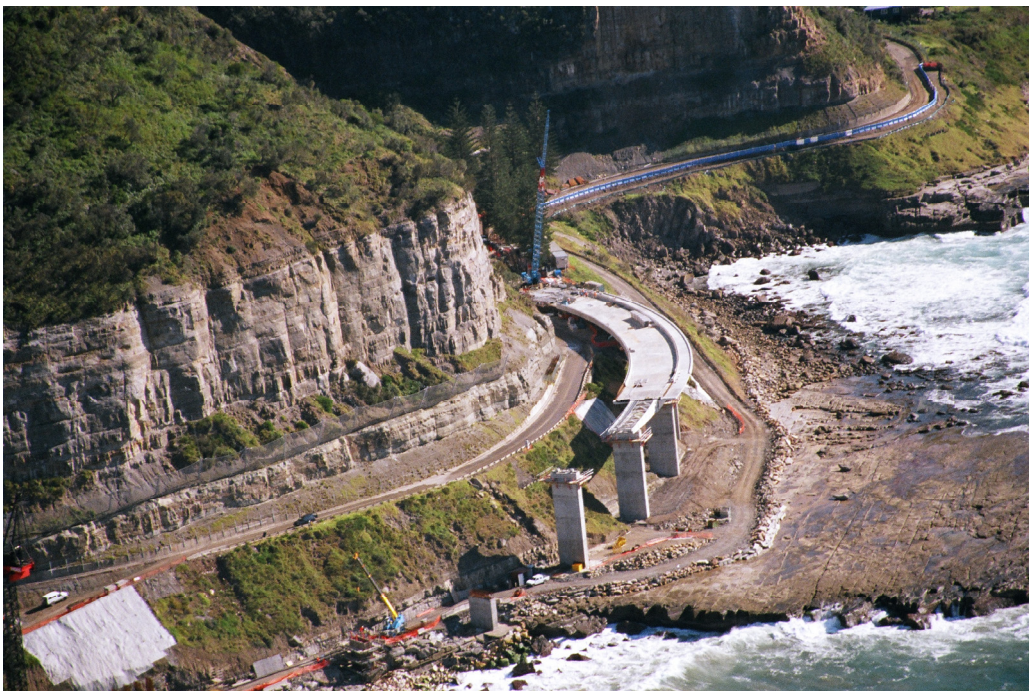
Overhead view of northern incrementally launched bridge
