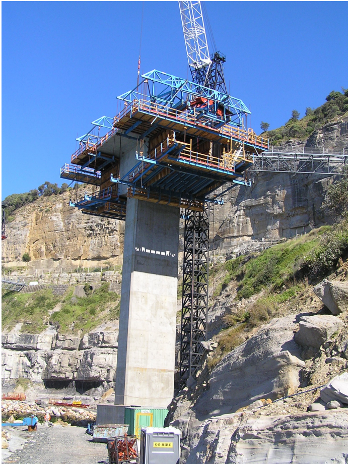
Pier C - travellers in place
