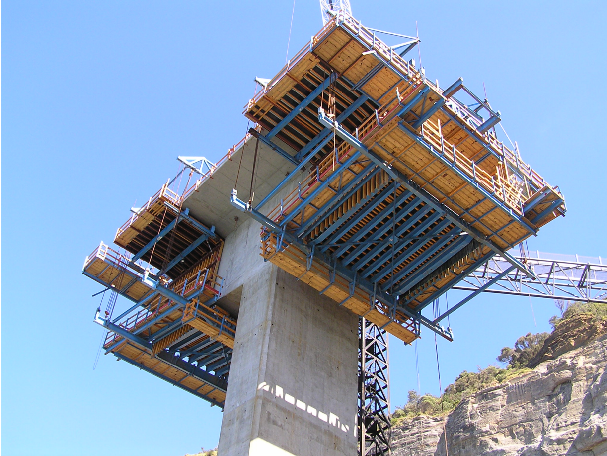
Commencement of balanced cantilever bridge spans
