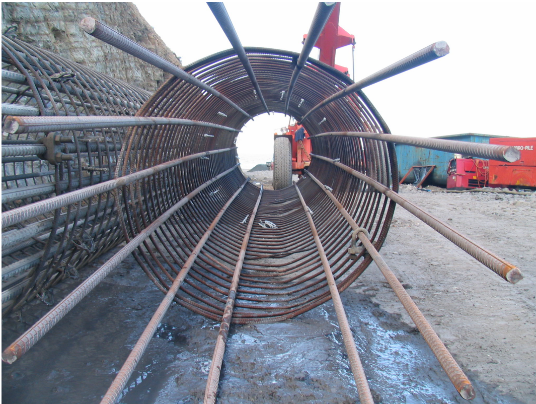
Pile reinforcement prior to placement into bored pile
