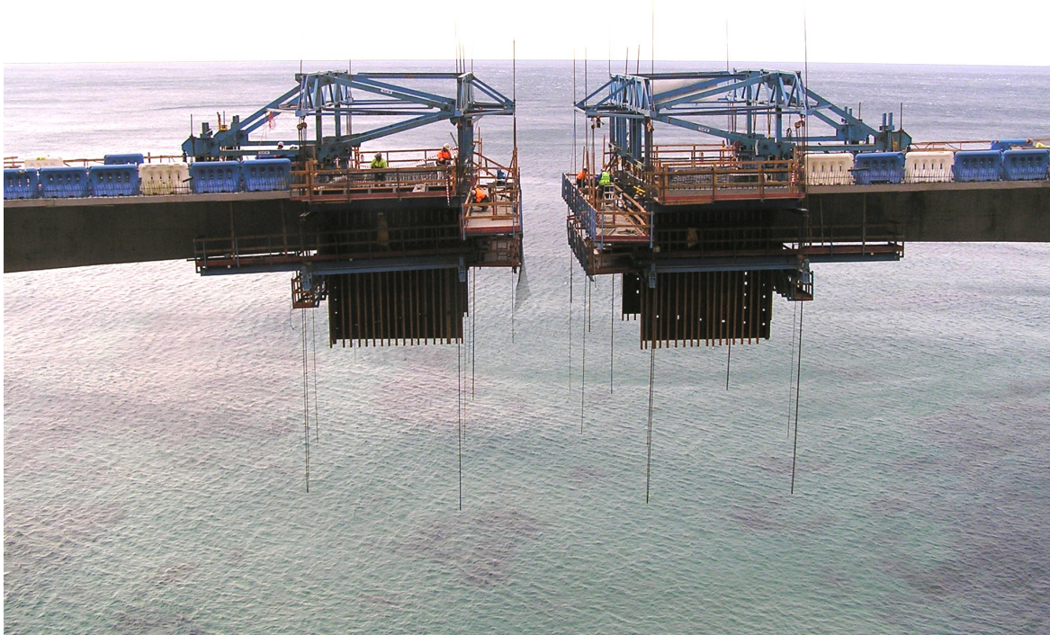
Balanced cantilever bridge spans about to meet
