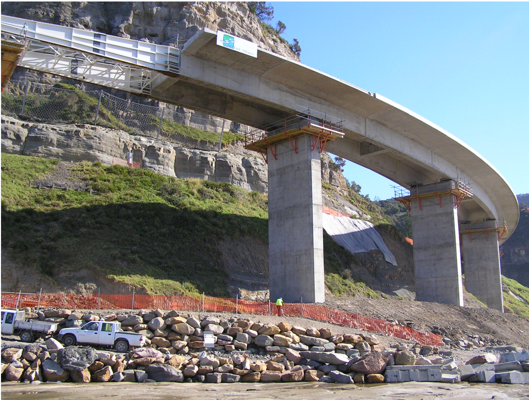
Northern incrementally launched bridge
