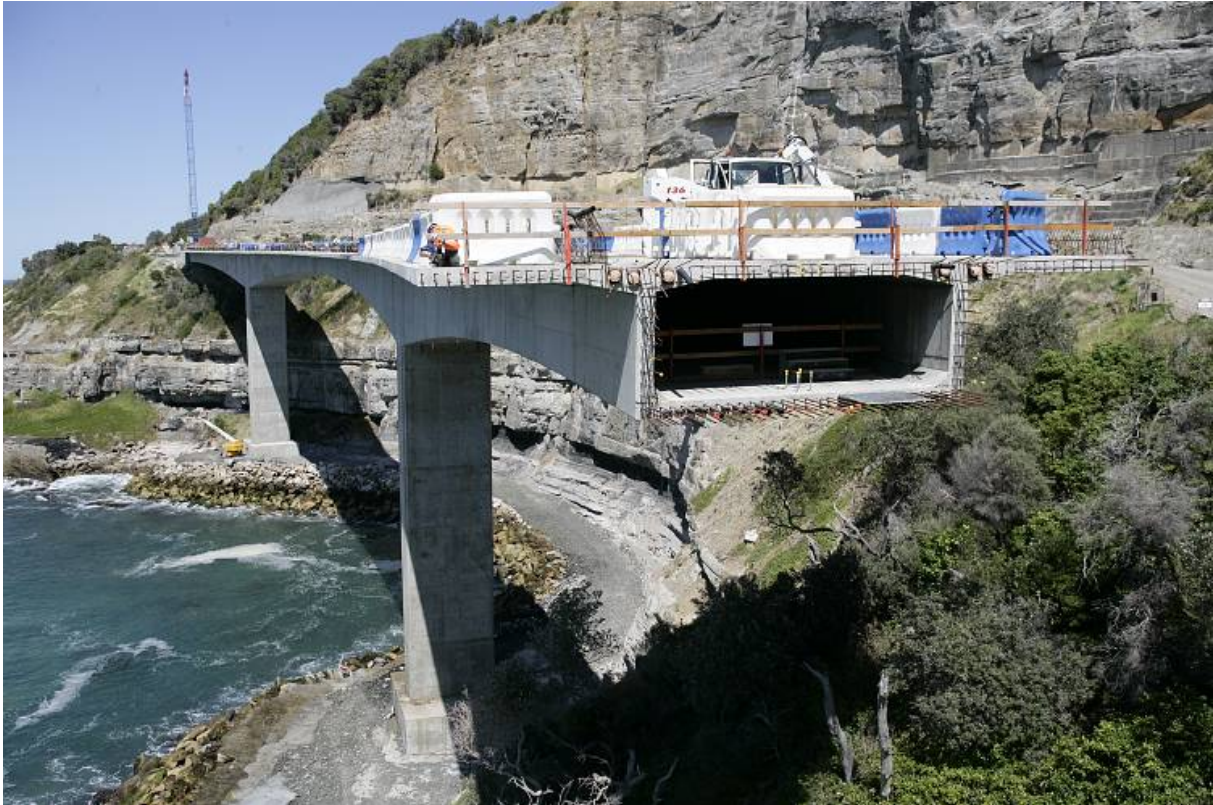
End of southern balanced cantilever bridge span
