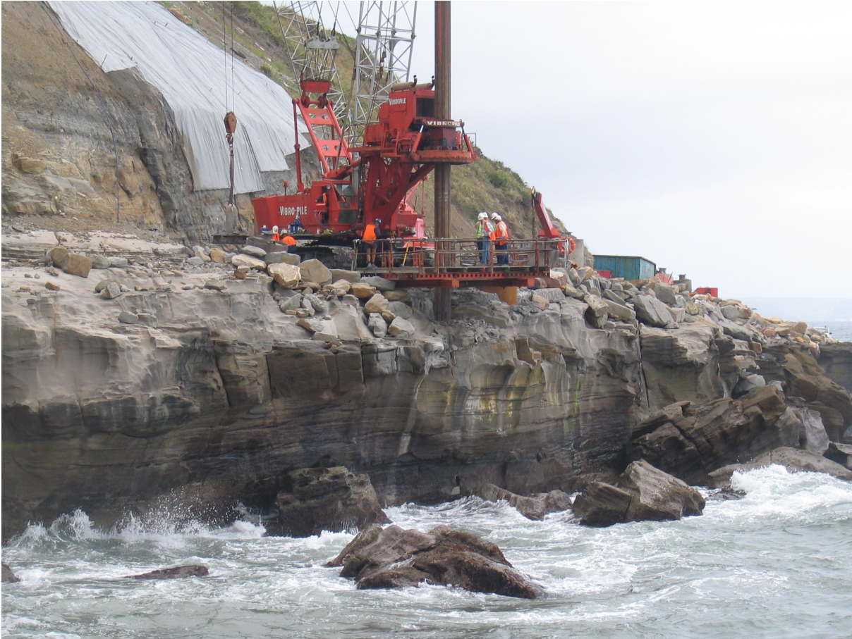
Boring piles – Pier A
