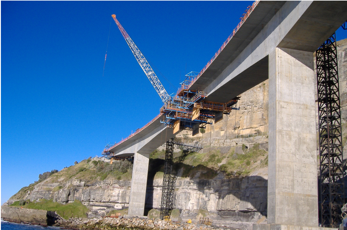
Balanced cantilever bridge spans about to meet
