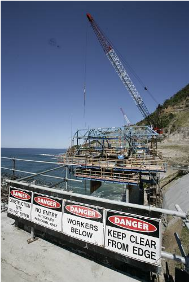
Looking south towards balanced cantilever bridge span
