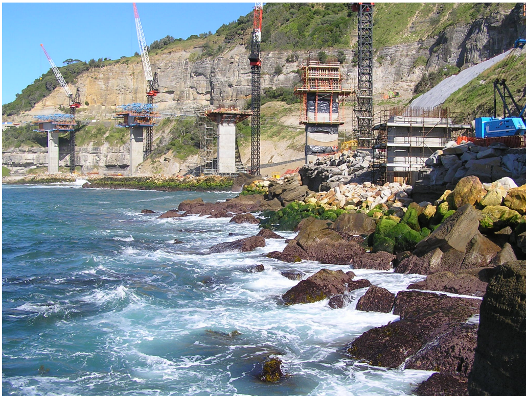
Southern piers almost complete
