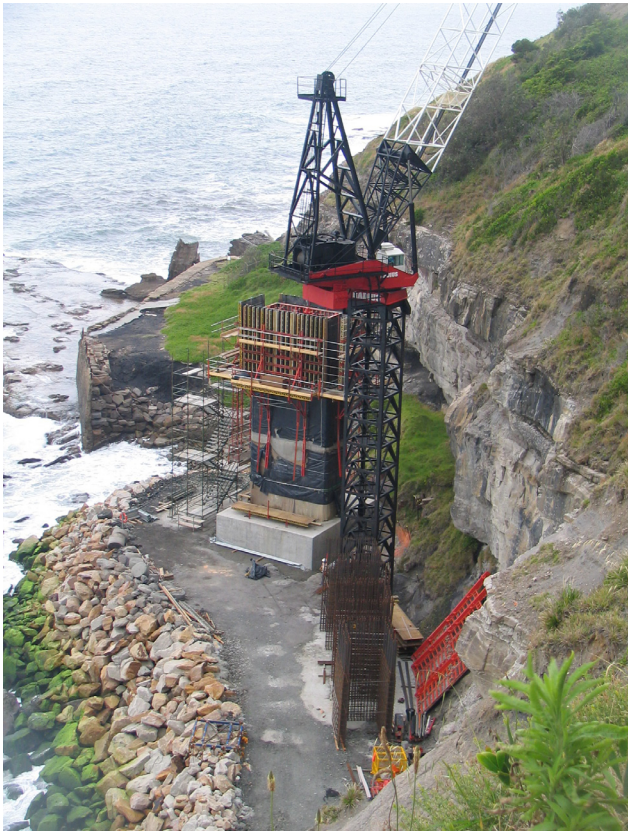
Pier D rising; old jetty behind on left
