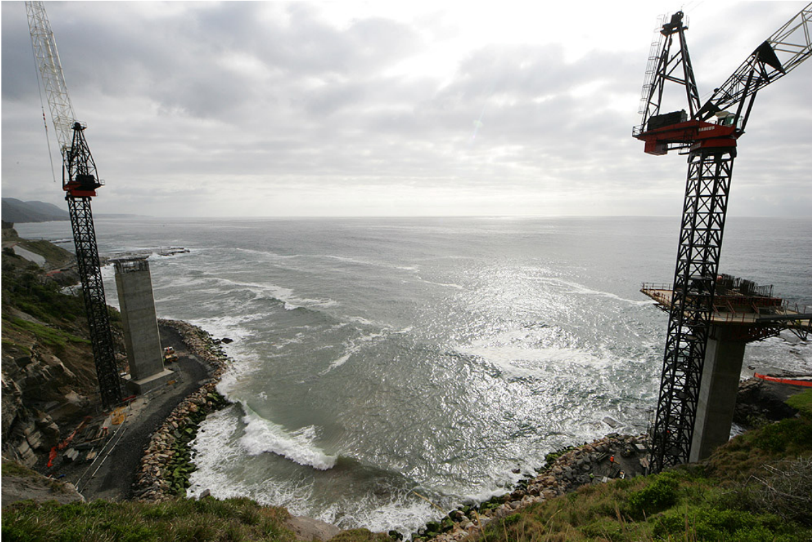
Southern balanced cantilever bridgework
