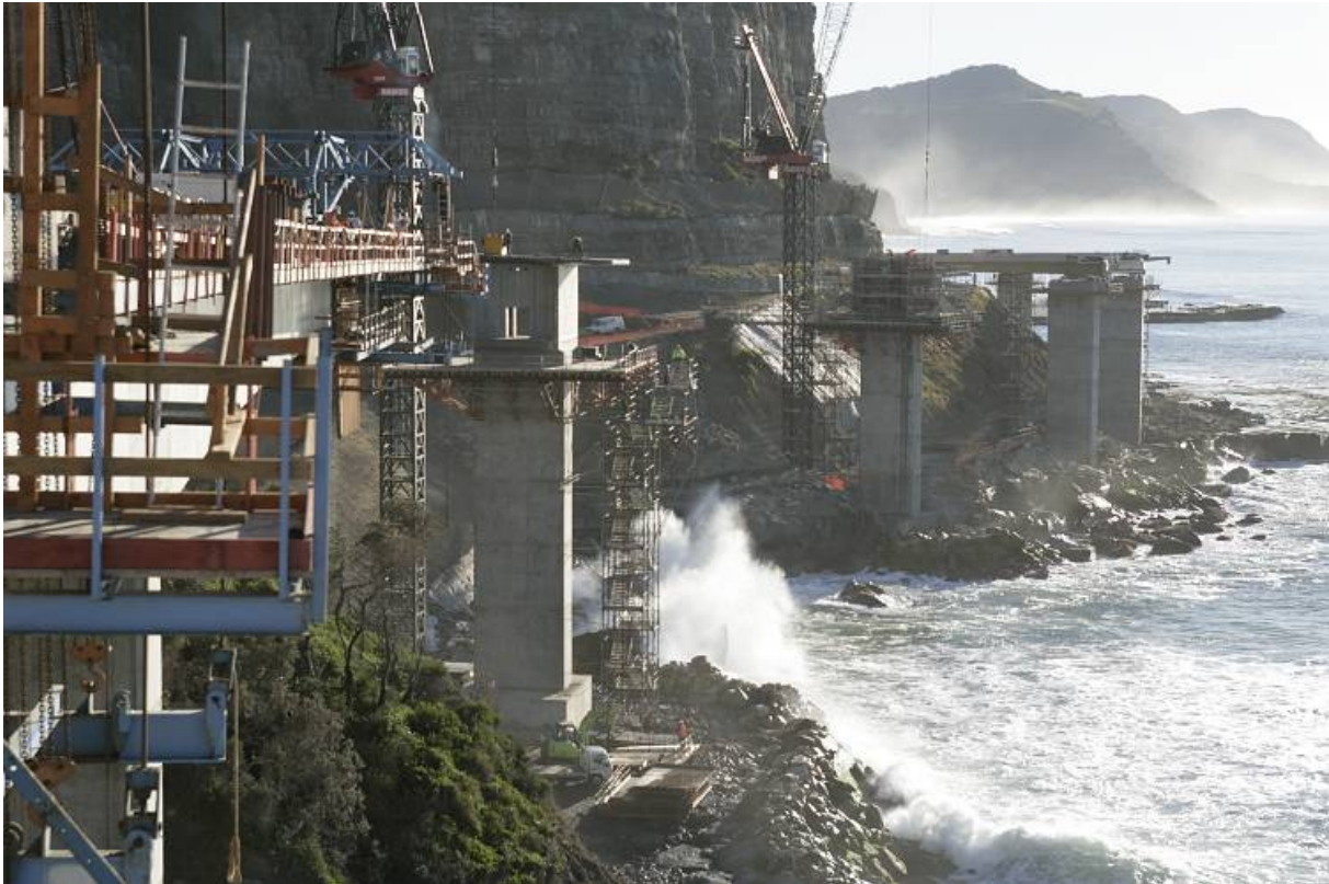
Looking north towards incrementally launched bridge
