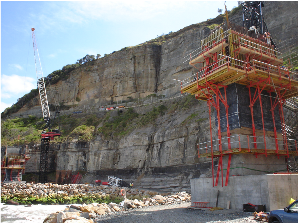
Pier work proceeding, southern amphitheatre
