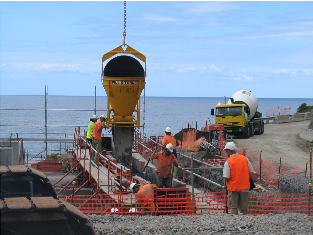
Concrete pour underway – spine beam in northern casting yard
