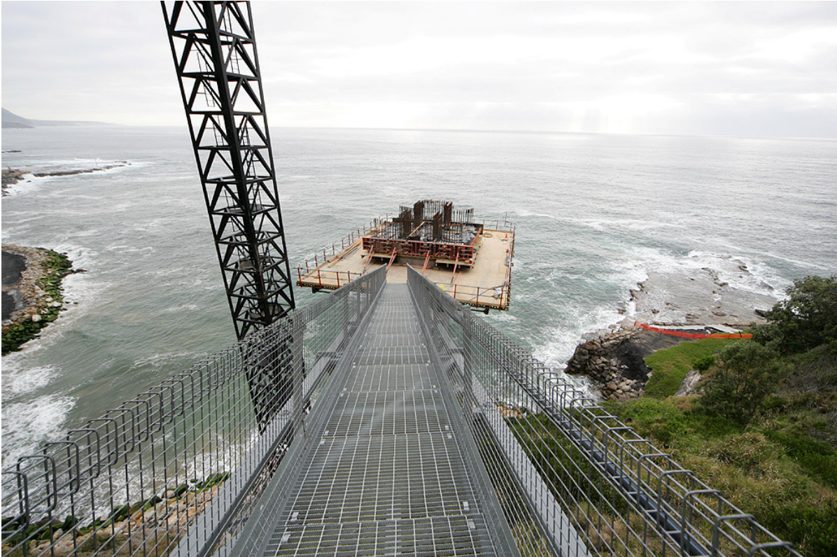
Access ramp to southern pier
