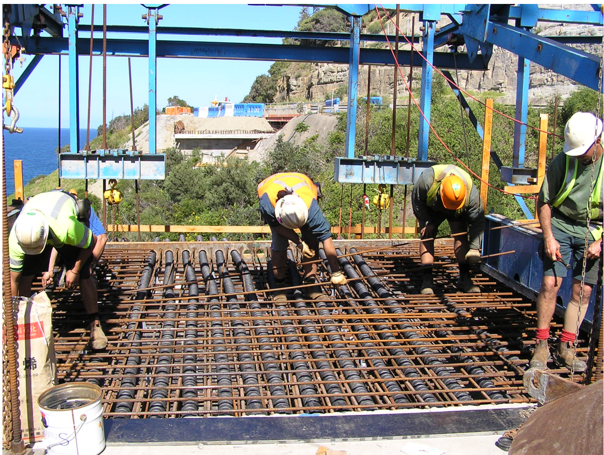
Placing reinforcement
