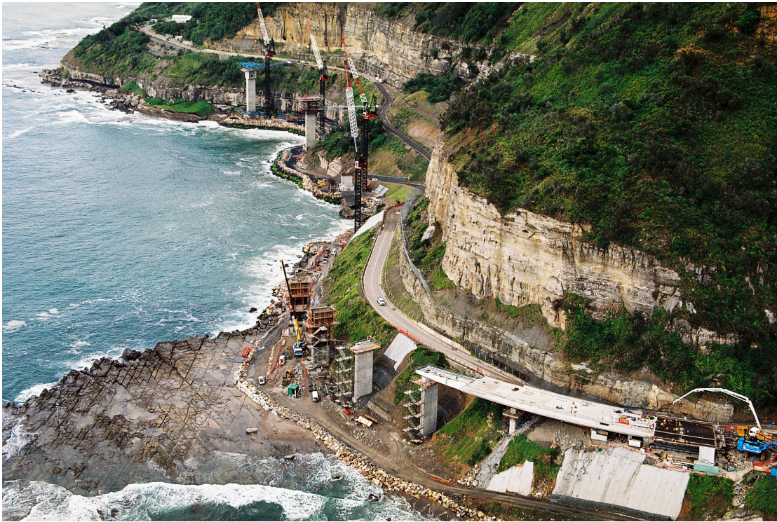
Bridgework underway – balanced cantilever (top of photo) and incrementally launched (bottom)
