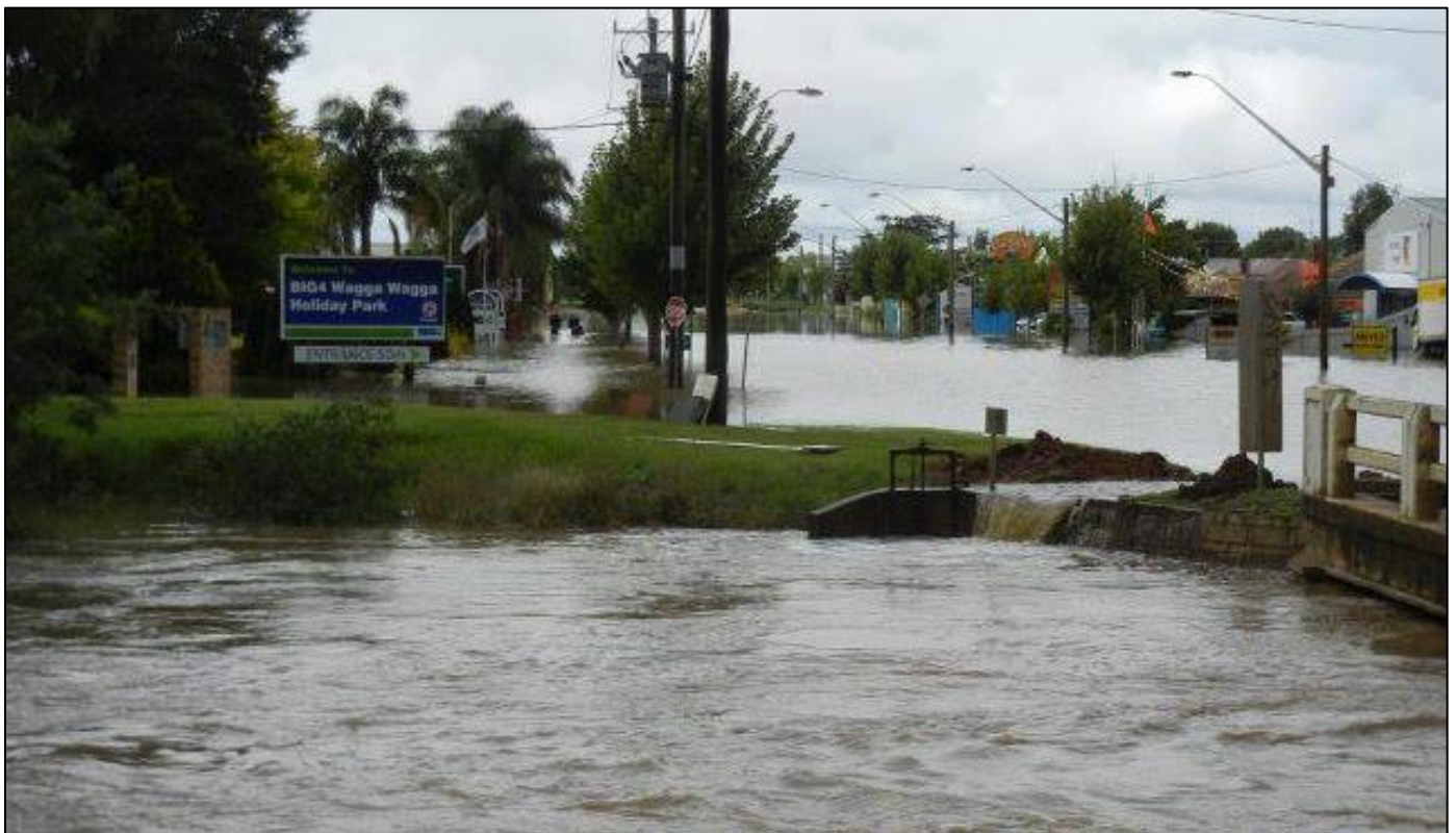
Figure 6-8 Marshalls Creek Bridge March 2012.
