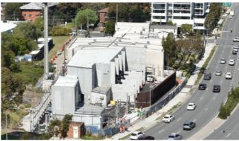
Progress photo of the fence installation taken in September 2023. The upper fence will reach 10.5 metres and installation will continue in October 2023.
