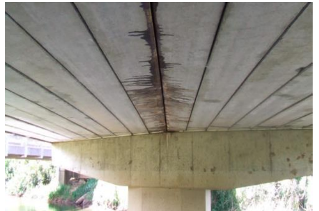
Unsealed longitudinal joints between concrete Super-T girders provide cavities/ habitat similar to gaps in concrete plank bridge decking which are known breeding roosts for Southern Myotis. Credit: GeoLINK.
