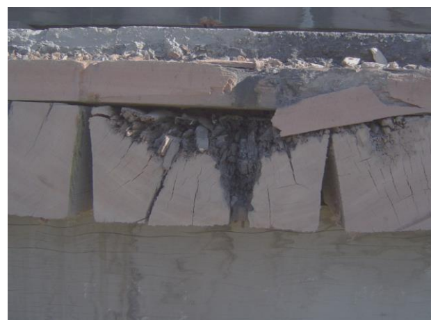
Old bridge decking providing suitable microbat habitat. Credit: Transport for NSW.
