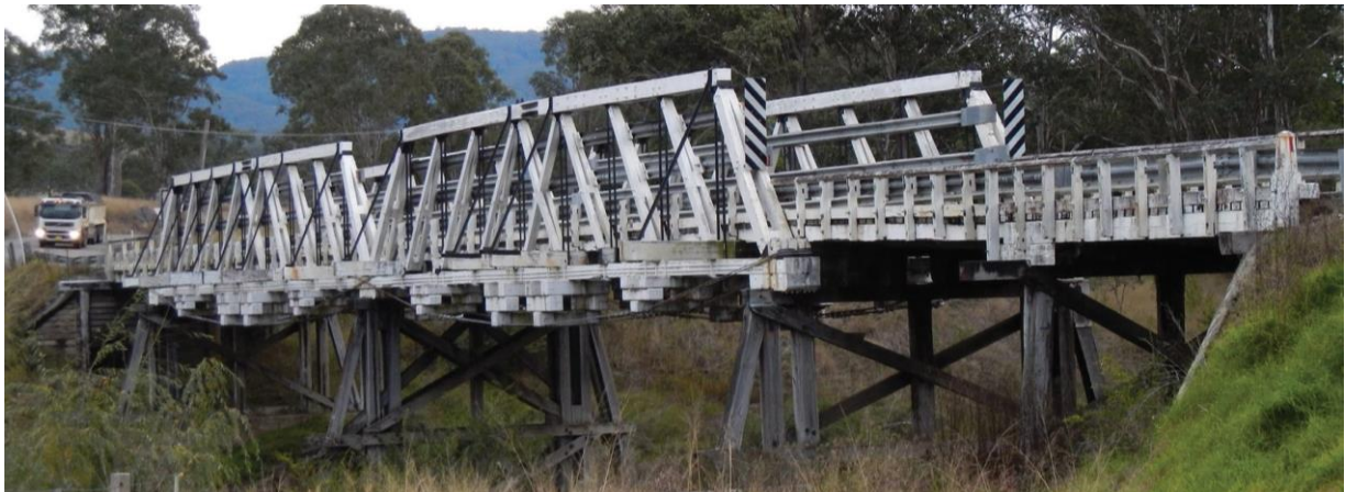
Barrington timber truss bridge. Credit: Amie Nicholas
