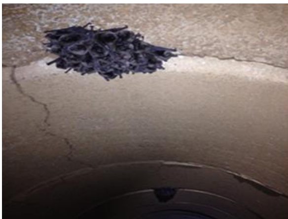
Known Southern Myotis breeding roost within unsealed joint gaps and voids within a 1200 mm 3-cell concrete pipe culvert. Credit: Veronica Silver, GeoLINK.
