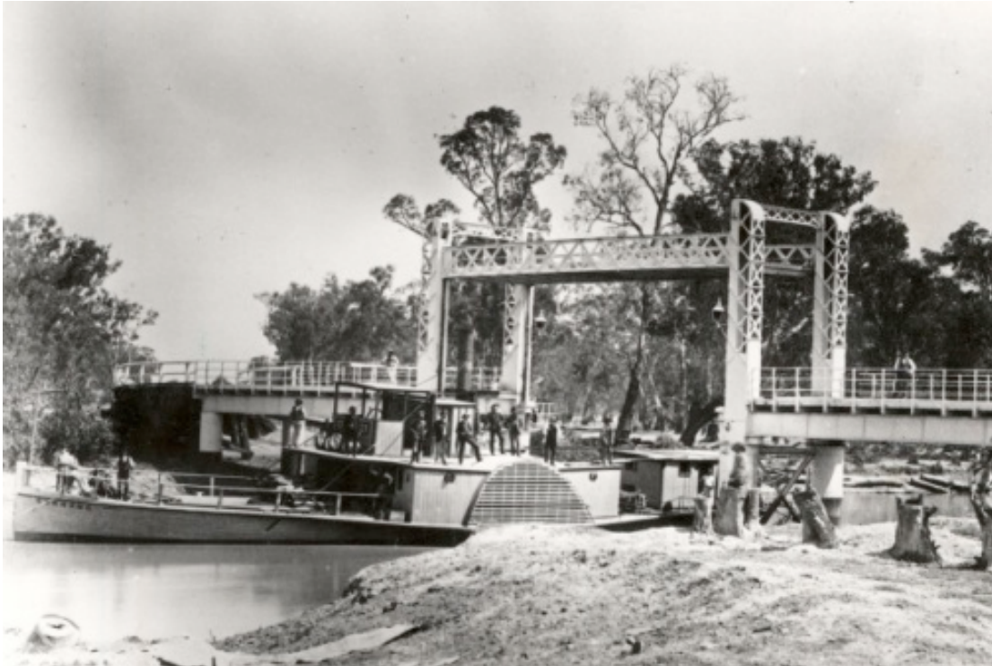
Figure 4.12 Paddle Steamer passing Balranald Bridge in the 1890s (Source: DMR HO23720)
