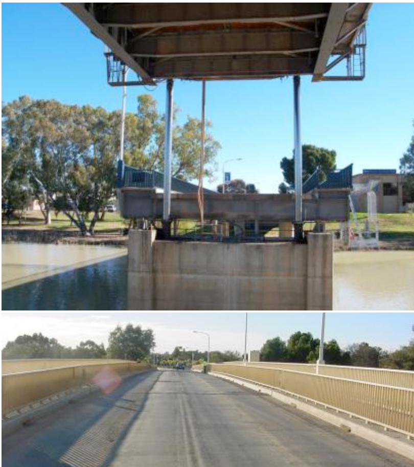
Figure 4.35 Wentworth Bridge (Source: RMS1969)
