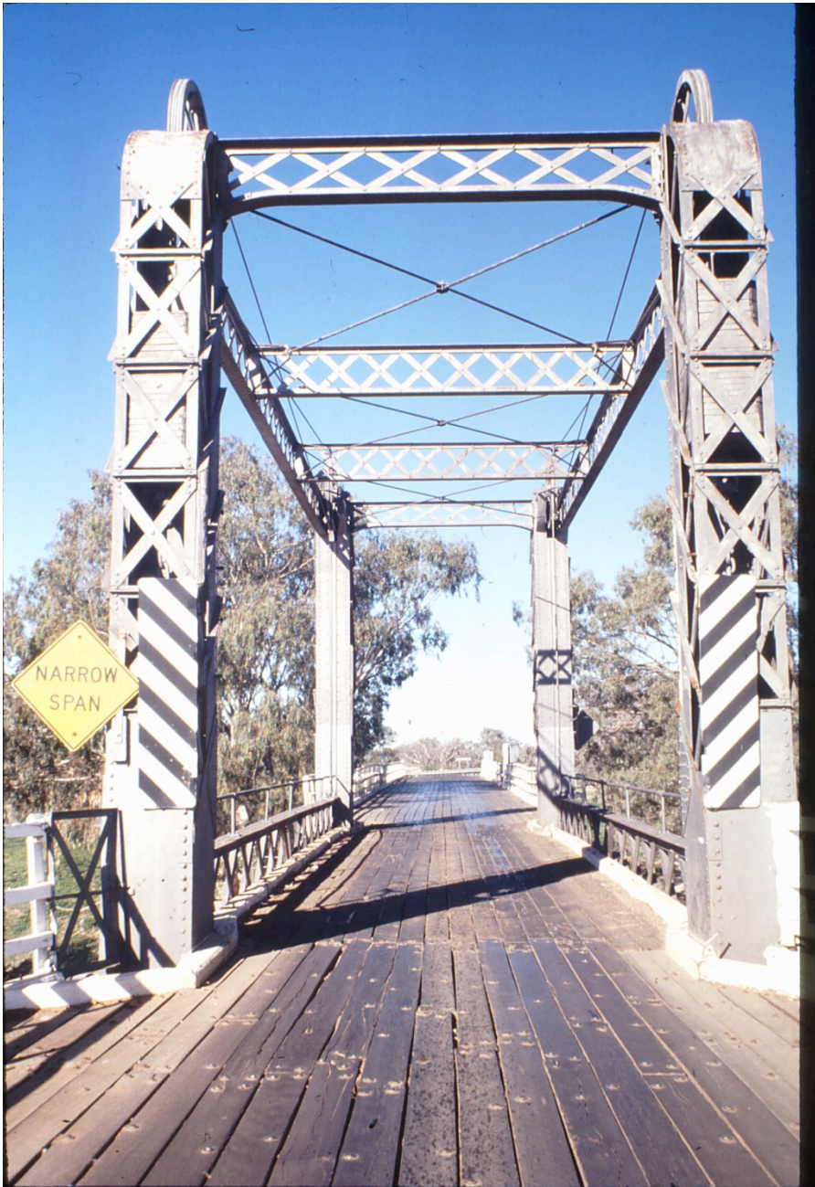
Figure 4.15 Current view of North Bourke Bridge detailing lateral bracing and stiffeners installed in 1896 (Source: RMS)
