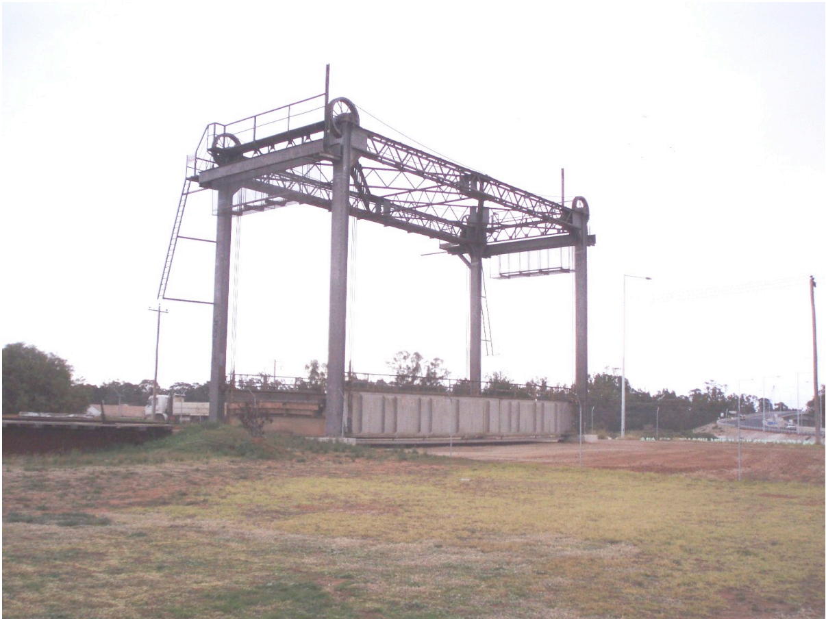
Figure 4.30 Robinvale Bridge lift tower with counterweights removed, established in a park near former bridge crossing
