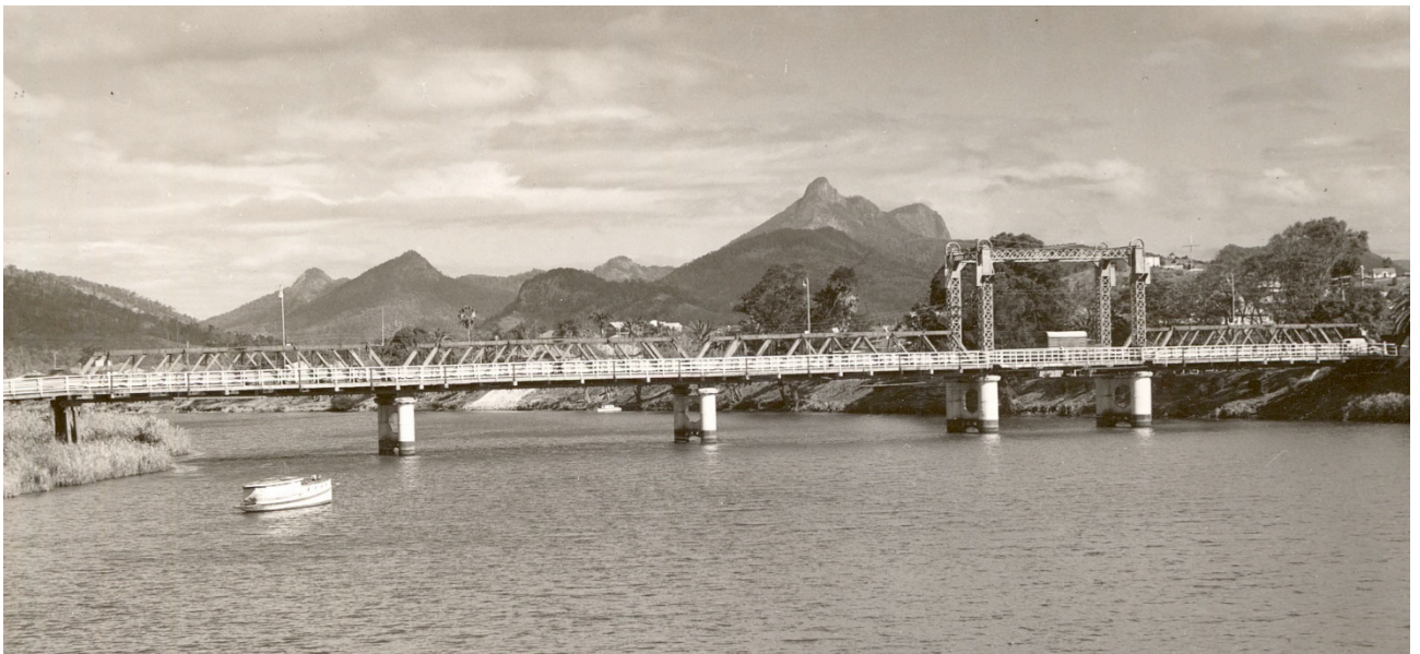
Figure 4.25 Murwillumbah Bridge with lift span and four Allan truss spans in 1947, replaced 1968 (Source: RMS photographic archives)
