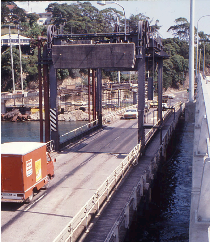
Figure 4.31 View of Boyd's Bay Bridge in 1985 just prior to replacement (Source: RMS photographic archives)
