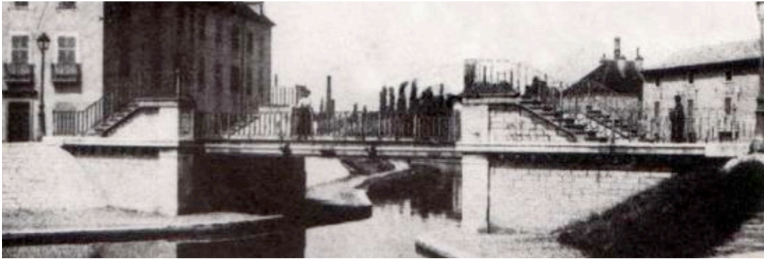
Figure 4.10 Pont De Larrey (1890)
