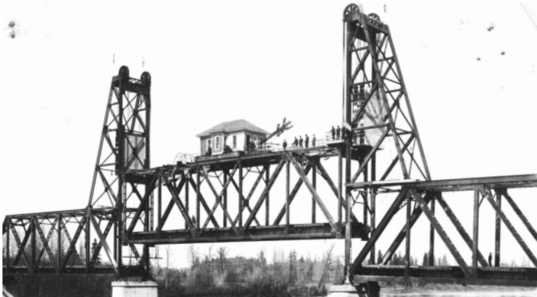
Figure 4.27 Rail bridge over the Willamette River at Salem, Oregon (Source: Gerald W. Williams Collection, Oregon State University Archives, Corvallis Oregon)
