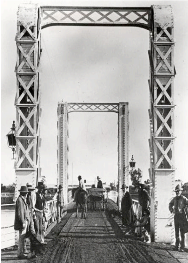
Figure 4.14 Formal opening of North Bourke Bridge in 1883 (Source: DMR HO23716).
