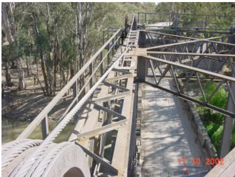
Figure 5.102 Wire ropes on Gonn Crossing Bridge
