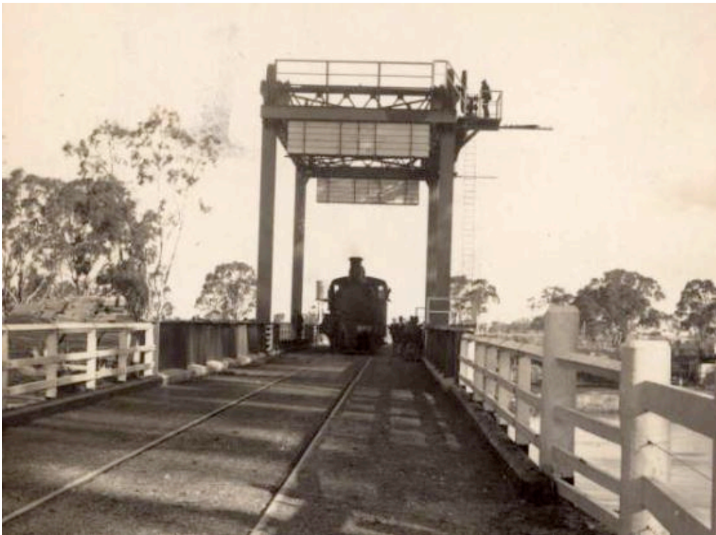
Figure 5.93 Train on Gonn Crossing Bridge 1926 (Source: State Library of Victoria, mp013888)
