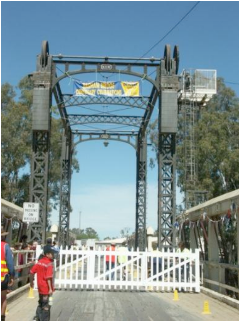
Figure 5.61 Decorative gate set up on bridge for Centenary celebrations, 9 th and 10 th October, 2004
