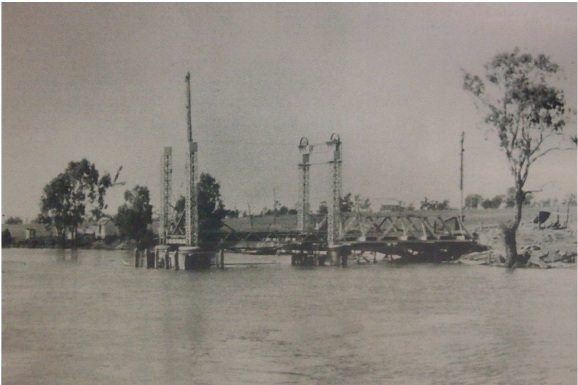
Figure 5.79 Lift towers assembly (Source: Swan Hill Regional Library)
