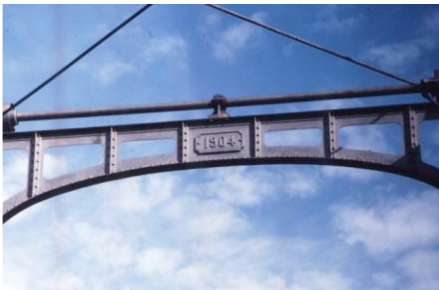
Figure 5.68 Date plaque on tower transverse brace member (Source: RMS)
