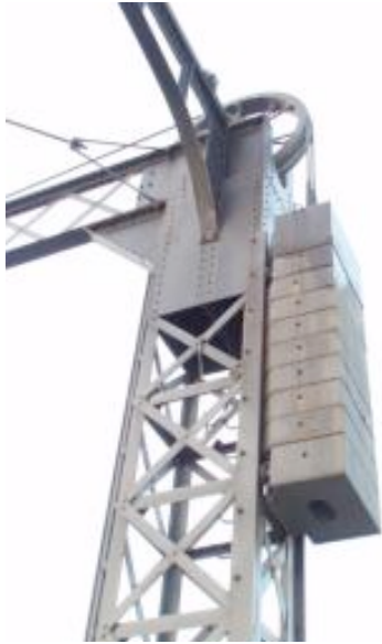
Figure 5.53 Cobram counterweights (Source: RMS)
