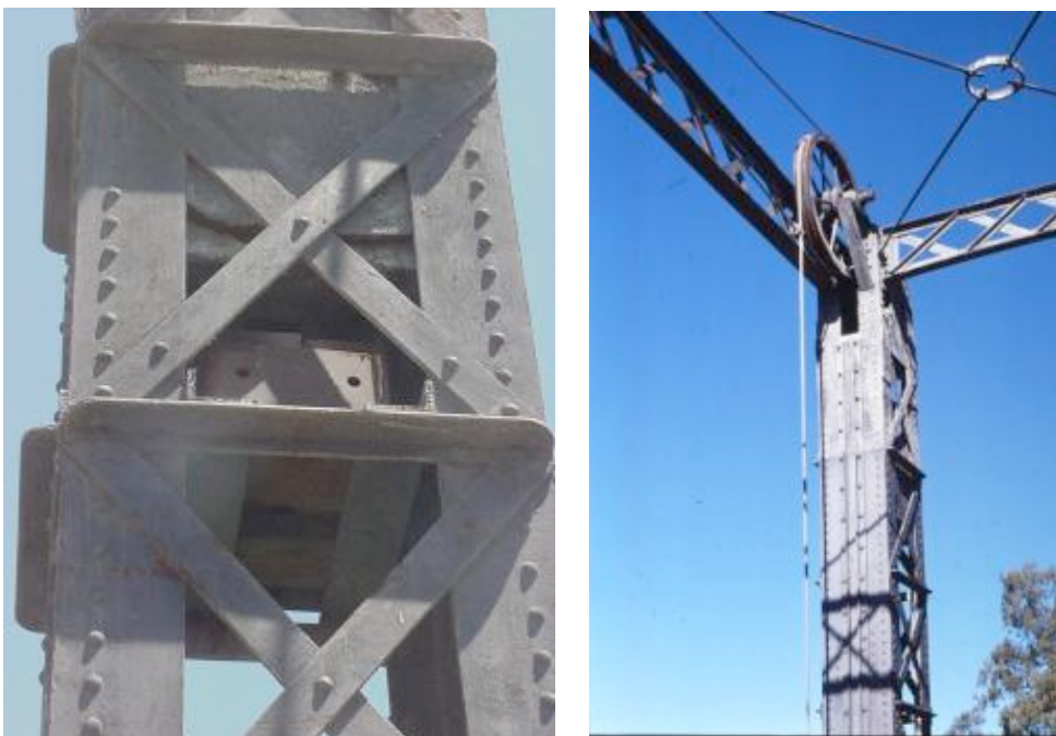
Figure 5.7 Propped counterweights and attached cables (Source: RMS)
