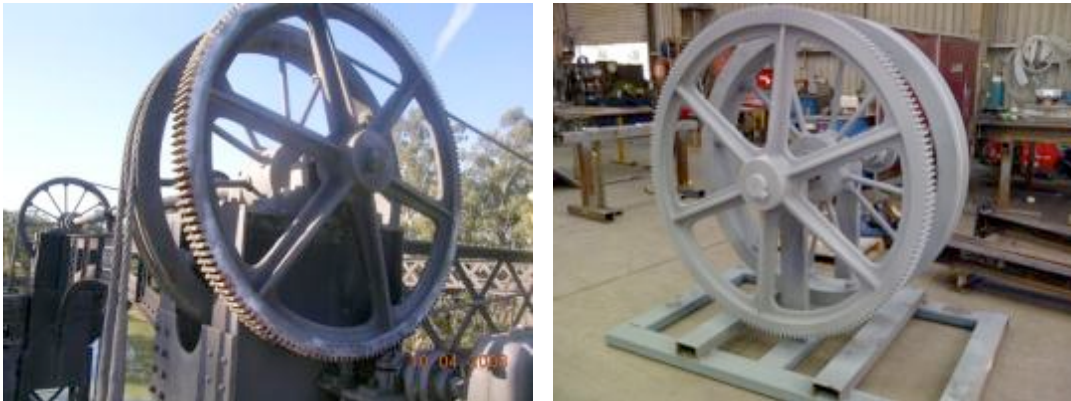
Figure 5.64 Sheave wheel testing on Barham Bridge
