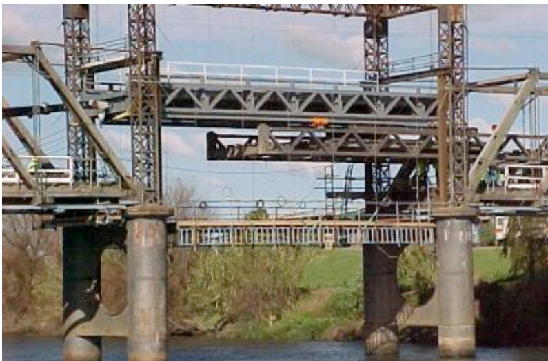
Figure 5.35 Replacement of Dunmore Bridge movable span (Source: RMS)
