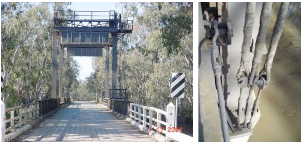
Figure 5.97 Bridge deck and Compensating bracket (Source: GHD)
