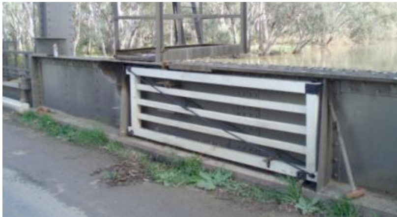
Figure 5.101 Gate on Gonn Crossing Bridge (Source: RMS)
