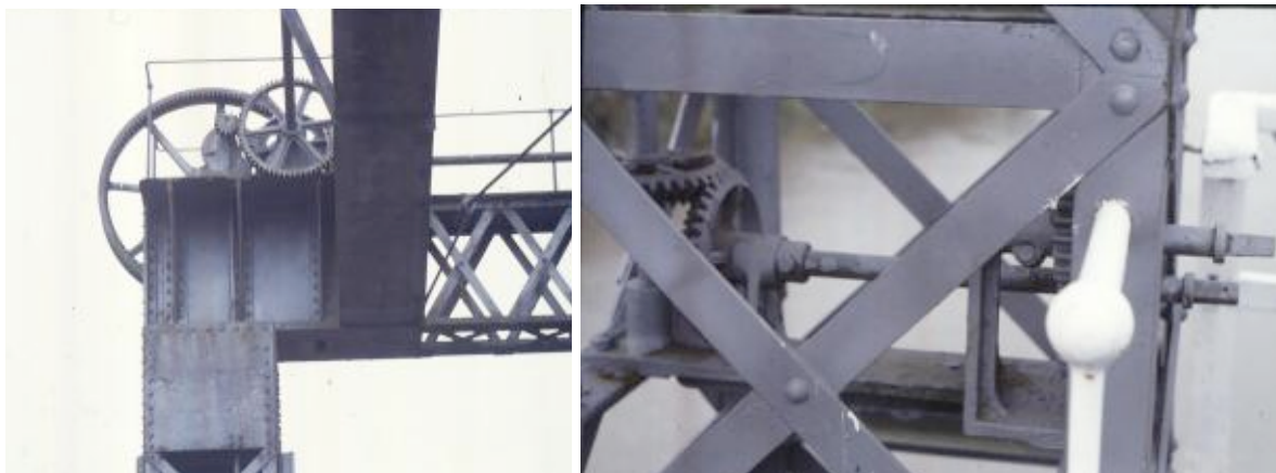
Figure 5.36 Top sheave & gearing and winch mechanism (Source: RMS)
