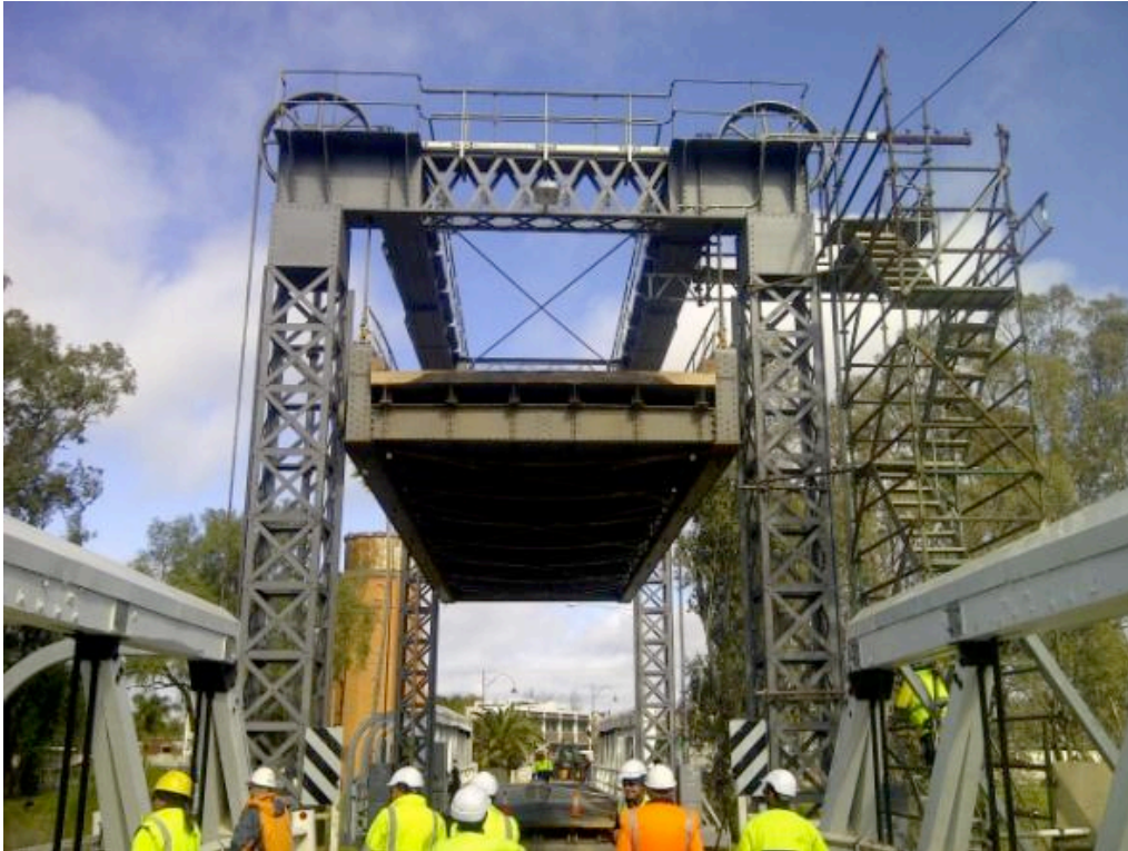
Figure 5.20 Lift span raised in 2013 during mechanical testing (Source: RMS)
