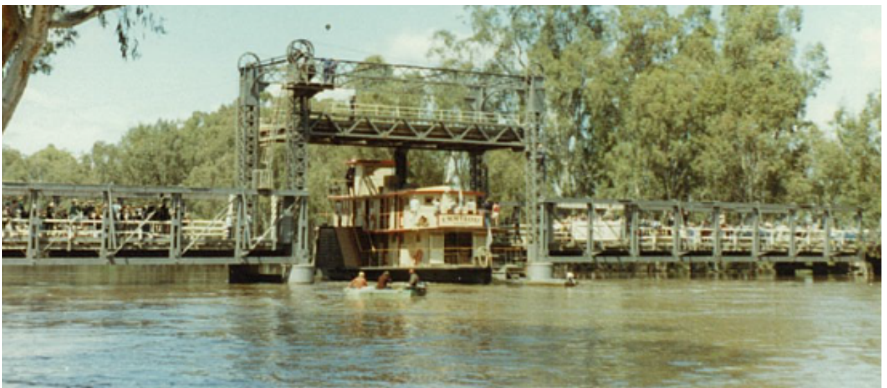
Figure 5.63 Lift span raised to full height in 1985 during a flooding event (Source: RMS Bridge File)
