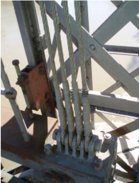
Figure 5.87 Lifting span attach point (Source: RMS)
