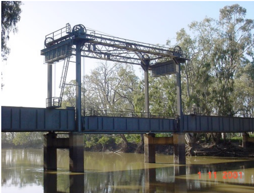
Figure 5.92 General View of Gonn Crossing Bridge (Source: GHD)
