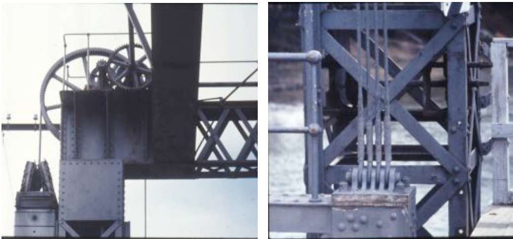
Figure 5.27 Lifting gears and winding platform on Swan Hill Bridge (Source: RMS)
