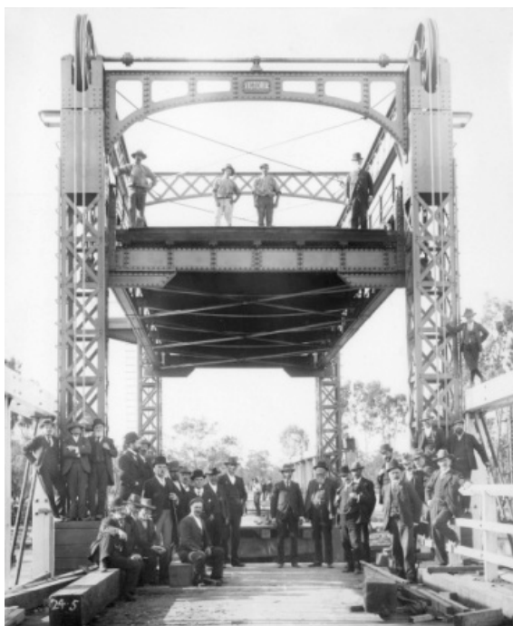
Figure 5.59 Lift span raised during the official opening of Barham Bridge in September 1904 (Source: University of Melbourne Library)
