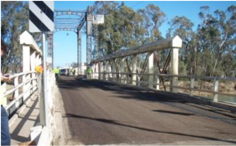
Figure 5.66 Image of re-surfaced bridge deck (Source: RMS)
