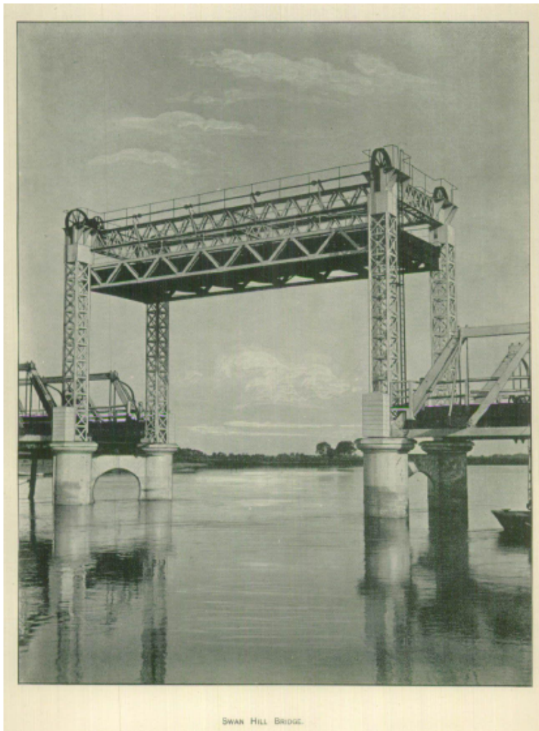
Figure 5.24 Bridge shown soon after completion with lift span at maximum opening height and counterweights at deck level (Source: Annual Report Department of Public Works, 1895)
