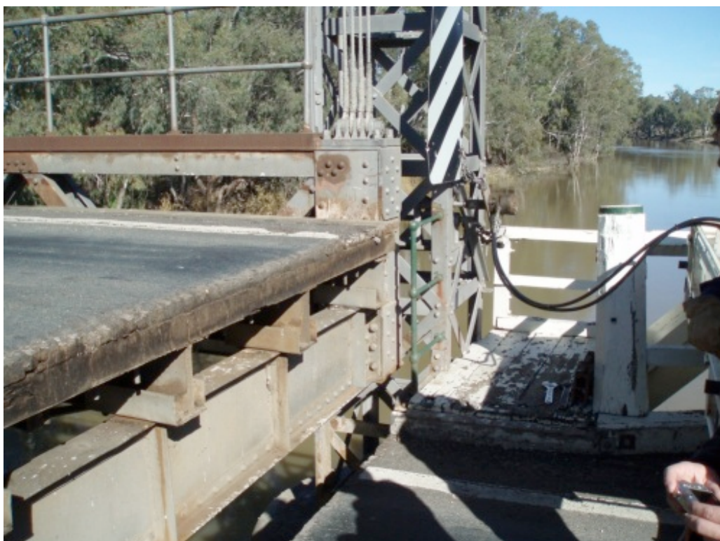
Figure 5.91 Portable motor fitted to Tooleybuc Bridge to raise the span
