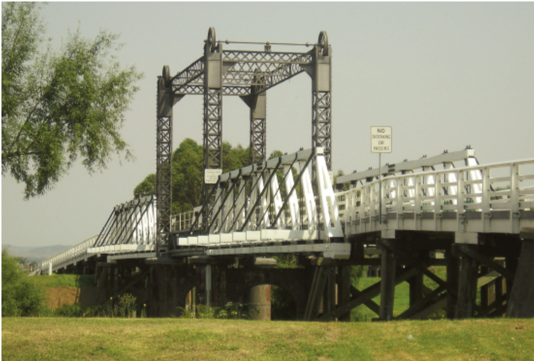
Figure 5.38 View of lift span and timber truss spans from riverbank
