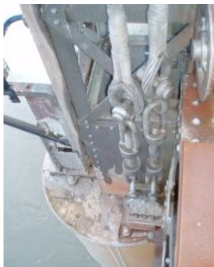
Figure 5.52 Compensating bracket for Cobram Bridge (Source: RMS)
