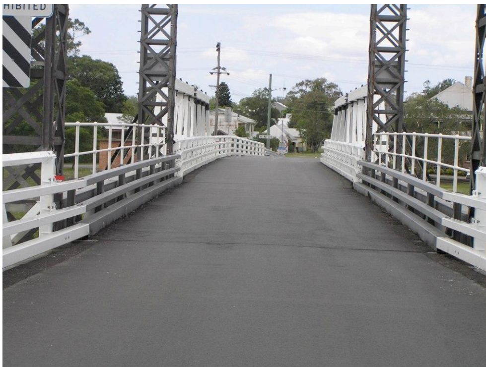
Figure 5.41 View of sealed lift span deck after replacement in 2006
