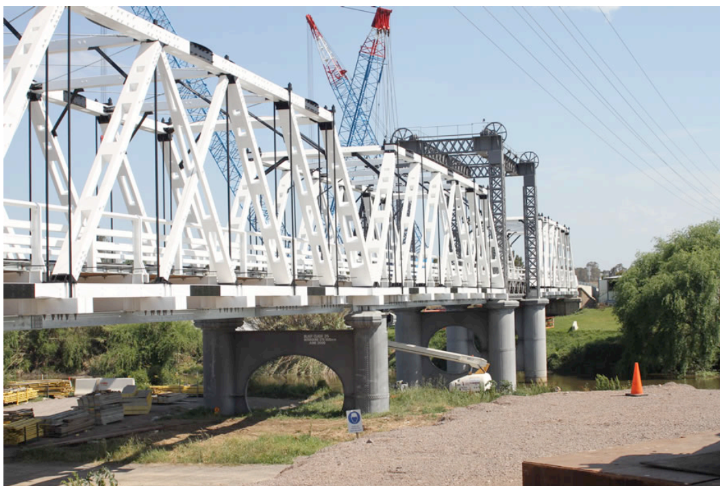
Figure 5.29 General view of Bridge following truss replacement in 2012
