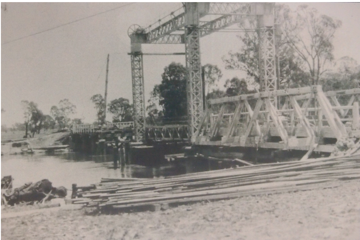
Figure 5.80 Tooleybuc Bridge during construction 1924 (Source: Hickey 1992)
