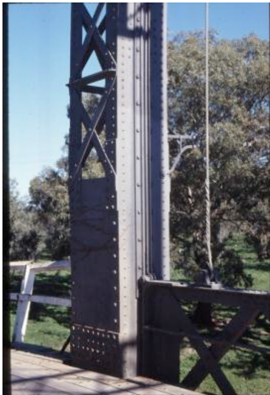
Figure 5.11 Tower and rope connection to movable span (Source: RMS)
