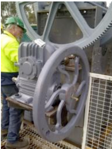
Figure 5.65 Repair works on Barham Bridge
