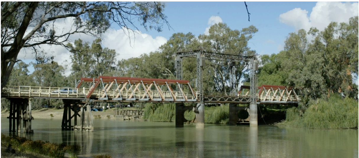
Figure 5.13 View of Bridge looking south
