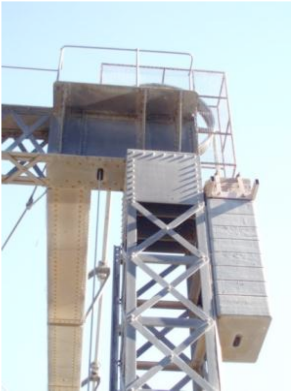
Figure 5.88 Tooleybuc Bridge Counterweights (Source: RMS)
