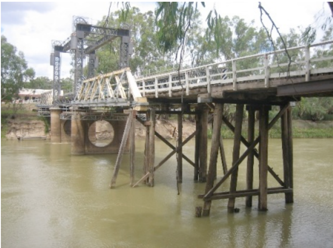
Figure 5.76 General View of Tooleybuc Bridge (Source: Victorian Heritage data base)
