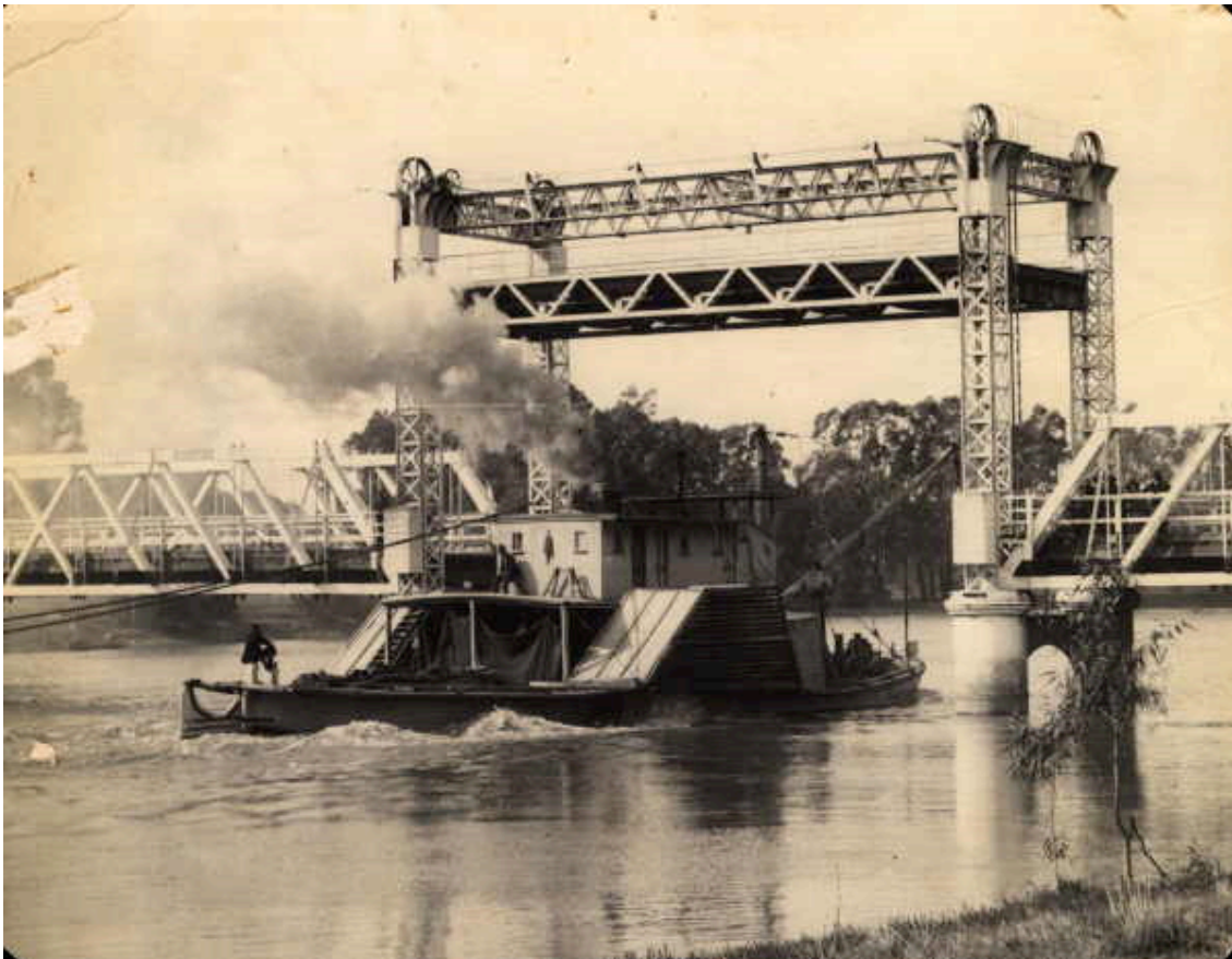
Figure 5.16 View of the lift span in raised position with passing paddle steamer – c.1900 (Source: State Library of Victoria, image number: pi000942)
