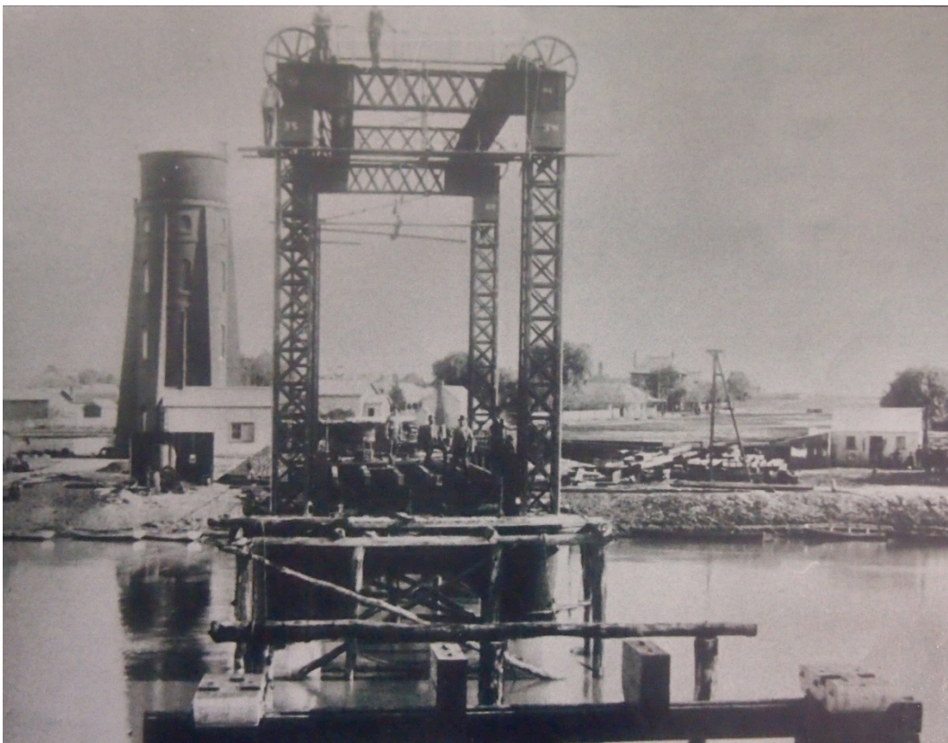
Figure 5.14 Swan Hill Bridge under construction with lift tower in place (Source: Swan Hill Regional Library)
