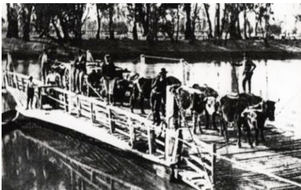
Figure 5.58 Punt unloading cattle at Barham-Koondrook (Source: Grant 1970)
