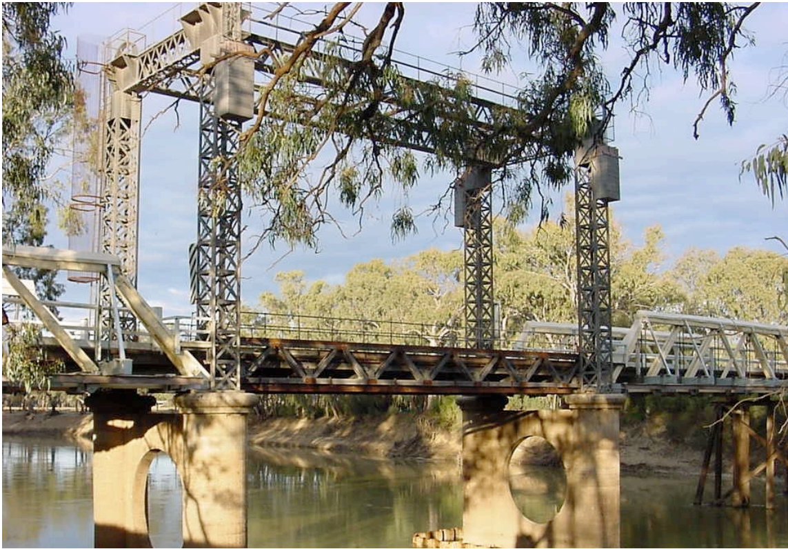
Figure 5.85 Detailed view of movable span of Tooleybuc Bridge (Source: RMS)
