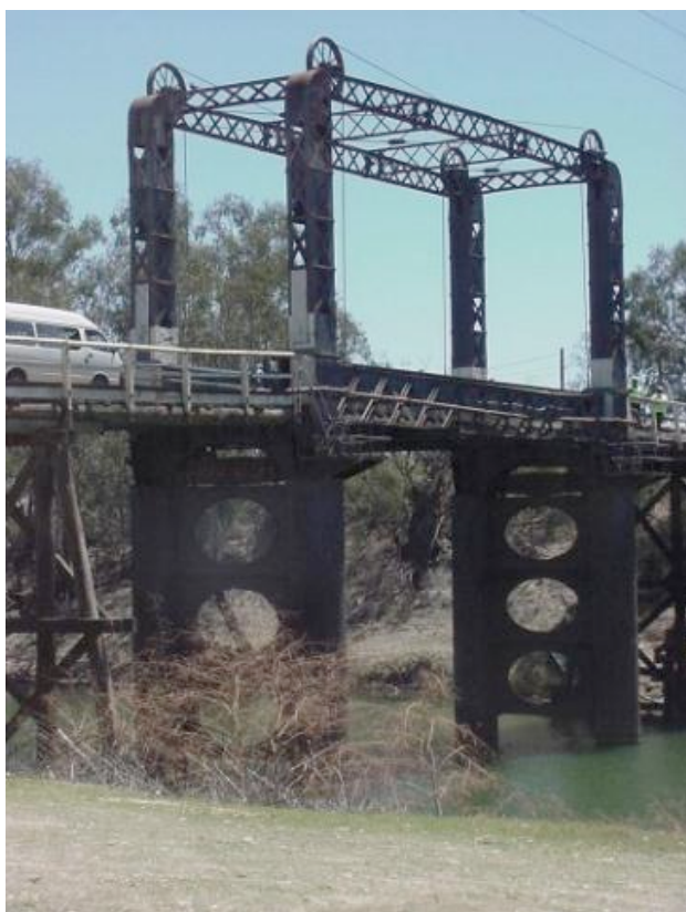
Figure 5.1 Oblique view of Brewarrina Bridge in 2008
