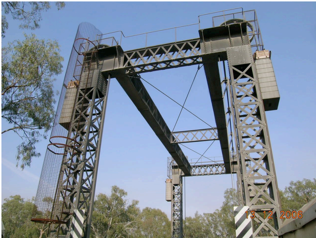
Figure 5.83 Towers and counterweights on Tooleybuc Bridge
