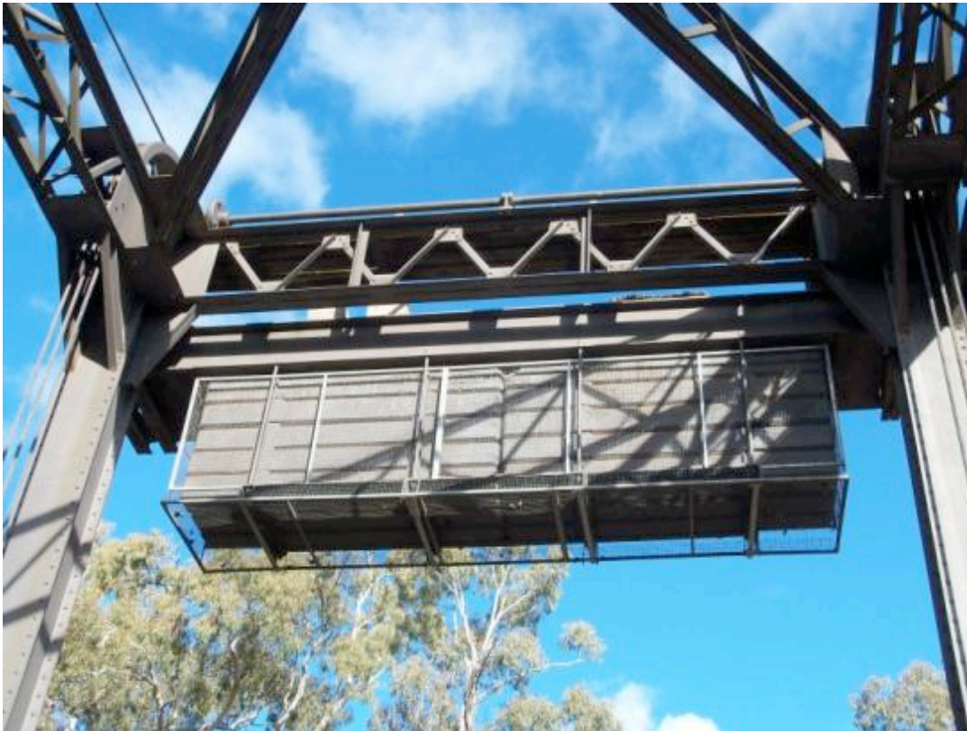
Figure 5.98 Gonn Crossing counterweights (Source: RMS)
