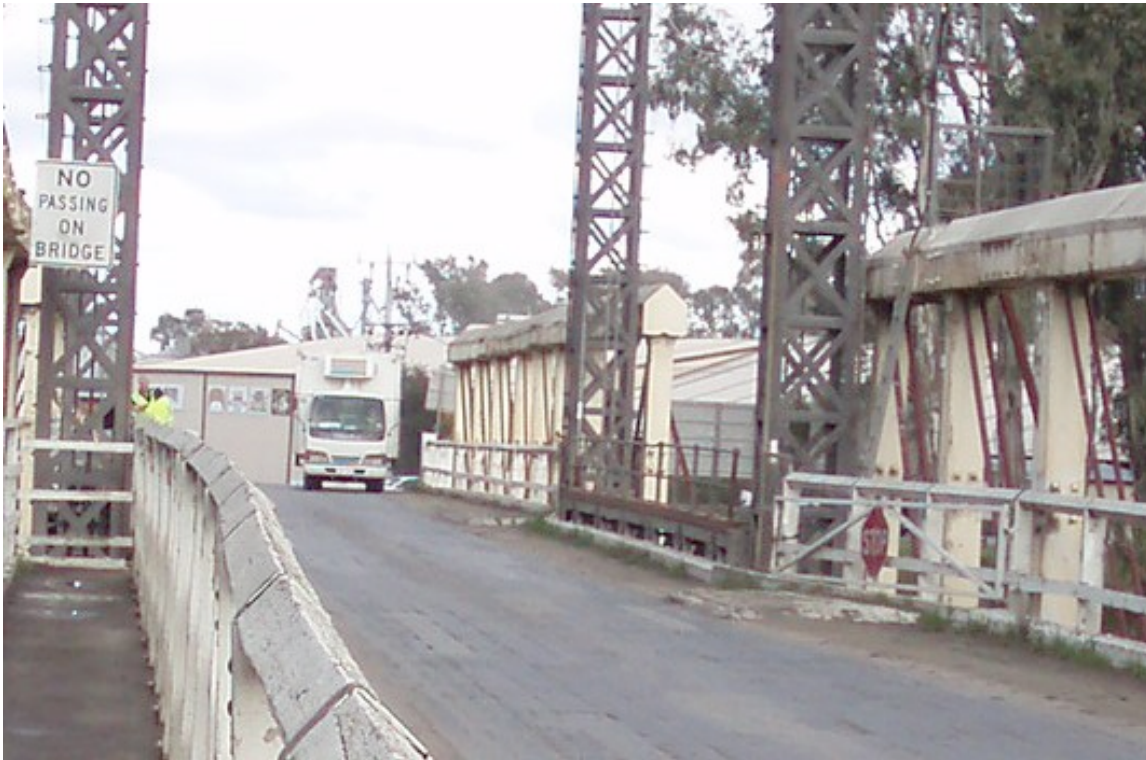
Figure 5.74 Current pedestrian barriers either side of movable span
