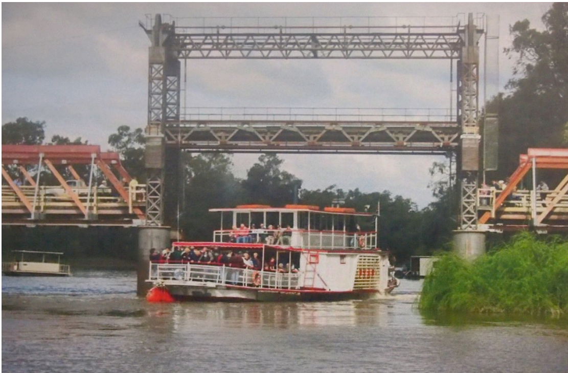
Figure 5.18 Recent view of lift span raised for paddle steamer traffic
