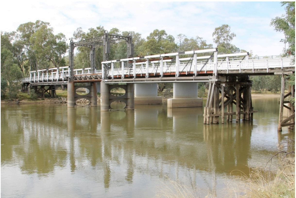
Figure 5.45 General view of Cobram Bridge (Source: RMS)
