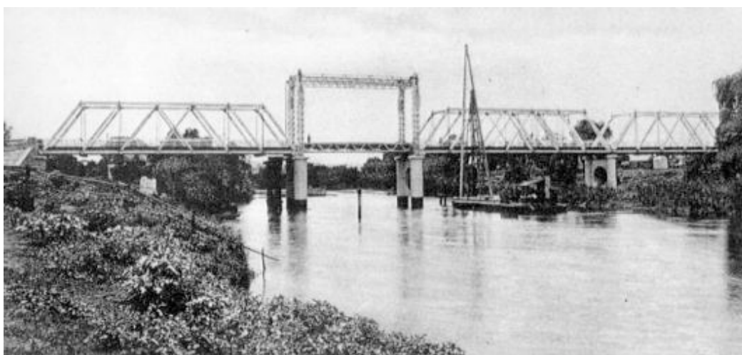
Figure 5.31 Dunmore Bridge in 1908 (Source: Digital Hunter, Newcastle Library)
