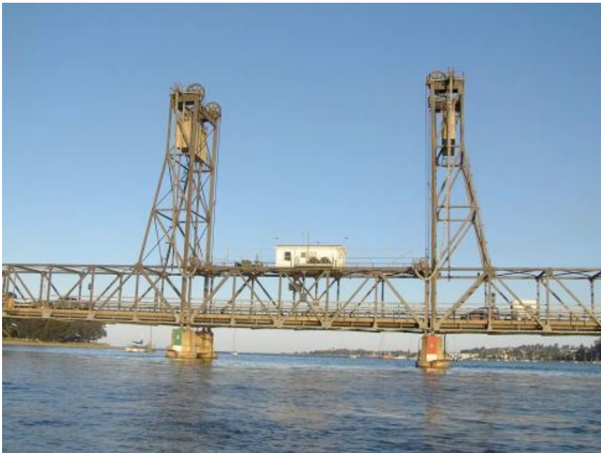
Figure 5.164 Detailed view of towers of Batemans Bay Bridge
