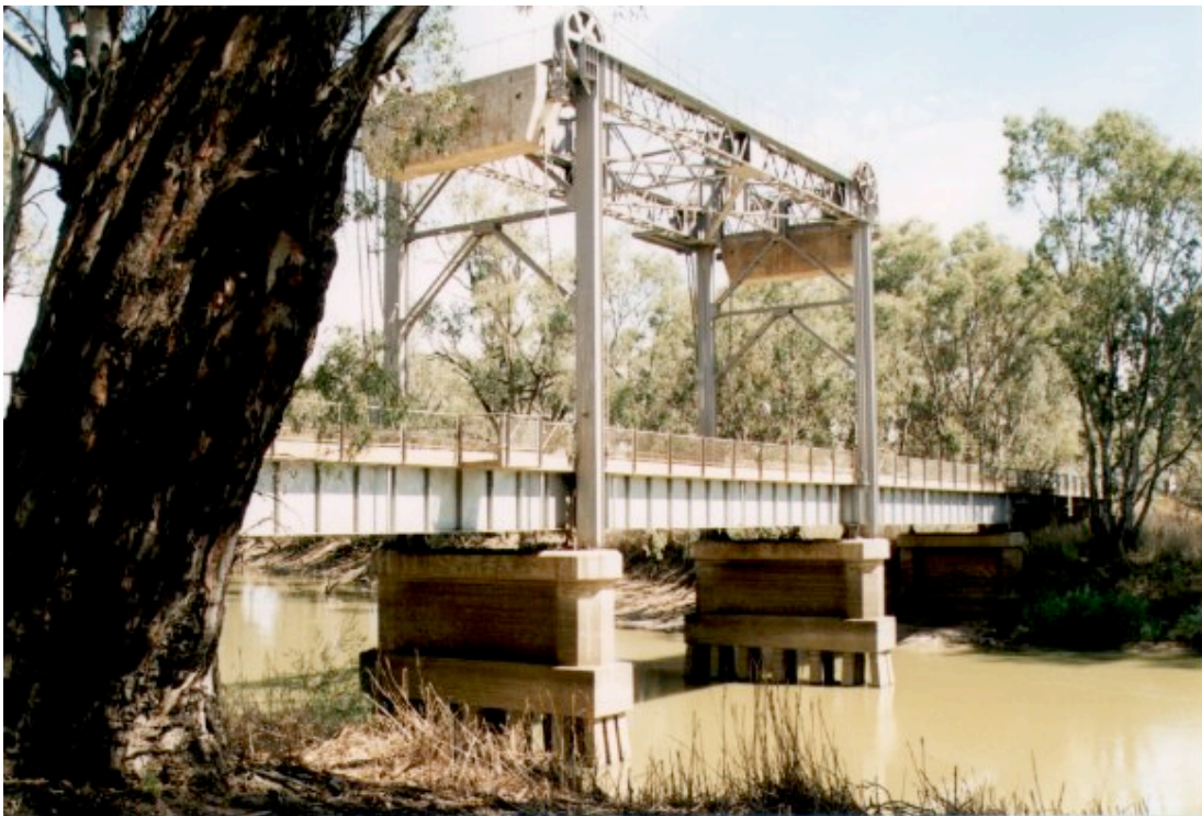
Figure 5.131 General View of Nyah Bridge
