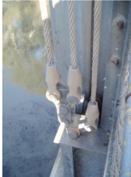
Figure 5.138 Nyah movable span attachment (Source: RMS)
