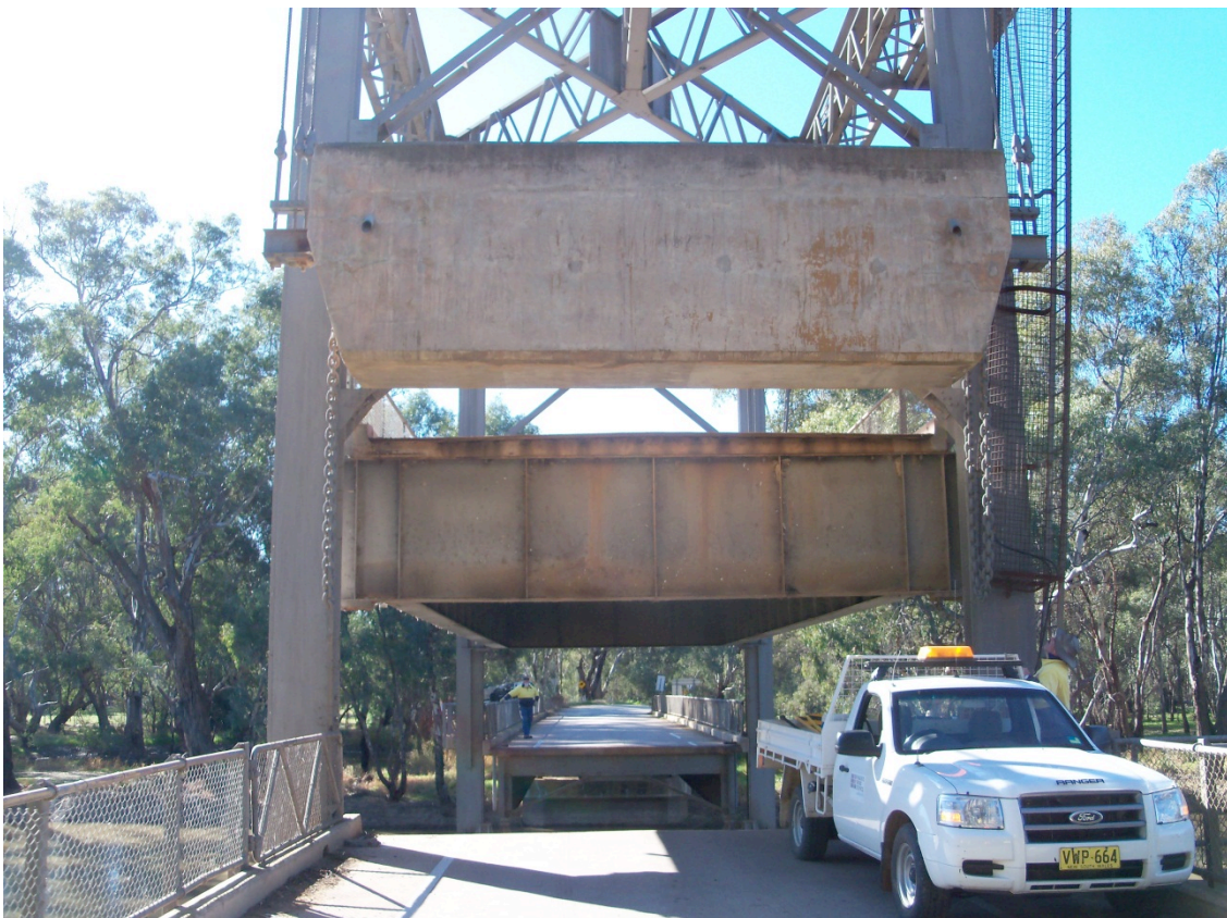
Figure 5.134 Lowered counterweights during a test lift (Source: RMS)
