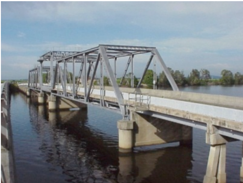
Figure 5.112 General View of Mororo Bridge from the 1993 south bound bridge
