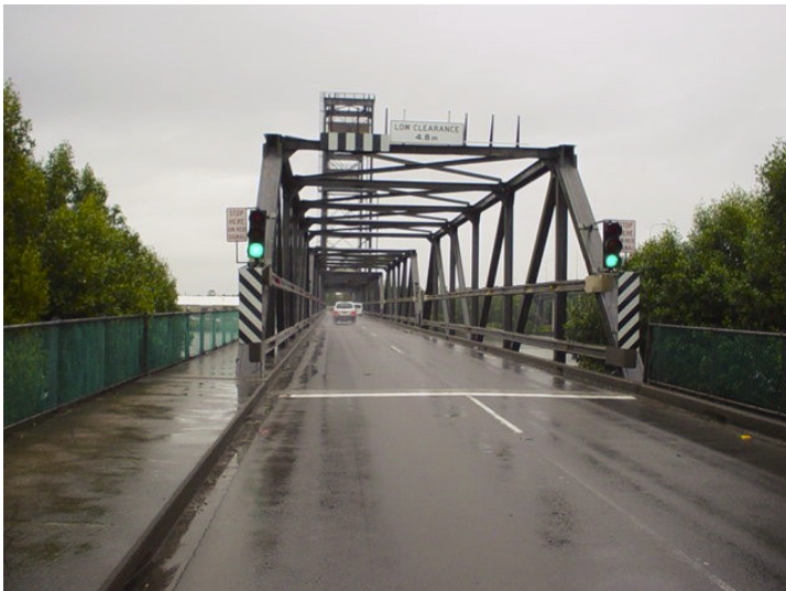
Figure 5.157 Traffic control system on Hexham Bridge
