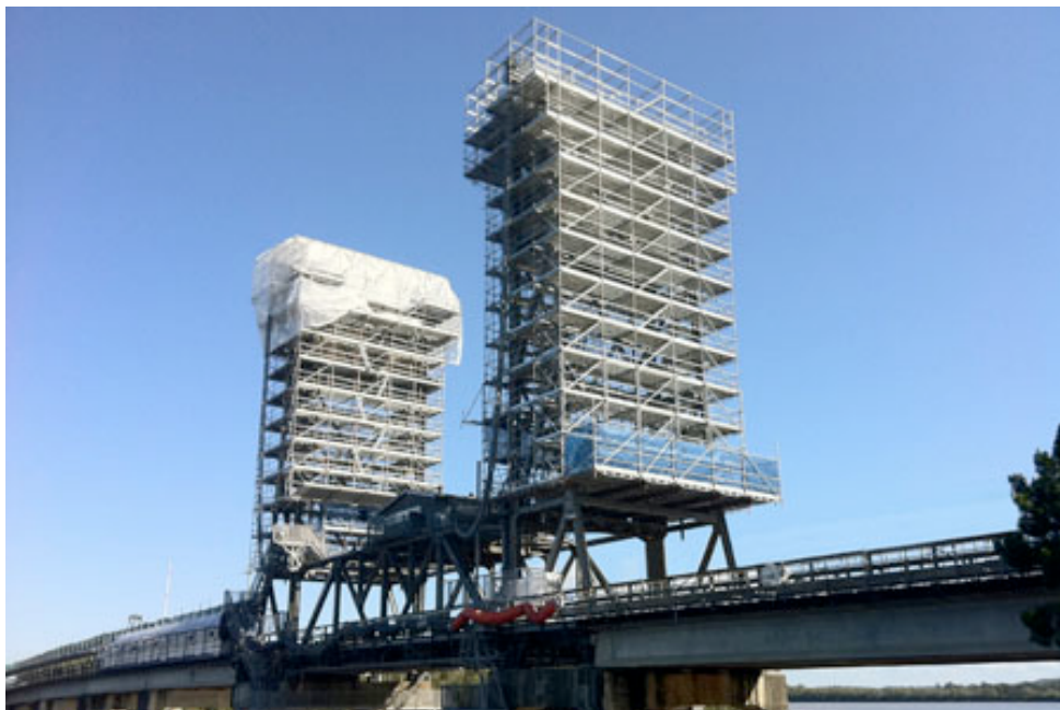
Figure 5.178 Scaffolding on lift towers in 2013, (Source: Layher Scaffold website)
