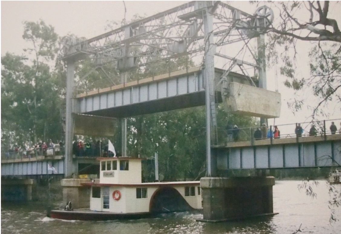
Figure 5.133 Lift span raised in 2000 (Source: Swan Hill Regional Library)
