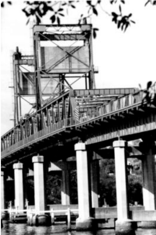
Figure 5.124 View of Ryde Bridge in 1970 with lift span closed and counterweights in regular position (Source: Photograph courtesy of Canada Bay Council)
