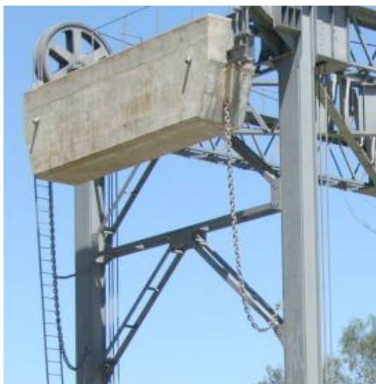
Figure 5.139 Counterweights for Nyah Bridge (Source: RMS)
