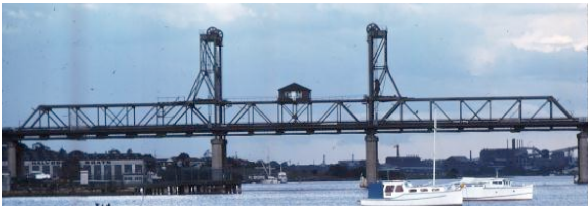
Figure 5.128 View of bridge in 1981. Engine house has since been removed
