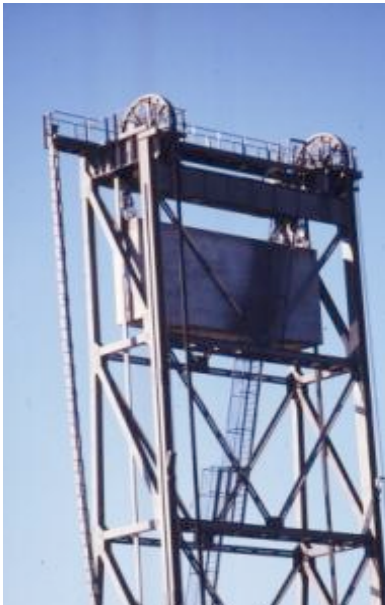
Figure 5.184 Wardell counterweights in 1985 (Source: RMS)
