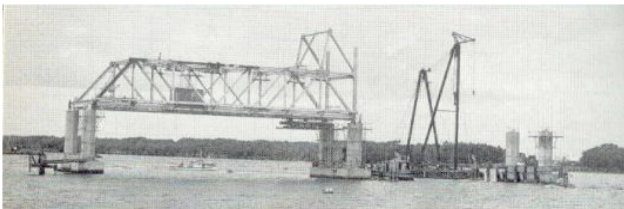
Figure 5.193 First stages of the tower span under construction (Source: DMR, 1967:5)
