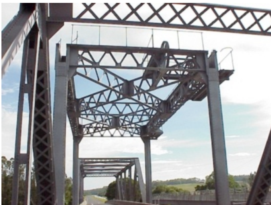
Figure 5.115 Towers of Mororo Bridge (Source: RMS)
