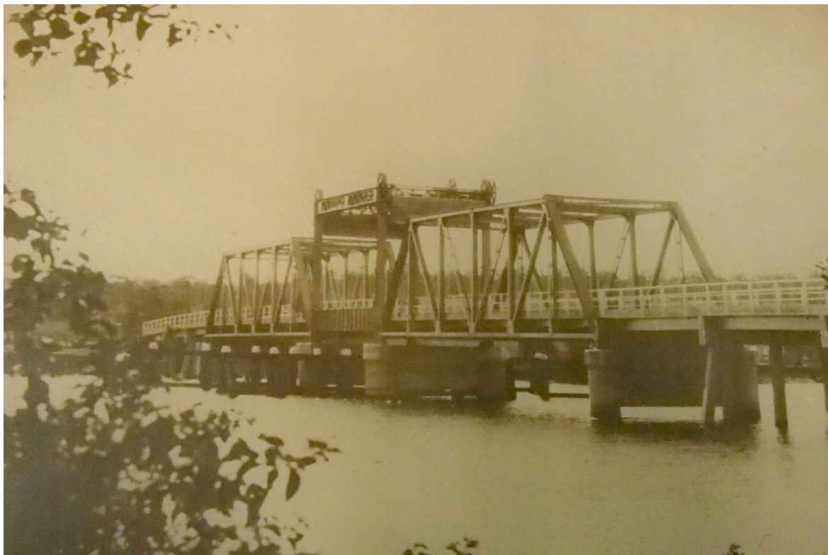
Figure 5.114 Mororo Bridge in 1935 with counterweights and ropes in place (Source: RMS photographic archives)
