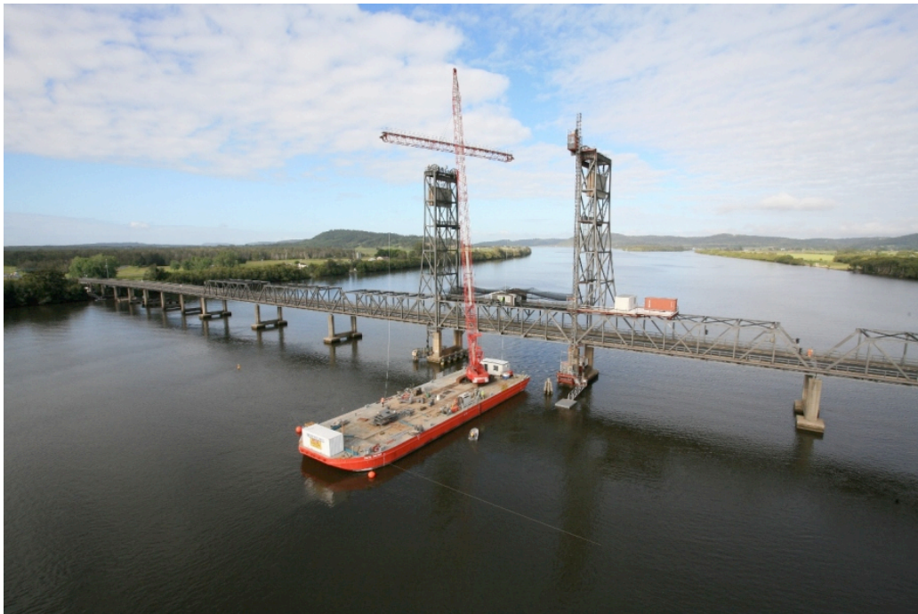
Figure 5.197 Barge and floating crane in position during access upgrading project in 2010
