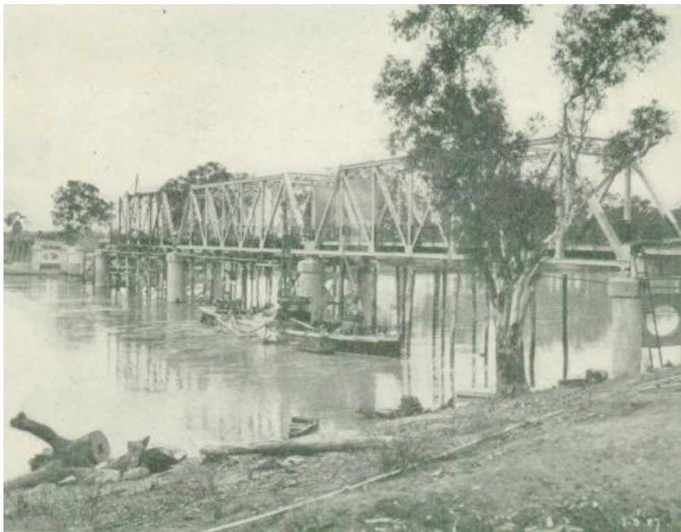
Figure 5.104 Abbotsford Bridge under construction in September 1927 (Source: PWD 1927)
