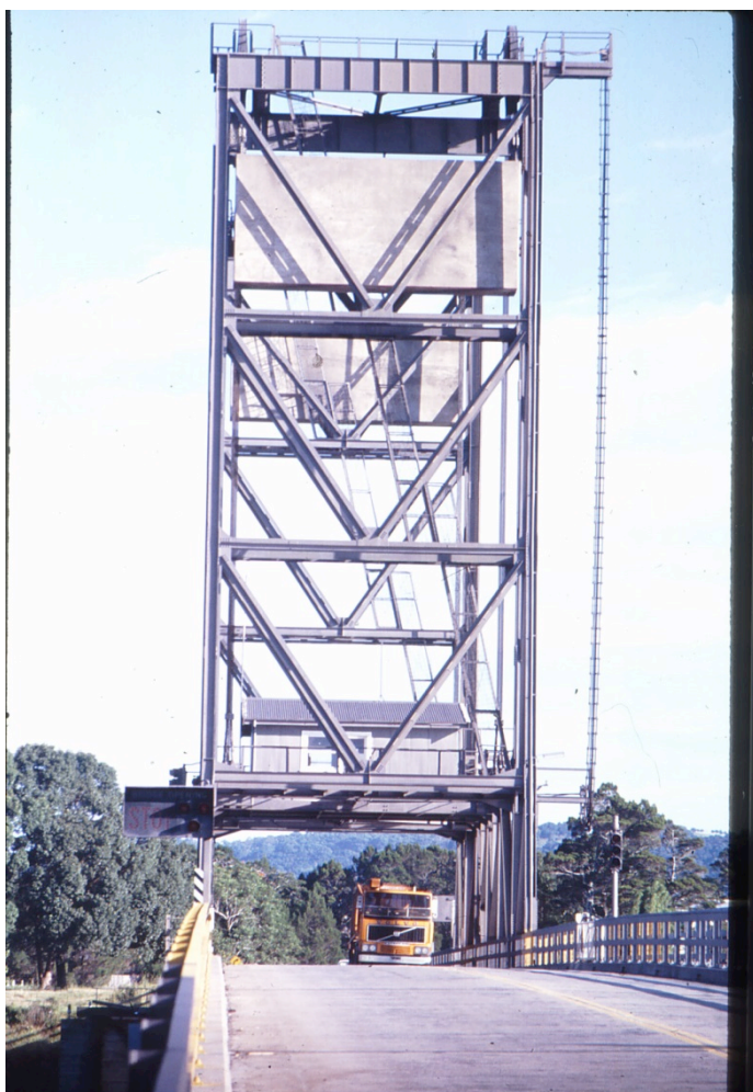
Figure 5.175 Wardell Bridge towers and counterweights
