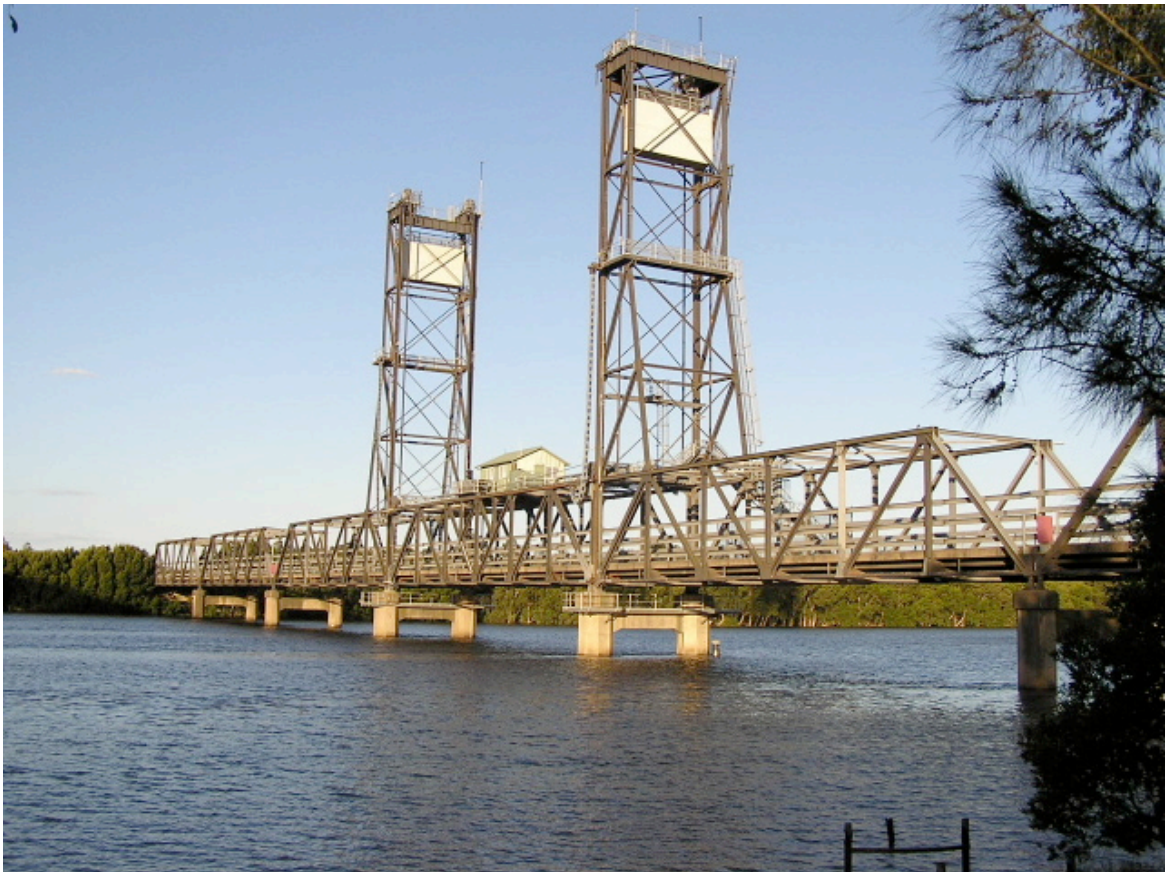
Figure 5.146 General view of Hexham Bridge
