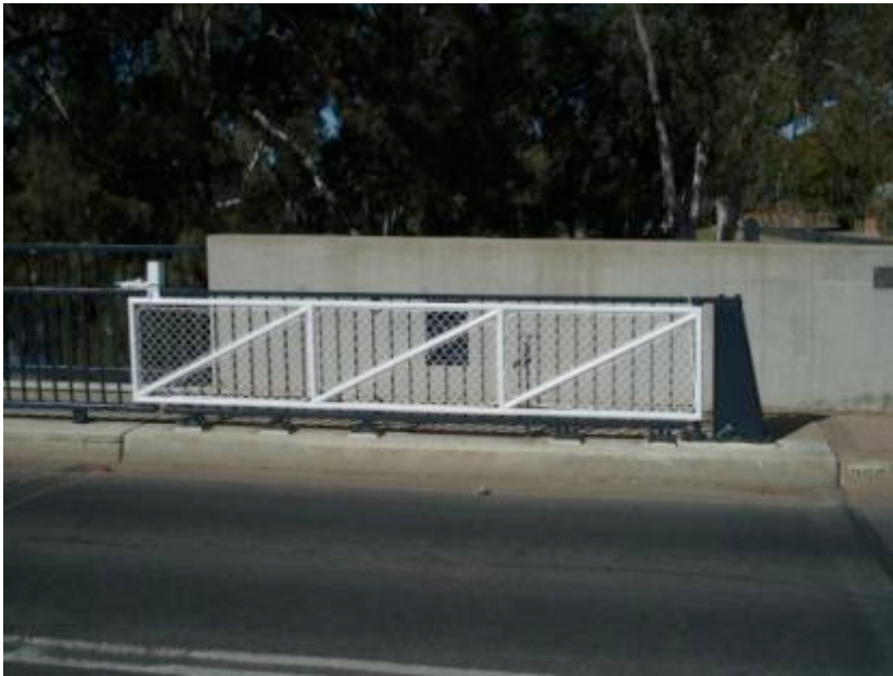
Figure 5.223 Vehicle barrier Wentworth Bridge
