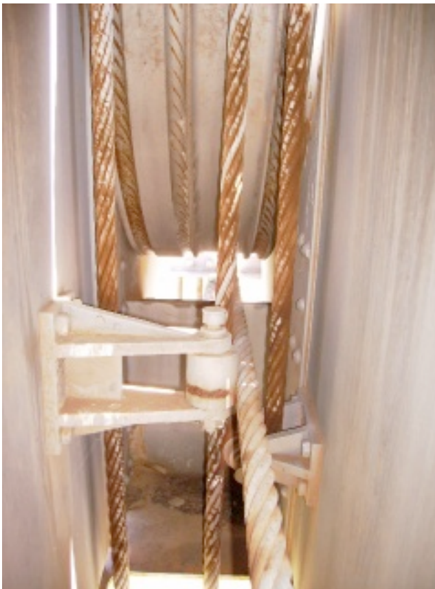
Figure 5.144 Ropes on Nyah Bridge (Source: RMS)
