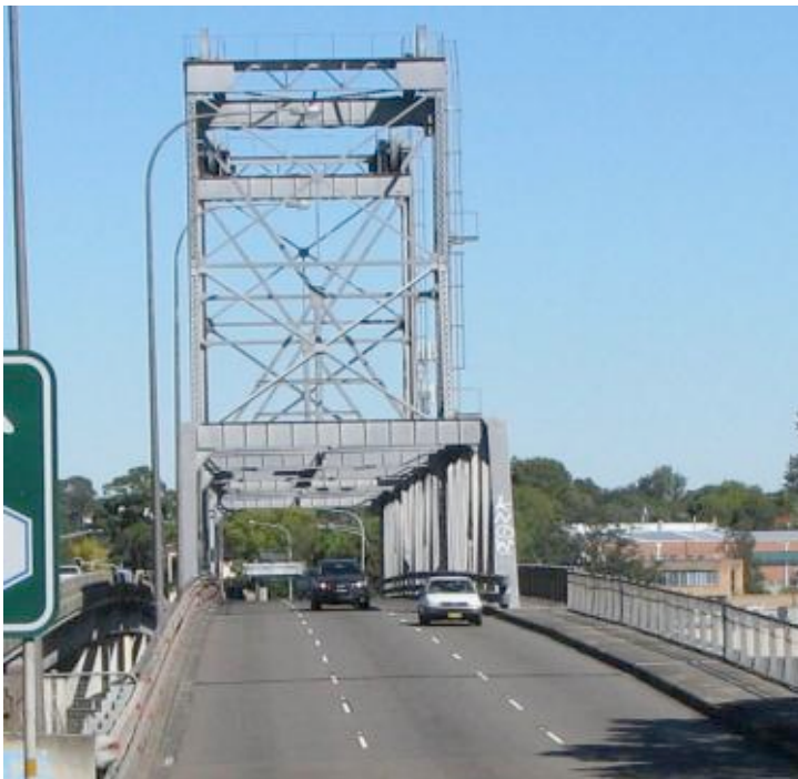
Figure 5.130 View in 2013 with counterweights removed
