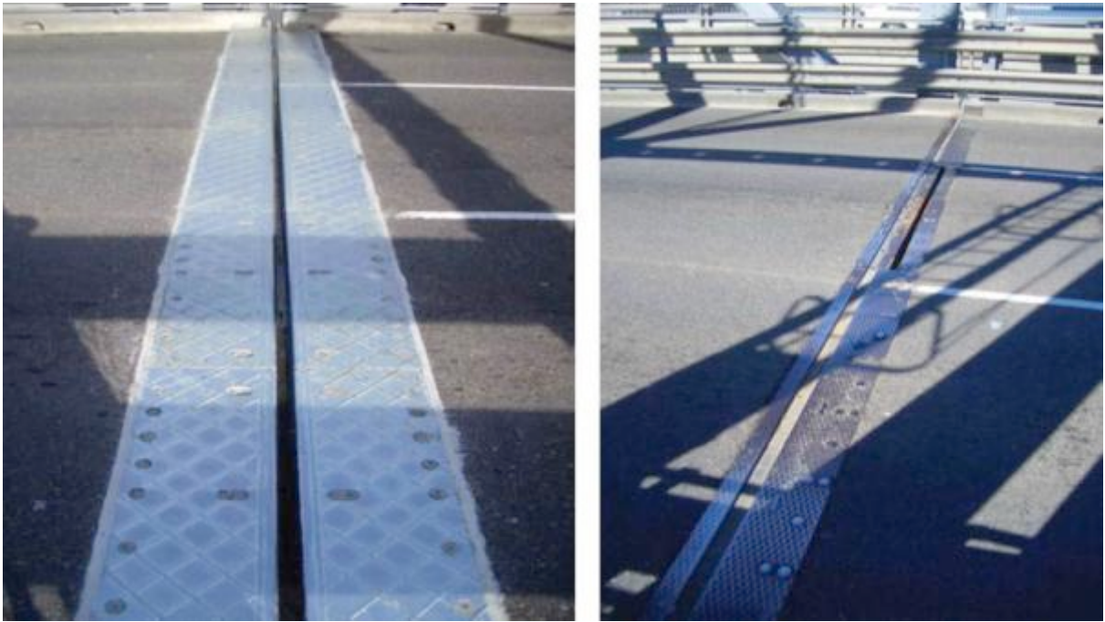
Figure 5.127 Replacement of deck joints by HMS Civils Pty Ltd
