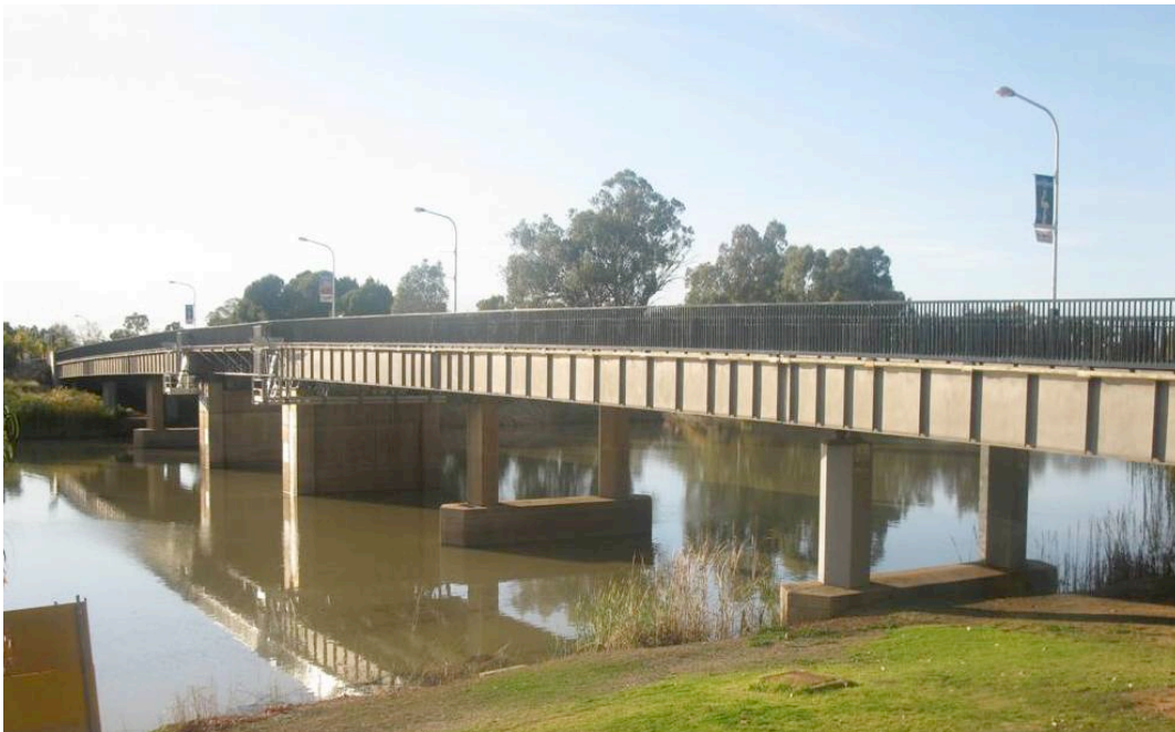
Figure 5.208 Profile view of Wentworth Bridge with lift span closed
