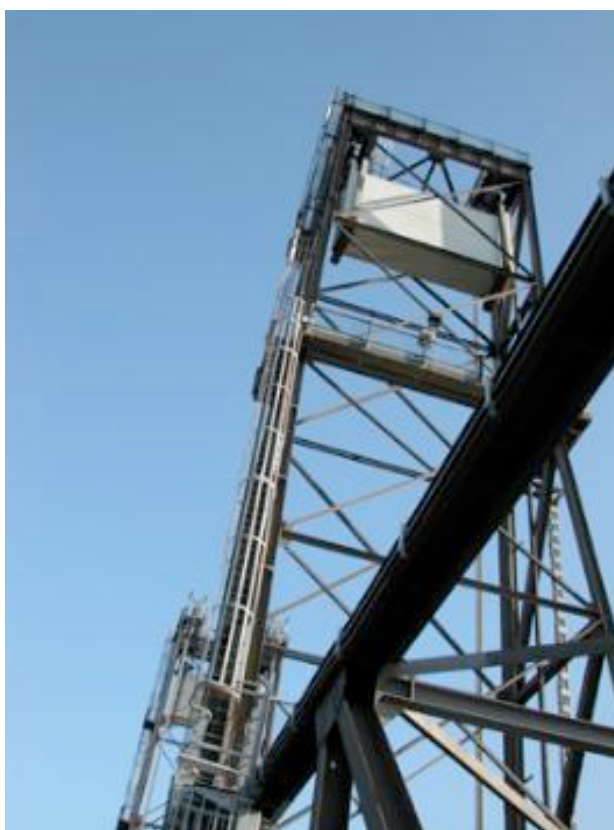
Figure 5.152 Hexham Bridge counterweight (Source: RMS)
