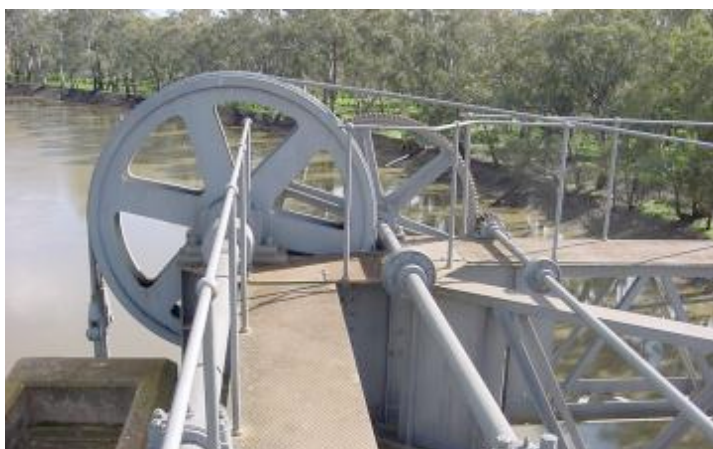
Figure 5.141 Sheaves on Nyah Bridge (Source: RMS)
