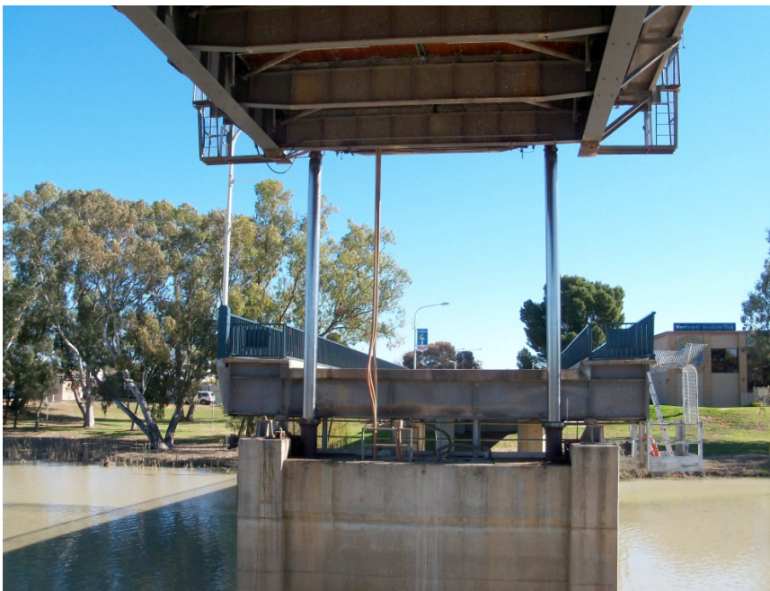
Figure 5.216 Wentworth Bridge open position
