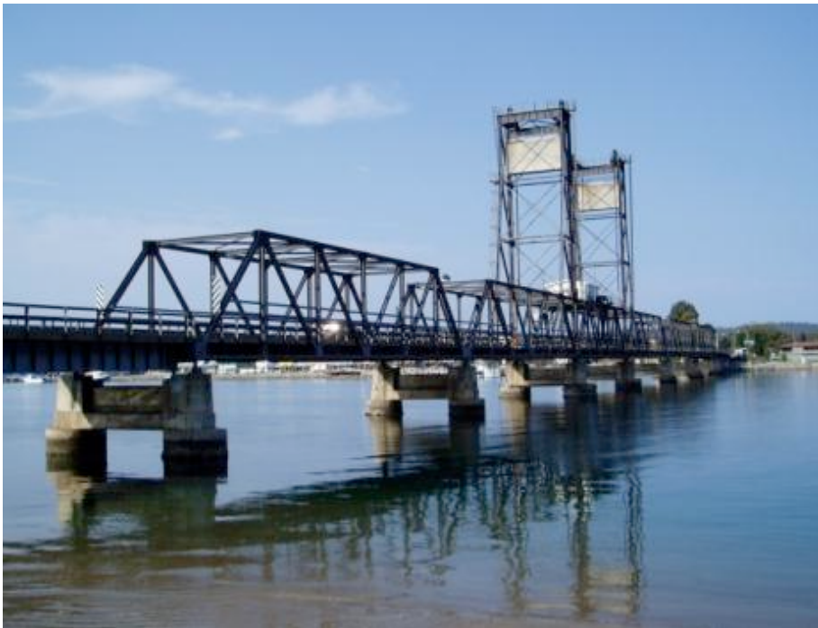
Figure 5.158 General view of Batemans Bay Bridge
