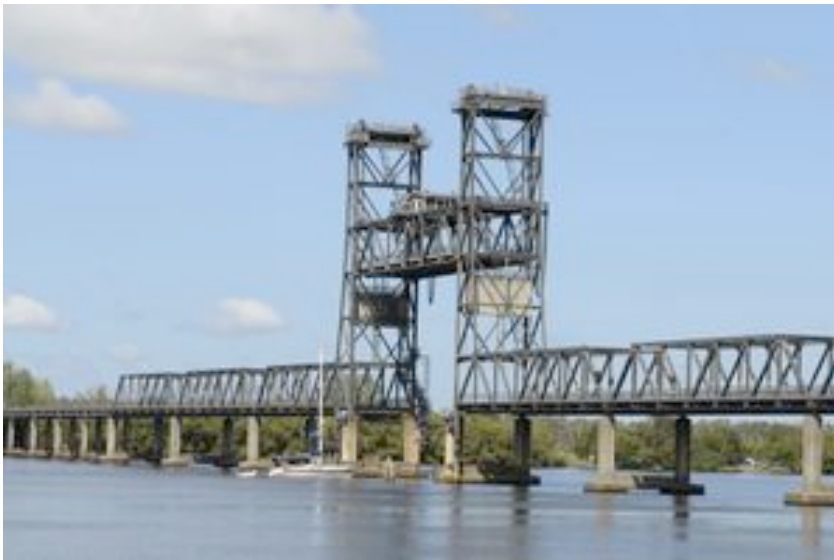
Figure 5.195 Lift span raised to allow for a yacht to pass under (Source: Daily Examiner, 27 January 2014)
