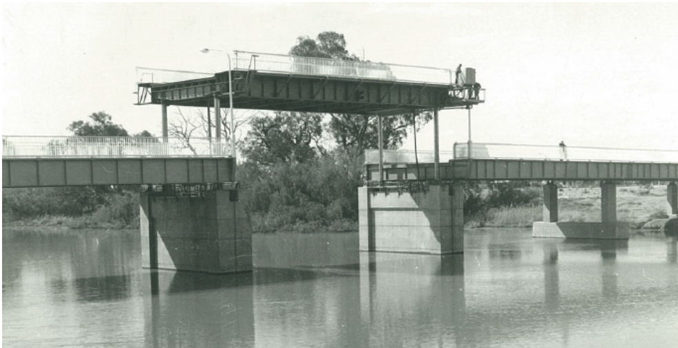
Figure 5.212 View of bridge raised to full height in December 1992. Note operator at right on lift span
