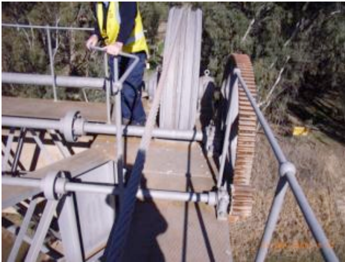
Figure 5.142 Spur wheels and sheave arrangement on Nyah Bridge
