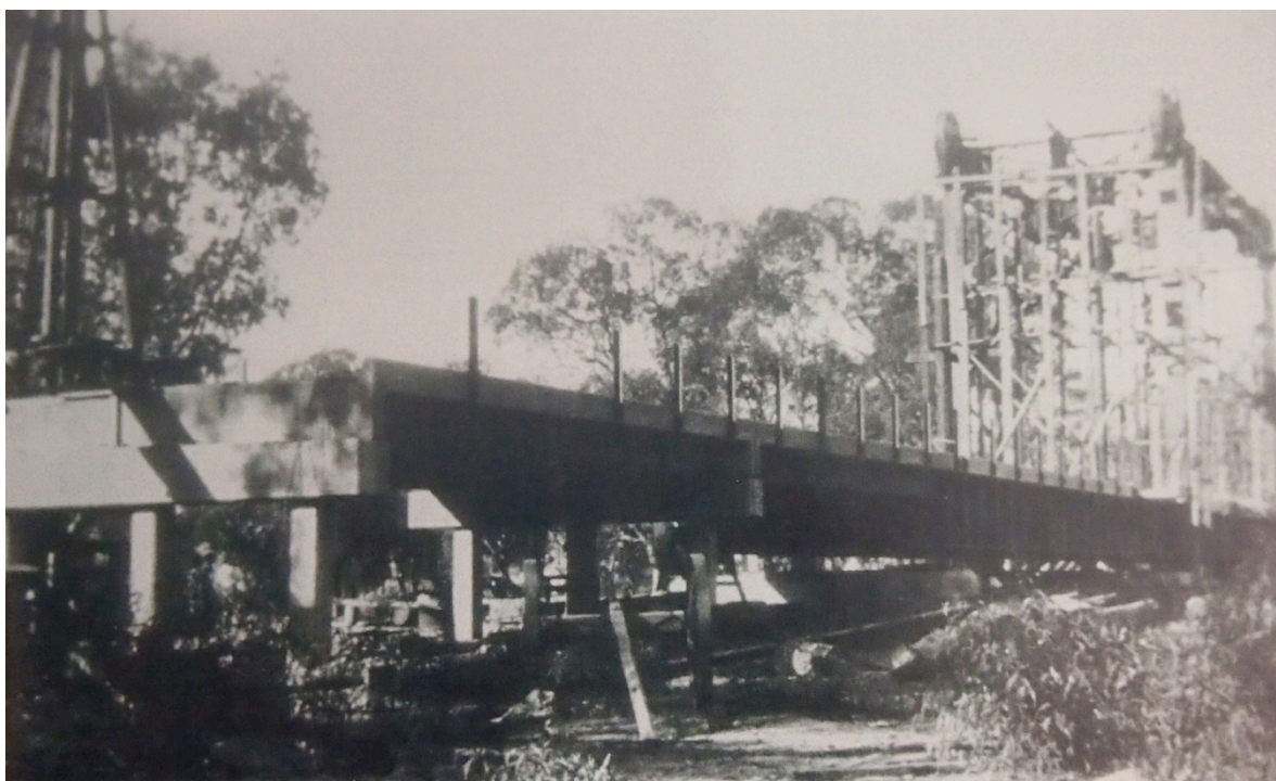
Figure 5.132 Nyah Bridge under construction (Source: Swan Hill Regional Library)
