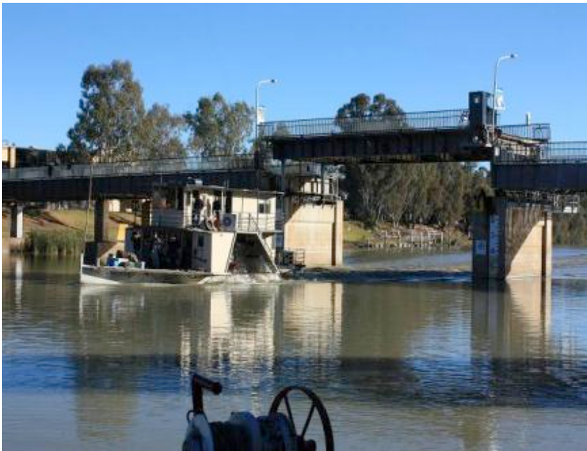
Figure 5.211 Paddle Boat “Bungunyah” passing under Wentworth Bridge with the lift span raised to half height (Source: RMS)
