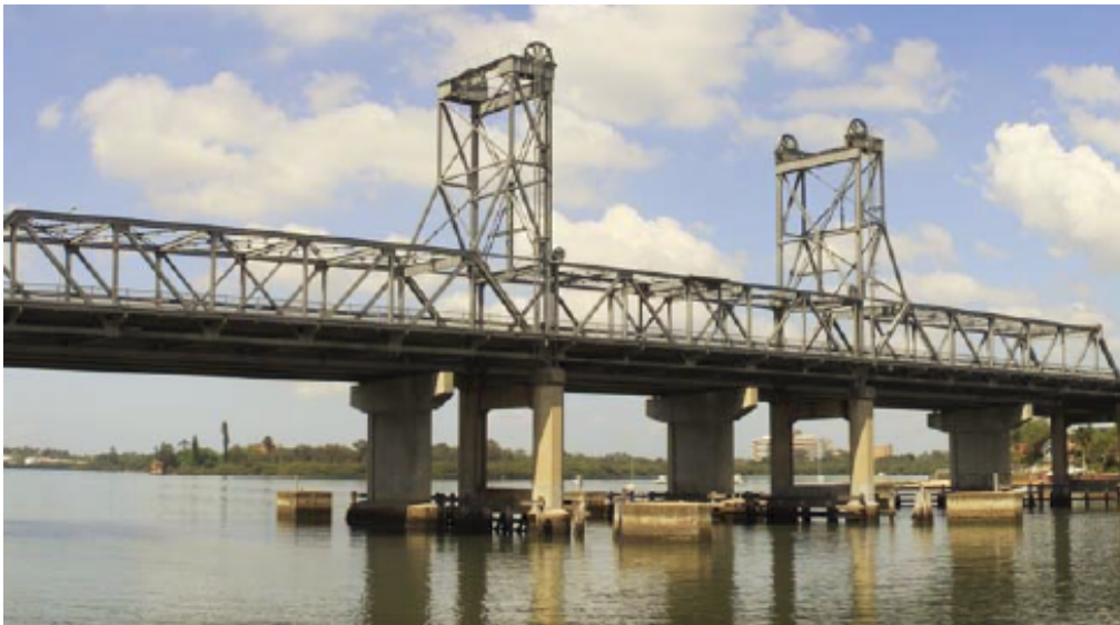
Figure 5.123 General view of Ryde Bridge in 2012 (Source: RMS Section 170 Register)
