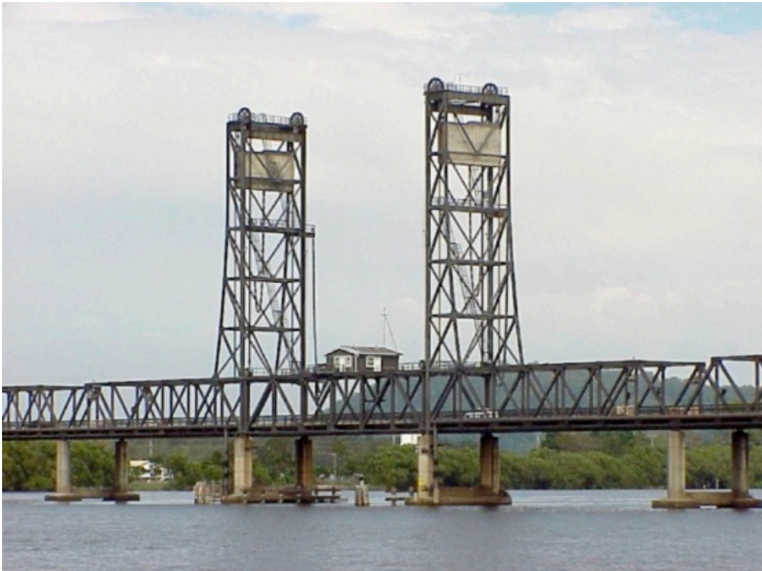
Figure 5.191 General view of Harwood Bridge
