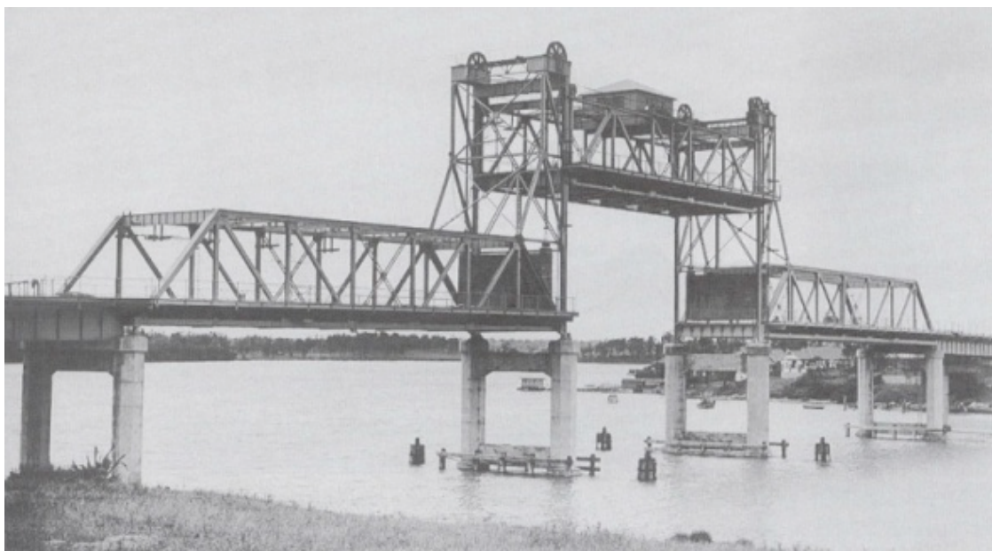
Figure 5.125 Ryde Bridge with lift span fully raised in the 1960s, note the counterweights are at rest just above deck level (Source: MCI Levy Collection, Ryde Library Service)
