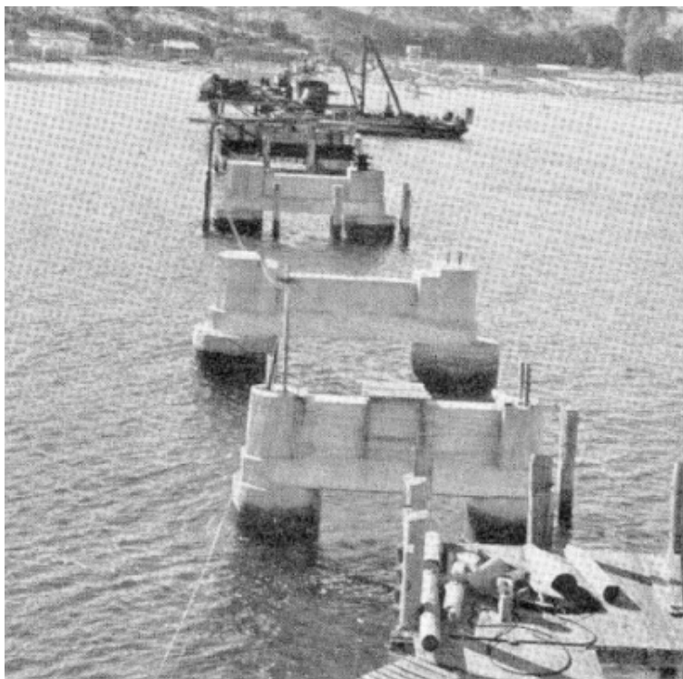
Figure 5.159 View of some of the completed piers in 1953 (Source: DMR, 1953:13)
