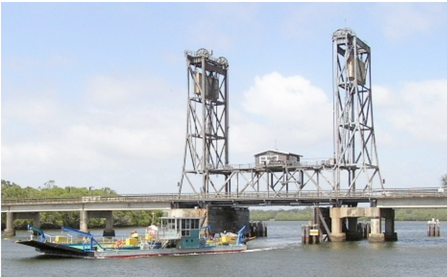
Figure 5.177 The Burns Point vehicular ferry floating beneath the bridge on its way back to Ballina after repairs
