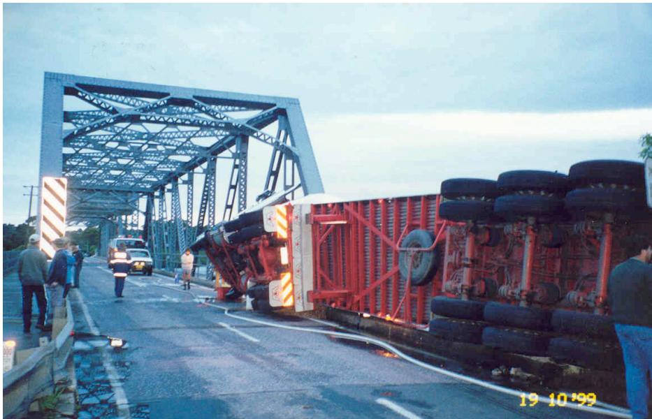
Figure 7.34 View of the overturned truck on the northern approach in October 1999 (Source: RTA Bridge File)
