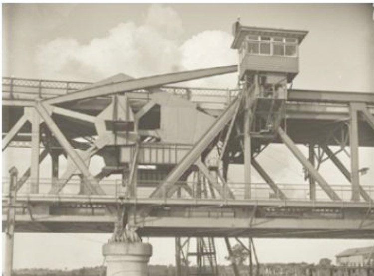
Figure 7.57 Grafton bridge mechanical components
