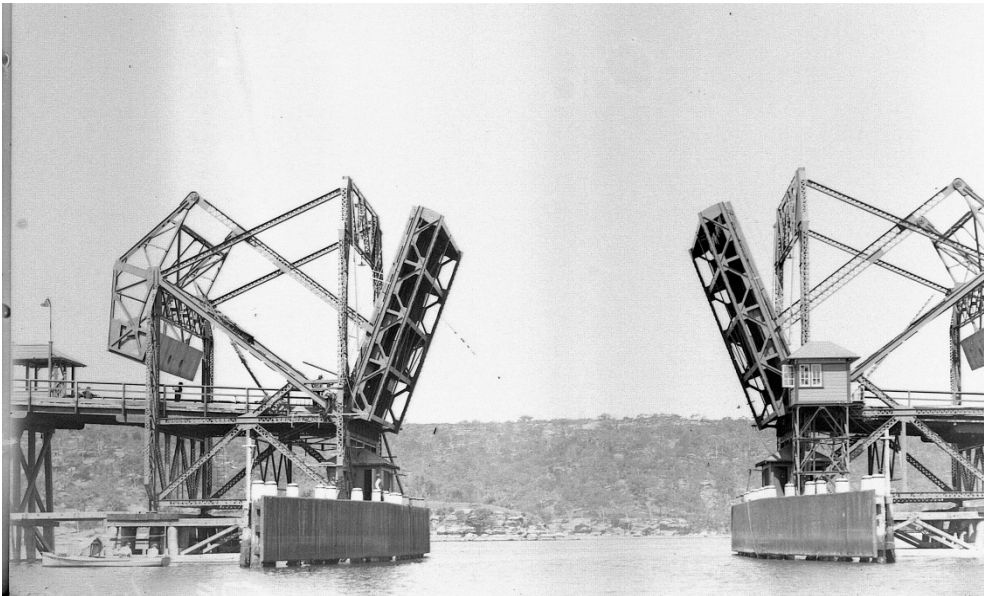
Figure 6.29 View of the first Spit Bridge raised looking east in November, 1924 (Source: MSBSR 579, RMS photographic archives). The controller’s cabin can be seen on the southern side
