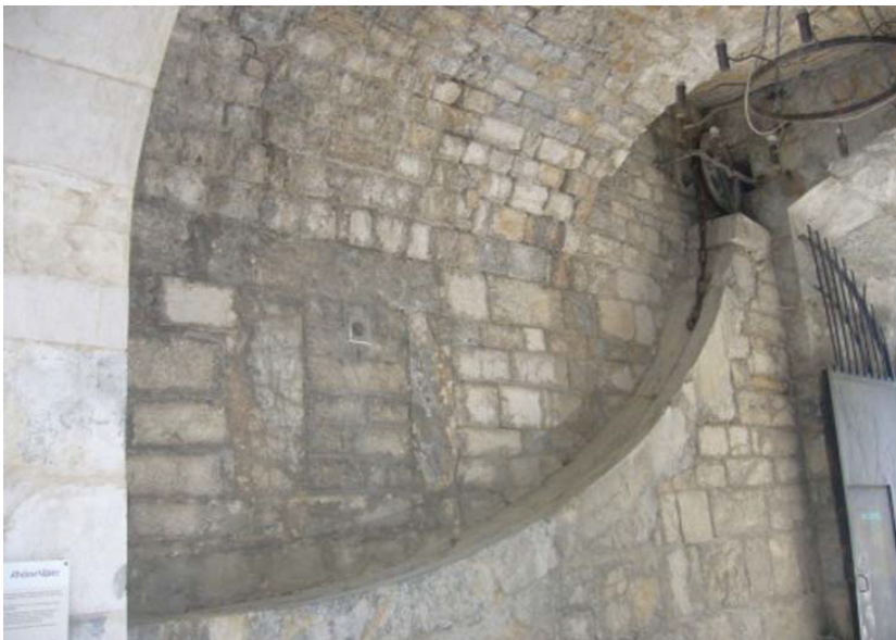
Figure 6.5 Fort l'Écluse, gate downstairs (Source: Barpi & Deakin, 2012)
