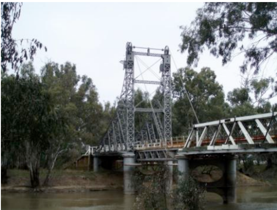
Figure 7.23 Image of Carrathool Bridge
