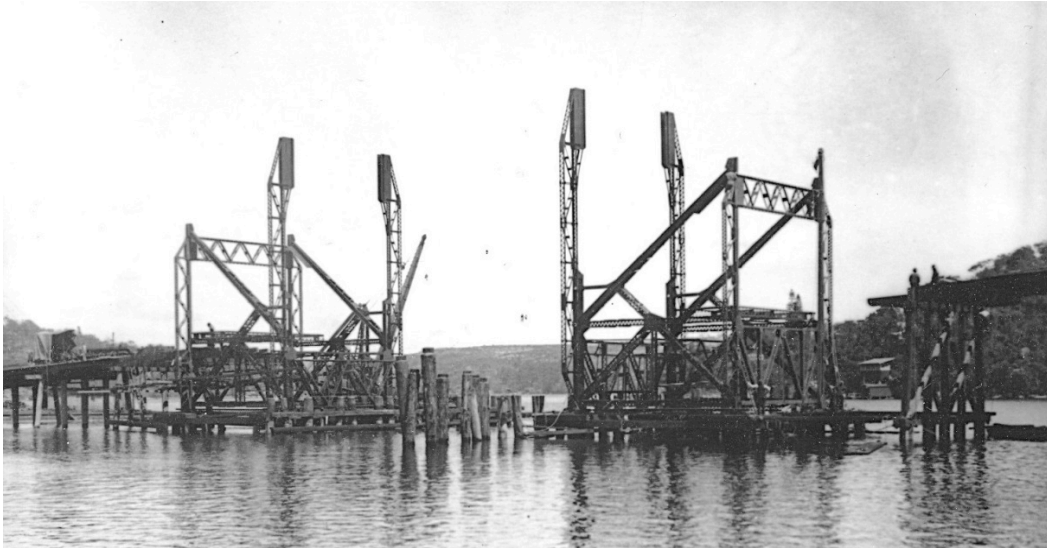
Figure 7.76 First Spit Bridge under construction in 1924 (Source: MSB 4881, RMS photographic archives)
