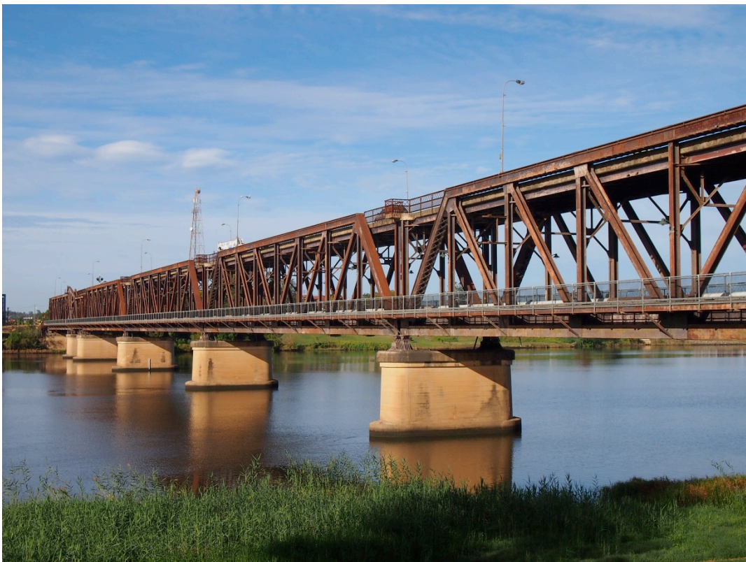
Figure 7.47 General view of Grafton Bridge looking south
