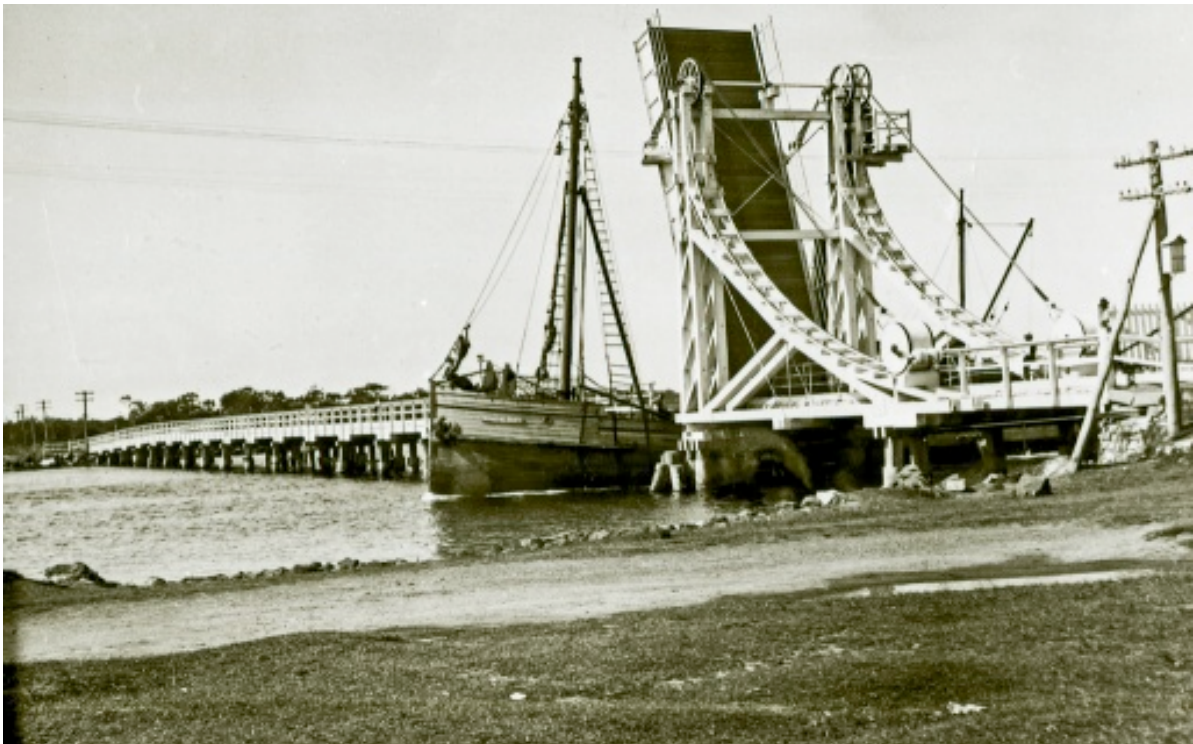
Figure 7.63 Swansea Bridge 1909 (Source: The Bert Lovett / Norm Barney Collection and Cultural Collections at the University of Newcastle)
