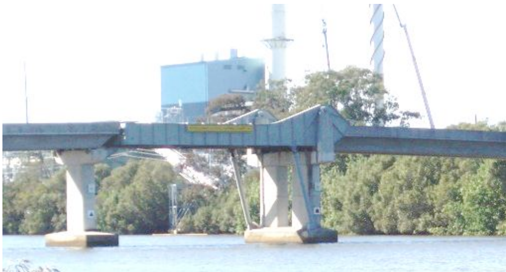
Figure 6.40 General view of Broadwater Bridge
