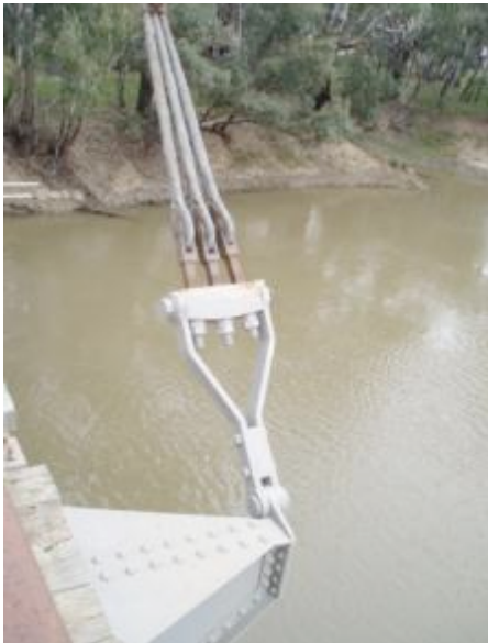
Figure 7.25 Carrathool Bridge wire rope to lift span attachment
