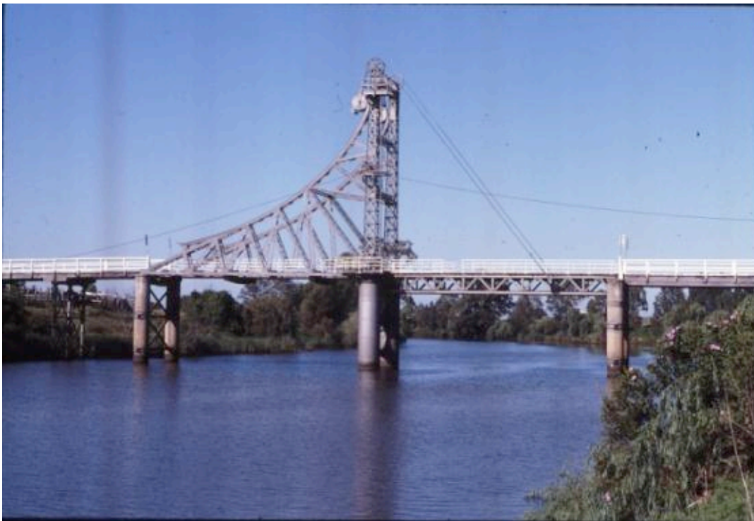
Figure 7.1 General view of Glebe Bridge
