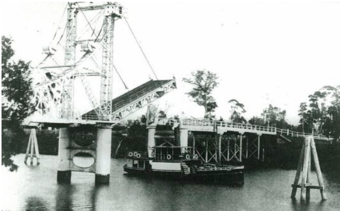
Figure 7.2 Glebe Bridge with lift span half raised (Source: Town and Country Journal 27/11/1912)
