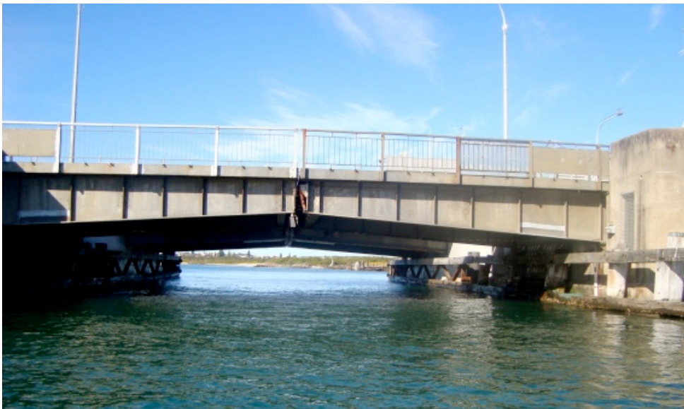
Figure 7.64 Swansea Bridge (1955) twin leaf bascule spans
