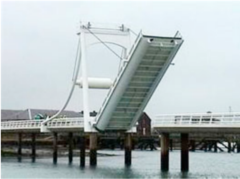
Figure 6.28 The 2011 Forton Lake Bridge, Portsmouth, UK (Source: A Torn Construction website)
