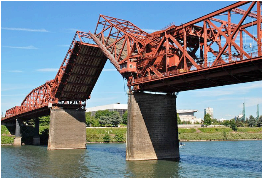
Figure 7.49 Broadway Bridge in Portland with double-leaf bascule span open (Source: Wikipedia)
