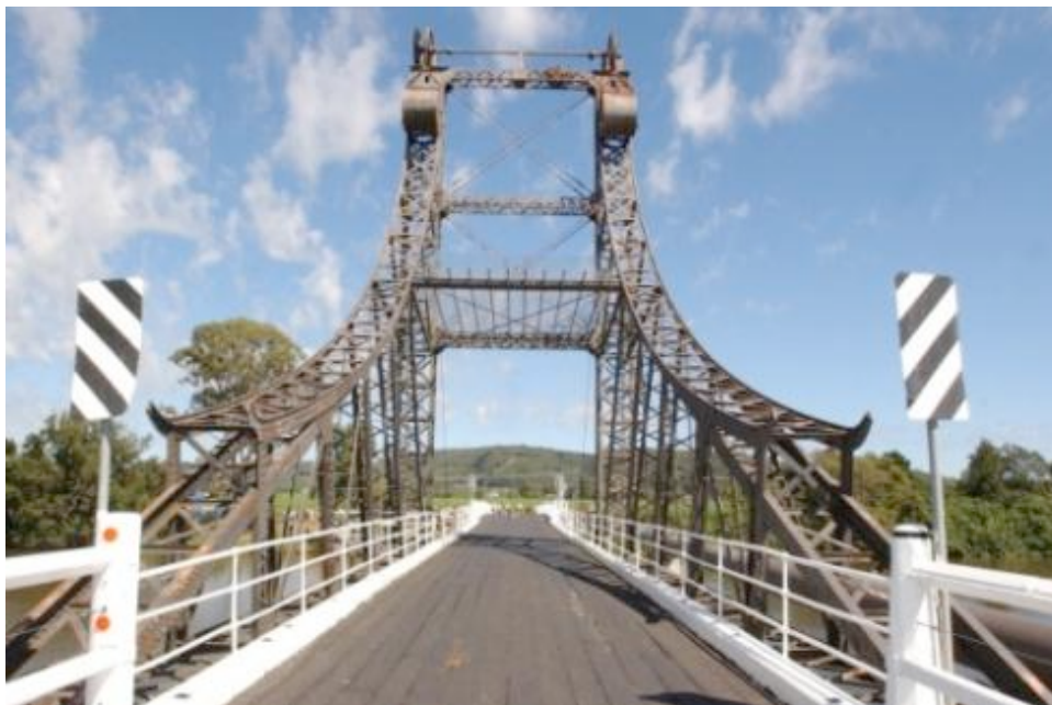
Figure 7.13 View of McFarlane Bridge along deck
