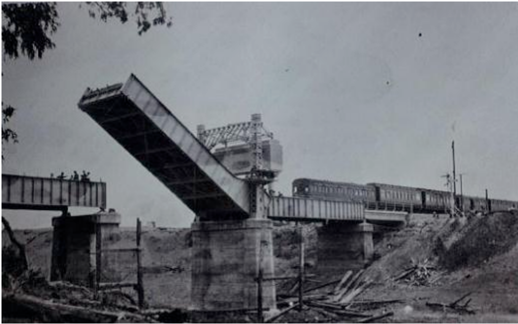
Figure 6.31 Menindee Bridge - counterweight lowered and bascule span raised, undated. The counterweight and tower were removed in 1970 (Source: SRA Archives)
