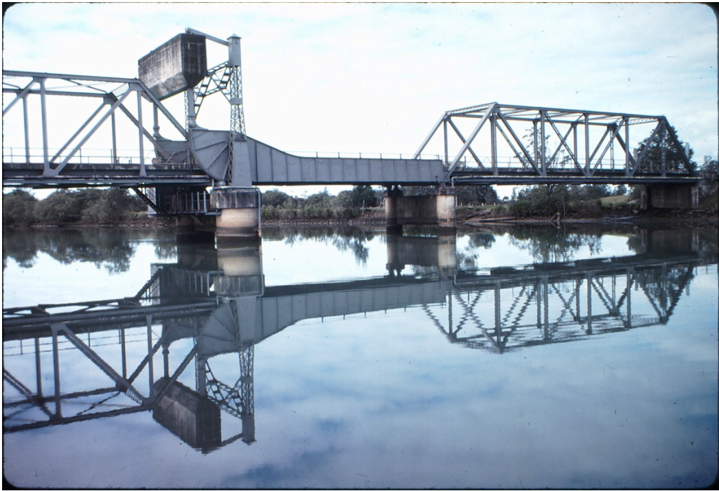
Figure 6.33 Lansdowne Bridge, replaced in 1987 (Source: RMS photographic archives)
