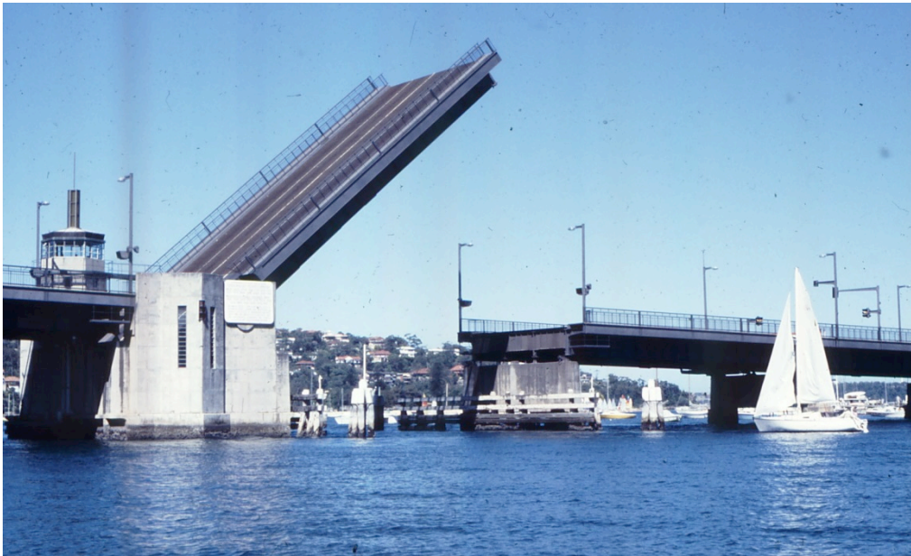
Figure 7.74 Spit Bridge with bascule span in the open position in 2002 (Source: RMS photographic archives)
