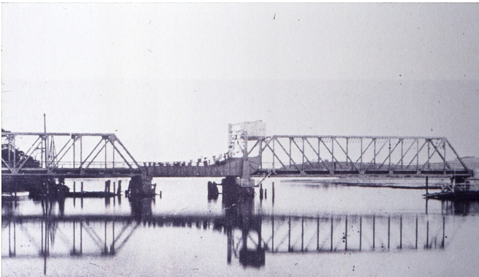
Figure 7.32 Narooma Bridge with bascule and tower wrapped with bunting at the formal opening (Source: RMS photographic archives)
