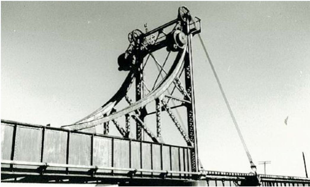
Figure 6.27 Shea's Creek railway bridge, Alexandria replaced in 1985 (Source: SRA Archives)
