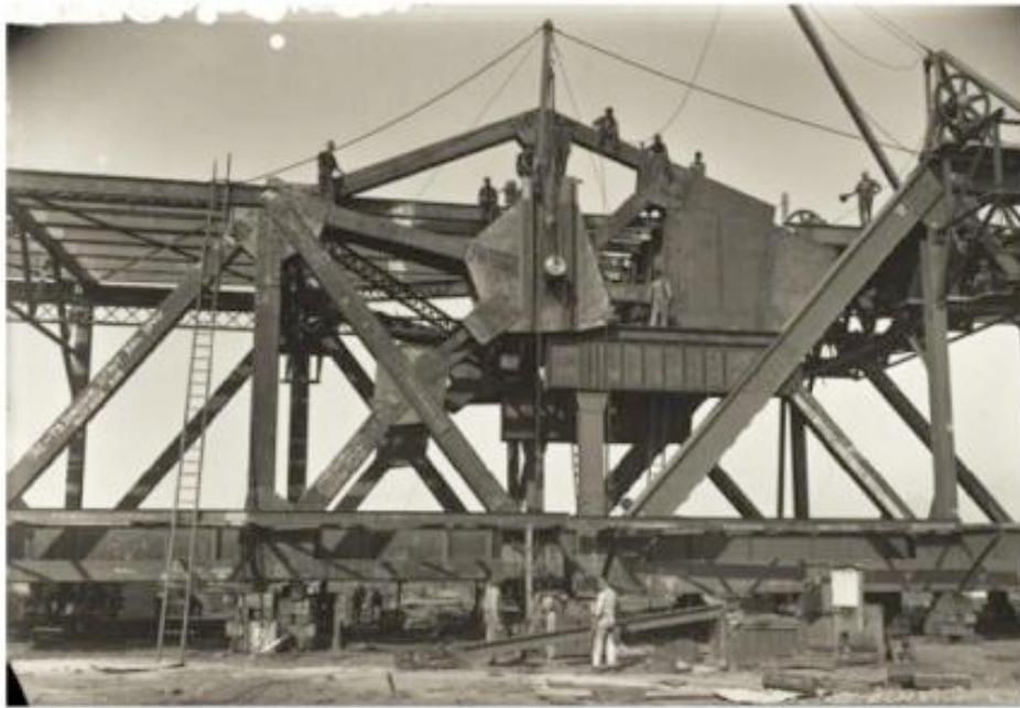
Figure 6.36 Trial assembly of Grafton Bridge
