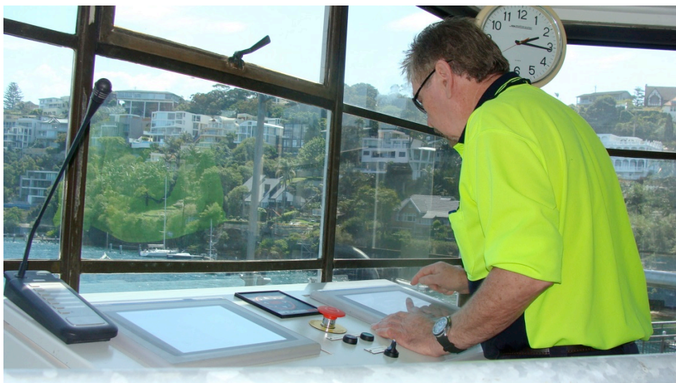
Figure 7.82 Operator using new touch screen controls installed as part of 2012 upgrade
