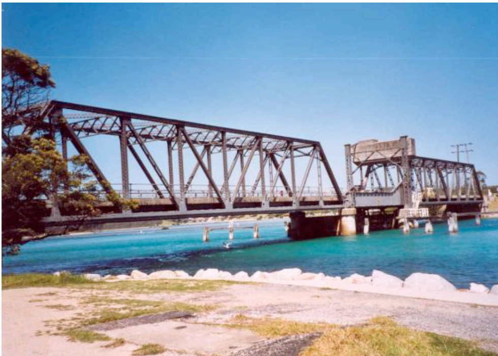
Figure 7.30 General view of Narooma Bridge with former ferry ramp in foreground
