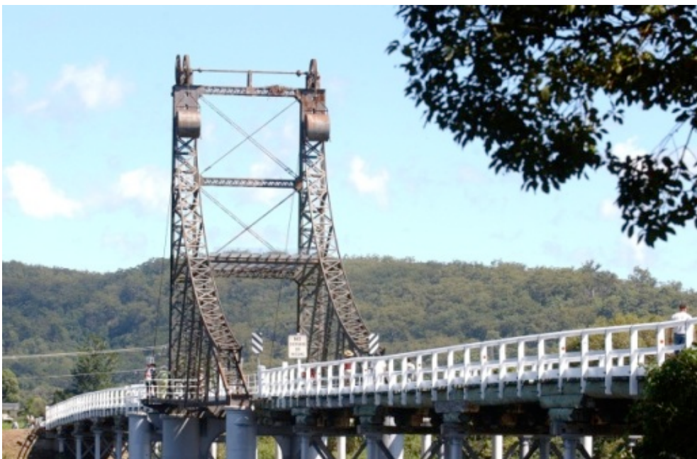
Figure 7.9 General view of McFarlane Bridge
