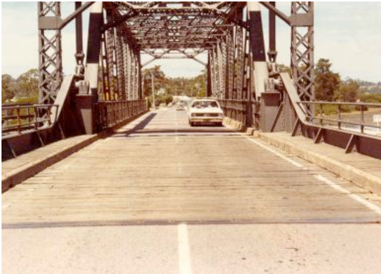
Figure 7.39 Original timber deck of bridge
