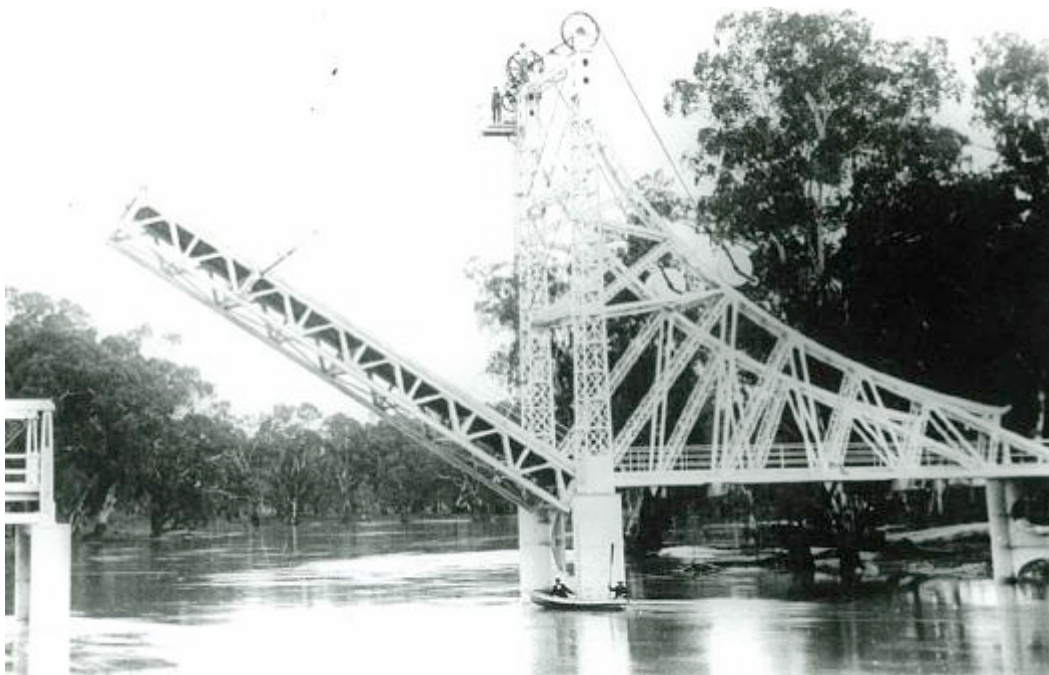
Figure 6.24 Lift span half raised on Darlington Point Bridge over the Murrumbidgee River (undated). Note operators on landing near top of track span (Source: RMS photographic archives)
