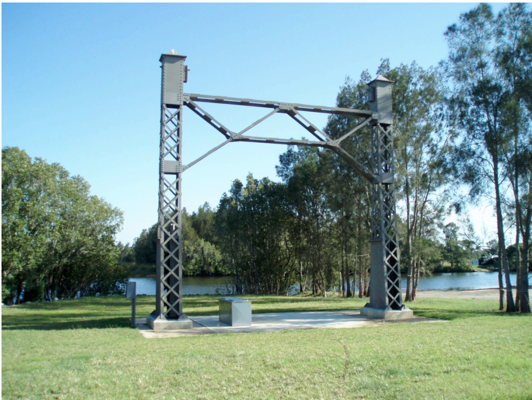
Figure 6.34 Portal frame of the Lansdowne Bridge erected in a park in Cooperbrook near the former bridge site
