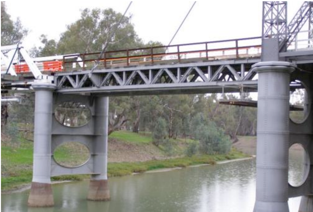
Figure 7.24 Carrathool Bridge Bascule Span
