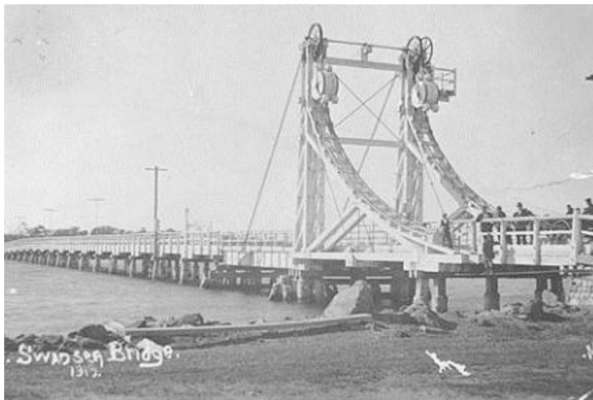
Figure 6.22 First Swansea Bridge replaced in 1955 (Source: Digital Hunter, Newcastle Library)
