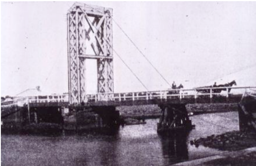
Figure 6.18 Shea's Creek Bridge (Source: Don Fraser collection, RMS archives)
