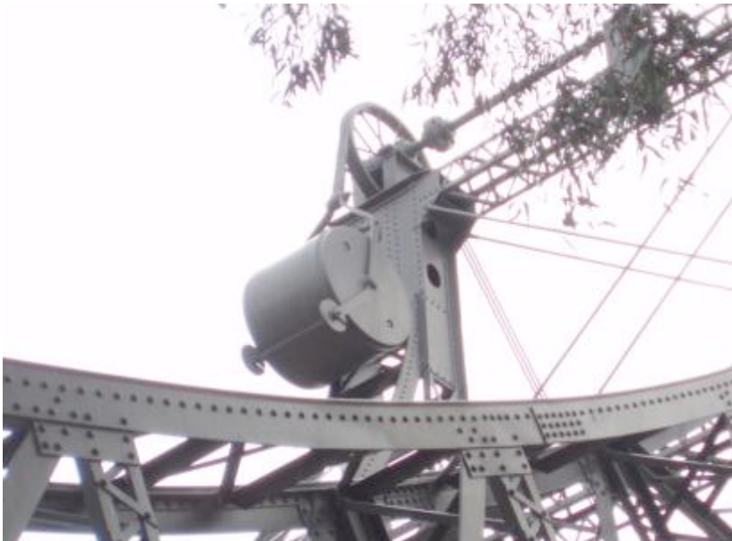
Figure 7.29 Balance weight and cradle for Carrathool Bridge
