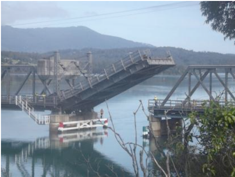
Figure 7.33 Image of bridge during opening (Source: RMS photographic archives)
