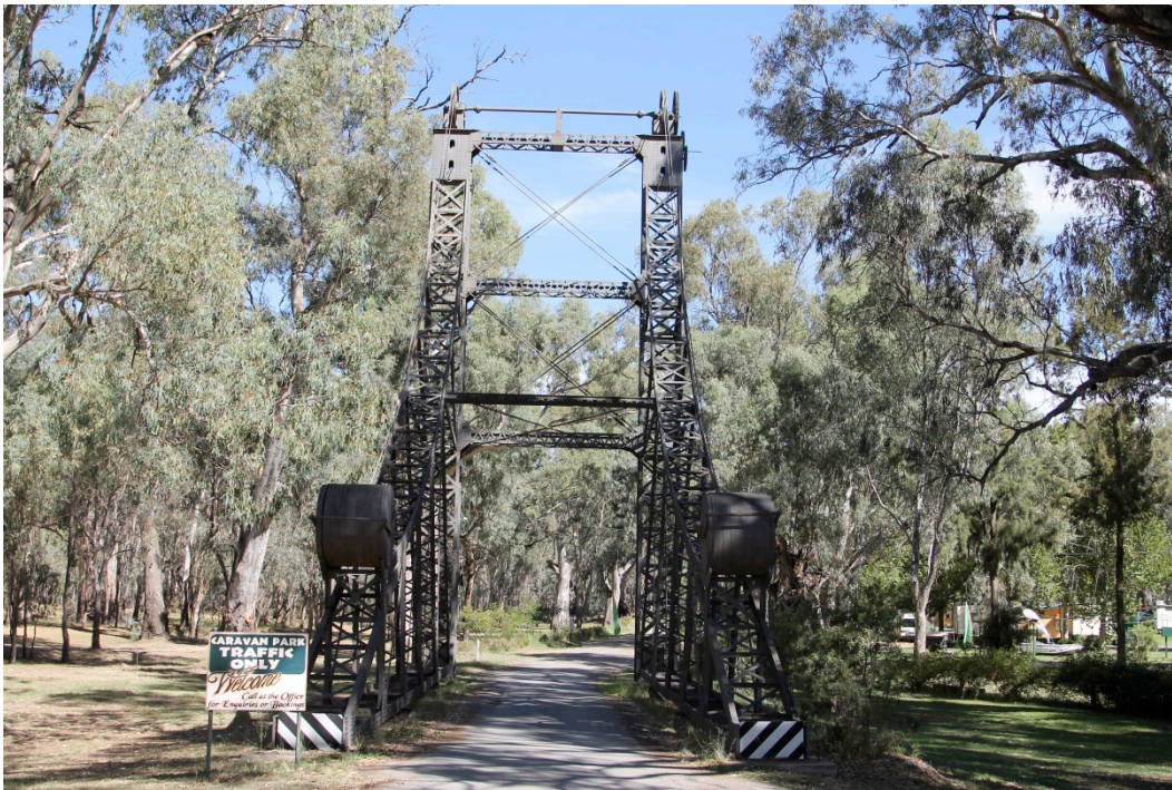
Figure 6.25 Following its replacement the Darlington Point Bridge track span was reconstructed at the entrance to Darlington Point Caravan Park (Source: Fraser, 1990)
