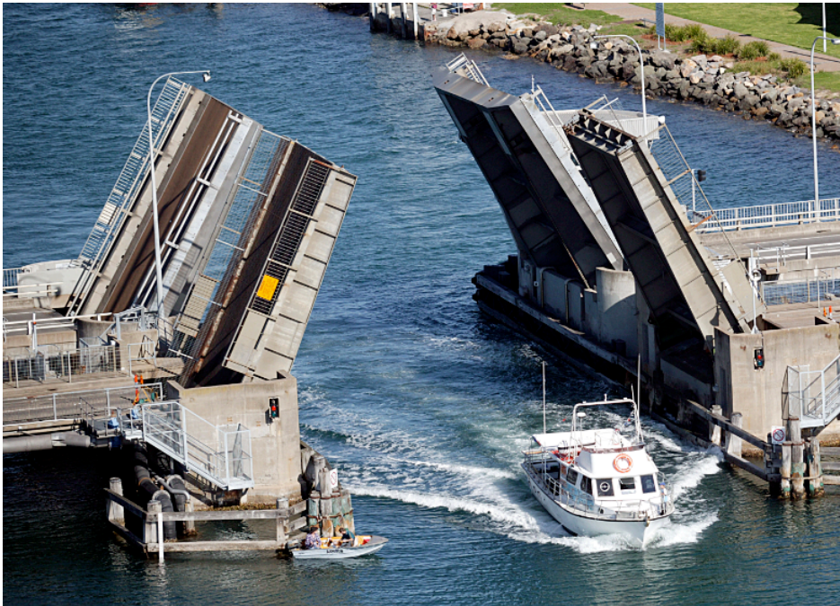
Figure 7.62 The two Swansea Bridges raised for a charter fishing boat in 2013. Swansea Bridge (1955) is in the foreground
