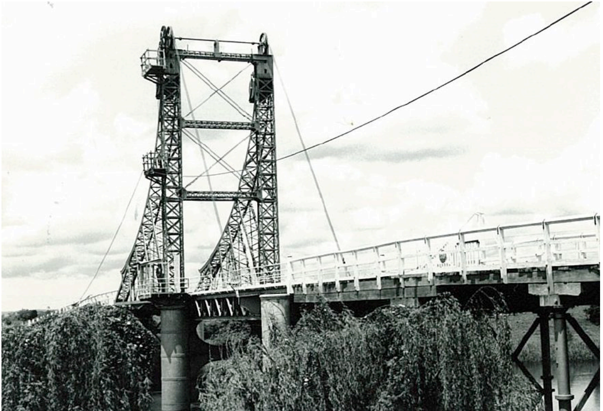
Figure 7.3 Image of Glebe Bridge with tie-back cables (Source: RMS bridge file)
