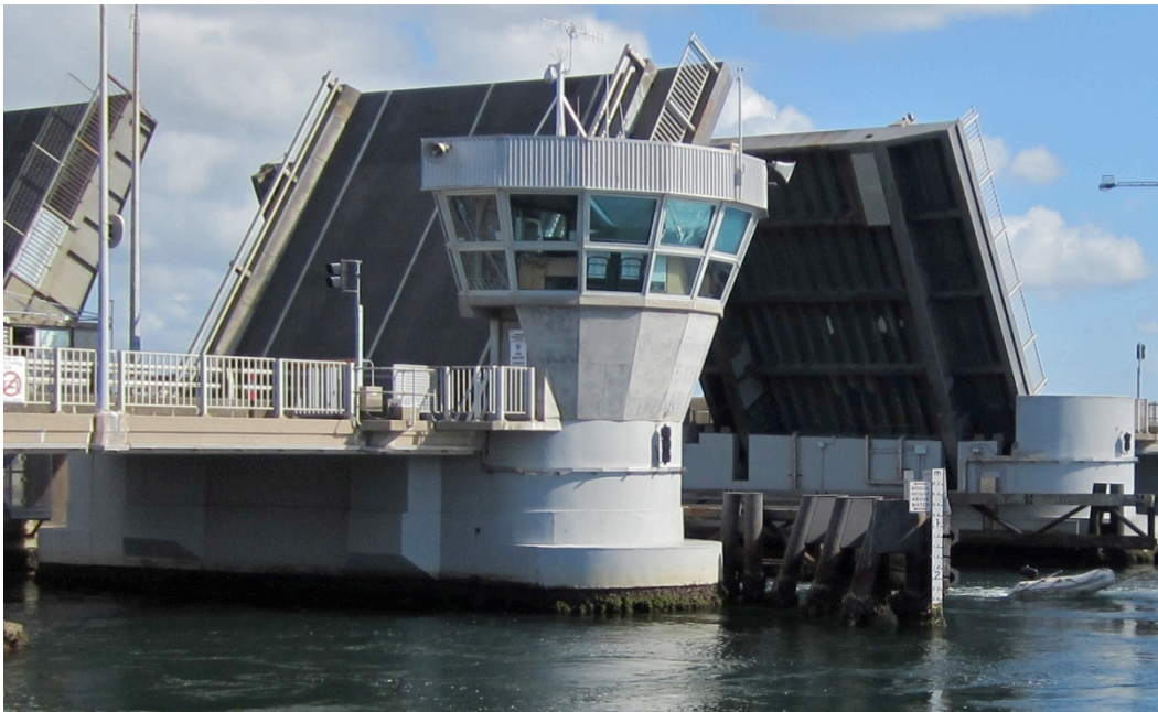
Figure 7.93 Control tower of Swansea Bridge (1989)
