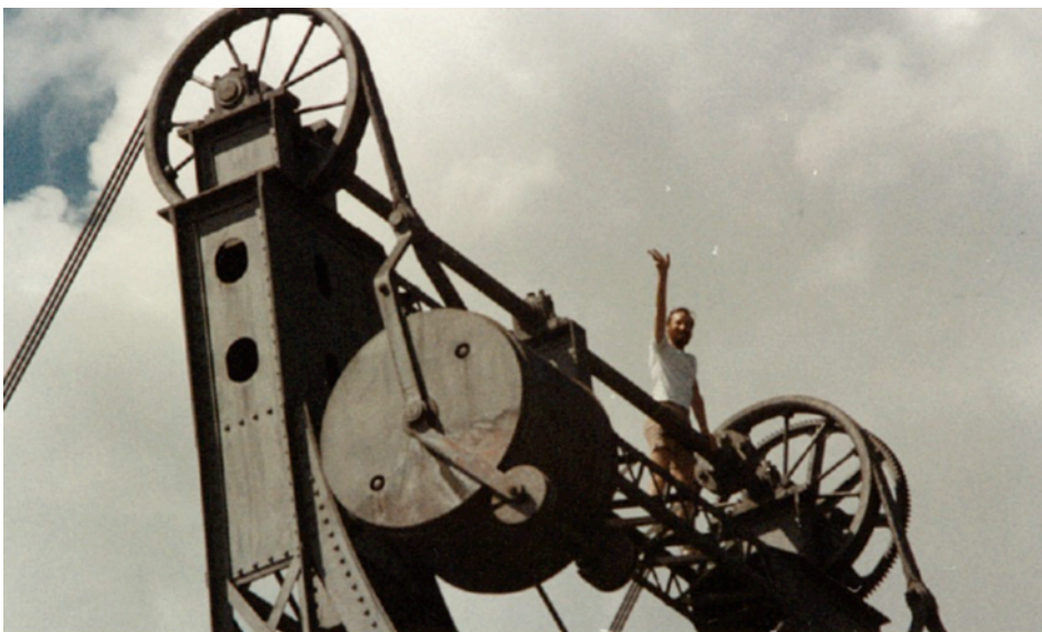
Figure 7.26 Sheaves and counterweights – with figure for scale
