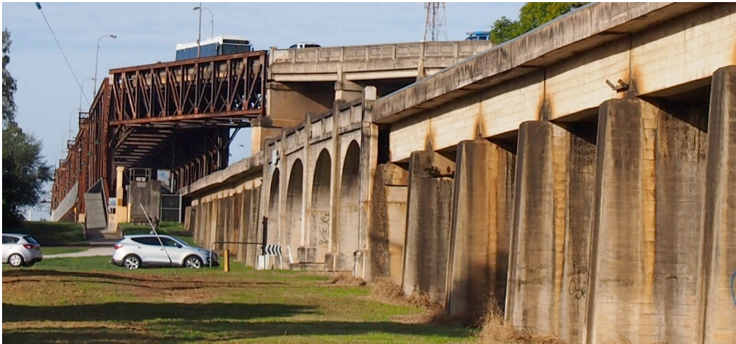
Figure 7.52 View of concrete railway viaduct extending straight from the truss spans. The road approach span piers are angled or “bent” at deck level leading on to the truss spans
