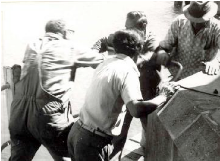
Figure 7.38 View of four men winding down the span at high gear in 1967
