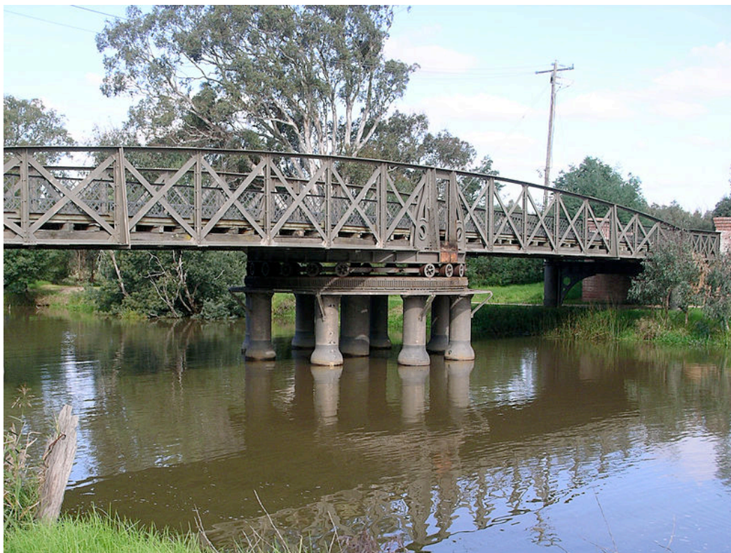
Figure 8.16 Sale Swing Bridge, Victoria in closed position
