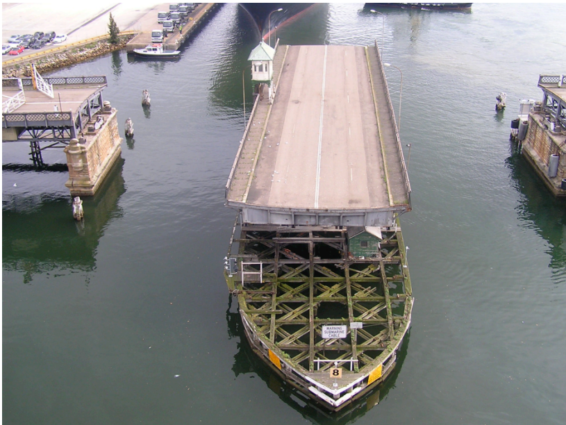
Figure 9.8 View looking north of the bridge with swing span in open position, fender in foreground and rest piers lining the channels to each side
