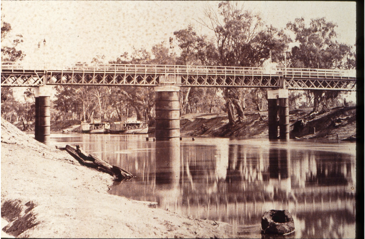
Figure 8.7 Hay Swing Bridge in closed position, undated (Source: Hay Historical Society)
