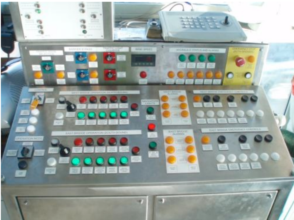
Figure 10.4 Control panel upgrade Swansea Bridge
