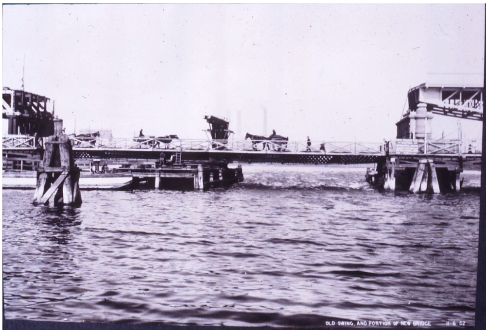
Figure 8.6 First Pyrmont Bridge built 1857, swing span at Pyrmont end, photo taken during construction of the 1902 bridge (Source: RMS, Government Printer)
