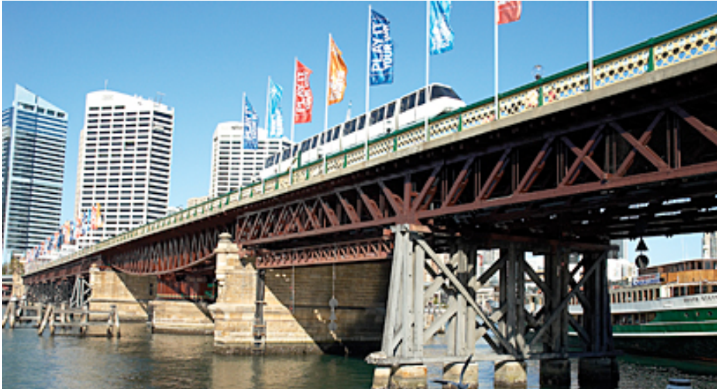
Figure 8.14 Pyrmont Bridge in closed position
