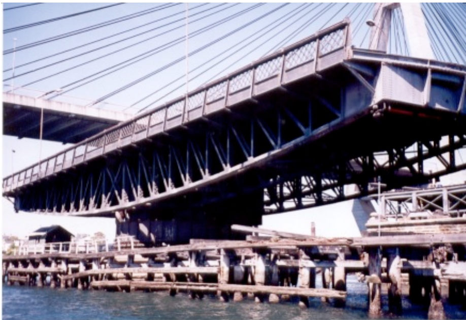
Figure 9.11 Detail of swing span in open position
