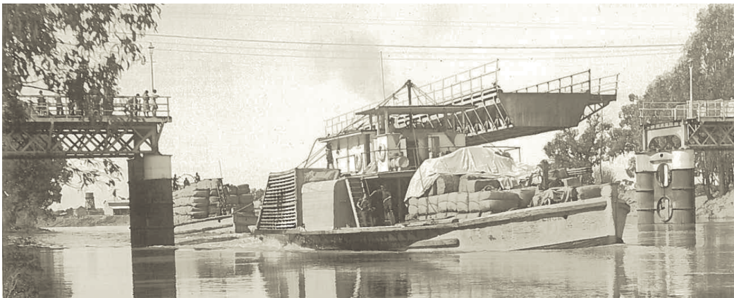
Figure 8.2 Hay Bridge opened to allow passage of the steamer Ulonga with barge in tow in 1932 (Source: Brown Collection, Hay Historical Society)
