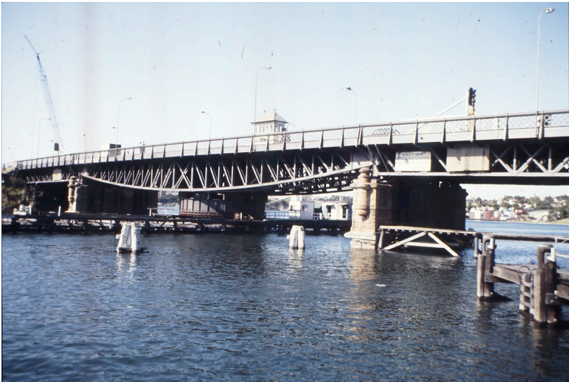
Figure 9.1 General view of Glebe Island Bridge in 1993 (Source: RMS)
