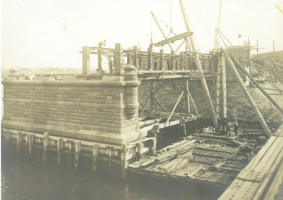
Figure 9.5 Rozelle side rest pier and approach span under construction in 1902 (Source: RMS photographic archives)
