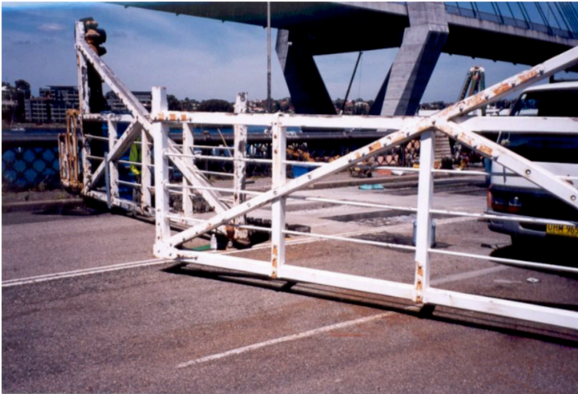
Figure 9.22 Glebe Island Bridge vehicle and pedestrian gates
