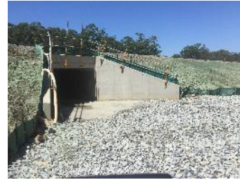
Plate 10: Design features and construction progress for Burkes Lane fauna underpass. Photo on top row was taken during spring 2014 sampling and photos on the bottom row taken during summer/autumn 2015 sampling.
