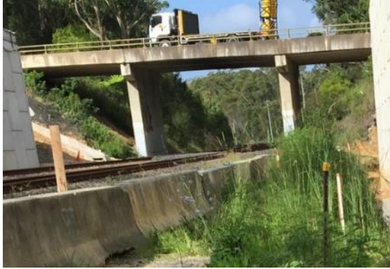
Plate 1: Habitat adjoining railway corridor underpass (ch.61800) on east side. Habitat was similar on both sides of the alignment.
