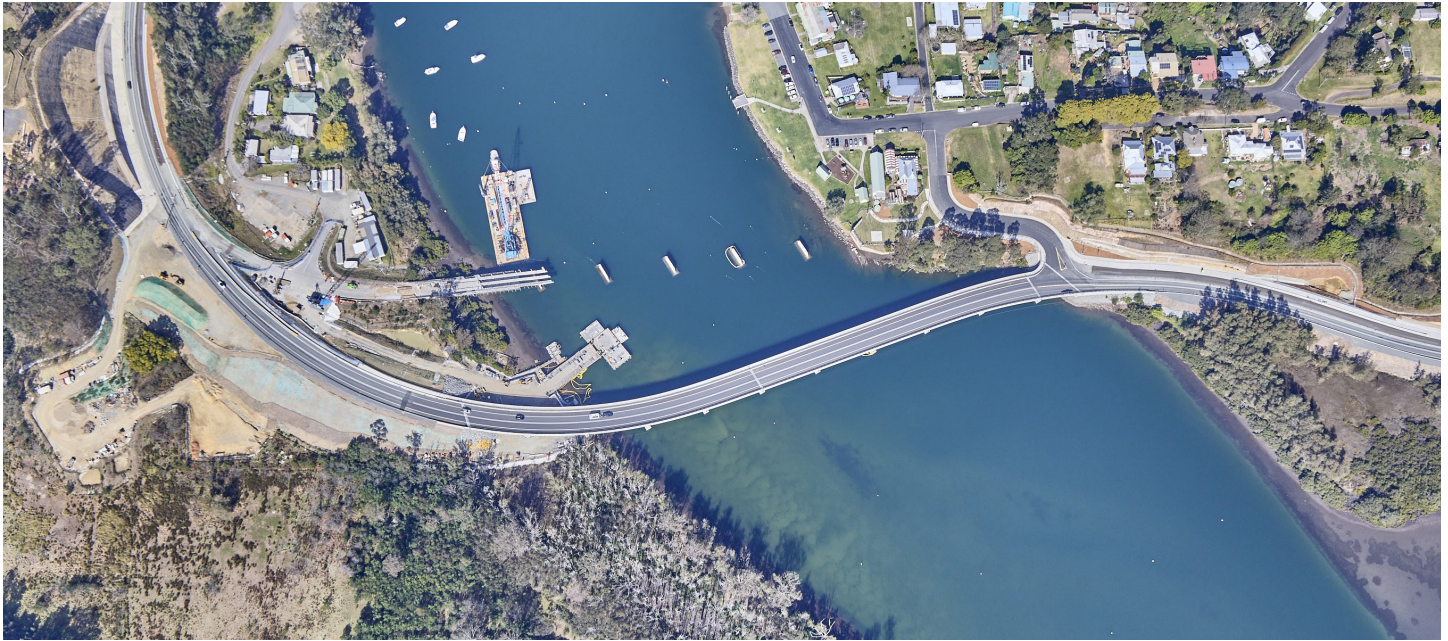
Aerial view of Nelligen Bridge Replacement project, August 2023.
