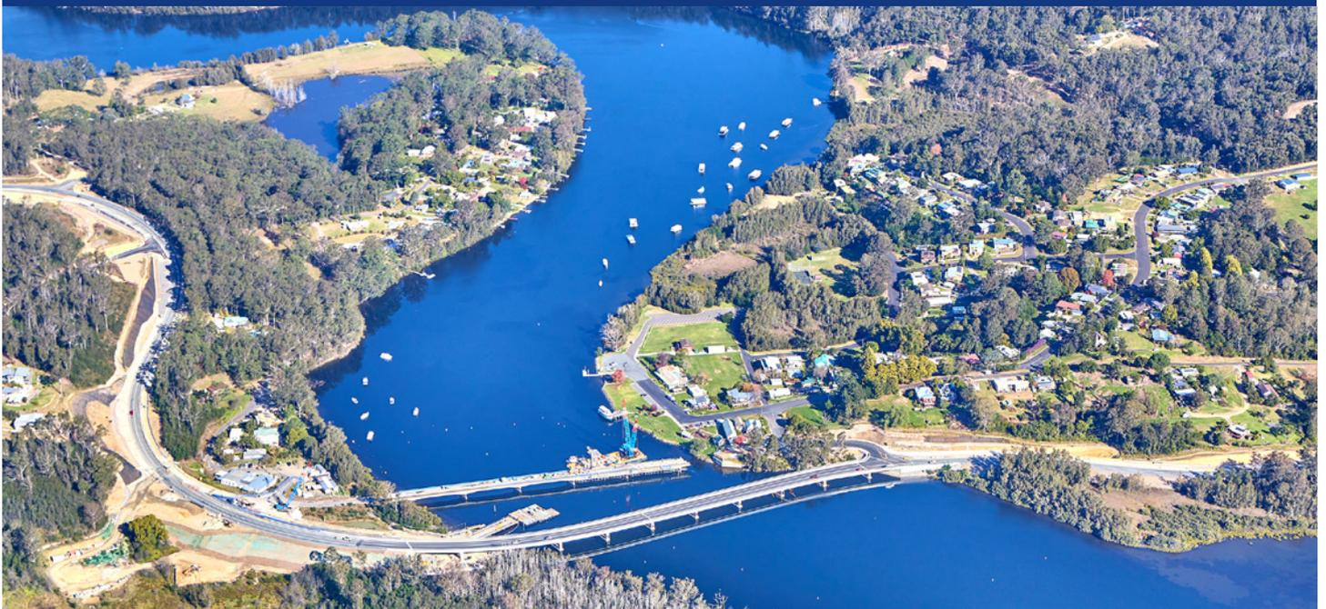
New Nelligen Bridge open to traffic and the old bridge being removed
