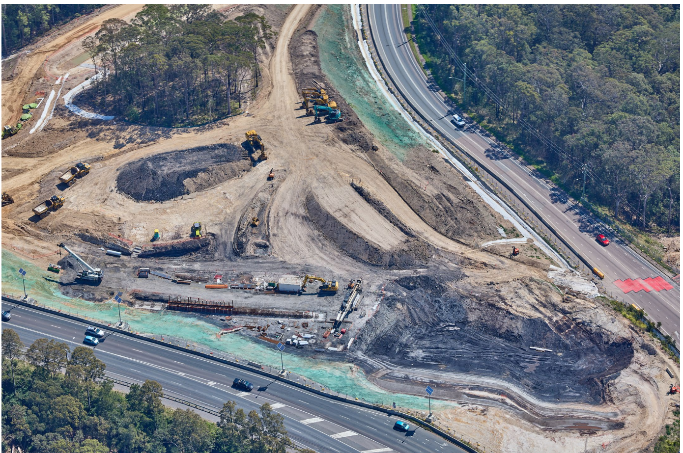
We use soil binders (coloured green) to minimise dust on stockpiles and exposed areas
