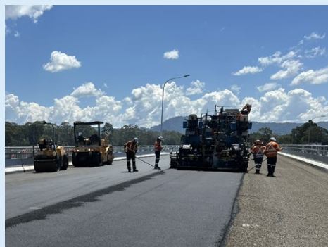
Left: Workers lay the first layer of asphalt on the bridge.
