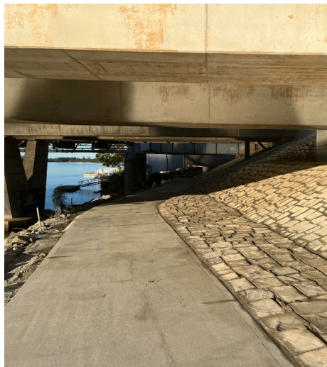
Stone pitching on the southern foreshore is complete and the underpass will open soon.
