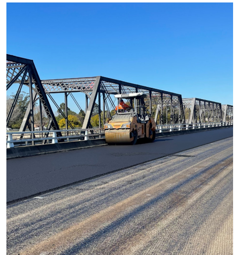
Applying the new asphalt surface on the middle bridge.
