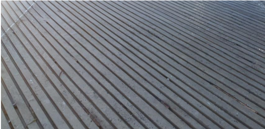
Figure 9: Moulded grooves in concrete
