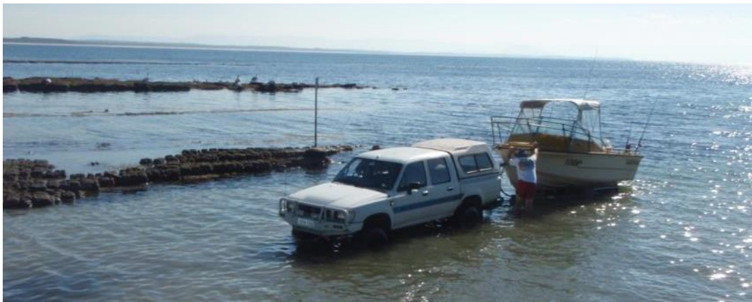
Figure 7: Boat launching on a ramp with insufficient slope with tow vehicle in the water
