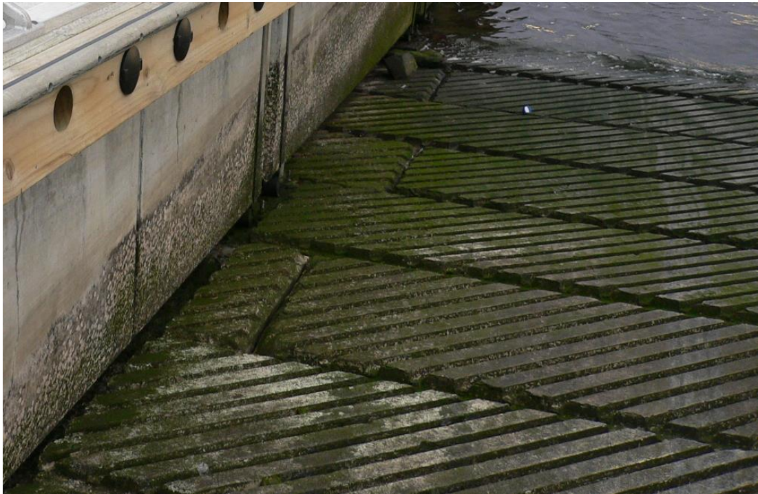
Figure 13: Marine growth on a boat ramp
