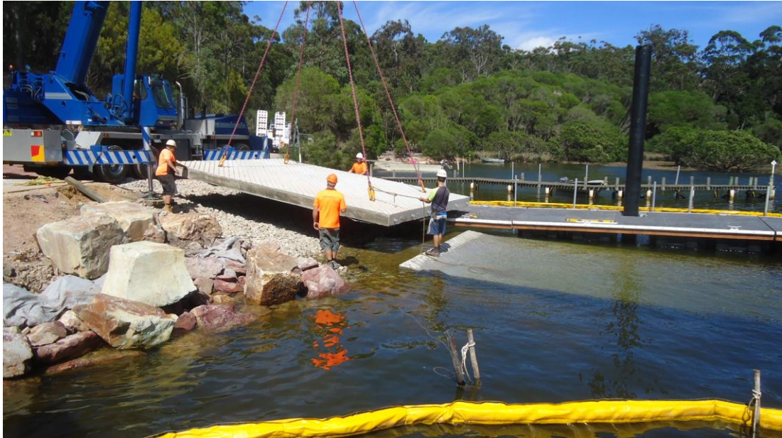
Figure 11: Installation of a large precast panel with a lifting crane
