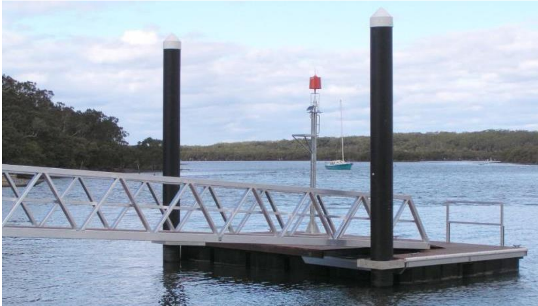
Figure 24: Gangway leading to rectangular pontoon
