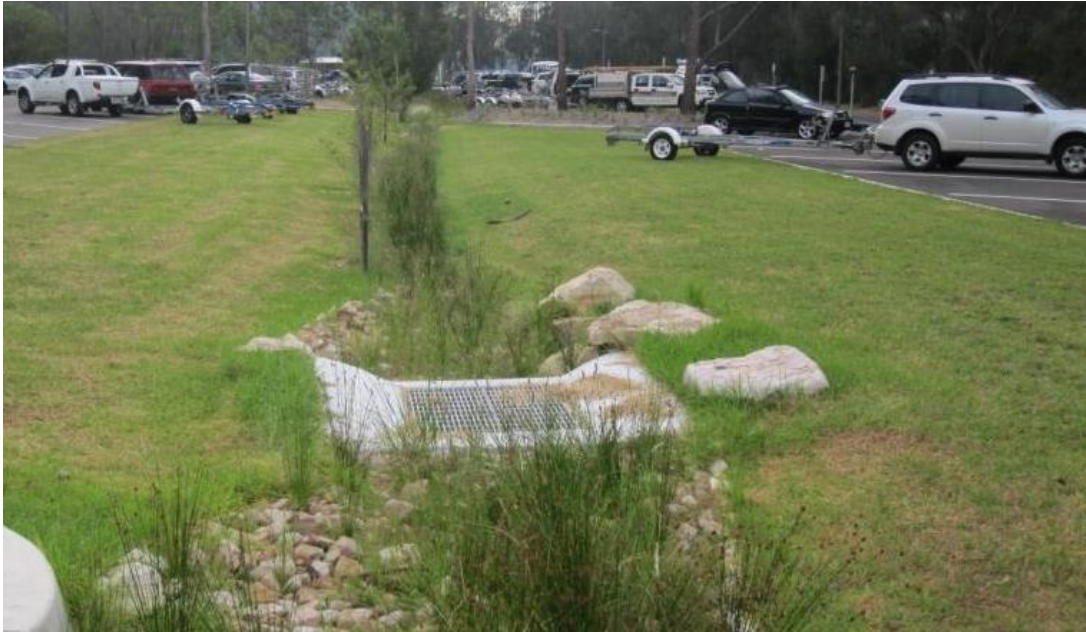
Figure 22: Vegetated swale in between car and trailer spaces
