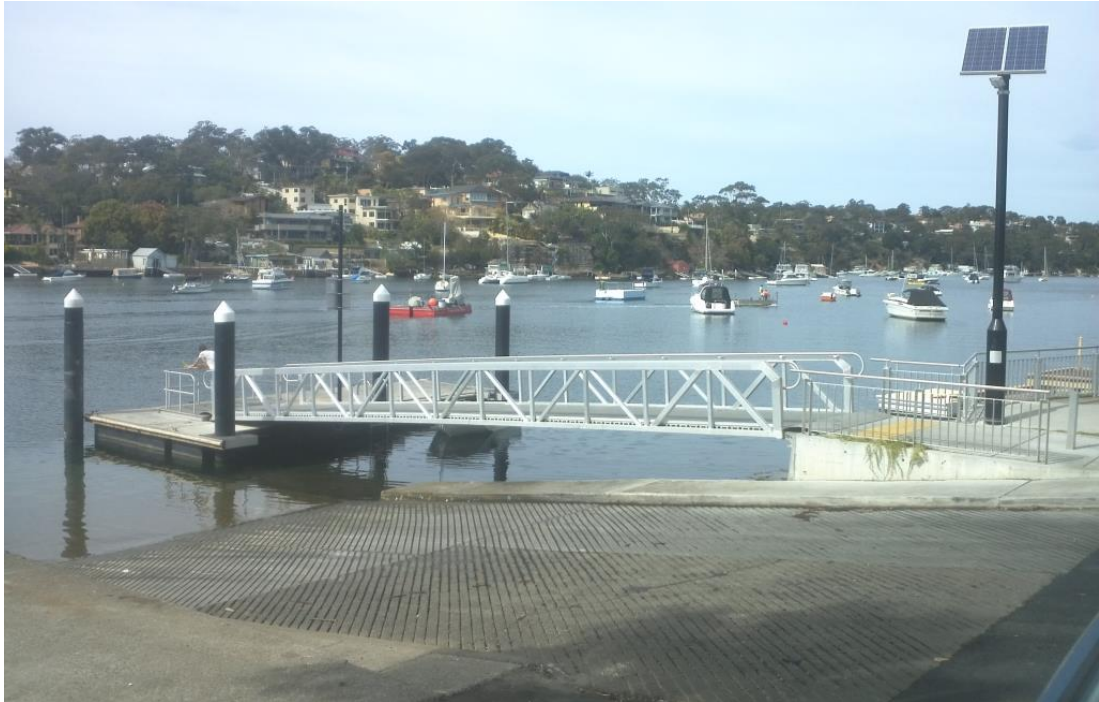
Figure 29: Aluminium gangway providing access from the foreshore
