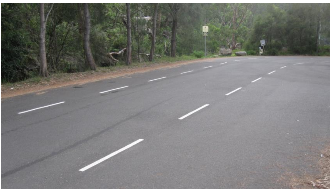
Figure 18: Rigging area provided along left hand side of ramp approach accessway
