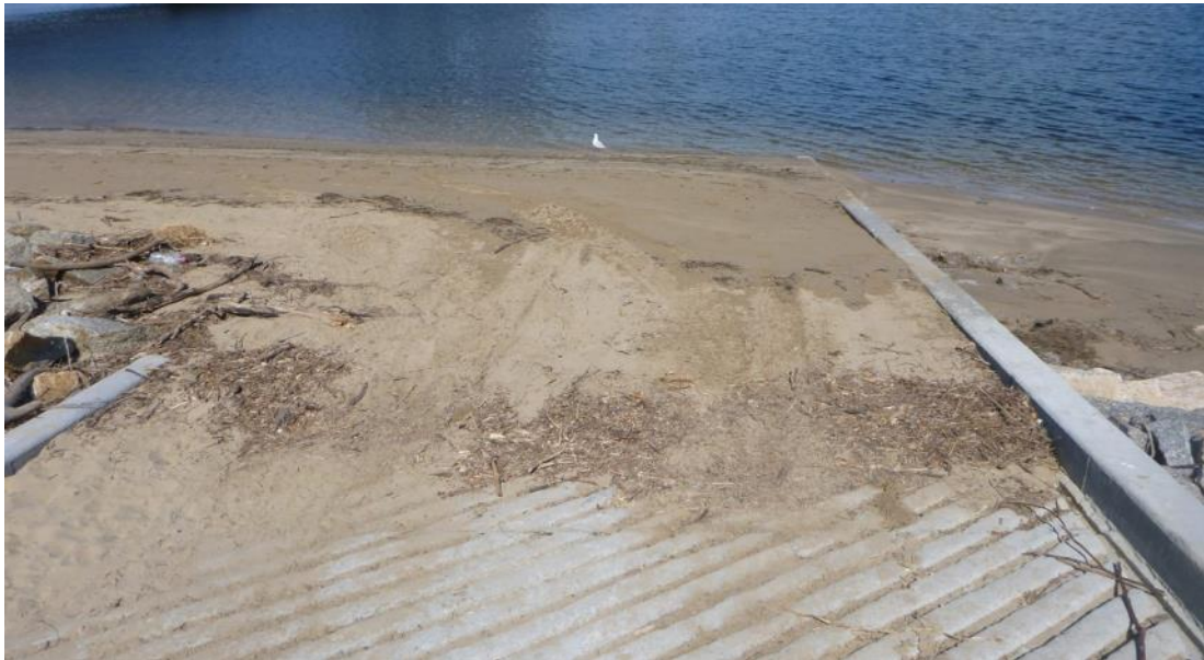
Figure 4: Boat ramp affected by sedimentation
