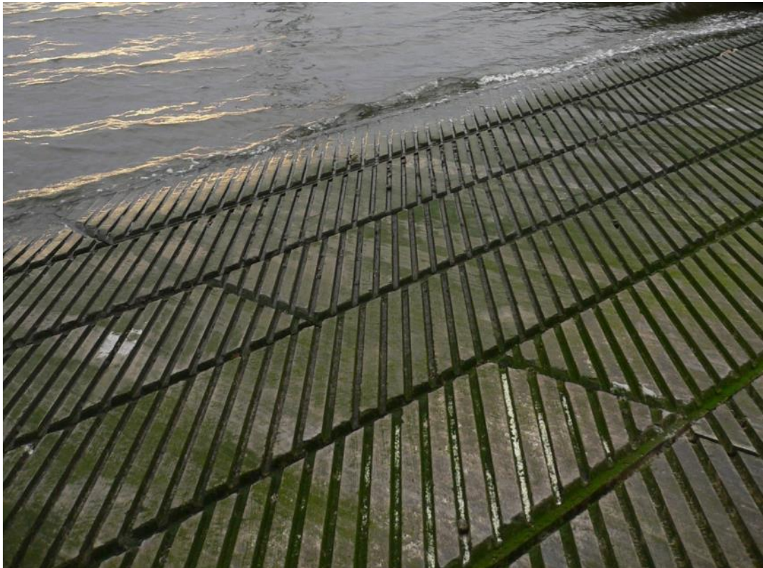
Figure 10: Precast planks installed below Mean Water Level
