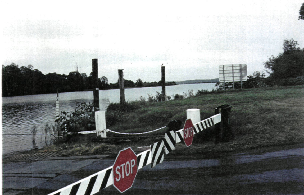
1998 - Bluff Point approach and ferry mooring piles
