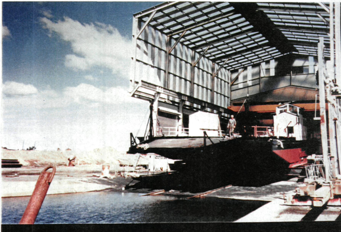
Settlement Point ferry on a local slipway after an overhaul, 1987
