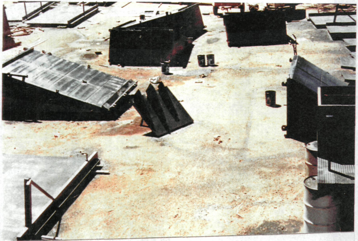
New Hibbard ferry pulled apart ready for sandblasting, 1984
