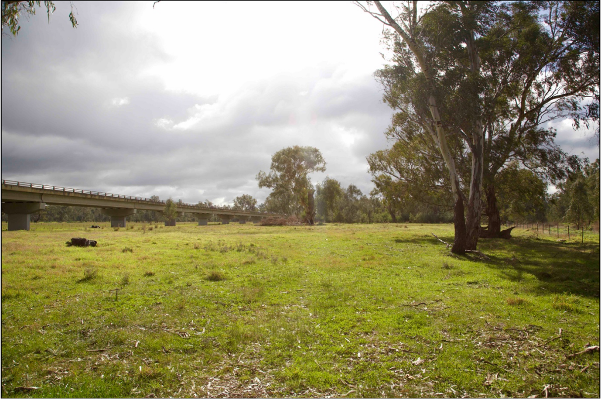
Image 10: Gobbagombalin Bridge. lxv
