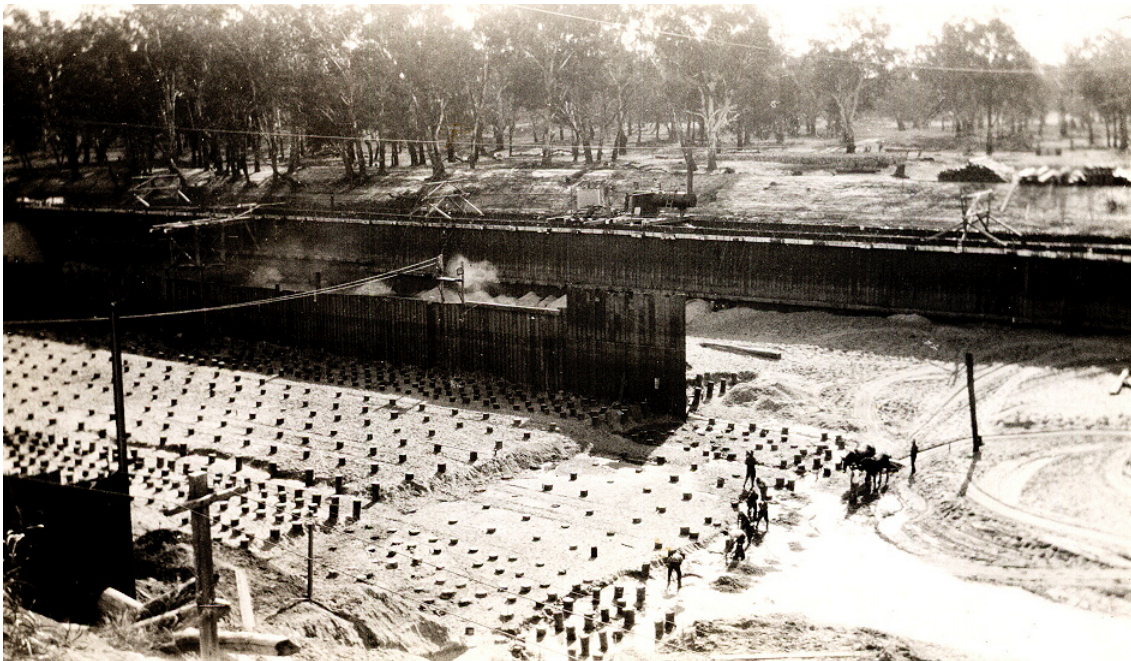
Cofferdam construction at the lock
