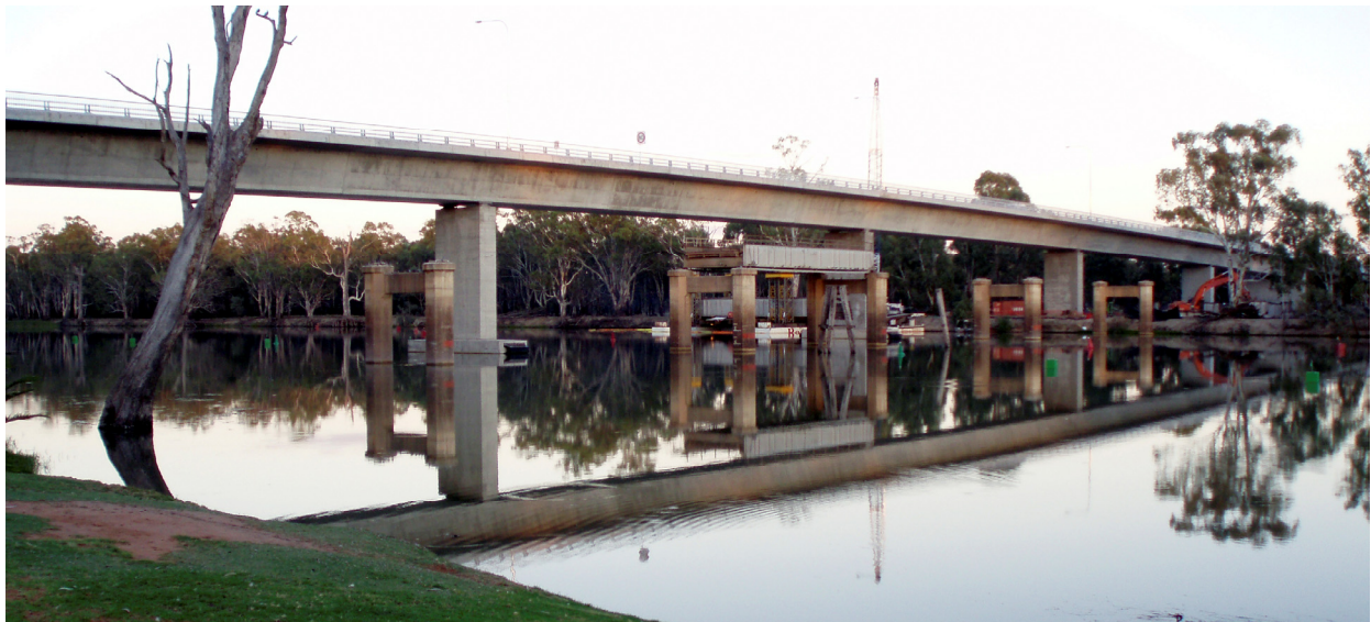
Partly dismantled old bridge in background
