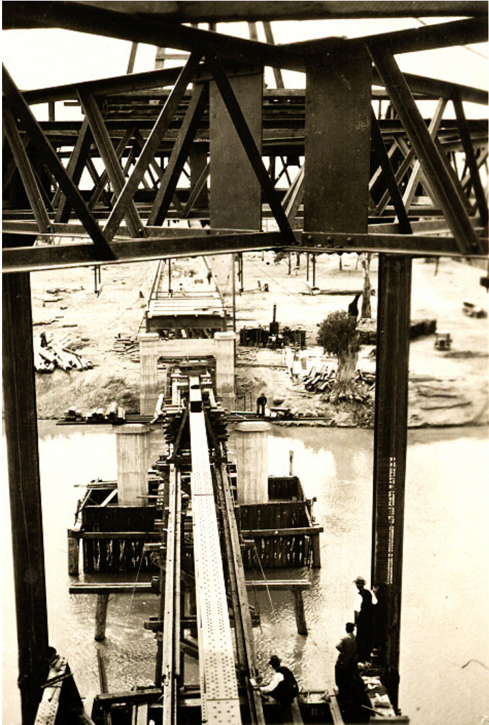
View of construction from lift span
