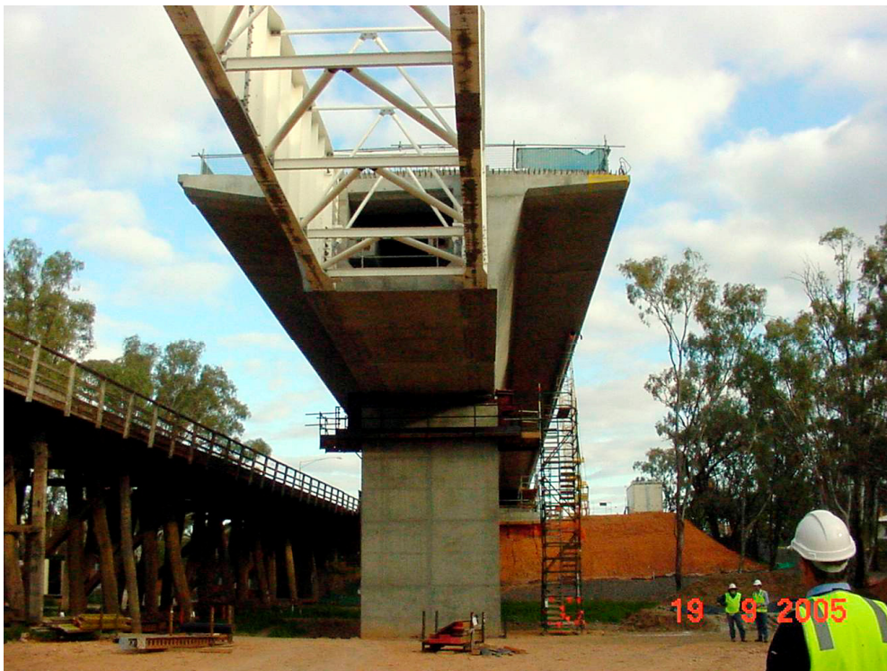
Box girder launched over pier
