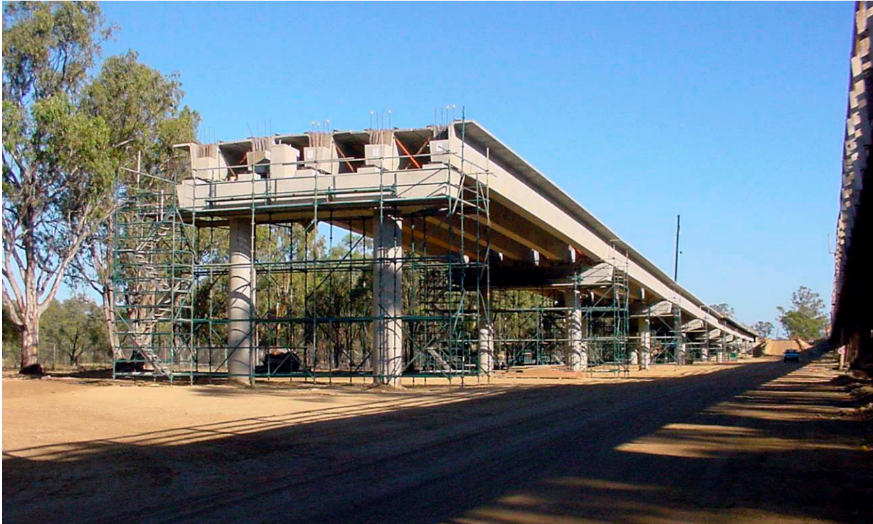
Girder installed to Pier 8
