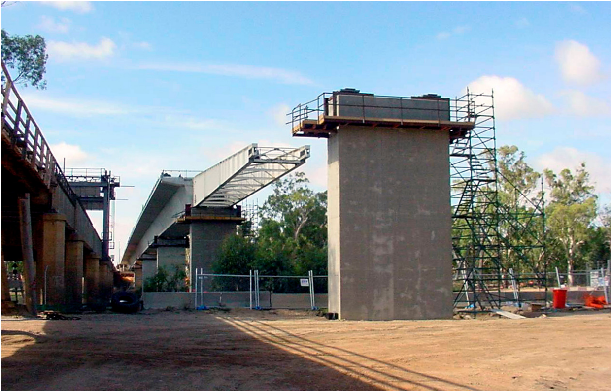
Box girder launched to Pier 4
