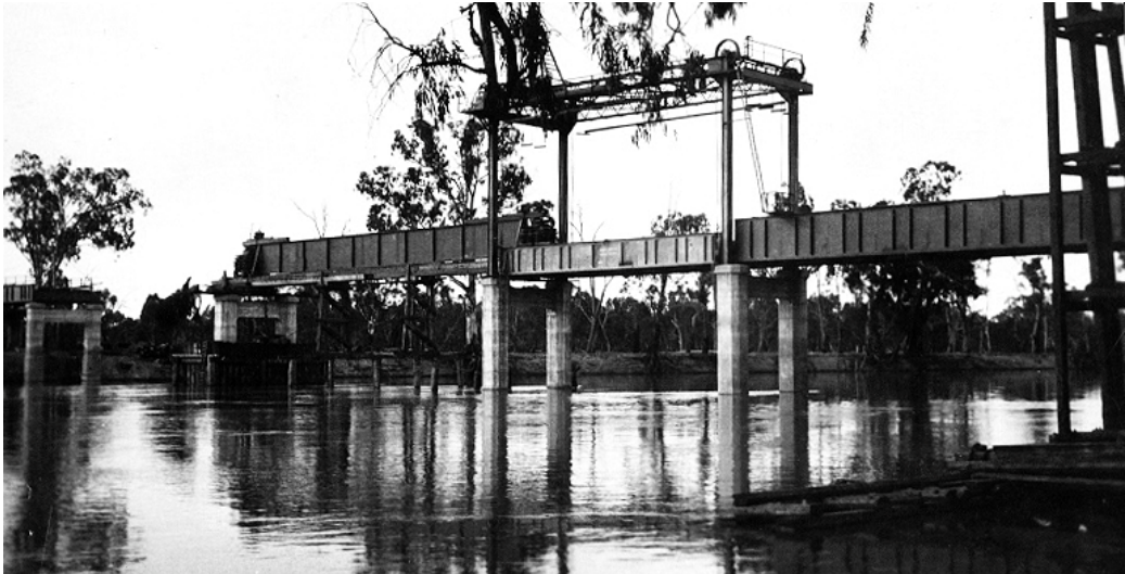
Bridge nearing completion, 1928
