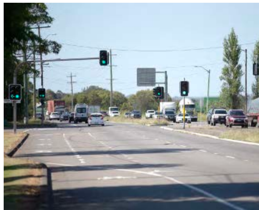
Maitland Road near Hexham Bowling Club
