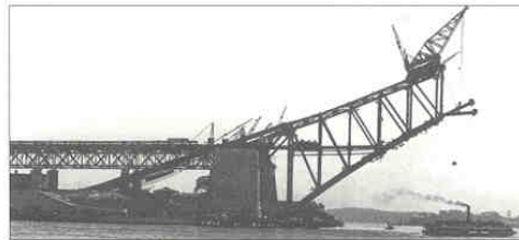
The Harbour Bridge being constructed, October 1929
