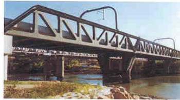
The Camellia Railway Bridge
