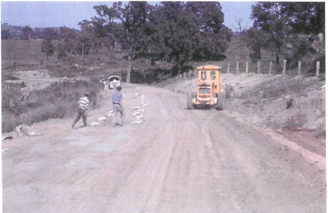
Two ways of adding cementitious binder
