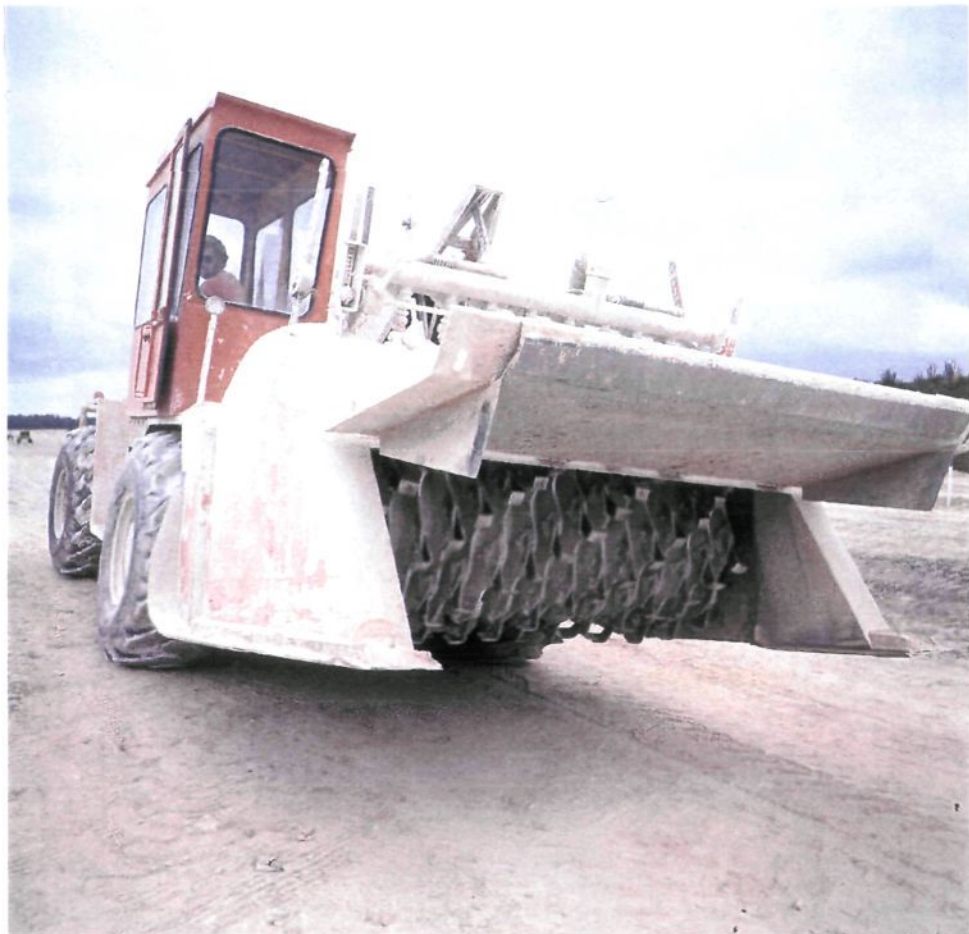
Pulvimixer at work on the South Western Freeway between Pheasants Nest and Avon Dam, 1979
