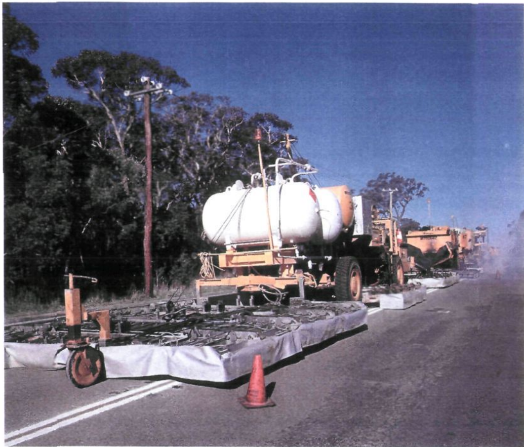
Hot in Place Asphalt Recycling – gas pavement heaters in use
