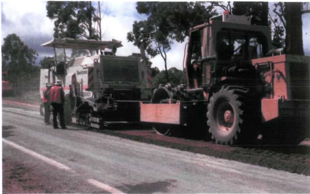
Wirtgen specialist mill & stabilise single pass machine in operation, followed by Vibromax 1801 compaction plant
