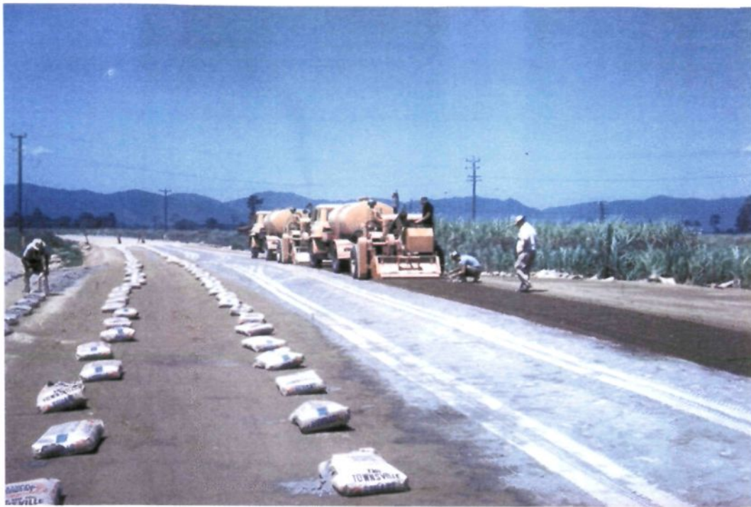
Spreading cement using bags, 1970s
