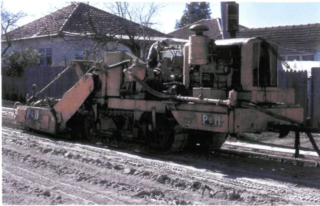
P&H stabiliser at work on a typical Bankstown street, 1970s
