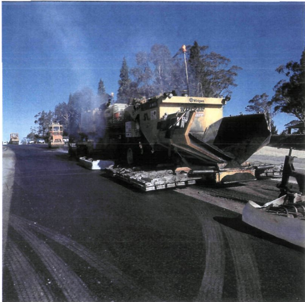
Hot in Place Asphalt Recycling
