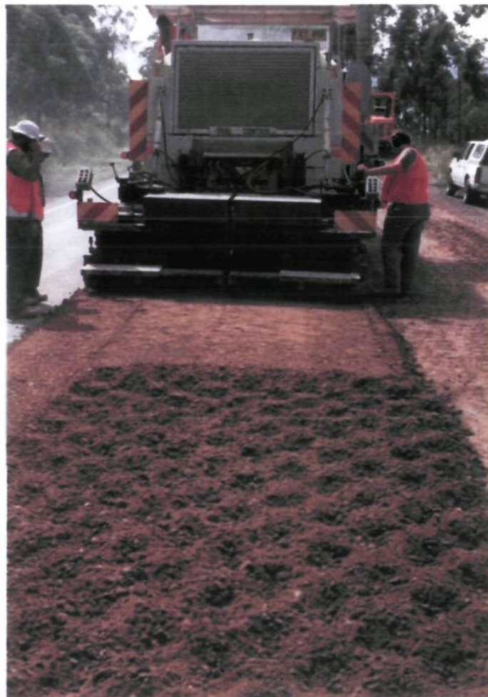
Wirtgen specialist mill & stabilise single pass machine in operation, followed by Vibromax 1801 compaction plant
