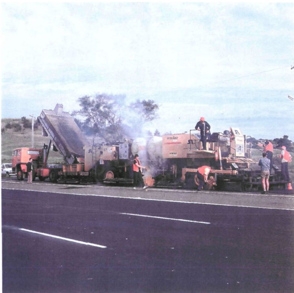
Hot in Place Asphalt Recycling
