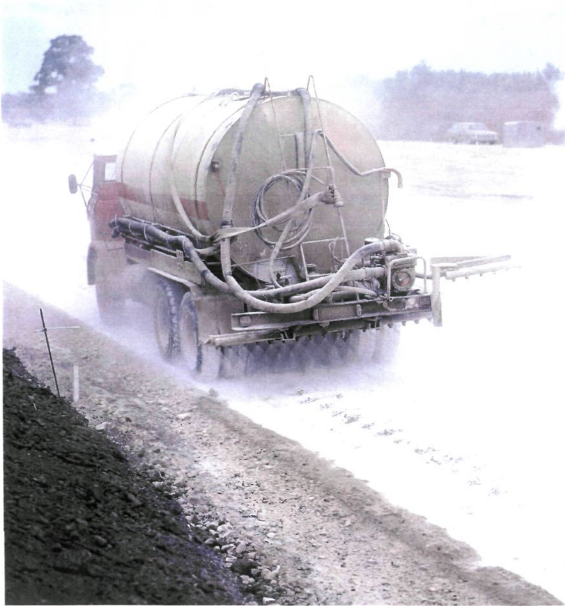
Slaking quick lime on the South Western Freeway between Pheasants Nest and Avon Dam, 1979
