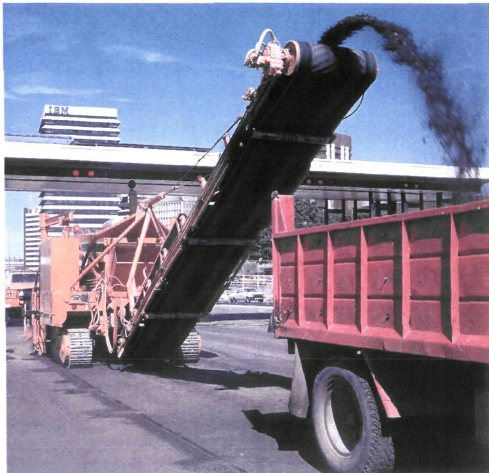
Pavement Profiler at work on the Sydney Harbour Bridge, 1978
