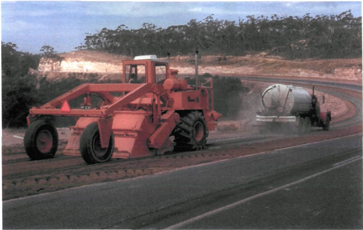
Stabilisation on the Hume Freeway in the 1980s
