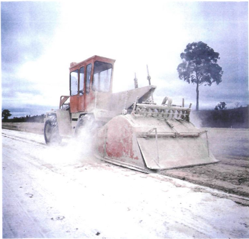
Pulvimixer at work on the South Western Freeway between Pheasants Nest and Avon Dam, 1979
